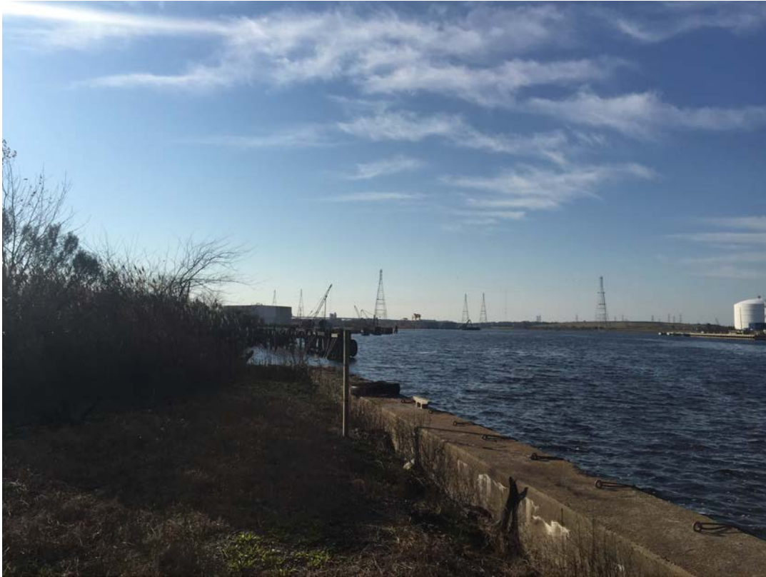
Waterbody data point schp001 facing west upstream.
