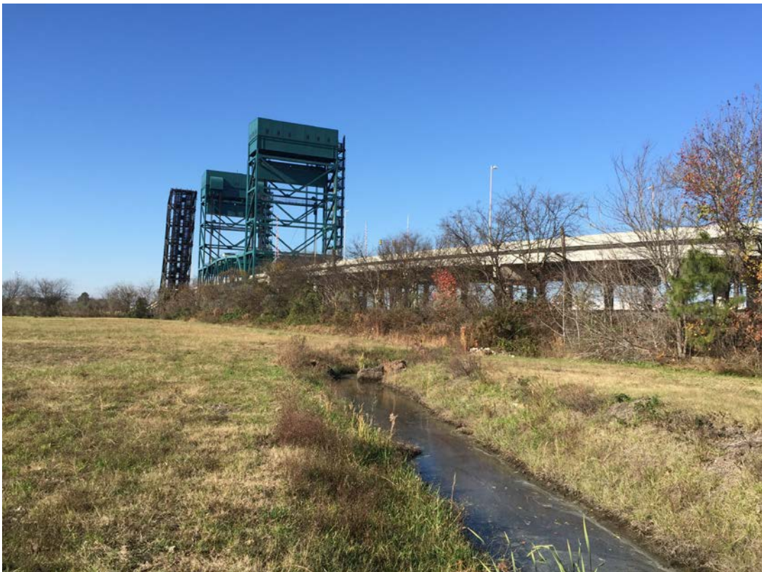
Waterbody data point schp004 facing west downstream.
