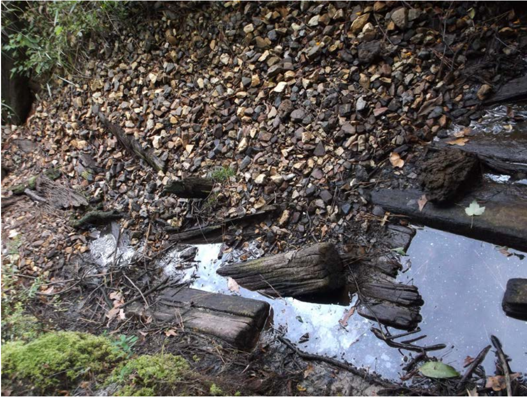
Waterbody scho003 facing north across bank.
