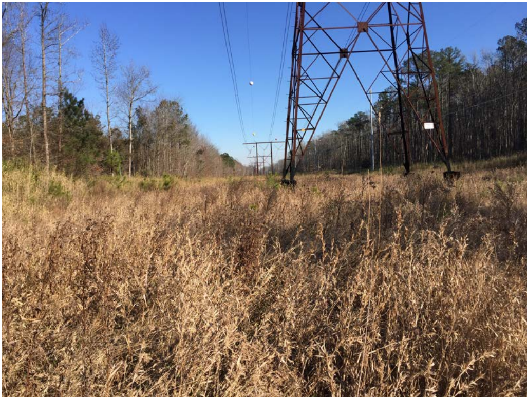
Wetland data point wchr002e_w3 facing southeast
