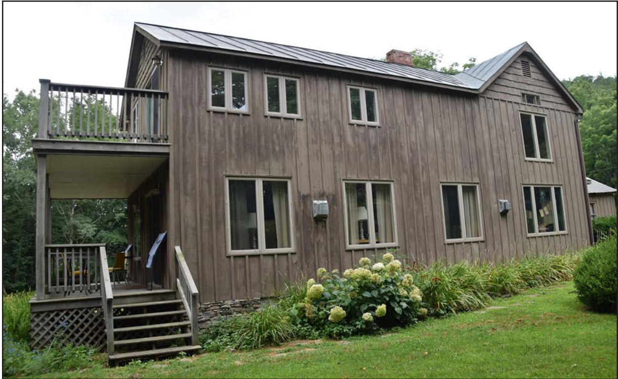
Figure 225. 045-0007, view of additions, view south.
