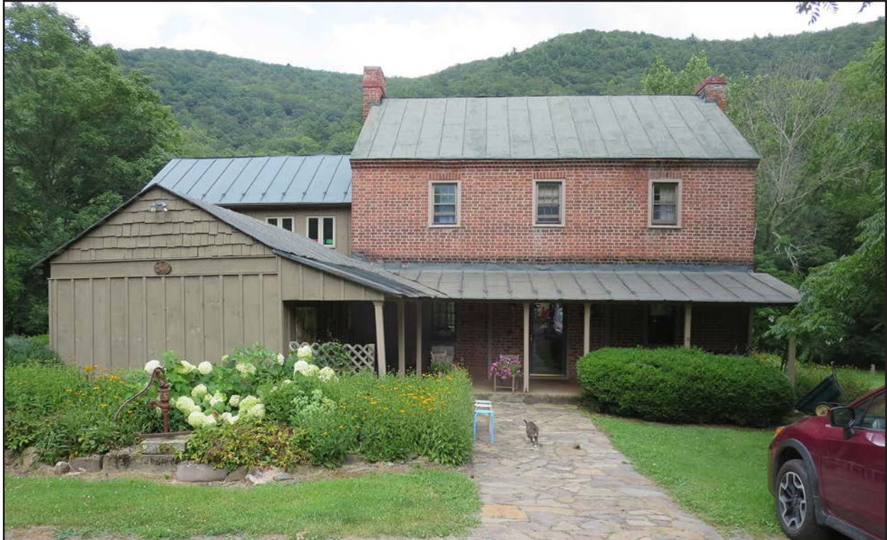
Figure 224. 045-0007, view of west elevation, view east.
