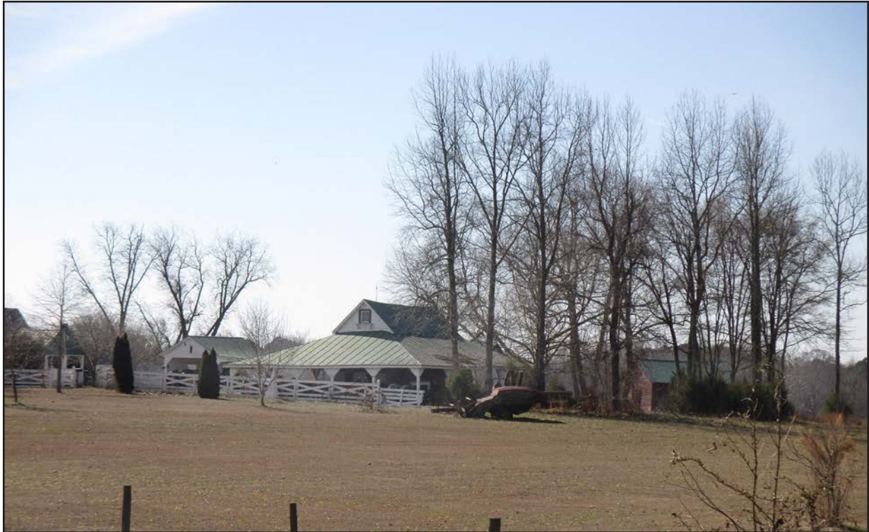
Figure 329. 087-5505, outbuilding, view southwest.
