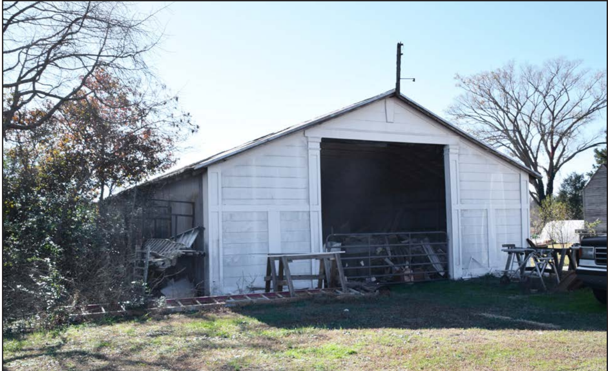
Figure 363. 133-0101, barn, view southwest.
