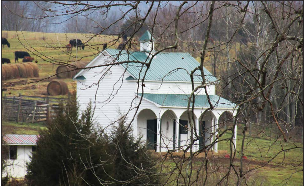
Figure 269. 062-5121, stable, view north.
