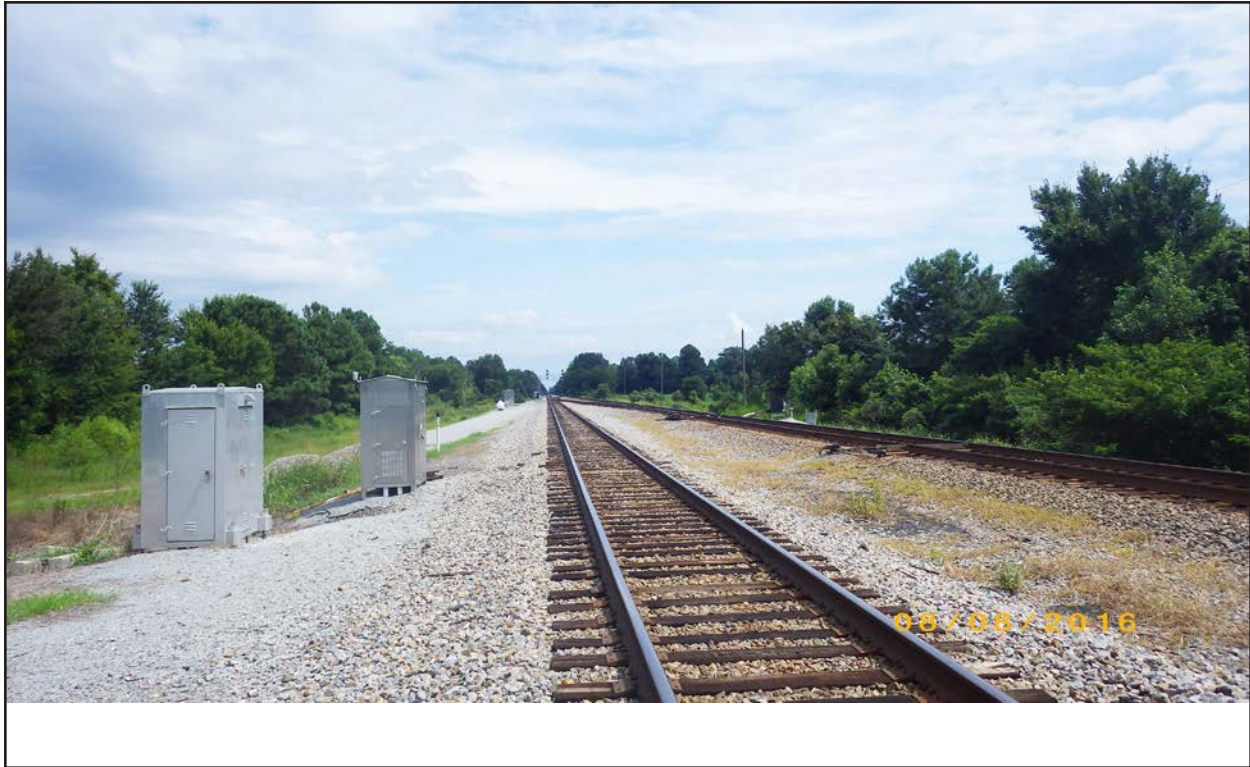
Figure 351. 091-5098, toward Project, view southeast
