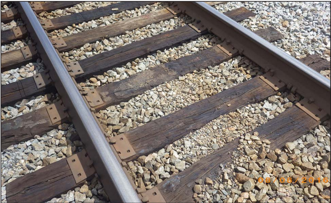
Figure 347. 091-5098, close up of rails, view southeast.
