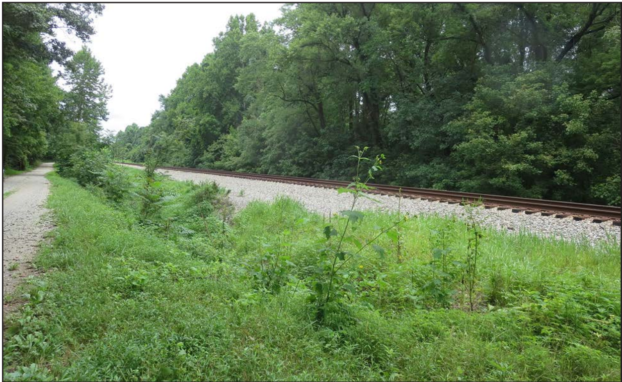
Figure 297. 062-5180, Chesapeake & Ohio Railroad from Midway Mills Lane, view north-northeast.
