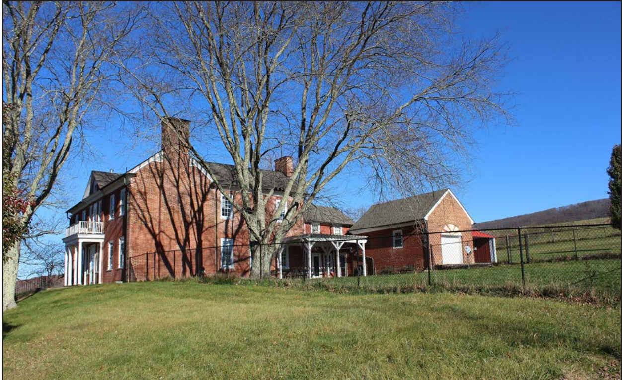
Figure 142. 008-0011, carriage house, view east.
