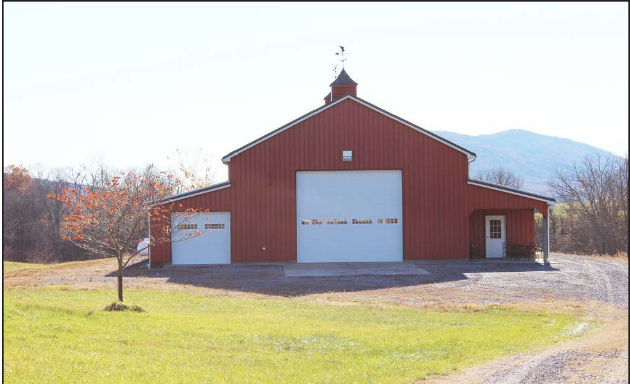
Figure 144. 008-0011, modern barn, view southwest.
