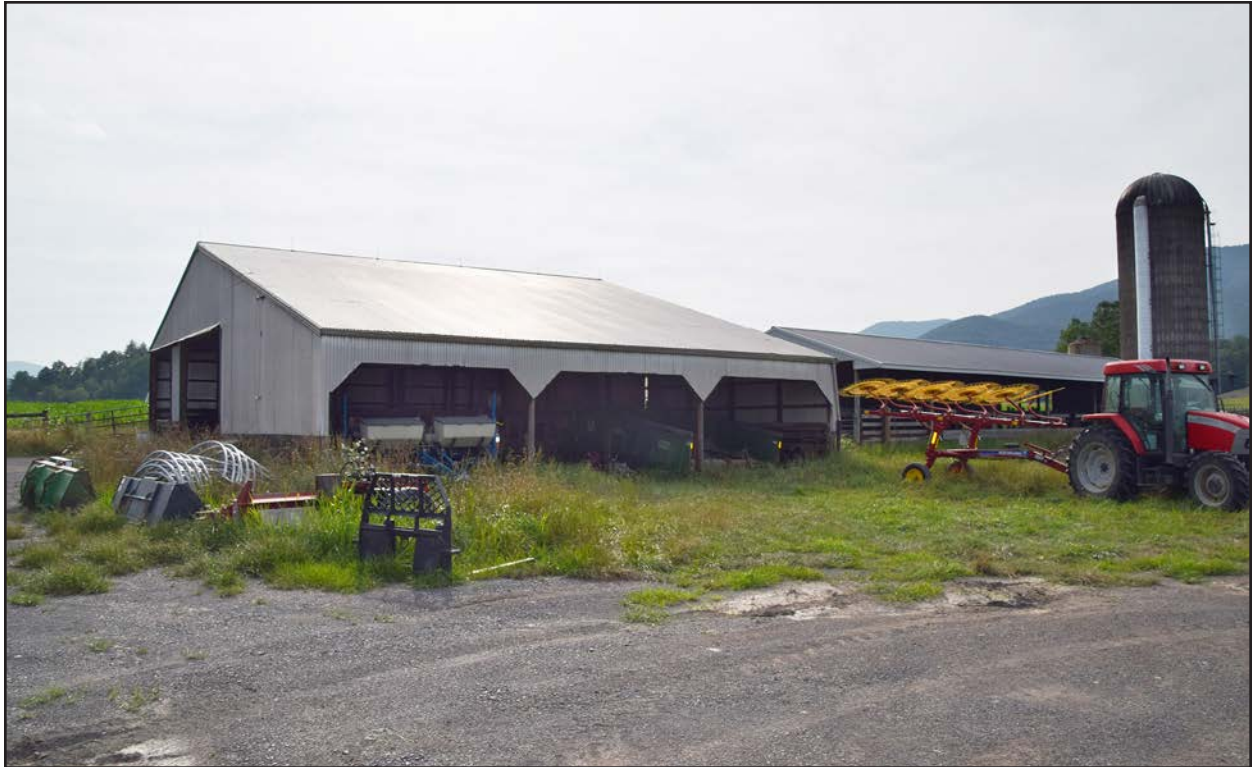
Figure 22. 007-0103, barn, view northwest.
