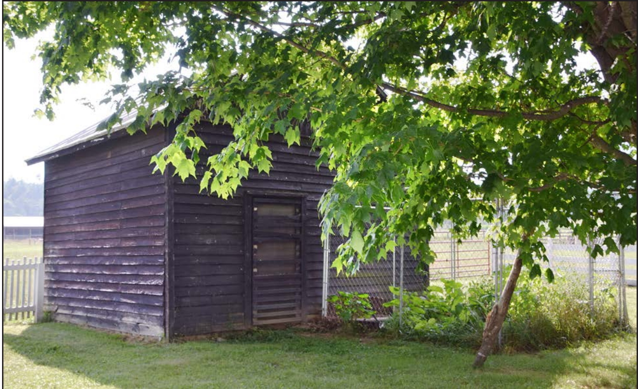
Figure 15. 007-0103, shed, view northwest.
