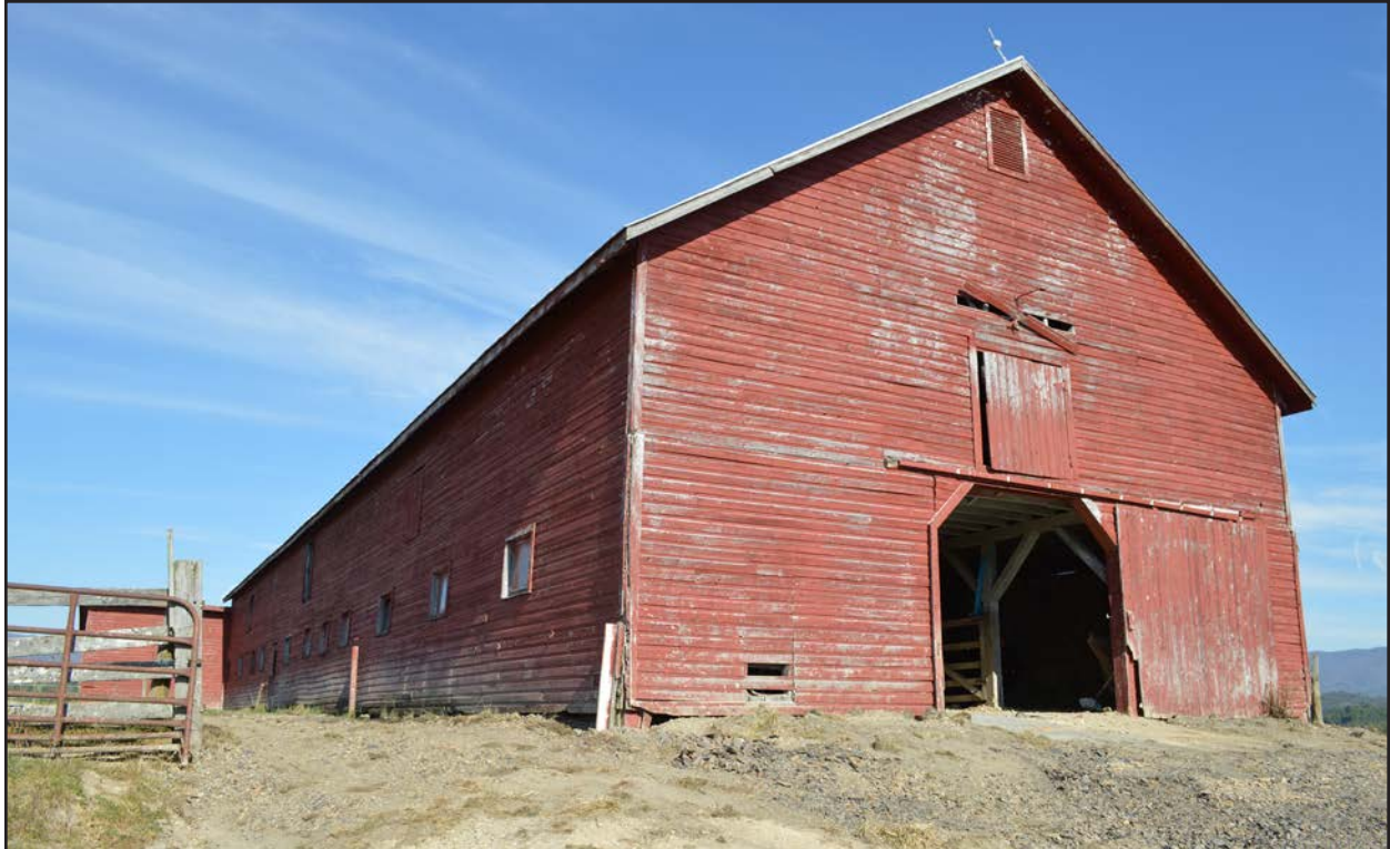
Figure 52. 007-0463, barn 2, view northeast.
