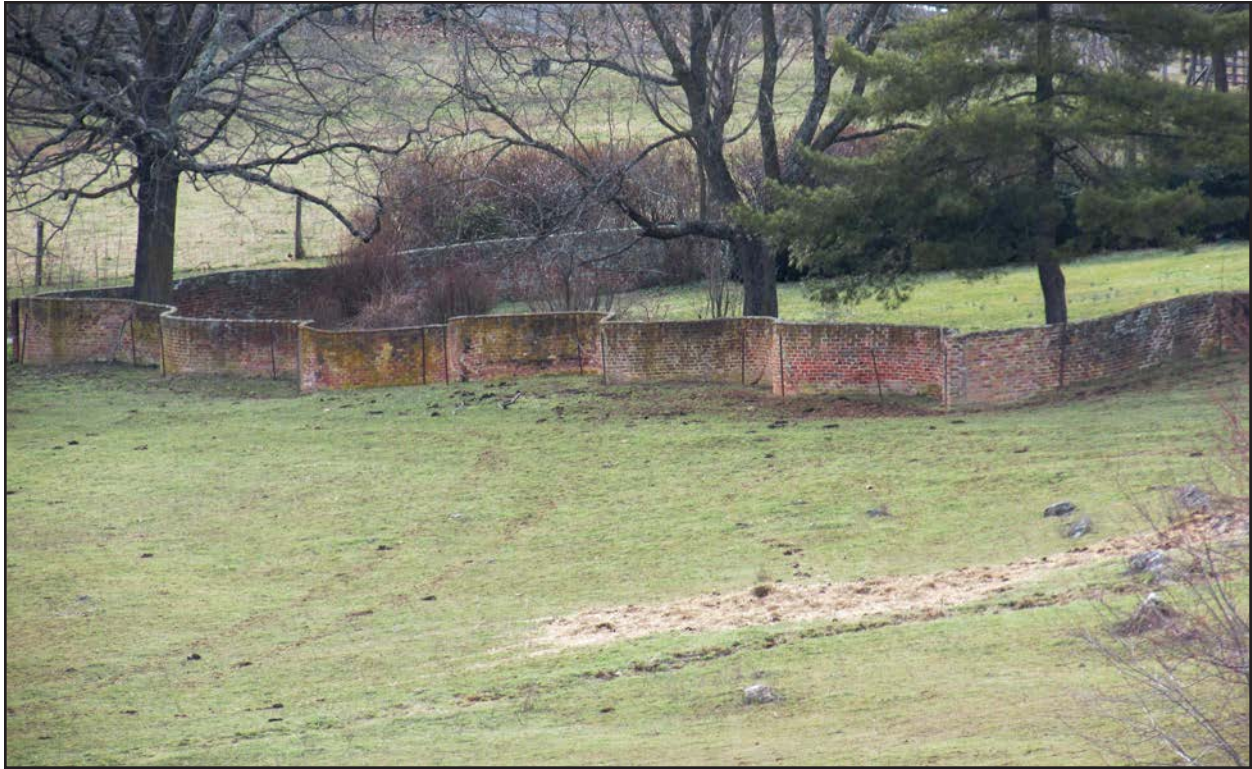
Figure 4. 007-0015, Serpentine Wall, view northeast.
