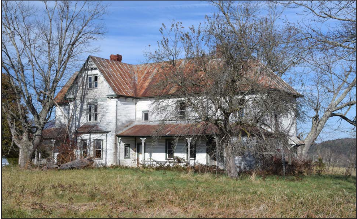
Figure 71. 007-0487, house, view east
