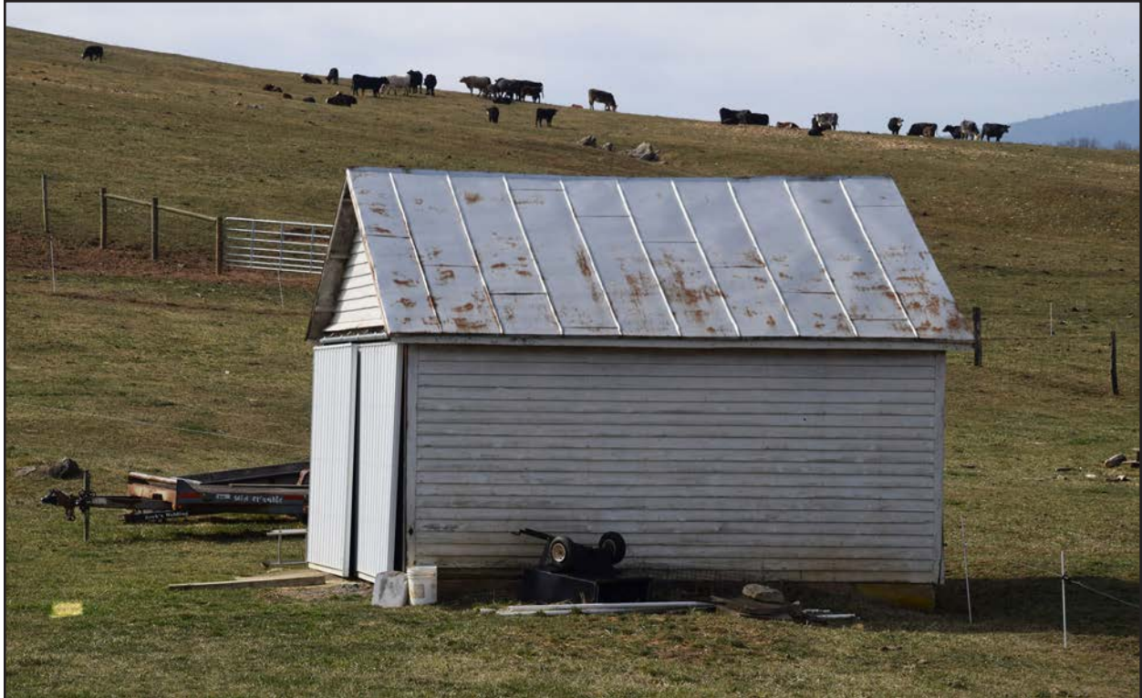
Figure 30. 007-0272, garage, view northwest.
