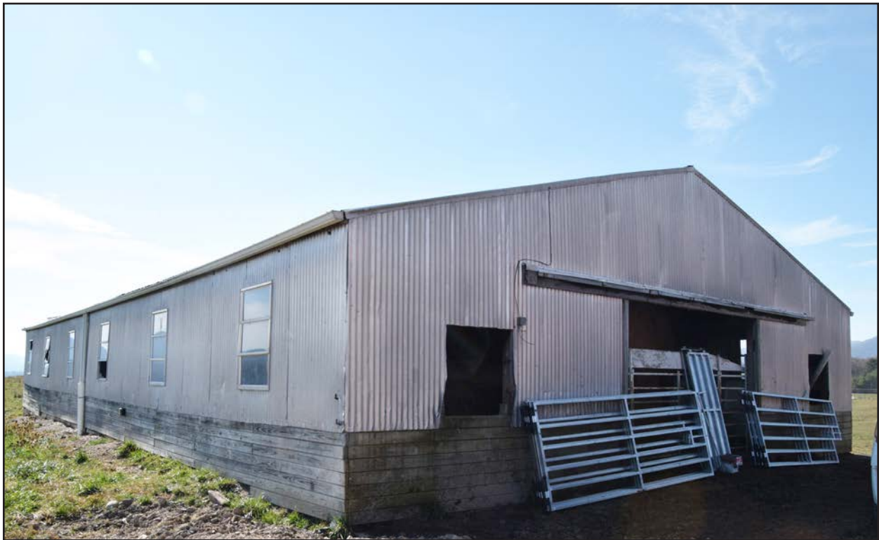
Figure 53. 007-0463, barn 3, view southeast.
