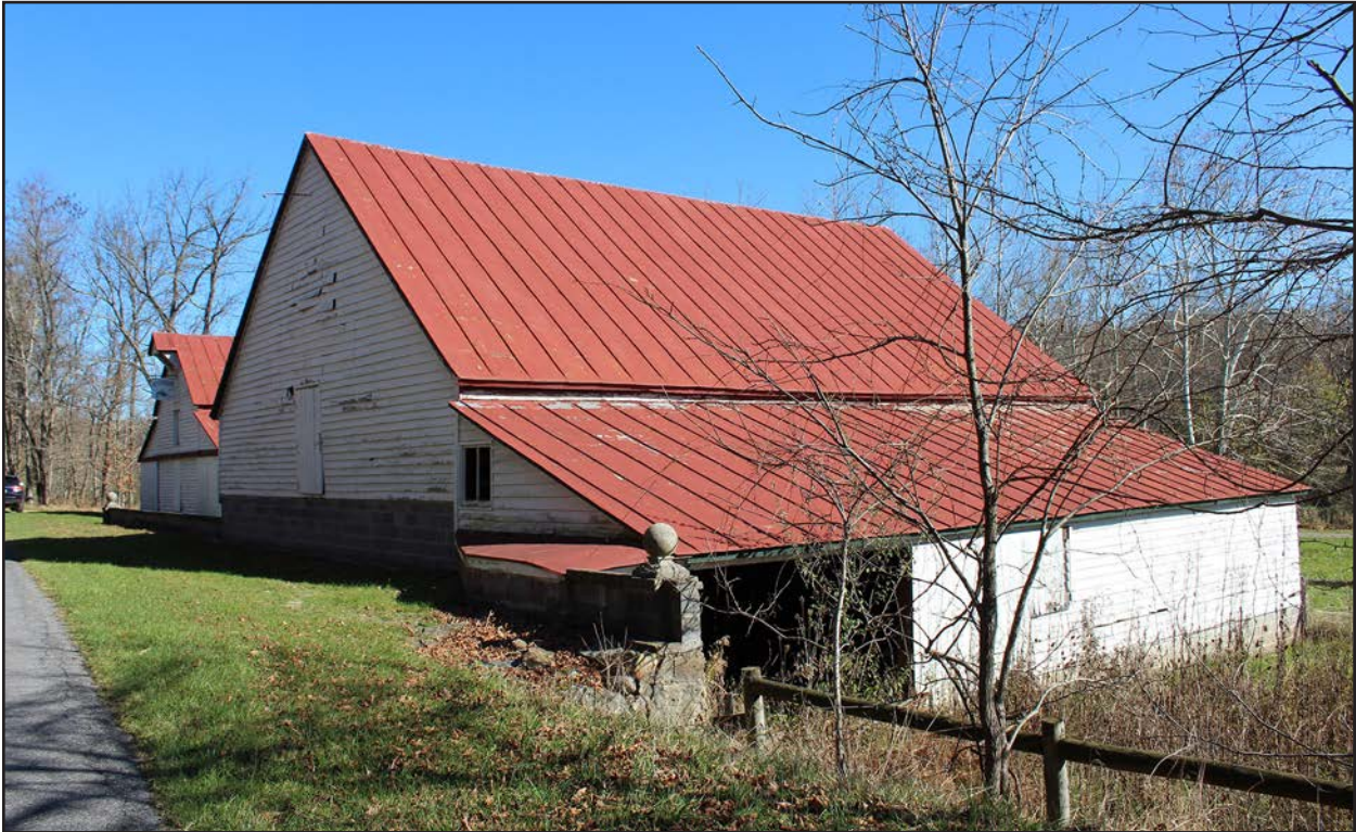
Figure 155. 008-0126, barn, view northeast.
