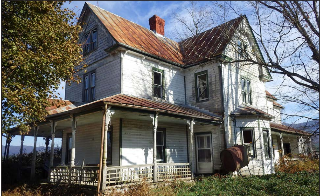
Figure 70. 007-0487, house, view north.
