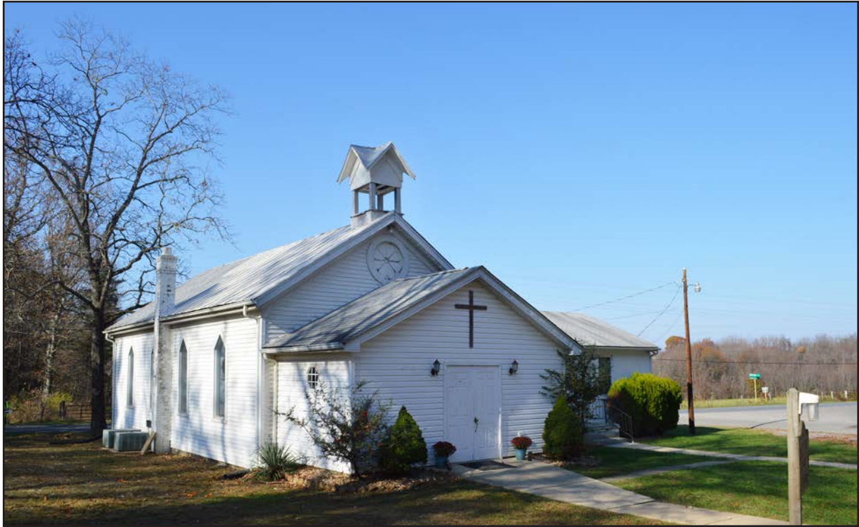
Figure 79. 007-0863, church, view southwest.
