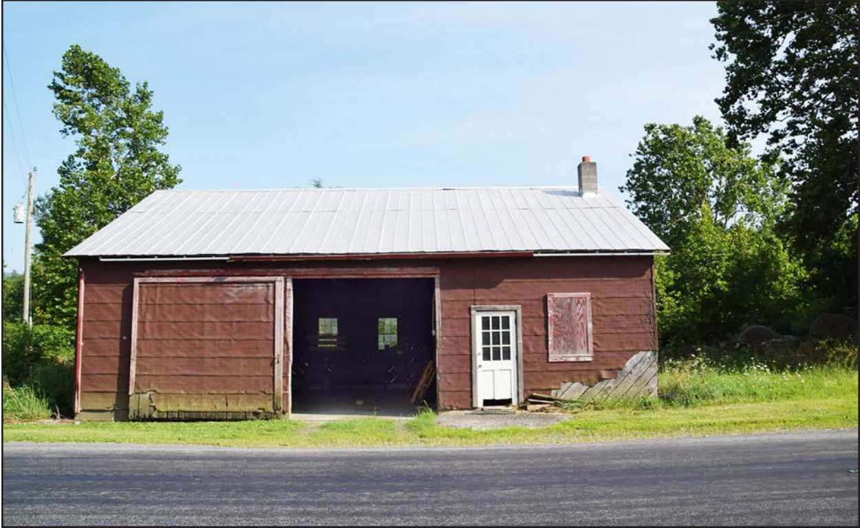
Figure 18. 007-0103, workshop, view south.
