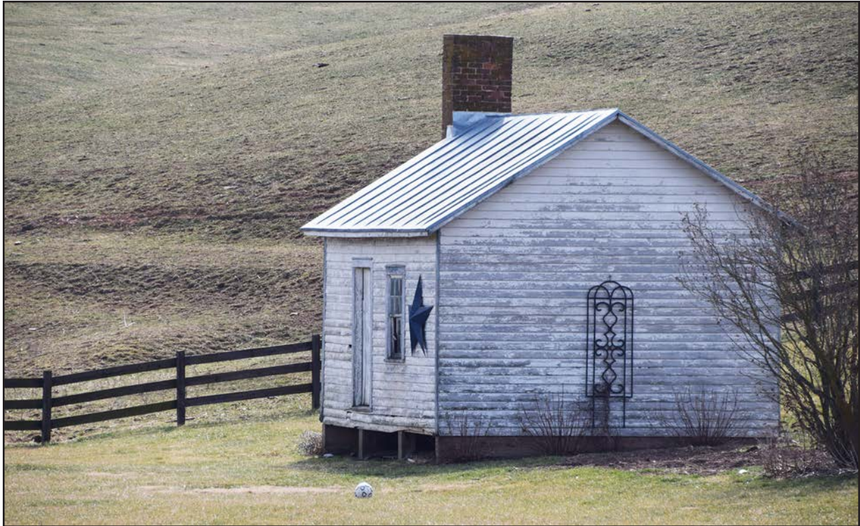
Figure 29. 007-0272, wash house, view southwest.
