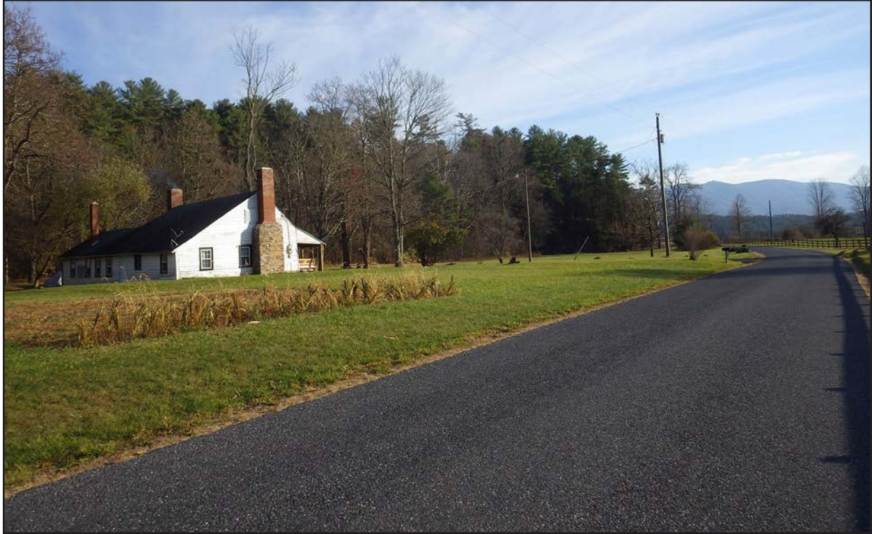
Figure 49. 007-0447, toward Project, view southeast.
