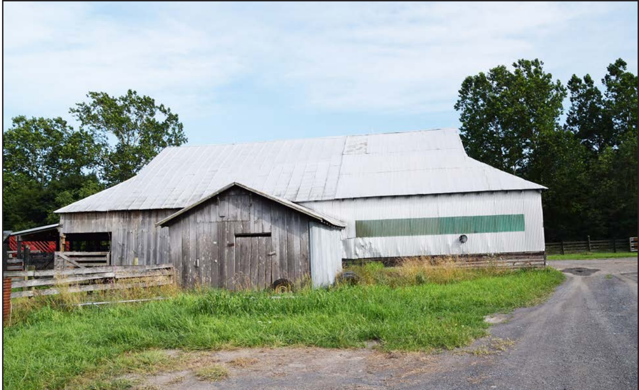
Figure 21. 007-0103, barn, view south.
