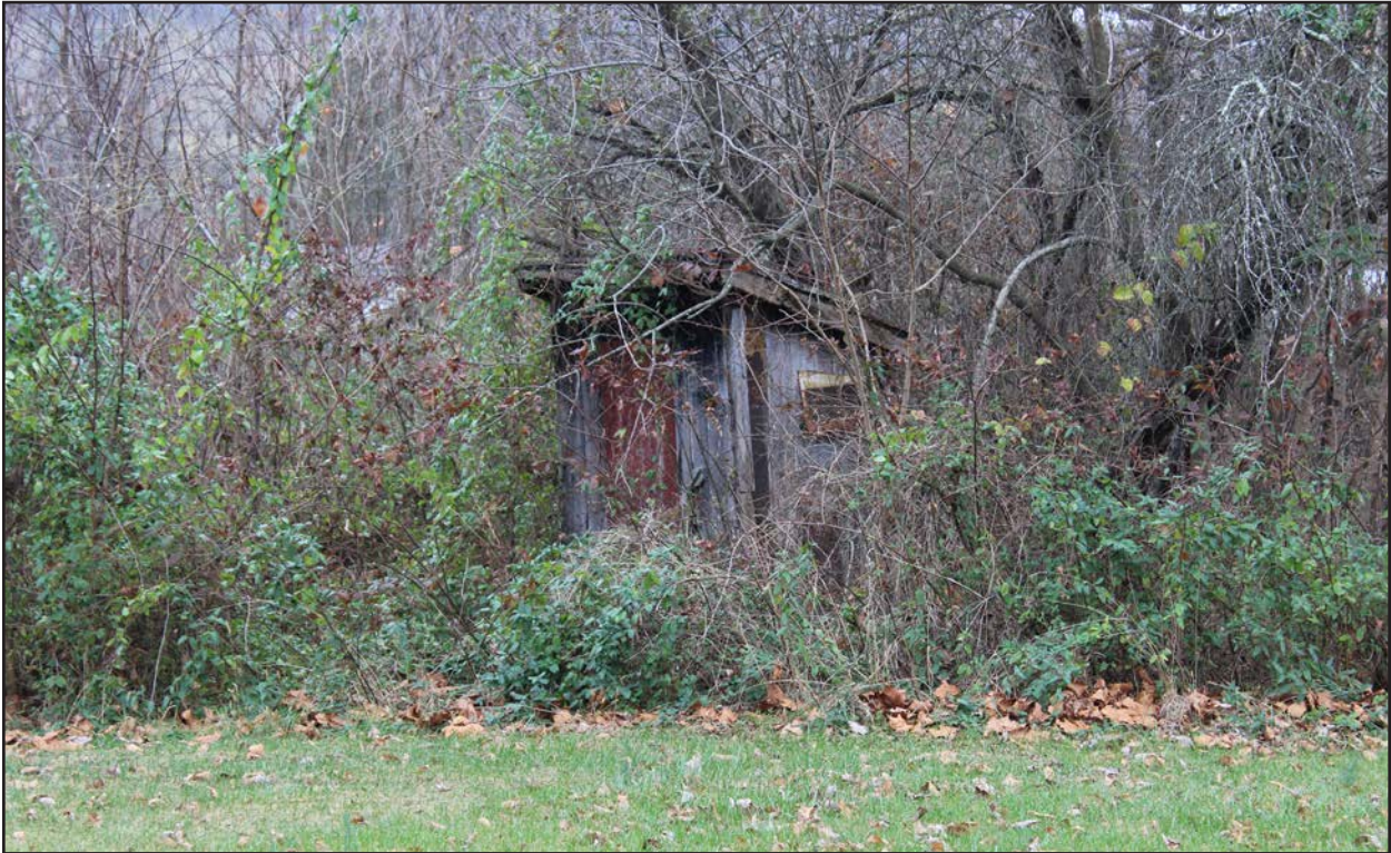
Figure 65. 007-0476, outhouse, view southwest.
