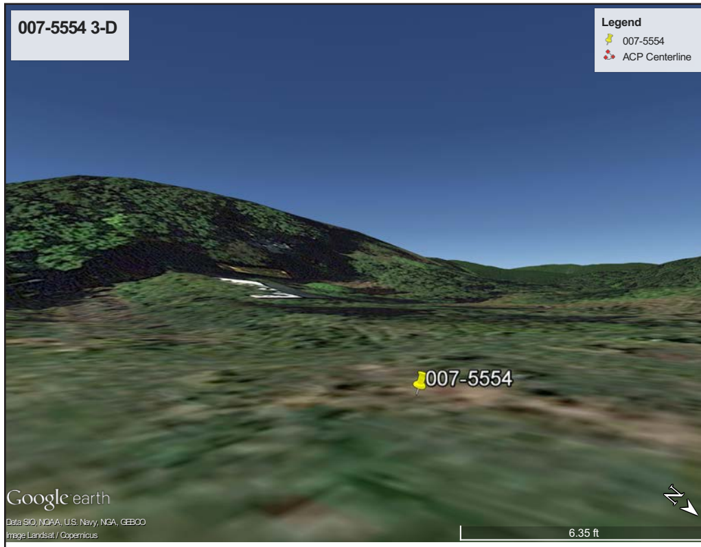
Figure 106. 007-5554, 3-D view toward Project.
