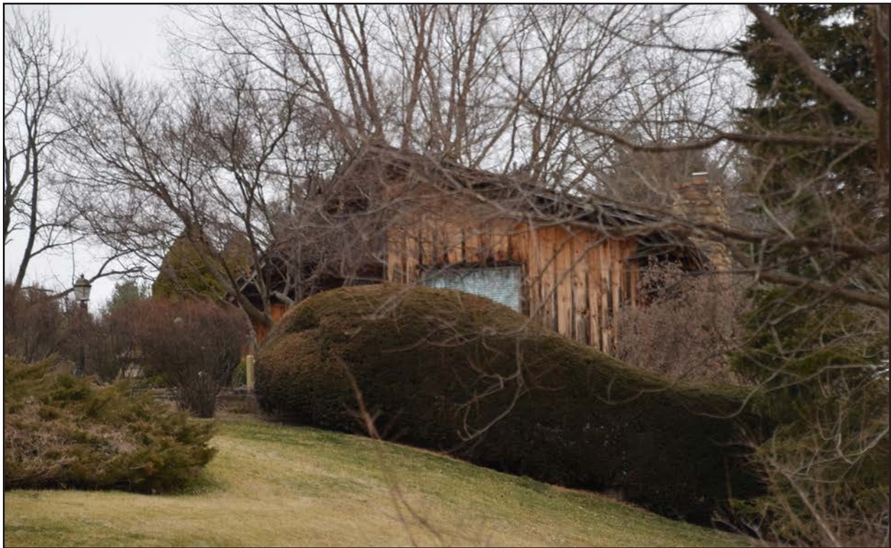
Figure 37. 007-0442, secondary dwelling, view north.
