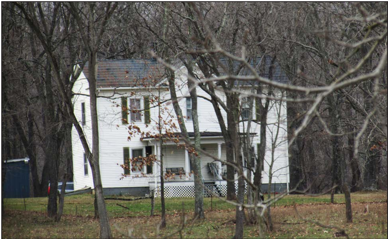
Figure 6. 007-0015, Secondary Dwelling, view north.
