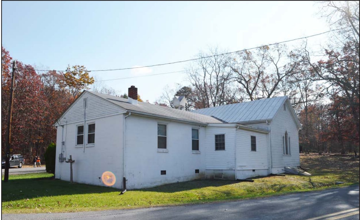
Figure 78. 007-0863, church, view southeast.
