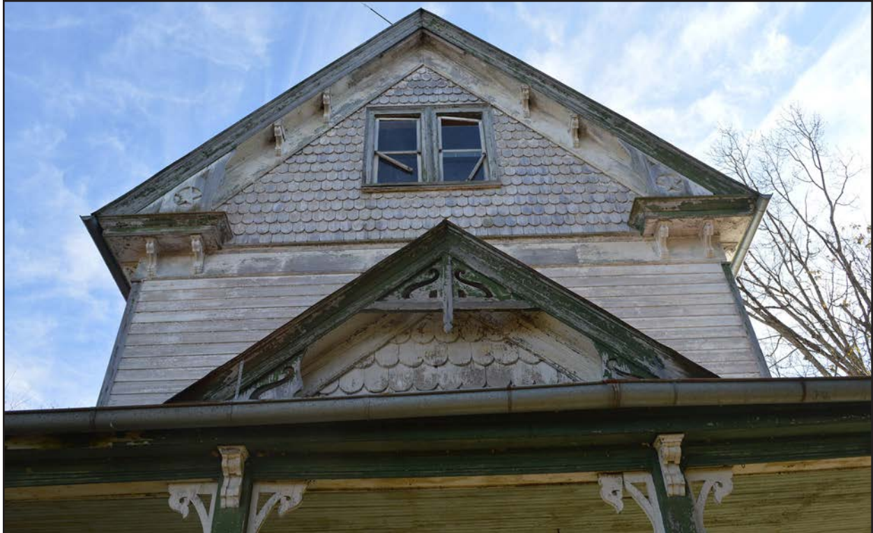
Figure 72. 007-0487, gable details on house, view southeast.
