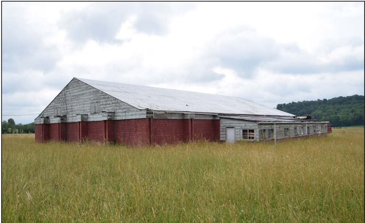
Figure 82. UP-0830, masonry hangar, facing southeast.
