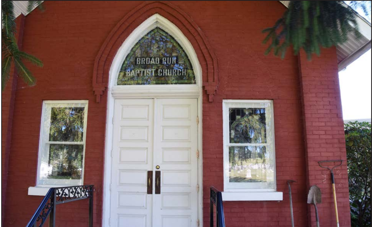
Figure 4. LE-0004, view of east façade of church, facing west.
