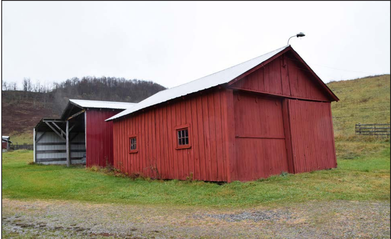
Figure 67. PH-0903, Barn 1 and Shed 5, facing northwest.
