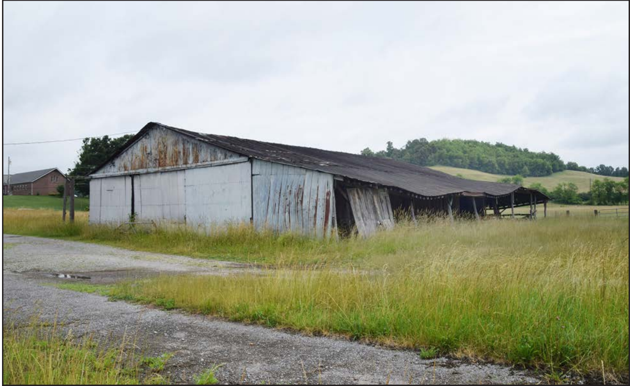
Figure 83. UP-0830, machine shop, facing northeast.
