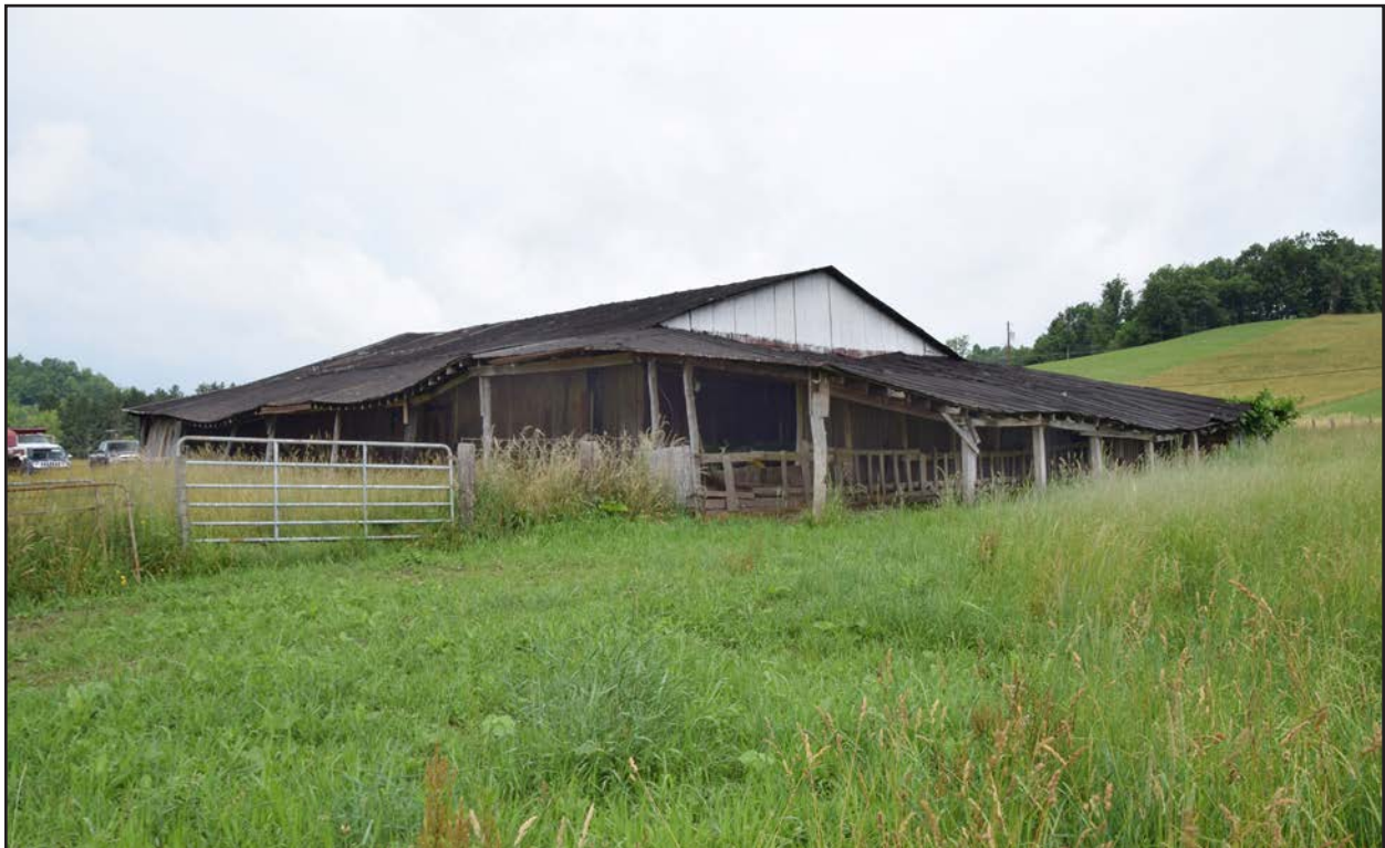
Figure 84. UP-0830, machine shop, facing northwest.
