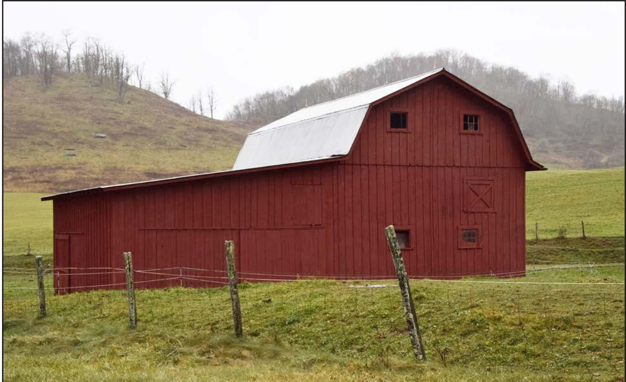
Figure 69. PH-0903, Barn 3, facing southwest.
