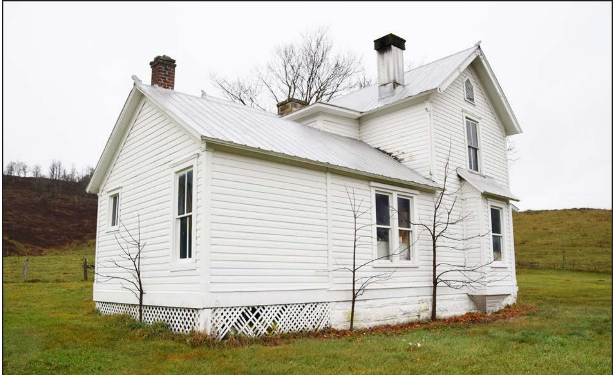
Figure 63. PH-0903, ca. 1890 house, facing north.
