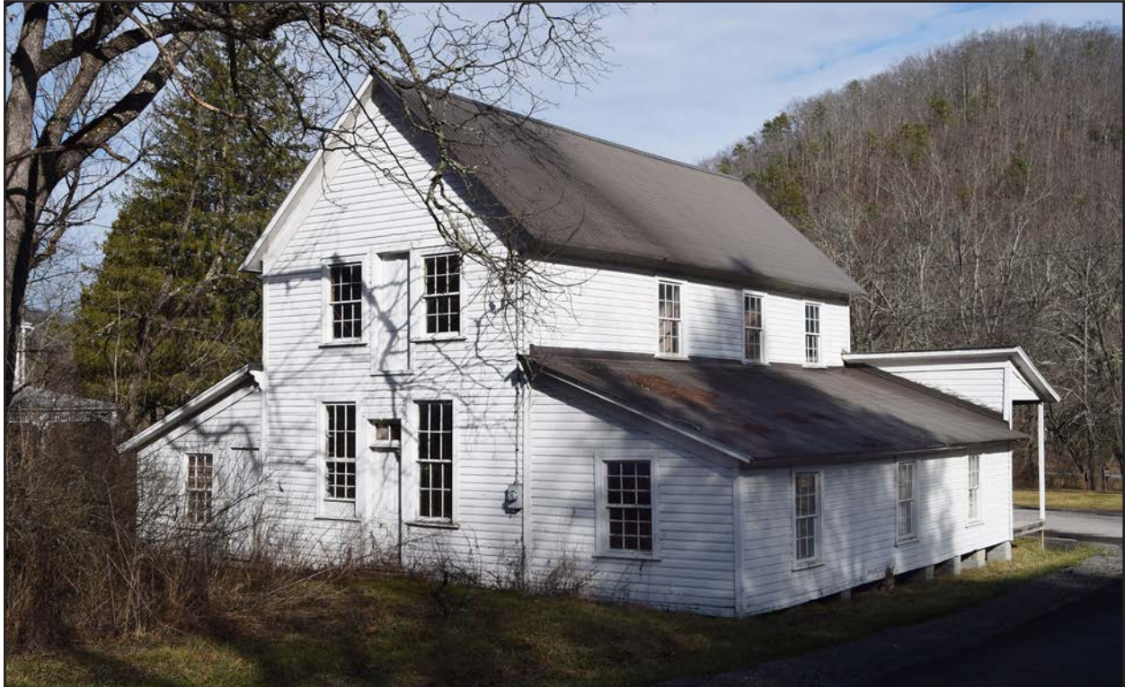
Photo 25. PH-0037-65, store, facing east.
