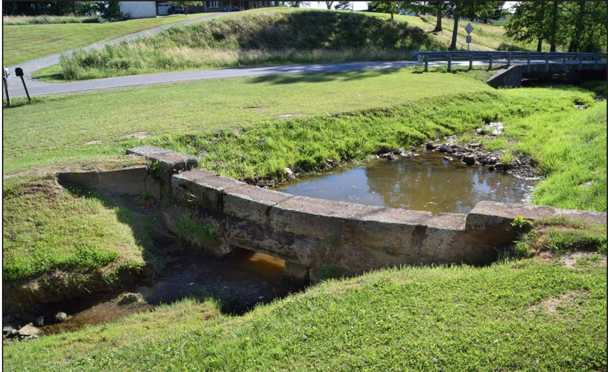
Figure 10. LE-0004 and 46LE61, baptismal pond and masonry dam, facing southwest.
