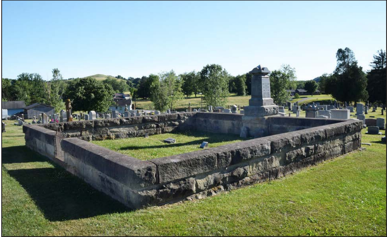
Figure 9. LE-0004 and 46LE61, view of Jackson family plot, Broad Run Cemetery, facing southwest.
