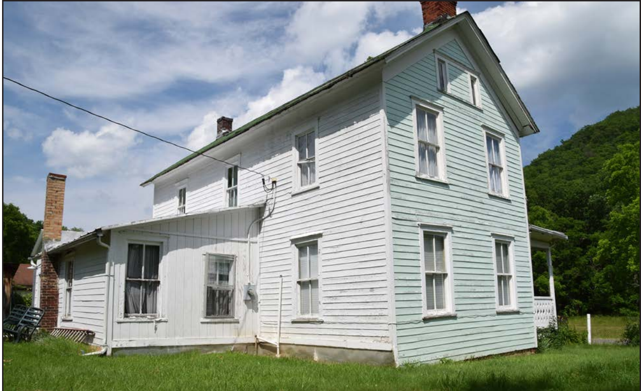
Figure 49. PH-0471, northwest and southwest elevations, facing east.
