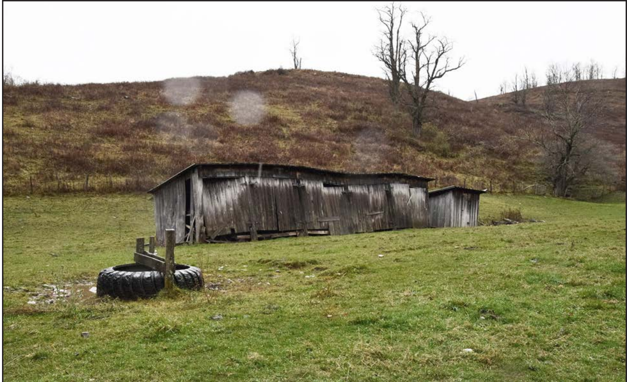
Figure 71. PH-0903, Shed 1 and 2, facing northwest.
