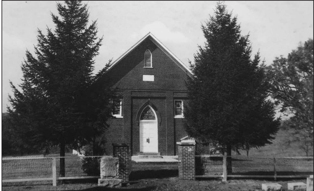
Figure 6. LE-0004, view of east façade of church in 1954, facing west.
