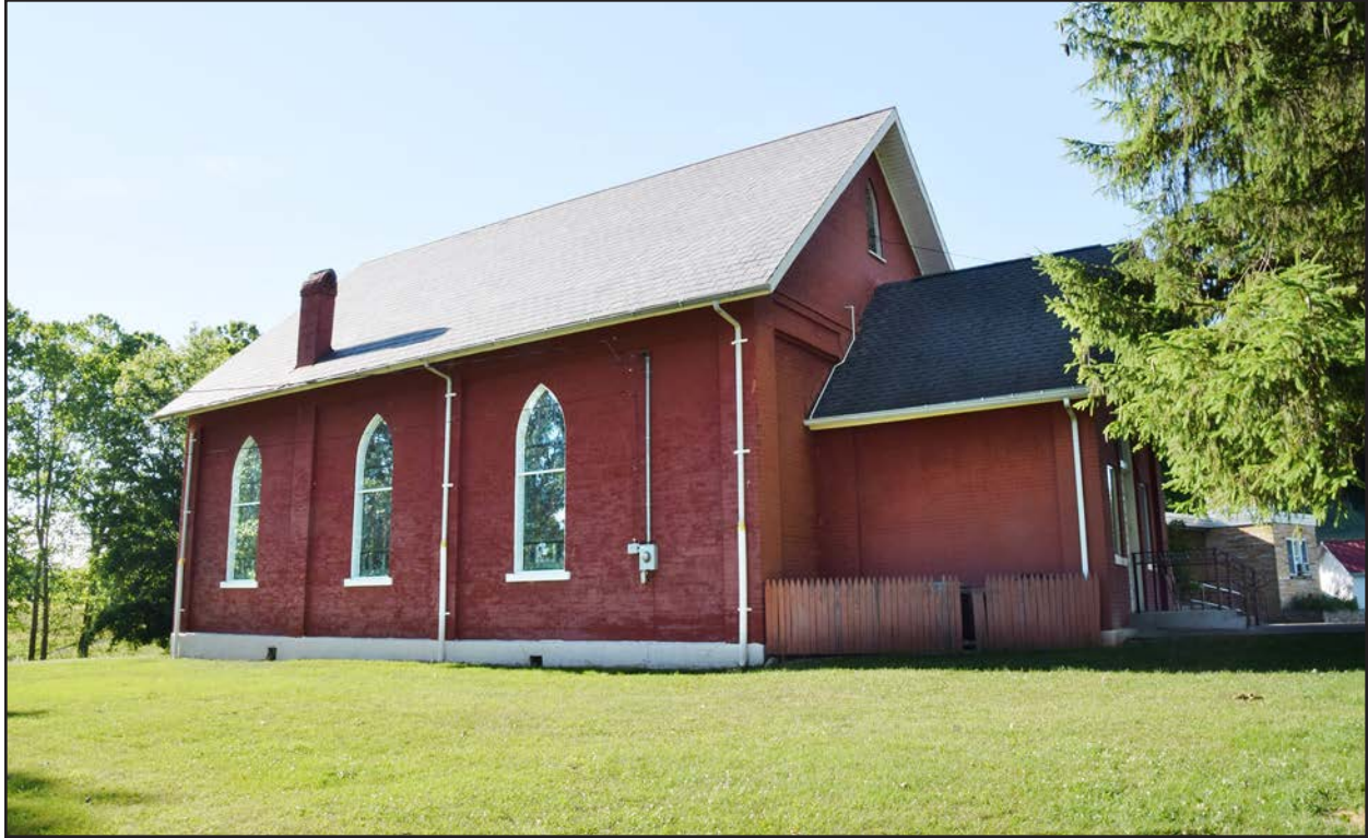
Figure 1. LE-0004, view of Broad Run Baptist Church, facing north-northwest.
