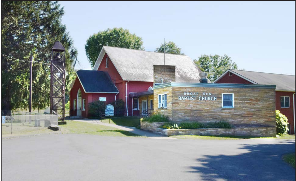
Figure 7. LE-0004, view of Broad Run Baptist Church Annex, facing south-southwest.
