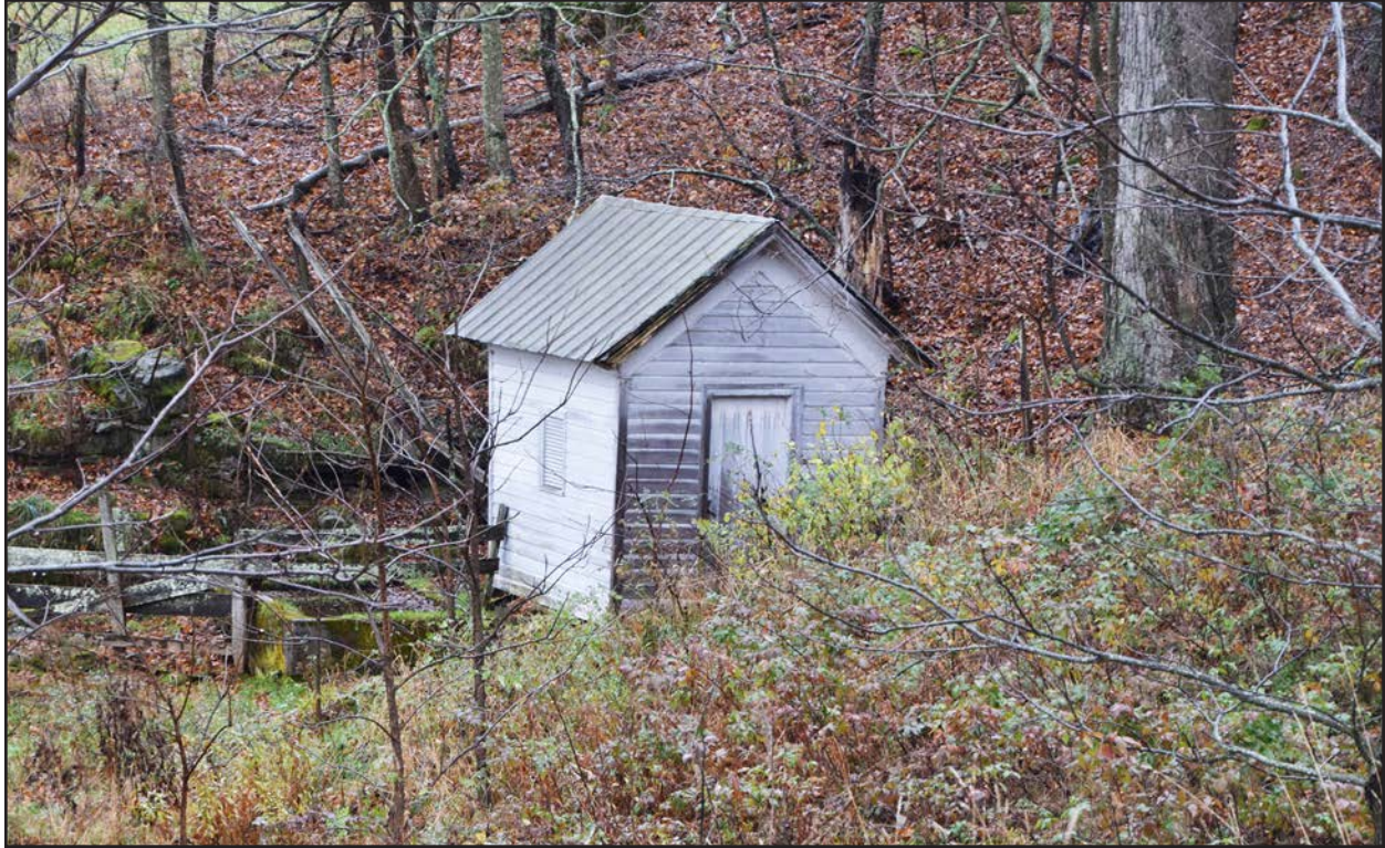
Figure 74. PH-0903, Well house, facing southeast.
