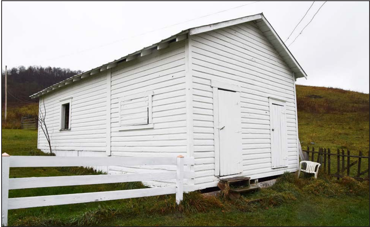
Figure 66. PH-0903, Outbuilding 1, facing north.
