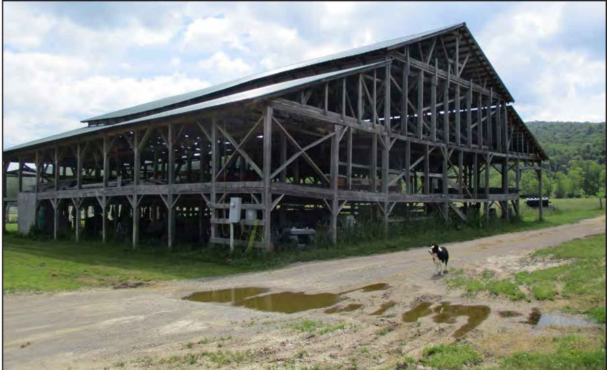
Photo 32. PH-0954, barn, facing east.
