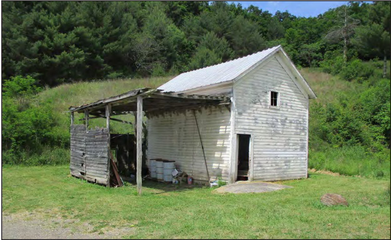
Photo 29. PH-0954, shed, facing west.
