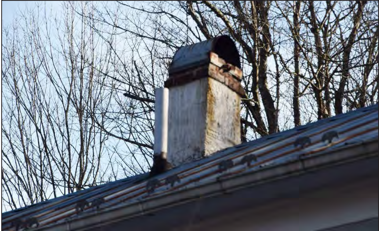
Photo 16. PH-0470, chimney detail, facing southwest.
