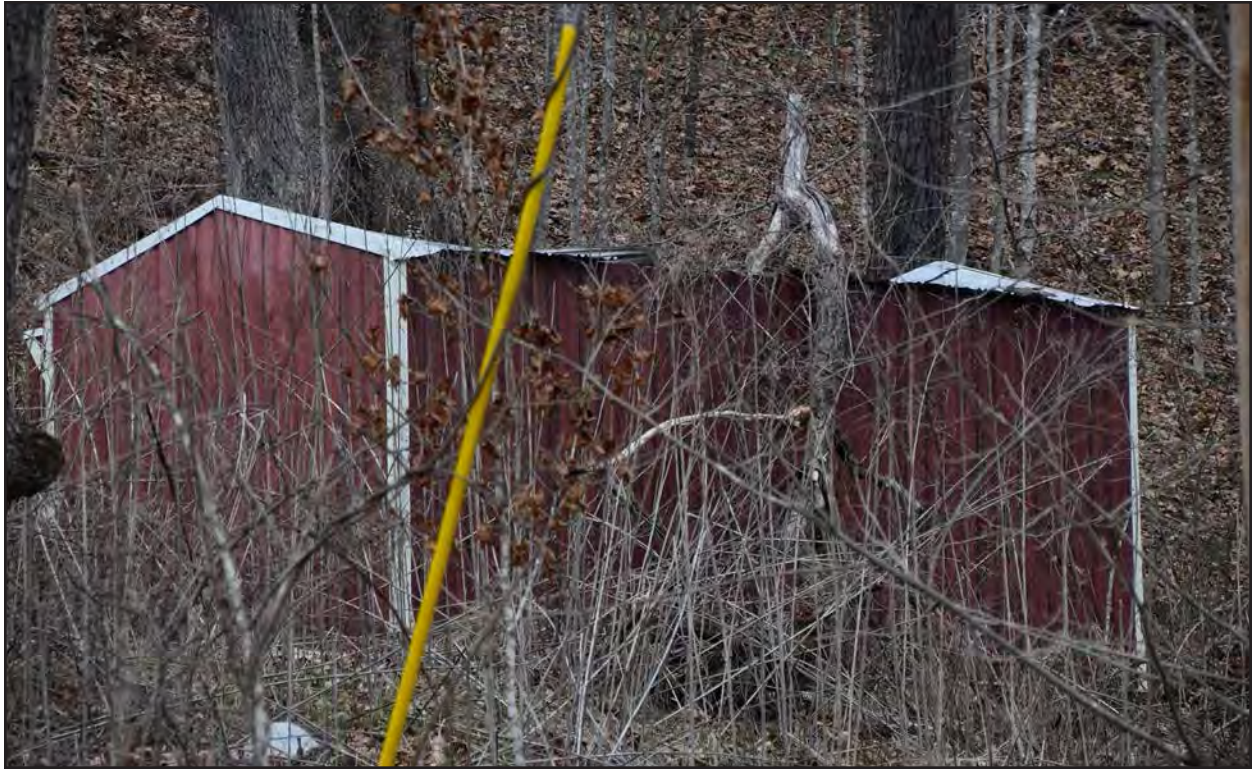
Photo 5. PH-0037-64, shed, facing north.
