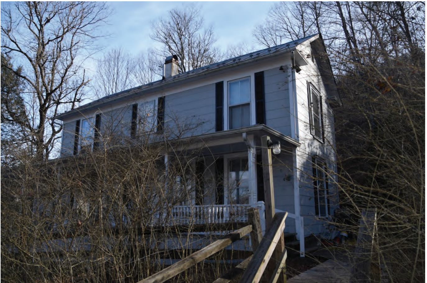
PH-0470, facing southeast.
