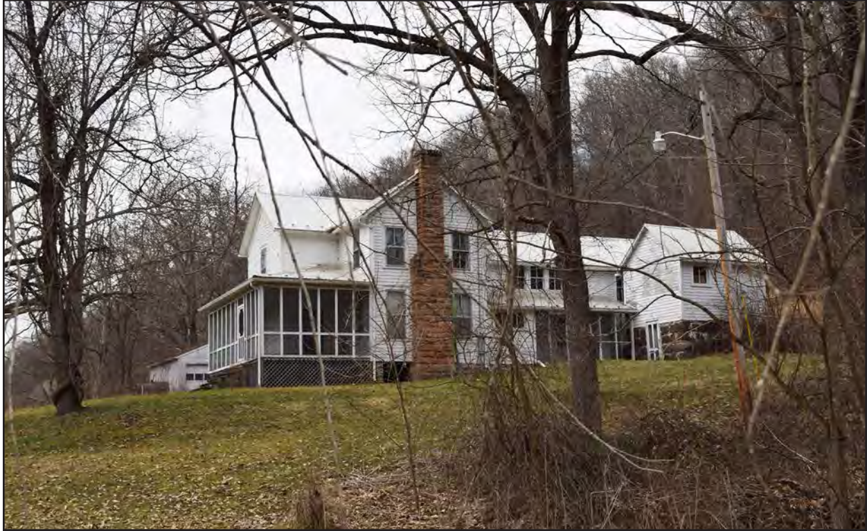
Photo 1. PH-0037-64, dwelling, facing northwest.
