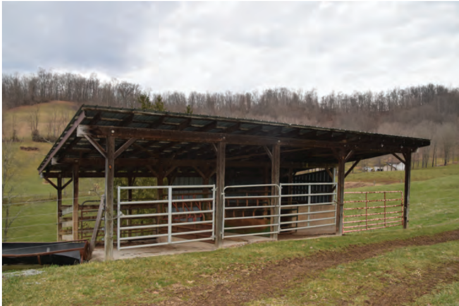
UP-0818, Shed, facing west.
