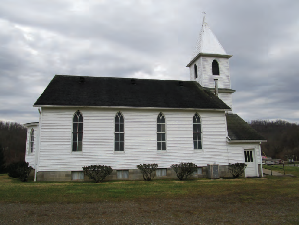
UP-0113, Gothic Revival Church, facing south.
