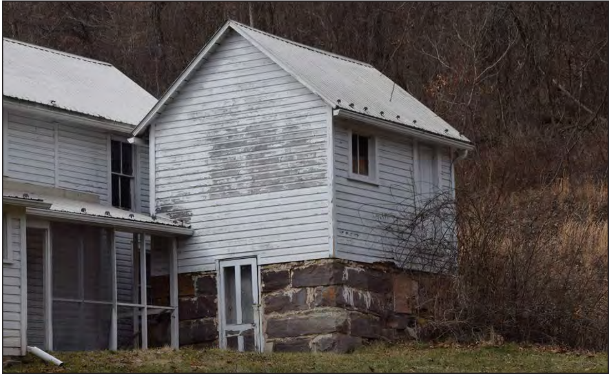
Photo 3. PH-0037-64 smokehouse/root cellar, facing northwest.
