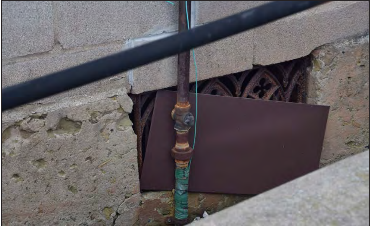
Photo 42. UP-0113, Gothic Revival Church, foundation detail, facing north.
