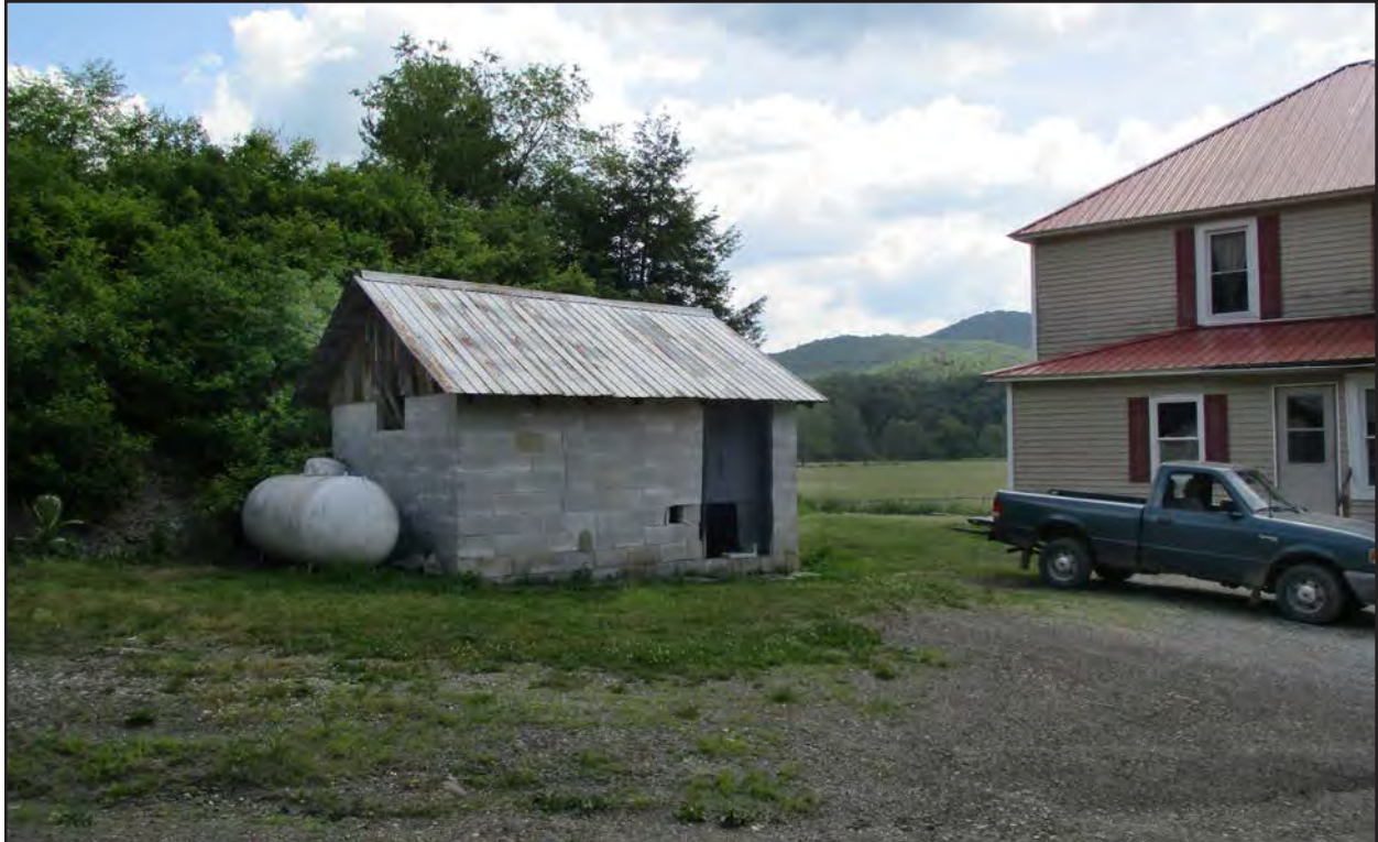
Photo 28. PH-0954, shed, facing east
