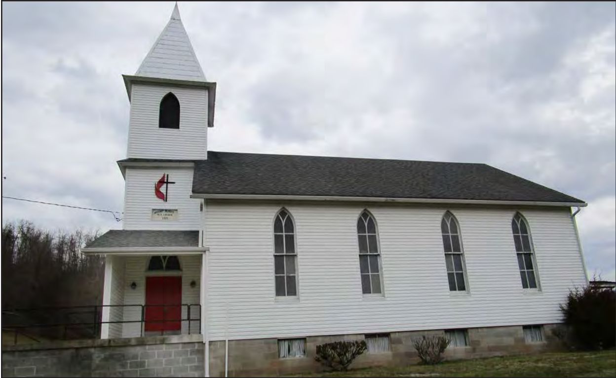
Photo 40. UP-0113, Gothic Revival Church, facing north.
