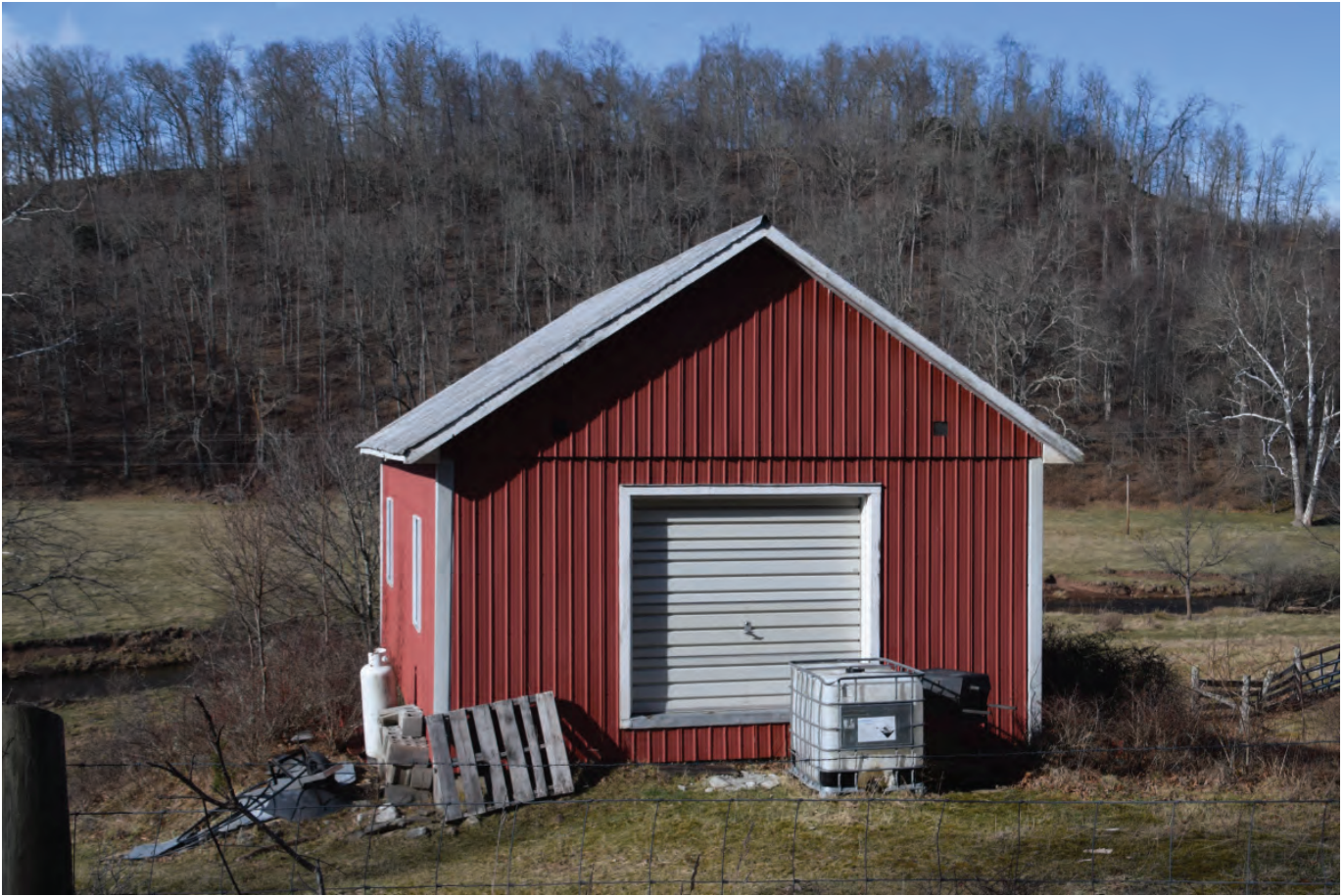
PH-0462, shed, facing north.
