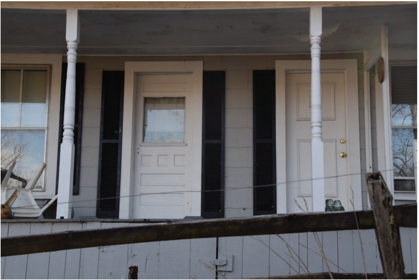
PH-0470, front detail, facing south.
