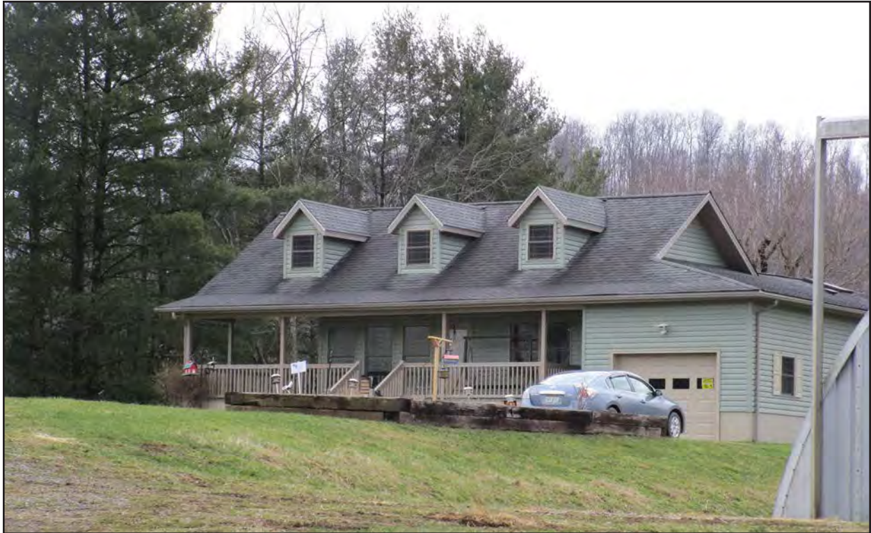
Photo 33. UP-0818, house, facing southeast.
