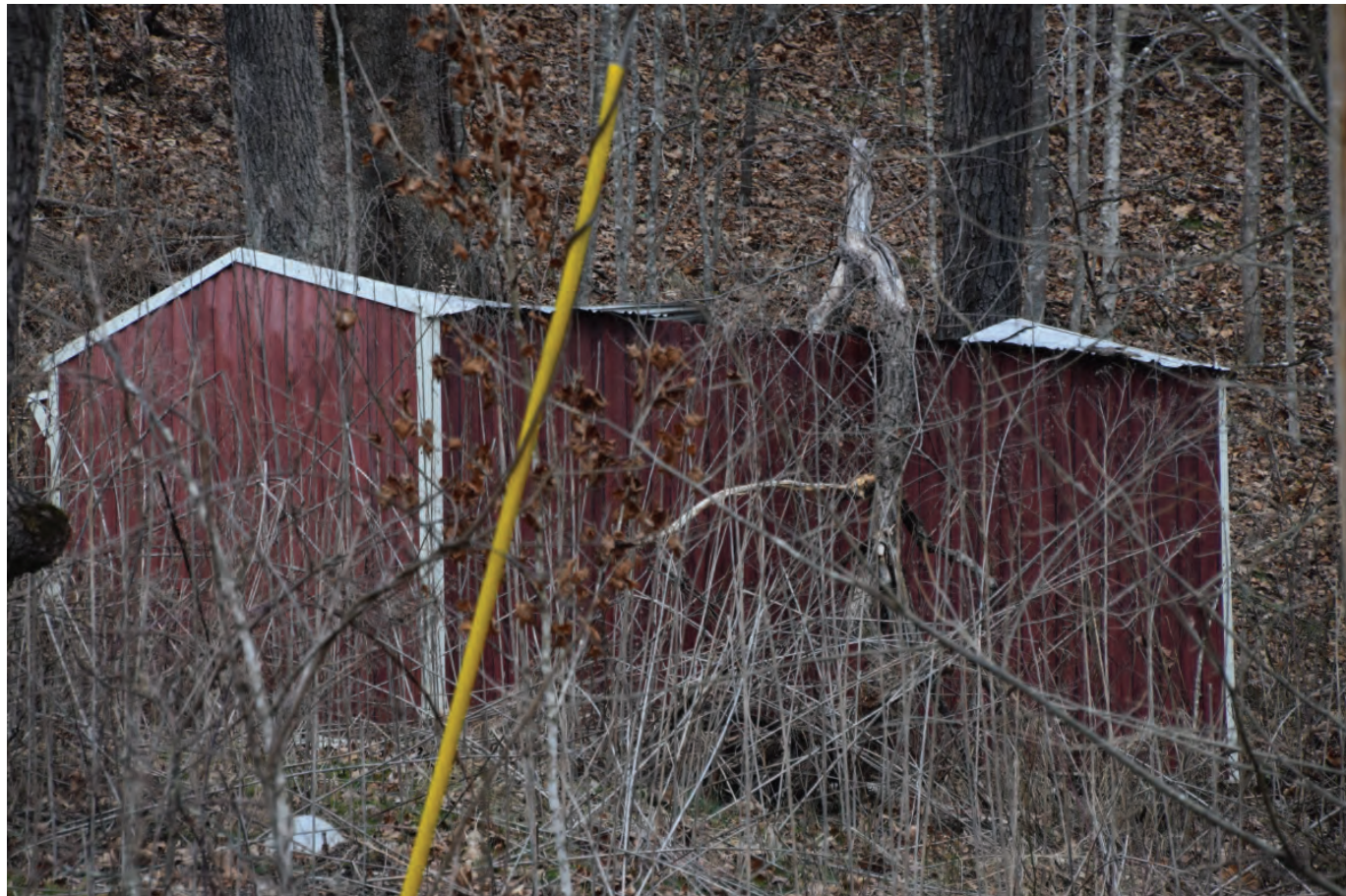
PH-0037-64, shed, facing north.
