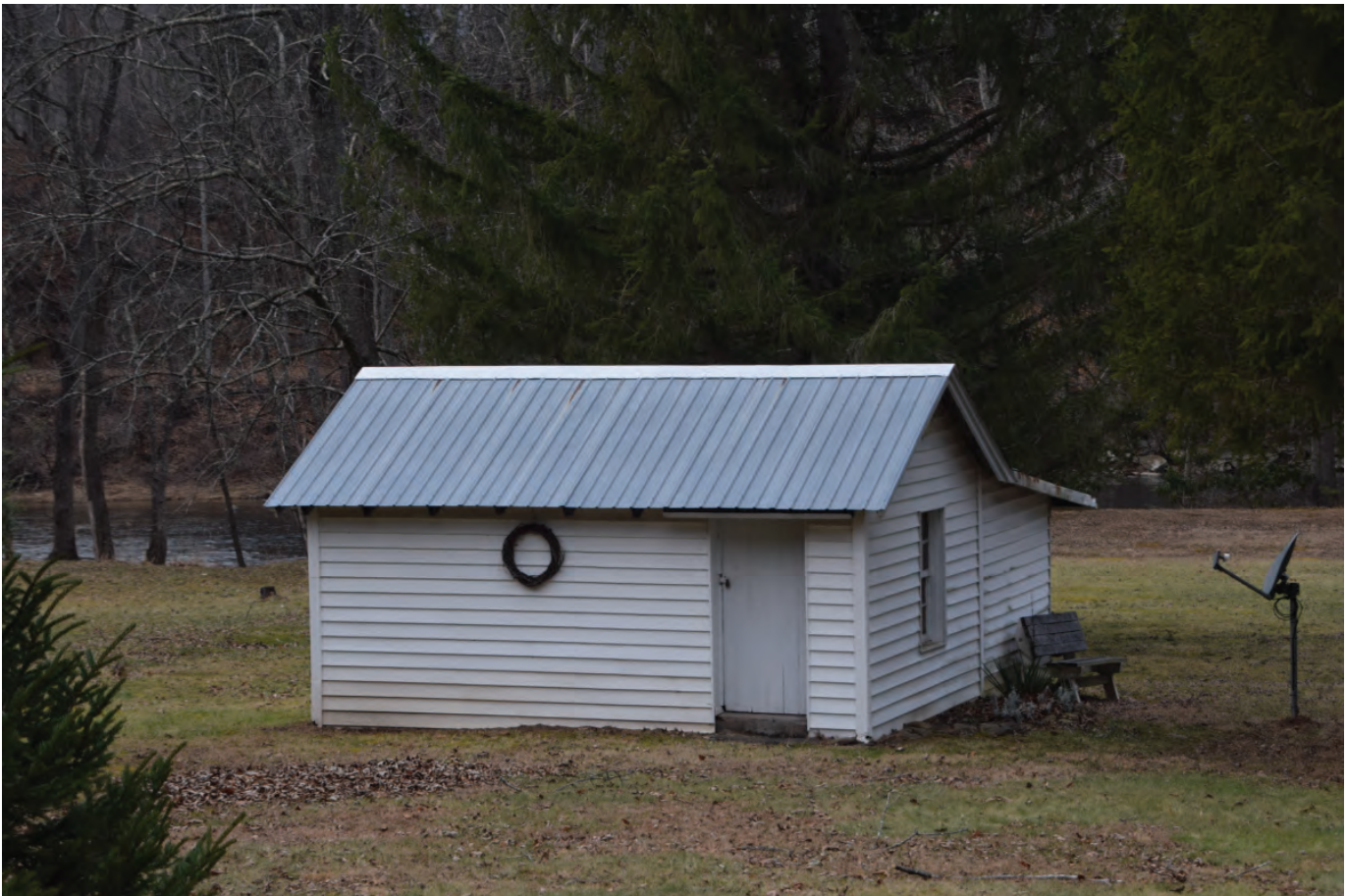
PH-0490, Shed, facing northwest.
