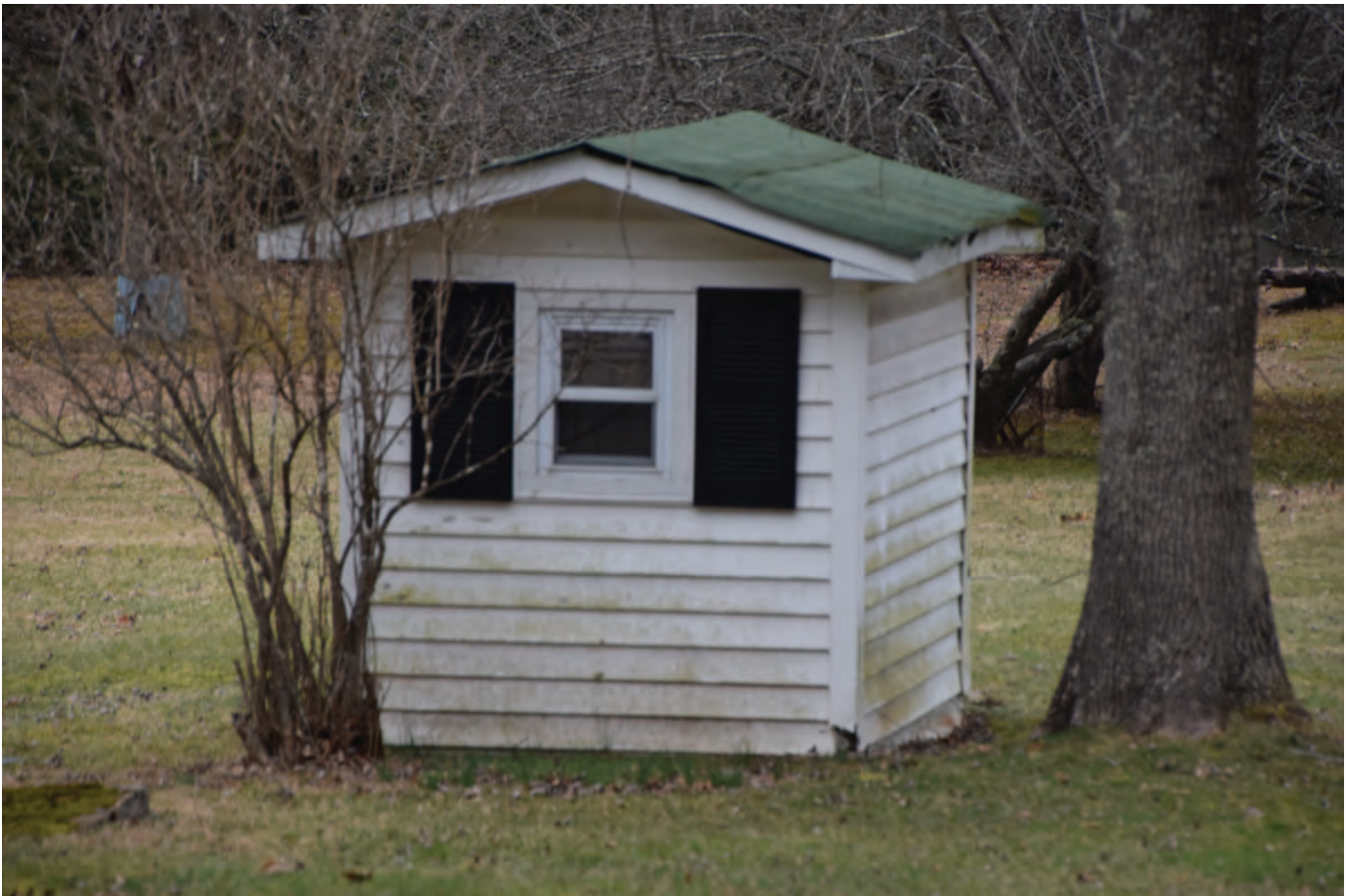
PH-0490, Well House, facing northwest.
