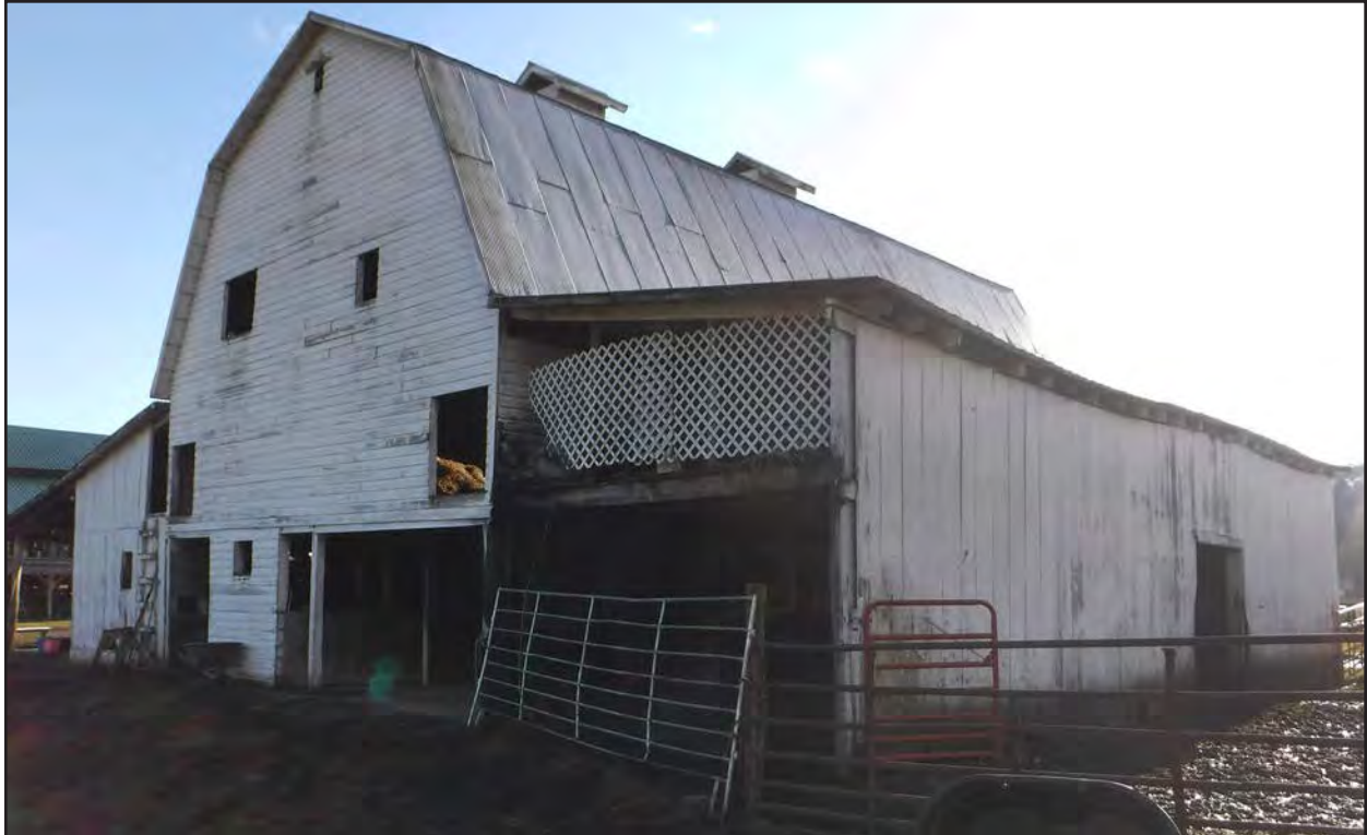
Photo 30. PH-0954, barn, facing south.
