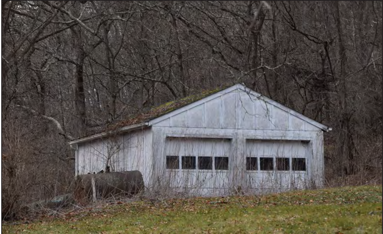
Photo 4. PH-0037-64, garage, facing west.
