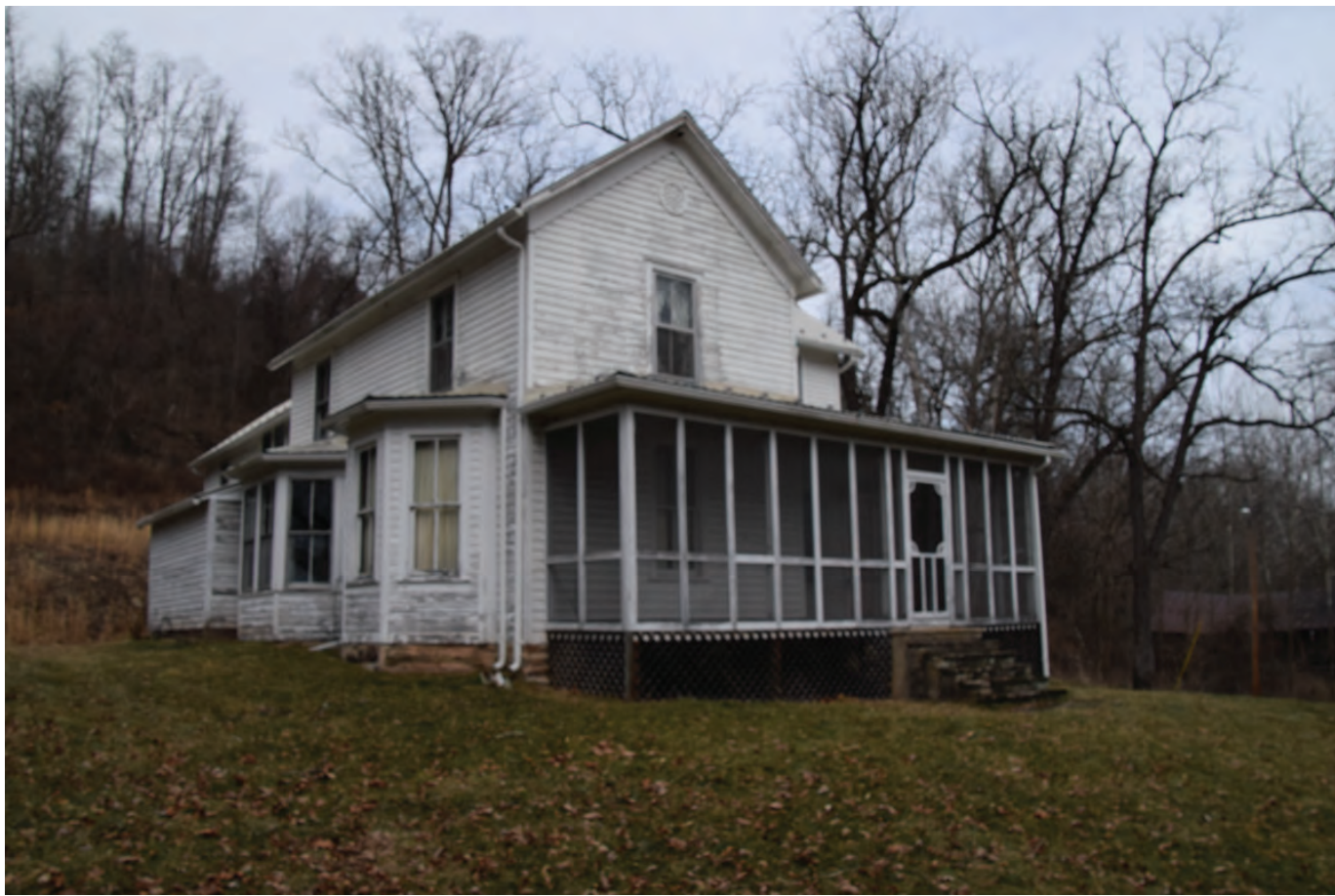
PH-0037-64, dwelling, facing northeast.
