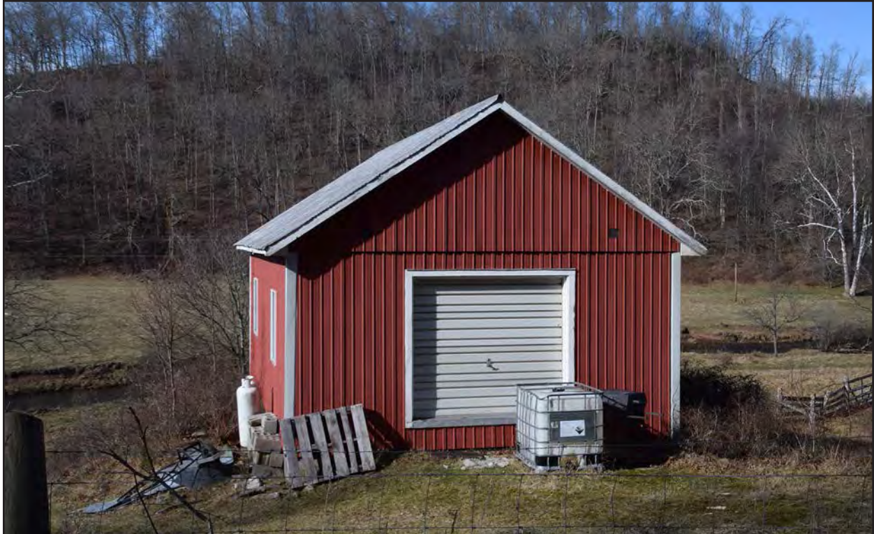
Photo 14. PH-0462, shed, facing north.
