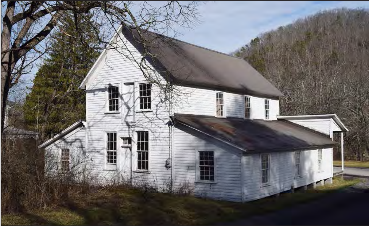
Photo 8. PH-0037-65, store, facing east.
