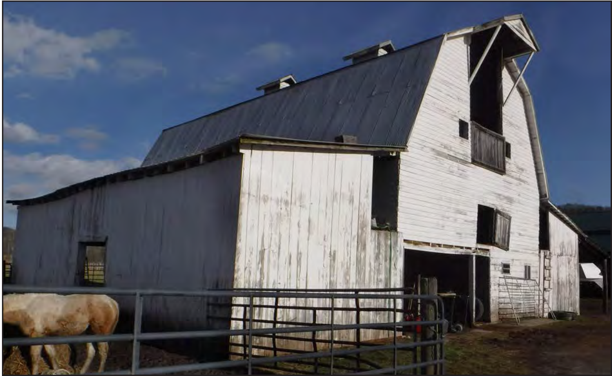
Photo 31. PH-0954, barn, facing east.
