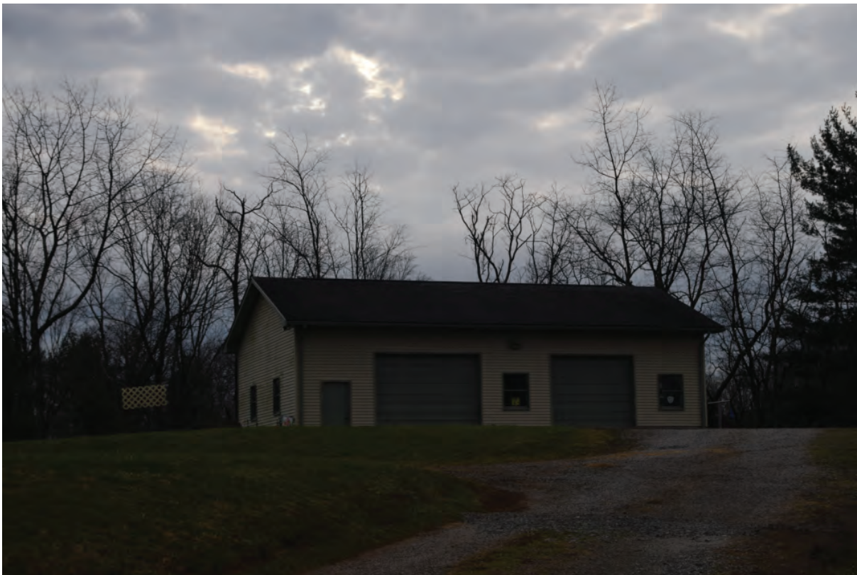
UP-0818, Garage, facing east.
