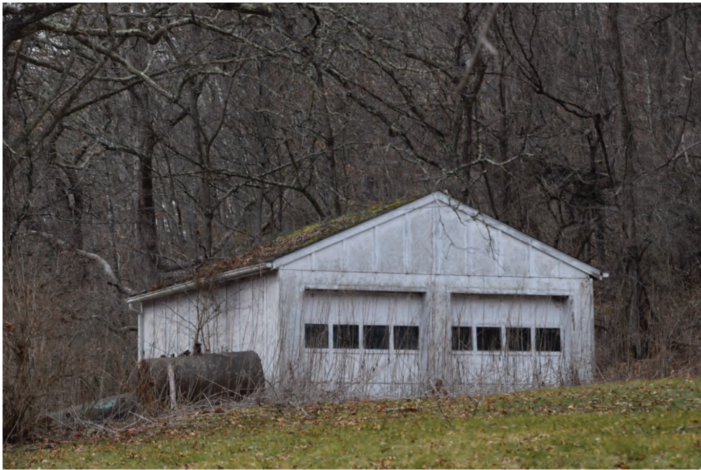
PH-0037-64, garage, facing west.
