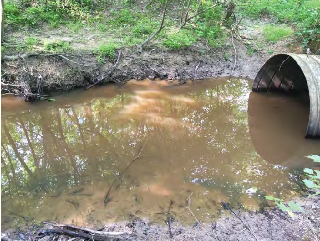
Waterbody data point sjoo009 facing south across.
