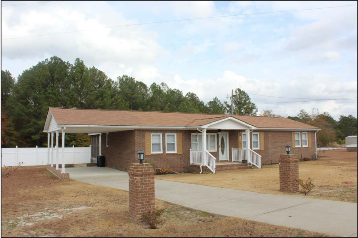
Photo 17. CD1469, facing east-northeast.
