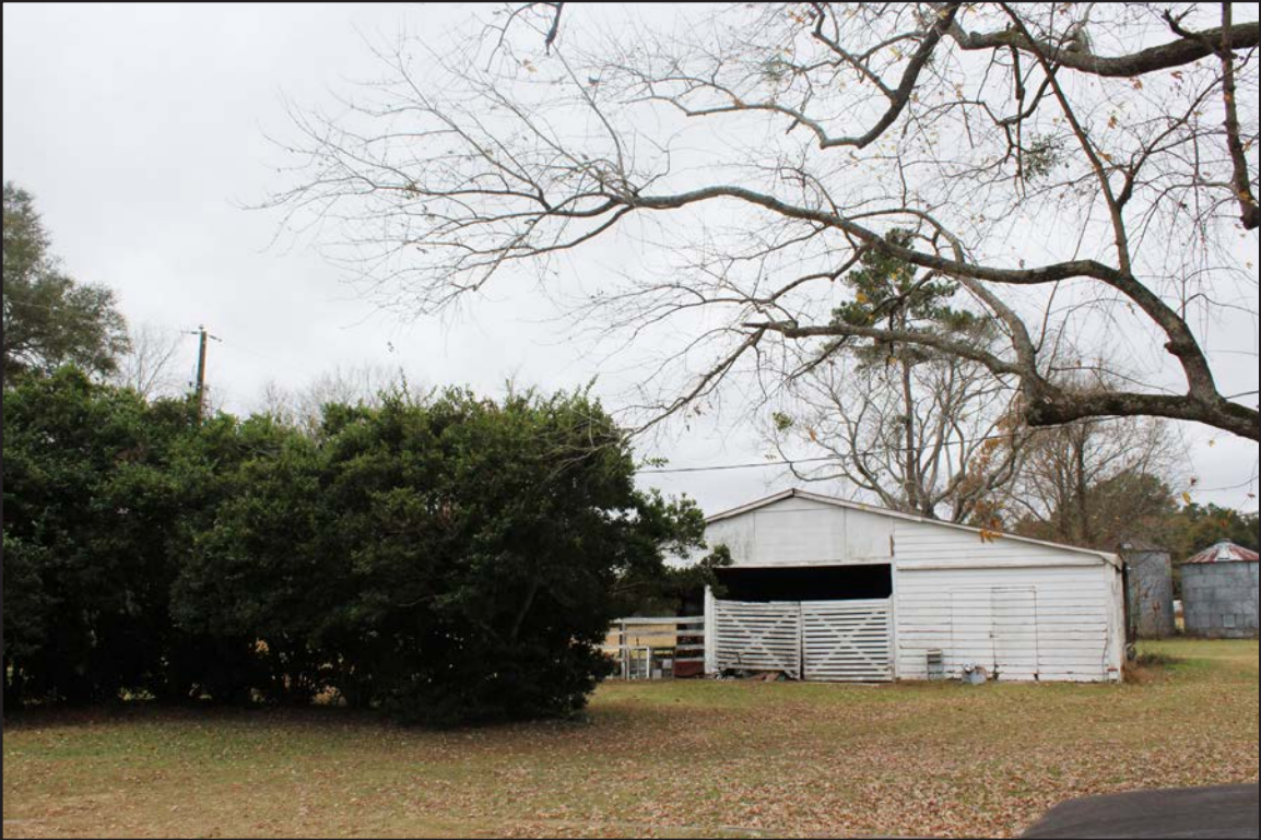
Photo 5. CD1465, Outbuilding 4, facing northwest.
