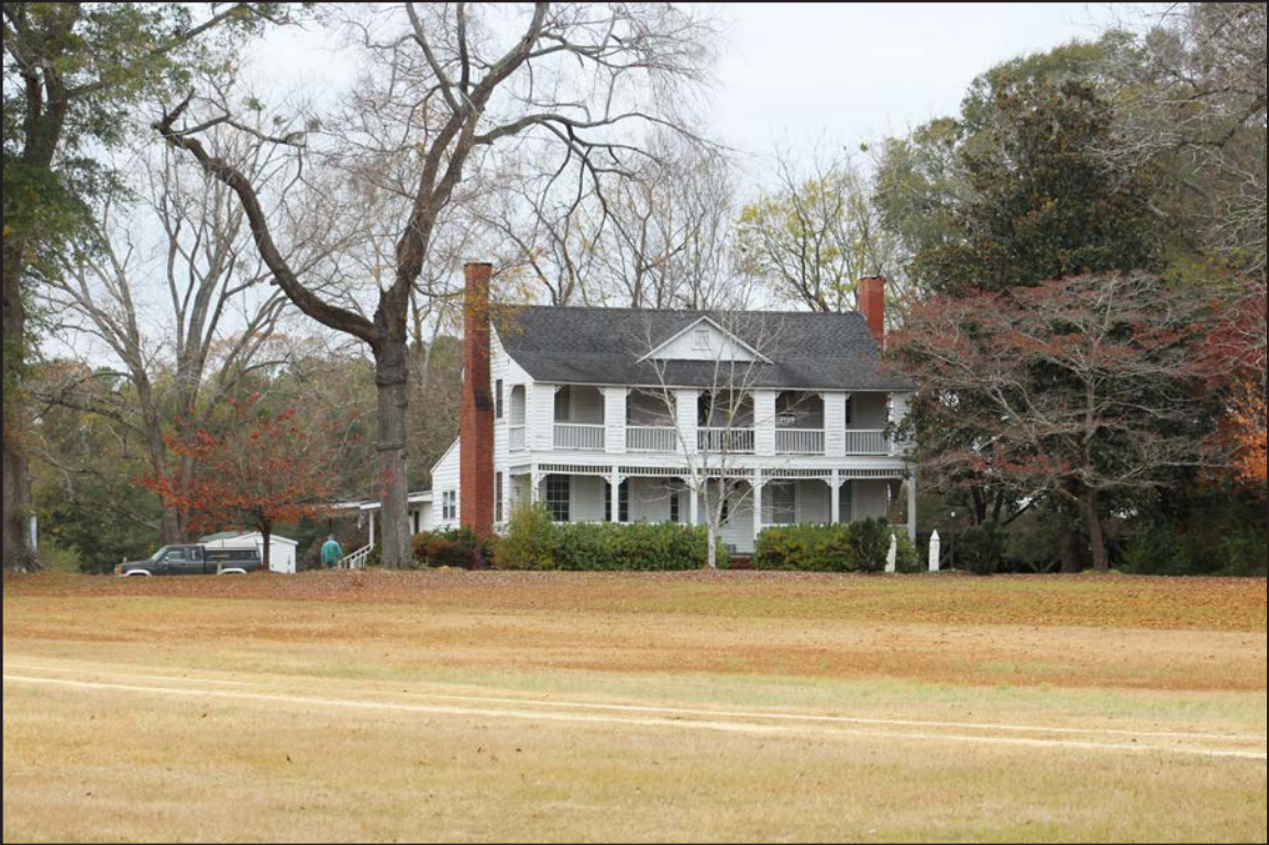
Photo 1. CD1465, facing northwest.
