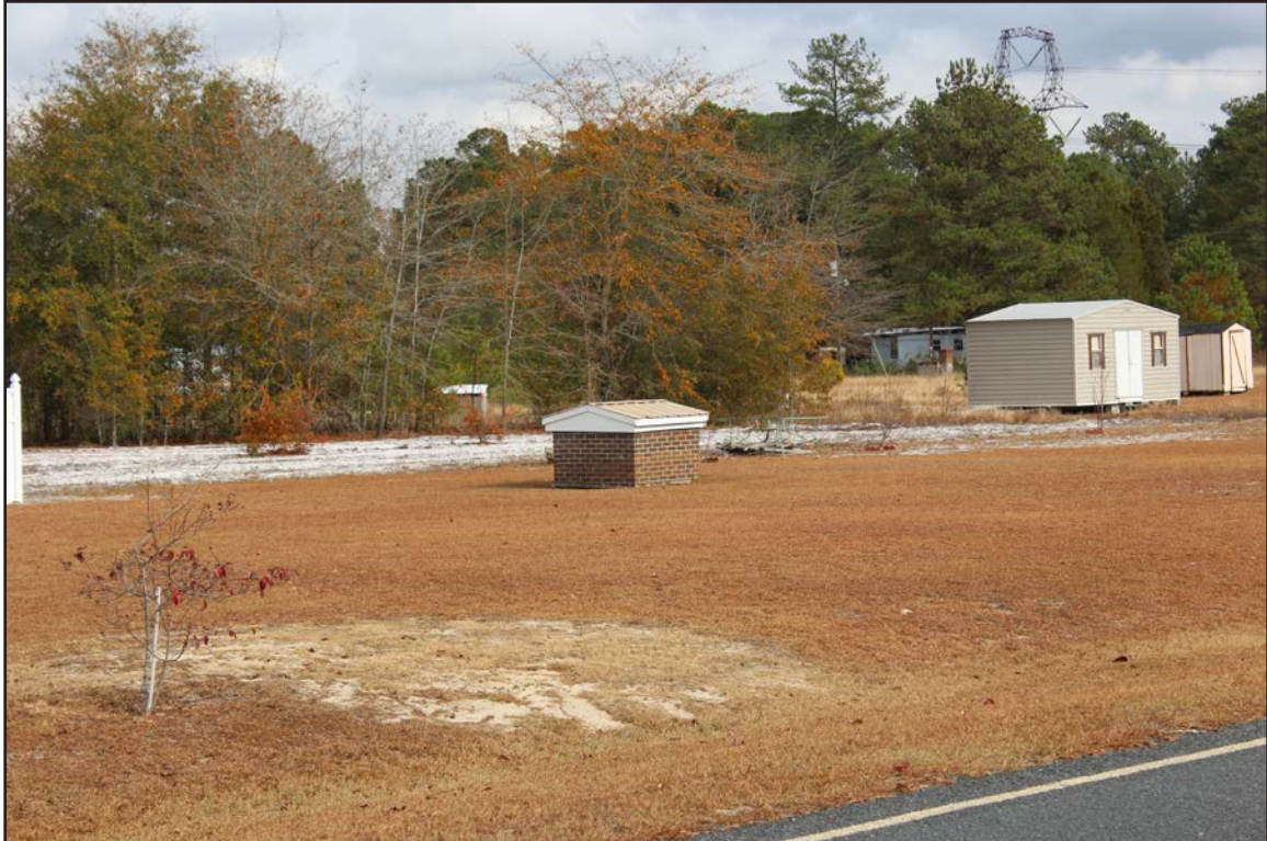
Photo 20. CD1469, well house, facing east.
