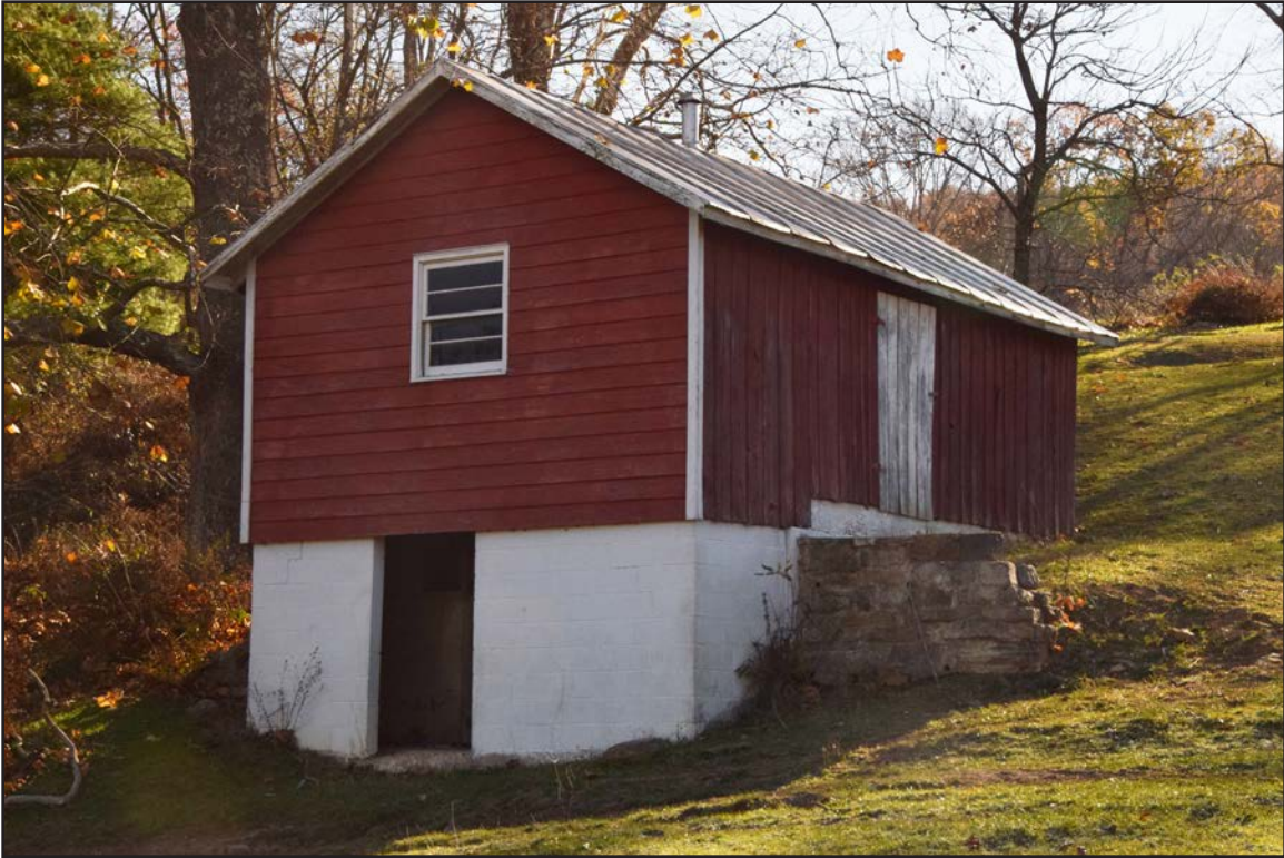
Figure 57. 007-5709, Outbuilding 1, facing southeast.
