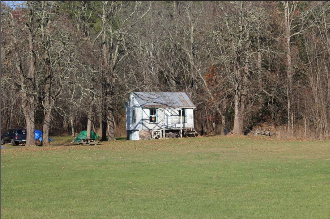
Figure 4. 007-0447. Outbuilding 1, facing southeast.
