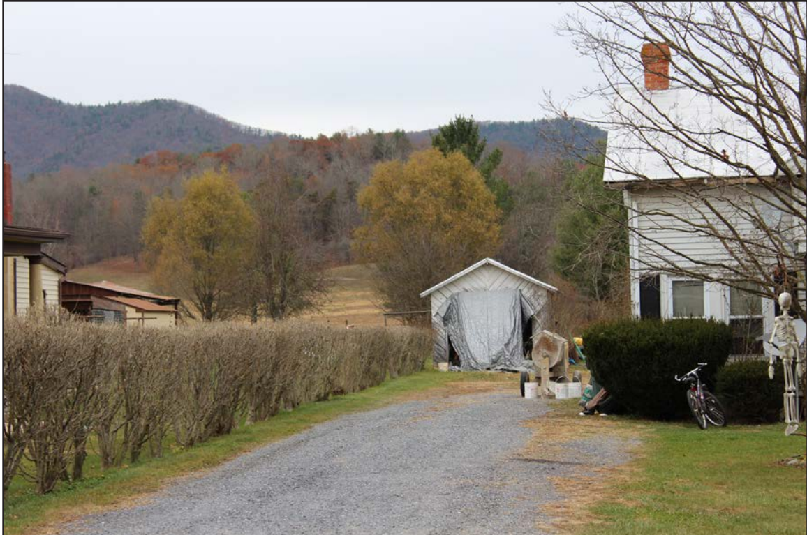
Figure 172. 007-5733, garage, facing north.
