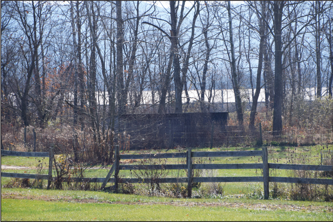
Figure 13. 007-0467, chicken house, facing southwest.
