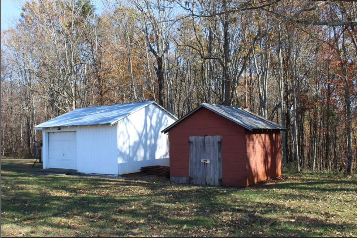
Figure 159. 007-5730, Shed 1 and Shed 2, facing northeast.
