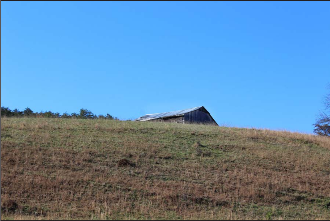
Figure 223. 008-5065, barn, facing west.
