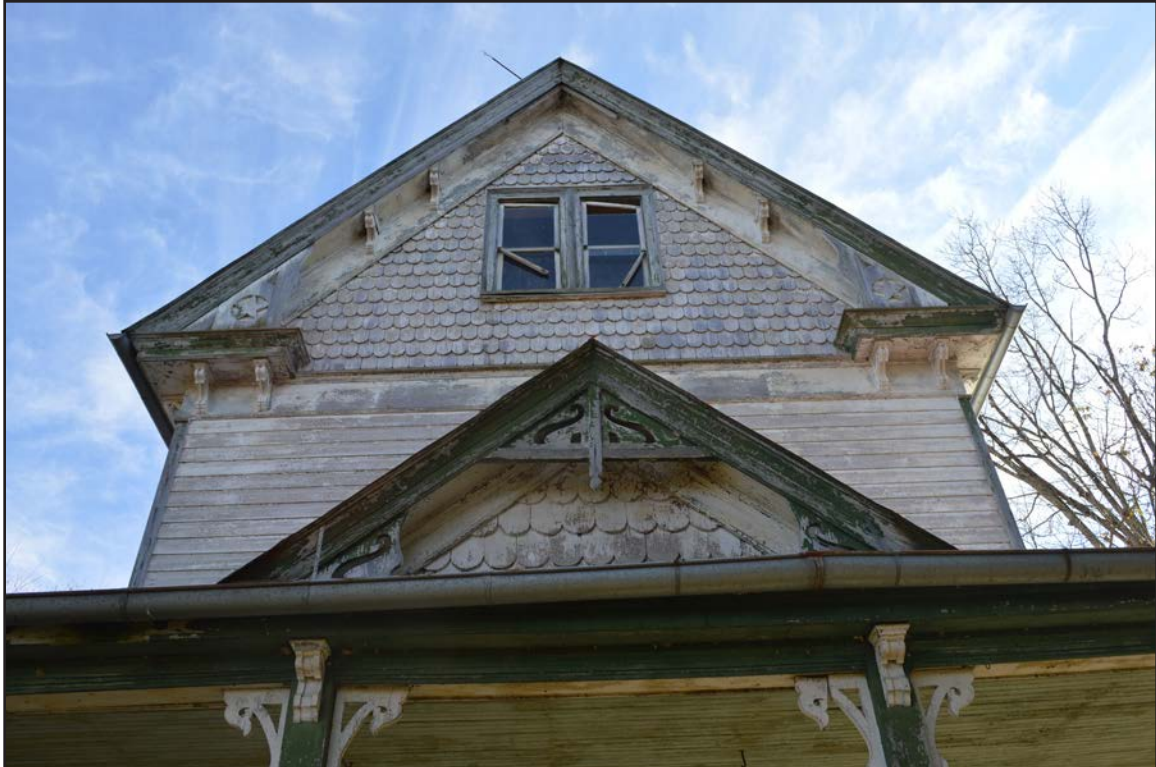
Figure 26. 007-0487, gable details on house, facing southeast.
