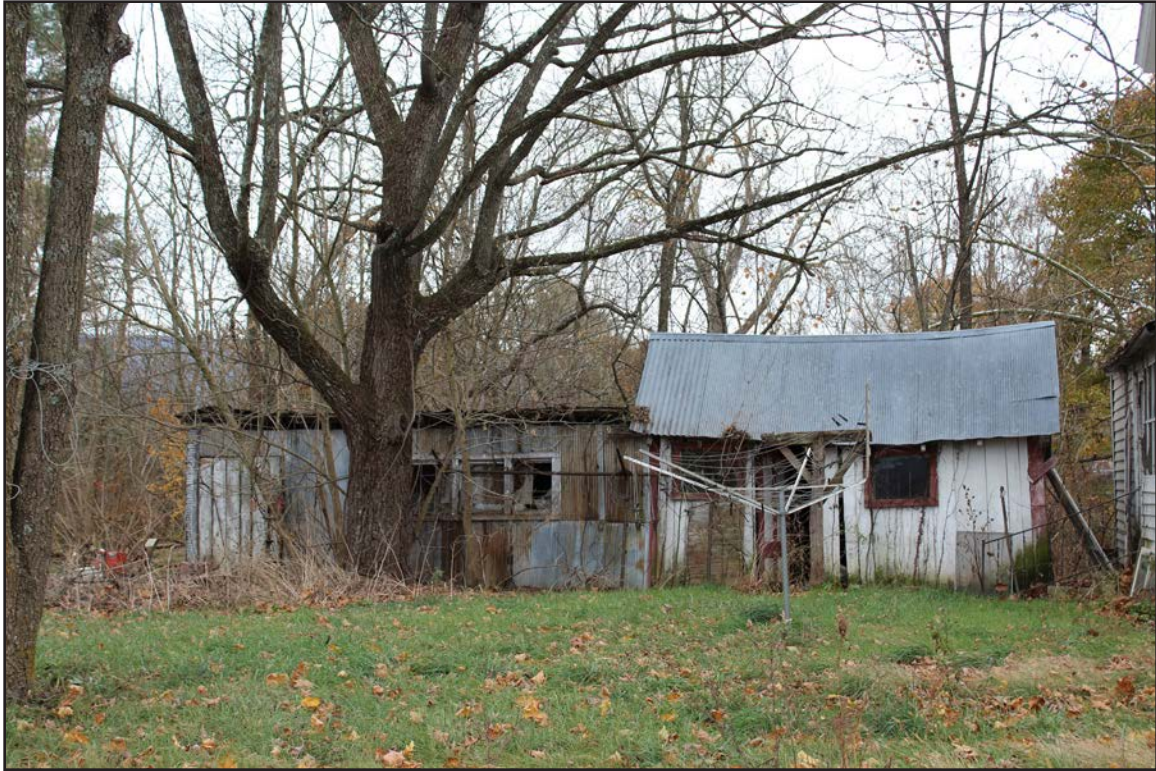
Figure 167. 007-5731, shed, facing south.
