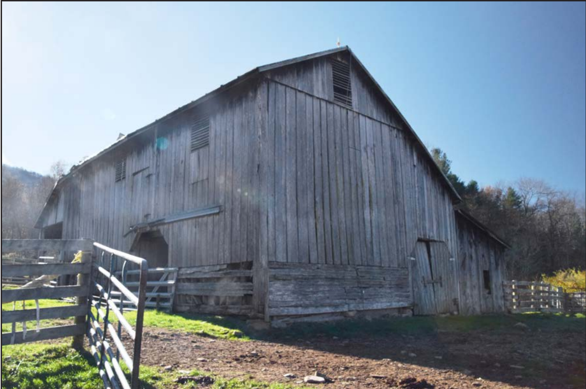
Figure 62. 007-5709, barn, facing south by southeast.
