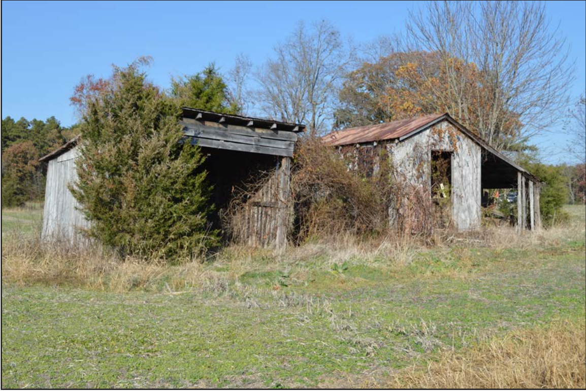
Figure 239. 014-5085, ca. 1920s sheds, facing northeast.
