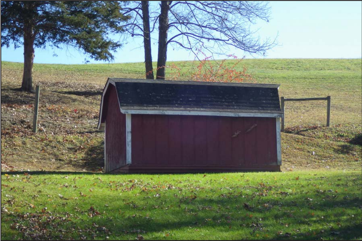
Figure 91. 007-5716, shed, facing southeast.
