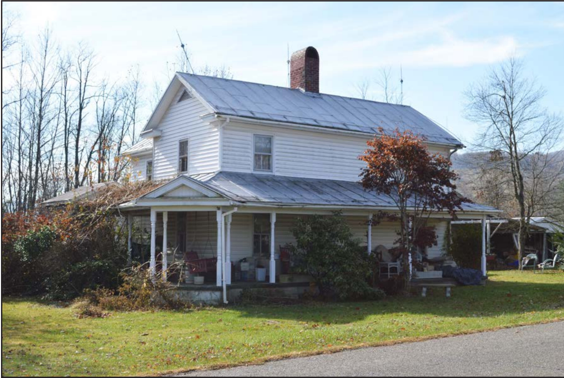
Figure 19. 007-0476, dwelling house, facing southwest.
