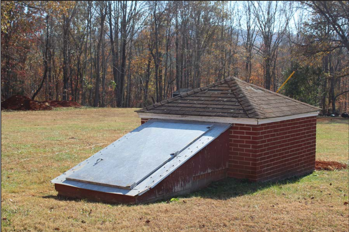
Figure 160. 007-5730, well house, facing southeast.
