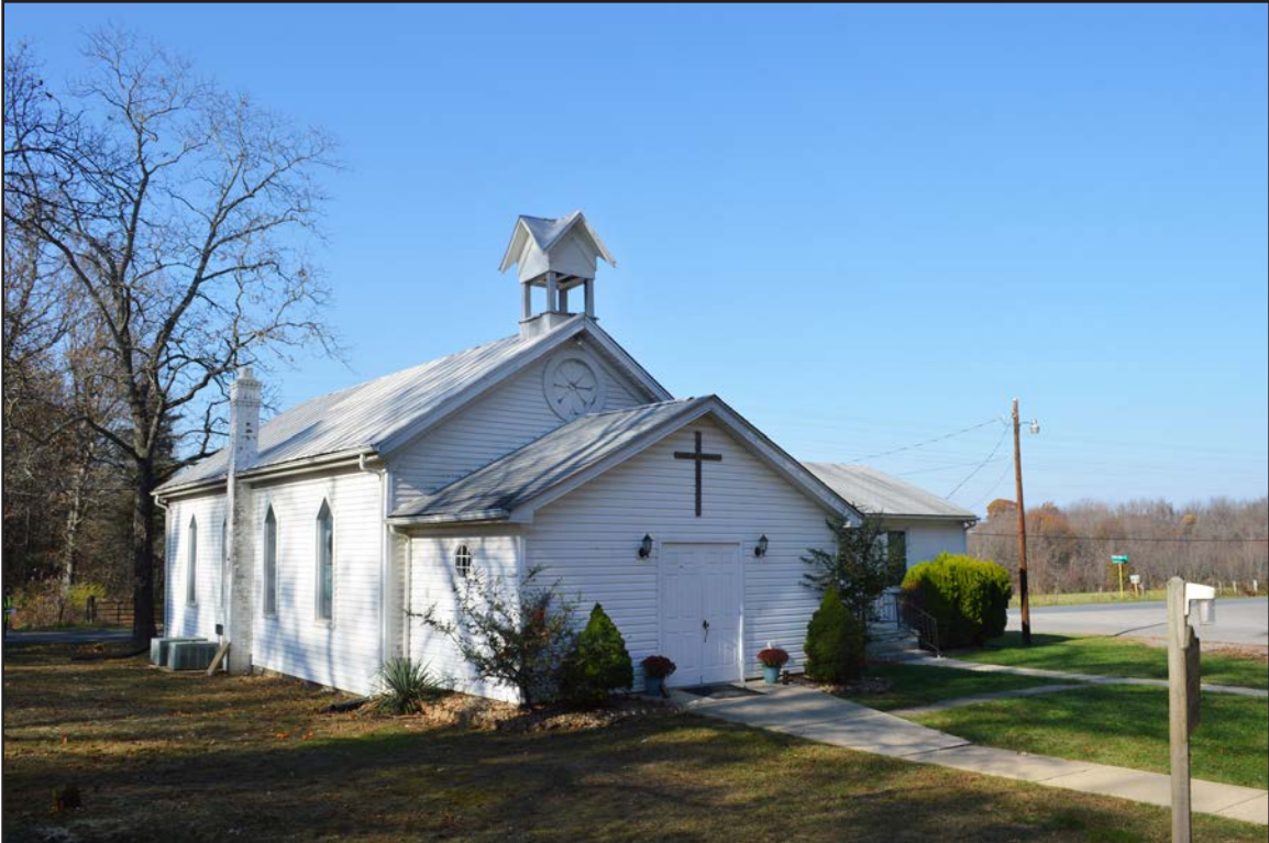
Figure 34. 007-0863, church, facing southwest.
