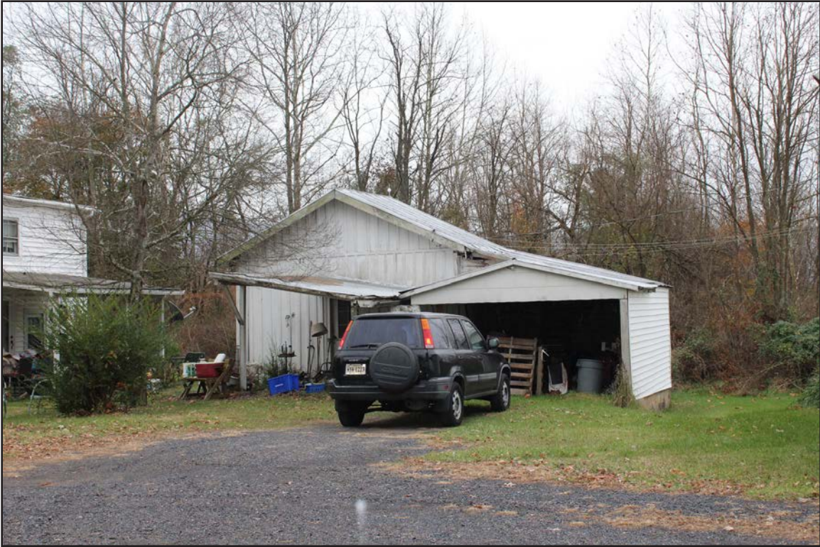
Figure 21. 007-0476, garage and shed, facing southeast.
