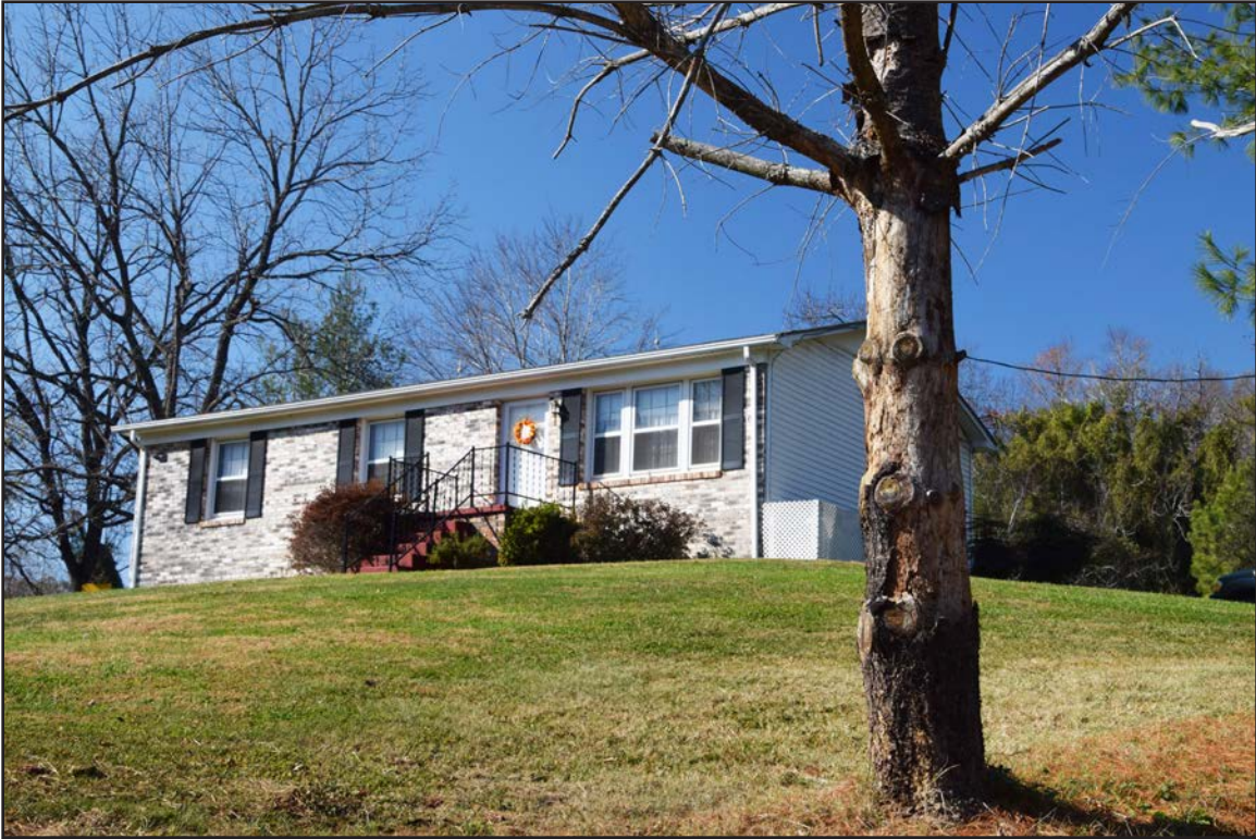
Figure 255. 062-5223, house, facing west.
