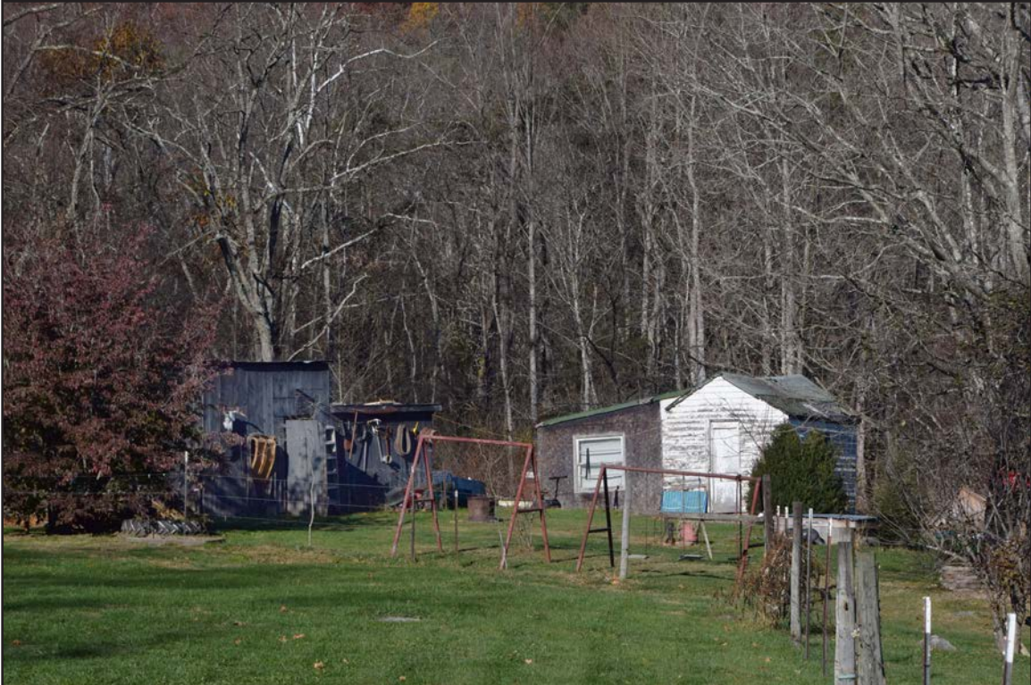
Figure 74. 007-5712, Shed 2 and Shed 3, facing west.
