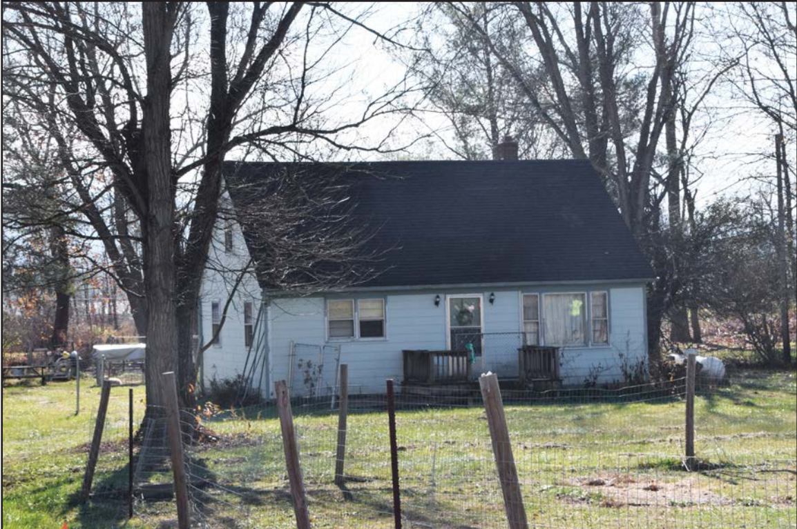
Figure 142. 007-5727, house, facing southwest.
