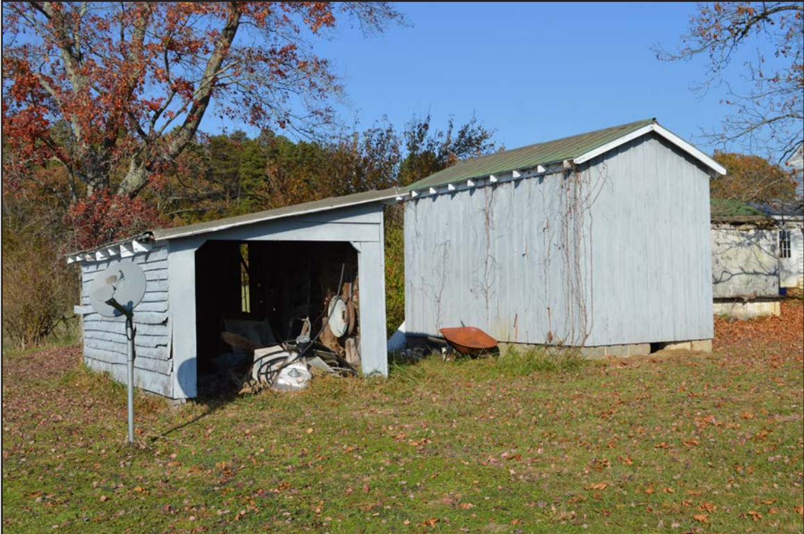
Figure 236. 014-5085, ca. 1930 outbuildings, facing northeast.
