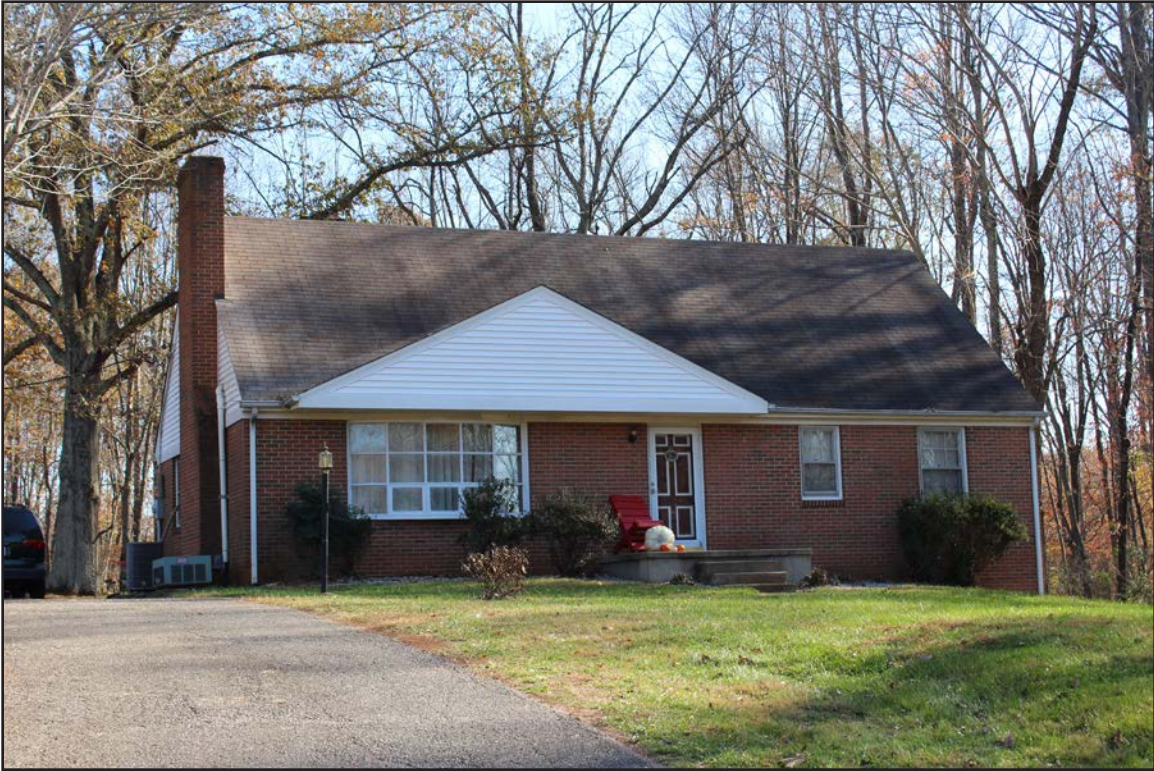
Figure 161. 007-5730, parsonage, facing east-southeast.
