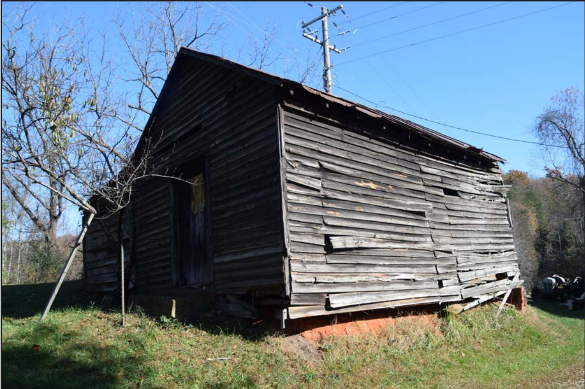
Figure 256. 062-5223, outbuilding, facing southeast.
