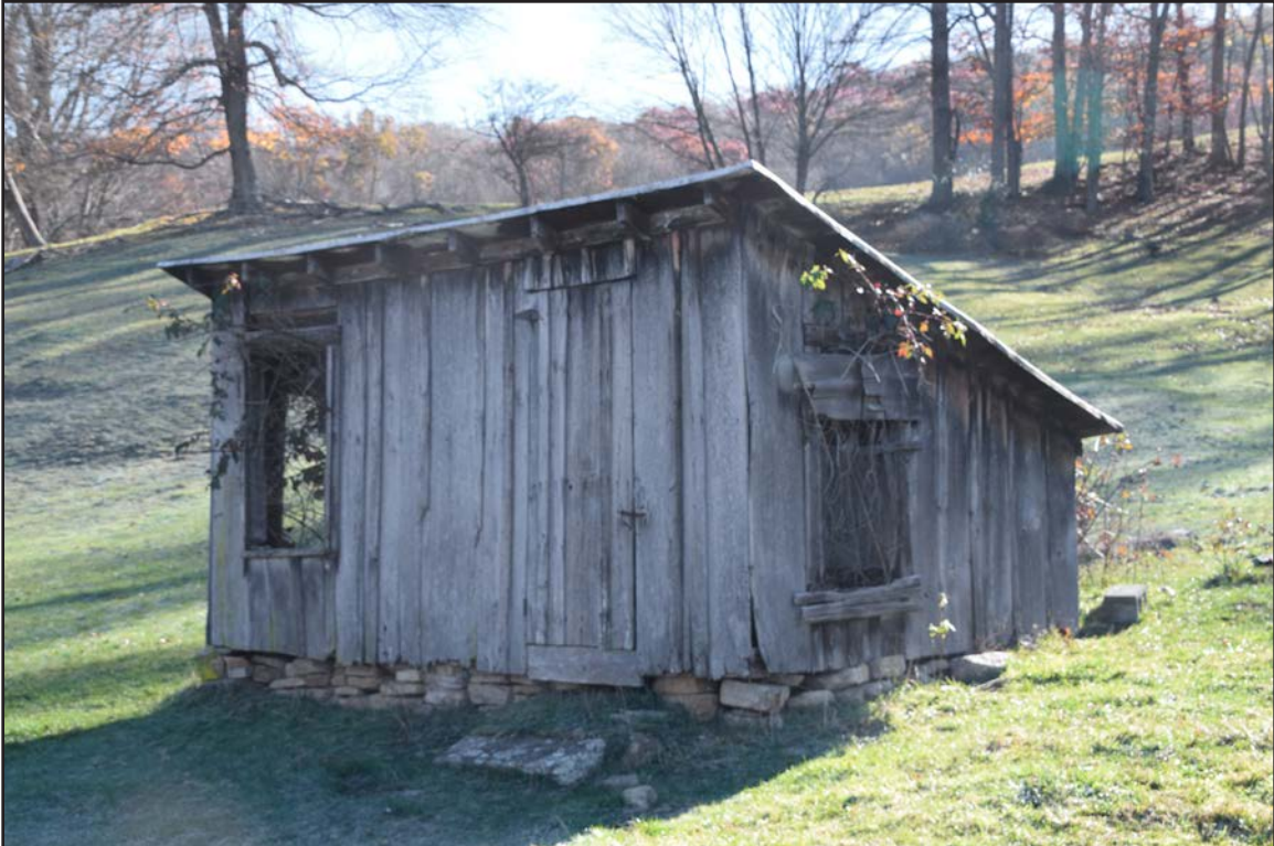
Figure 58. 007-5709, Outbuilding 2, facing southeast.
