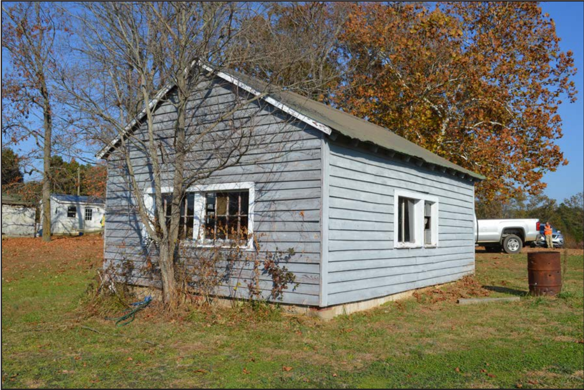
Figure 237. 014-5085, ca. 1930 outbuilding, facing northeast.
