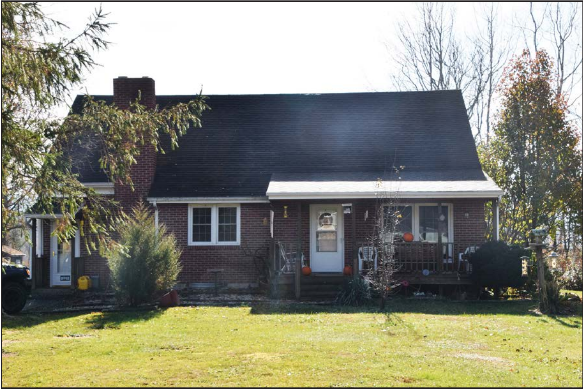
Figure 139. 007-5726, house, facing southwest.
