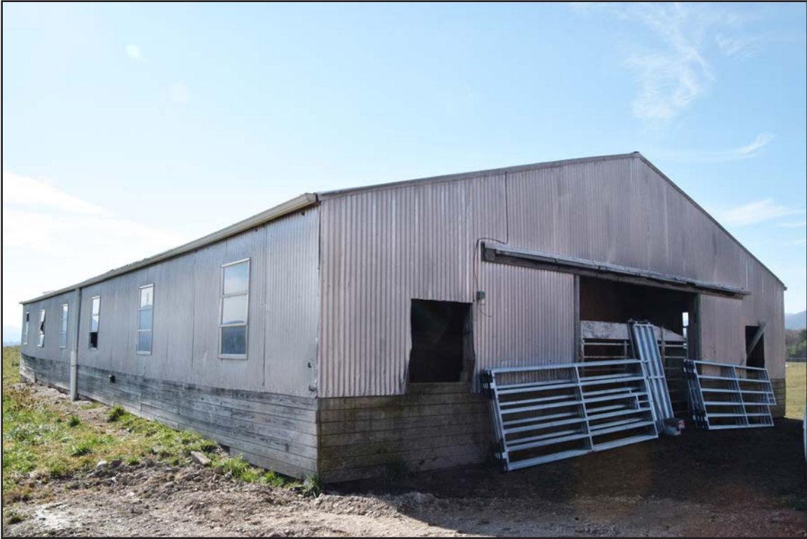
Figure 9. 007-0463, Barn 3, facing southeast.
