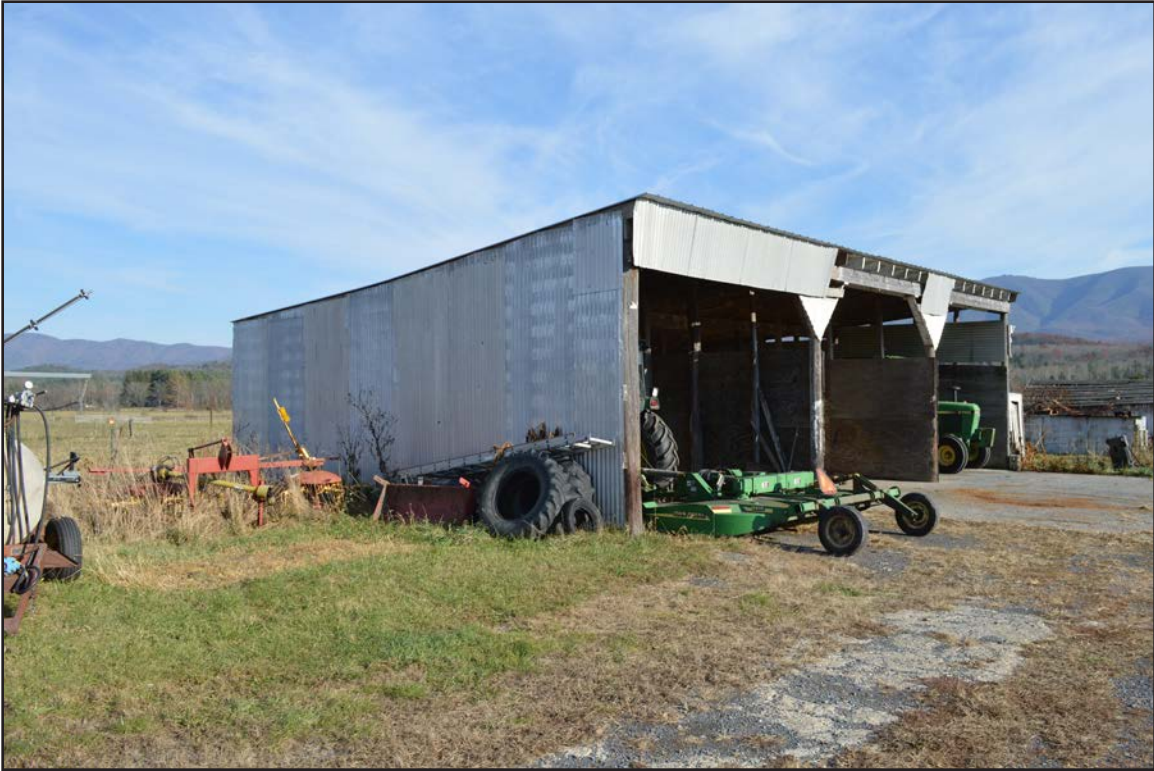
Figure 81. 007-5714, shed, facing east.
