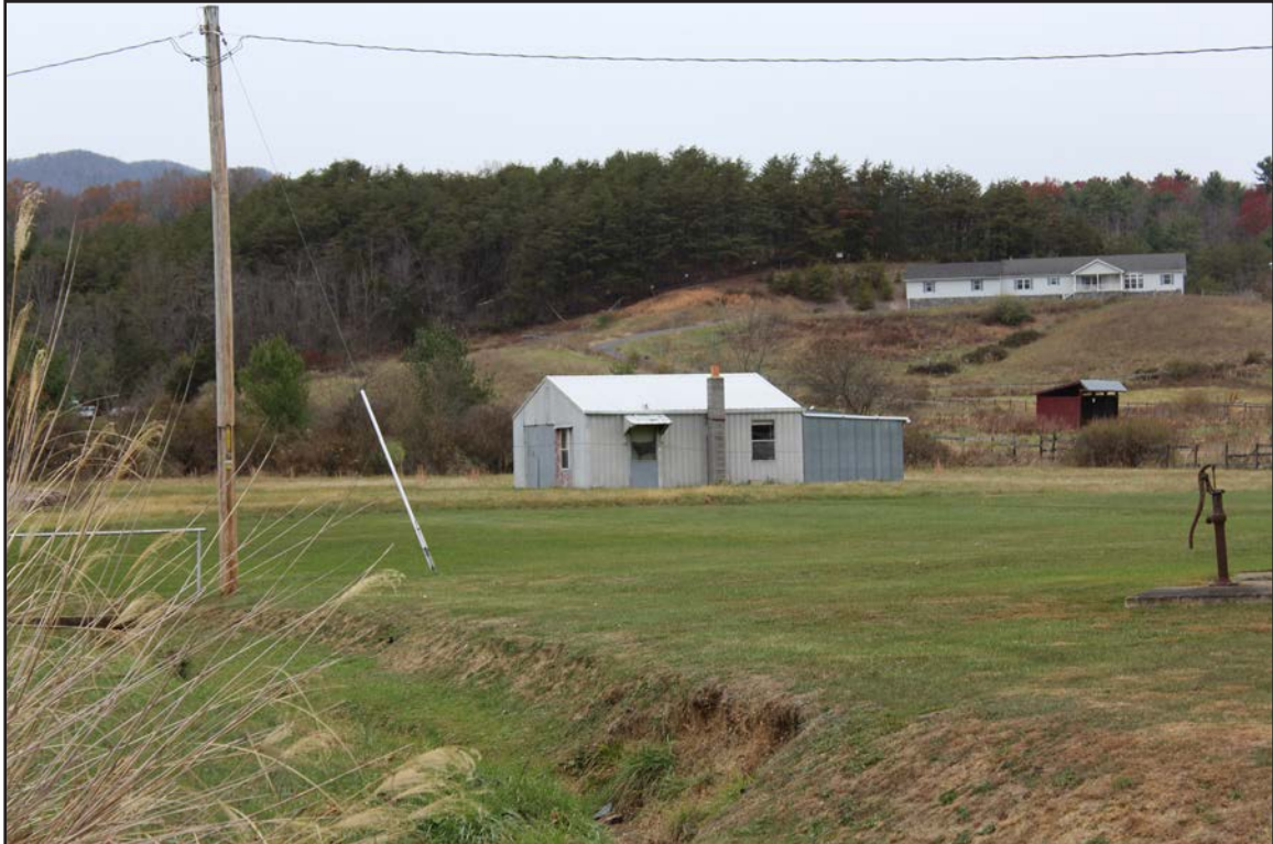
Figure 186. 007-5736, outbuilding, facing northeast.
