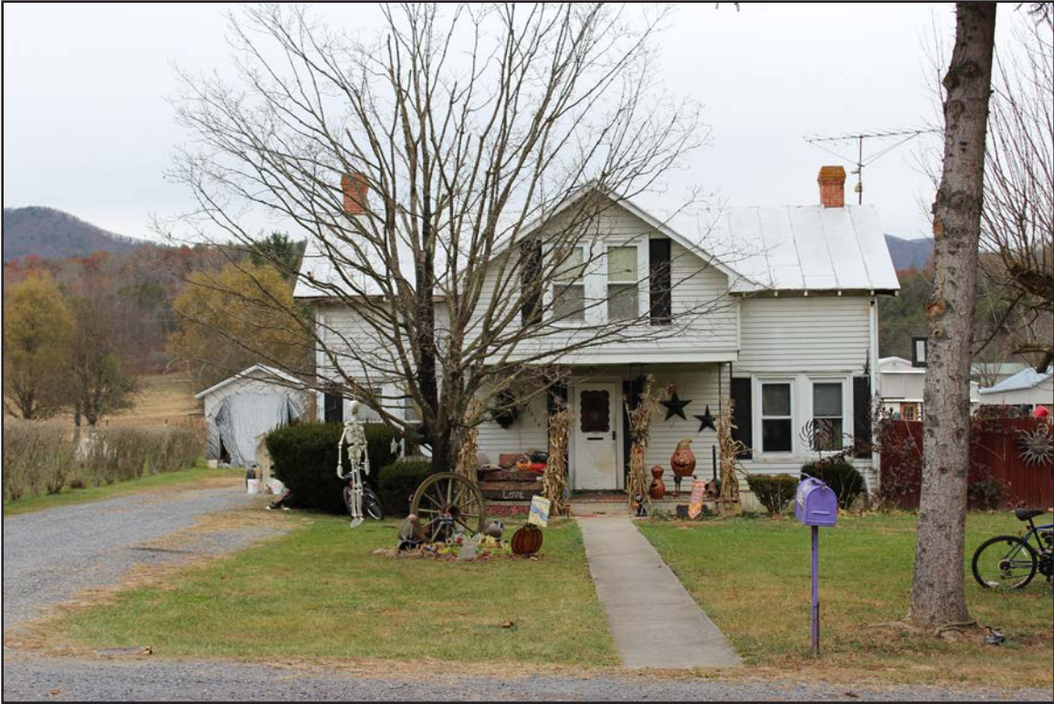
Figure 173. 007-5733, house, facing north-northwest.
