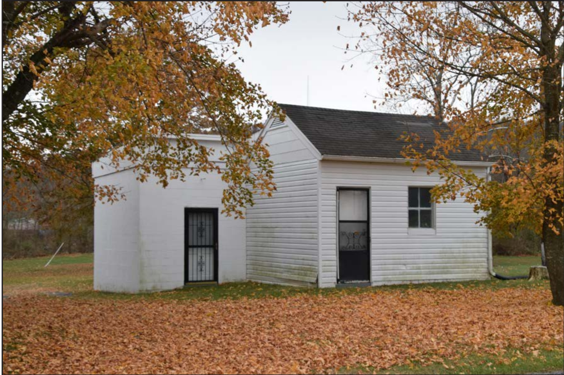
Figure 120. 007-5721, building, facing southeast.
