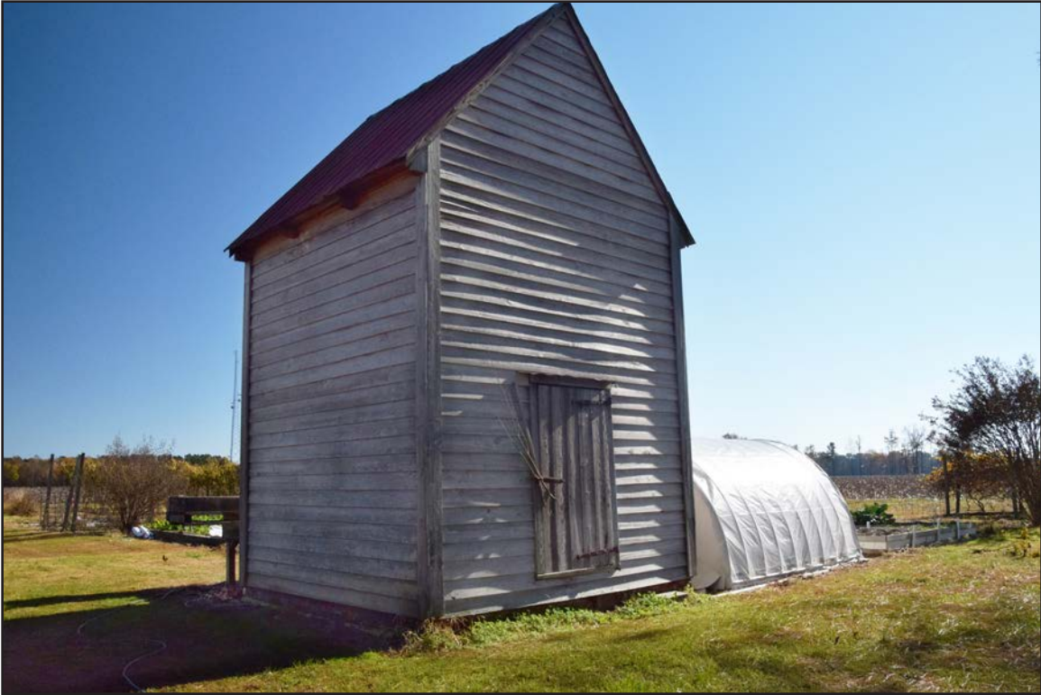
Figure 269. 133-0101, smokehouse, facing south.
