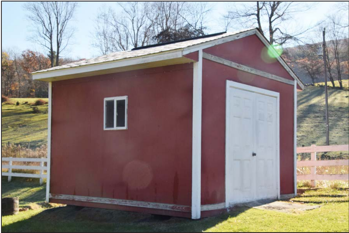
Figure 59. 007-5709, Outbuilding 3, facing southwest.
