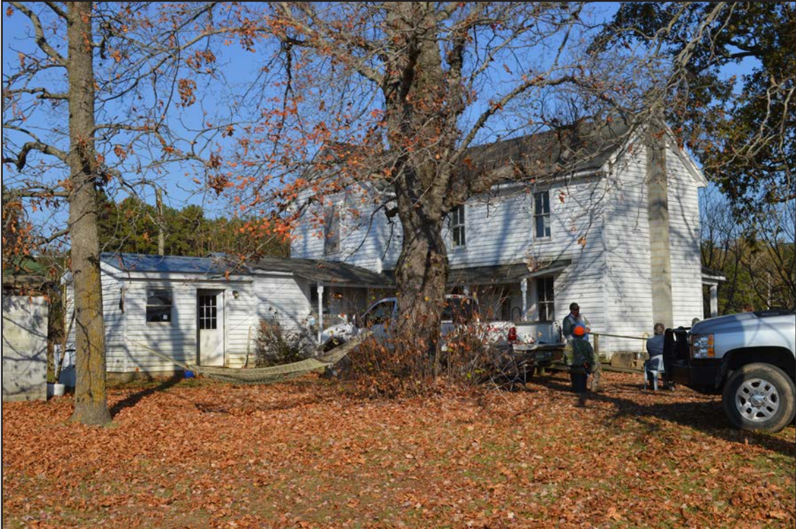
Figure 234. 014-5085, house, facing northeast.
