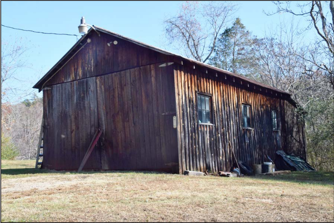
Figure 257. 062-5223, garage, facing southeast.
