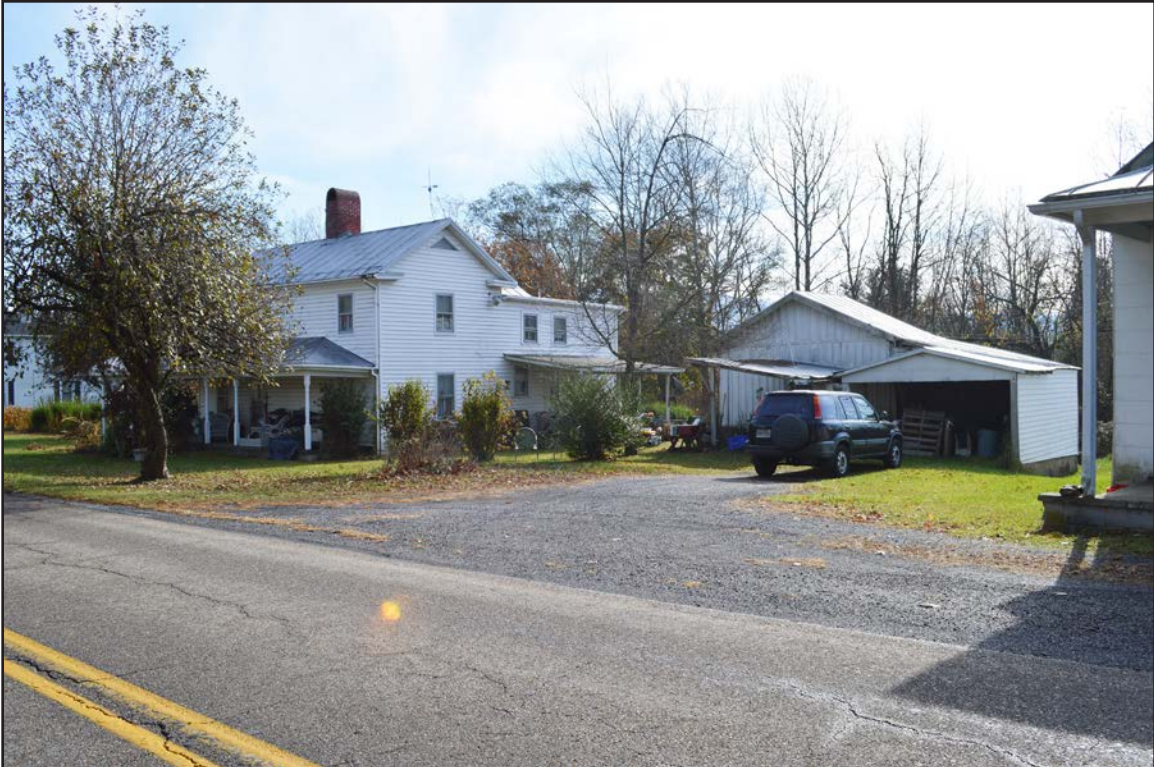
Figure 18. 007-0476, dwelling house, facing southwest.
