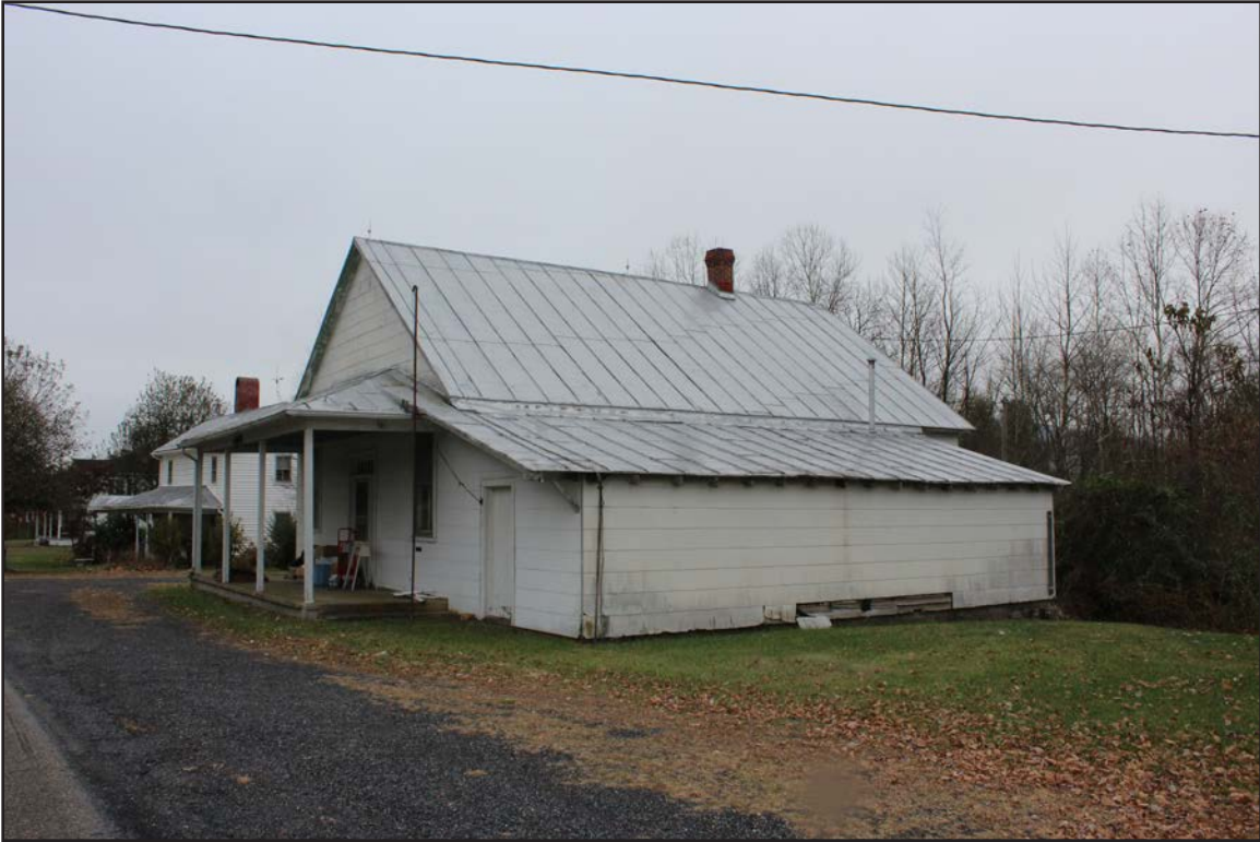
Figure 17. 007-0476, store, facing southeast.
