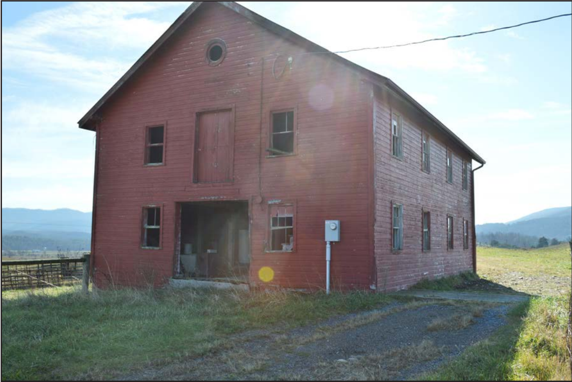
Figure 7. 007-0463, Barn 1, facing south.
