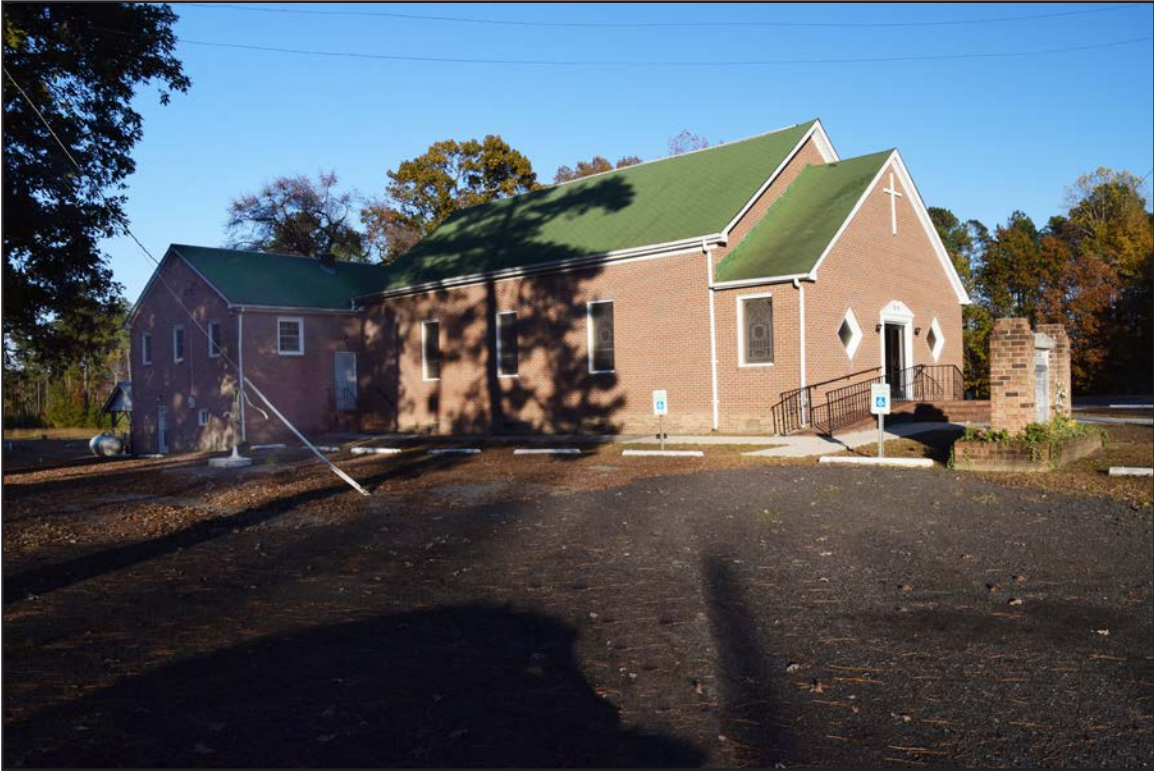
Figure 247. 026-5257, church, facing northeast.
