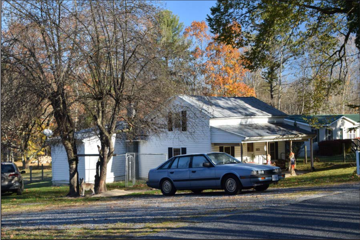
Figure 85. 007-5715, house, facing northeast.
