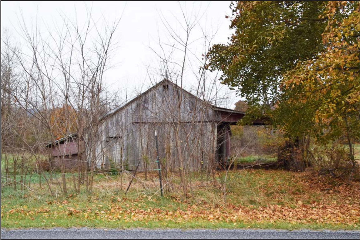
Figure 123. 007-5722, Barn 1, facing south.
