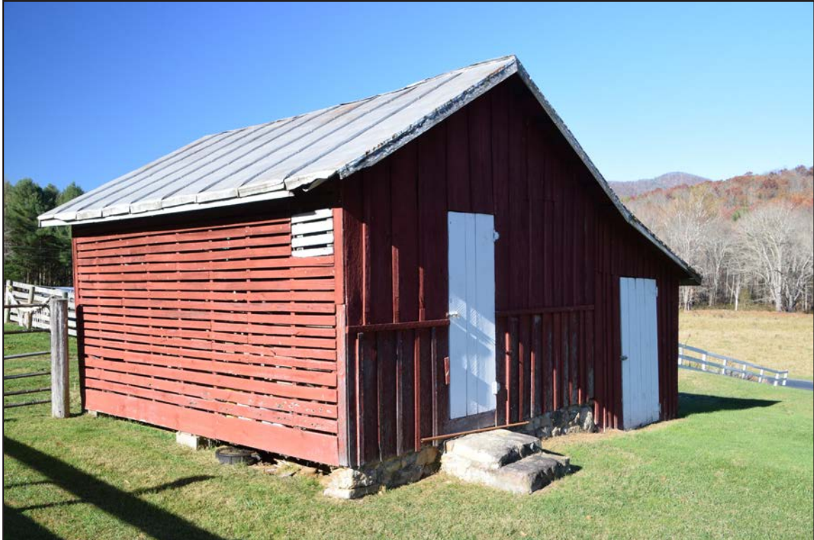
Figure 60. 007-5709, Outbuilding 4, facing southwest.
