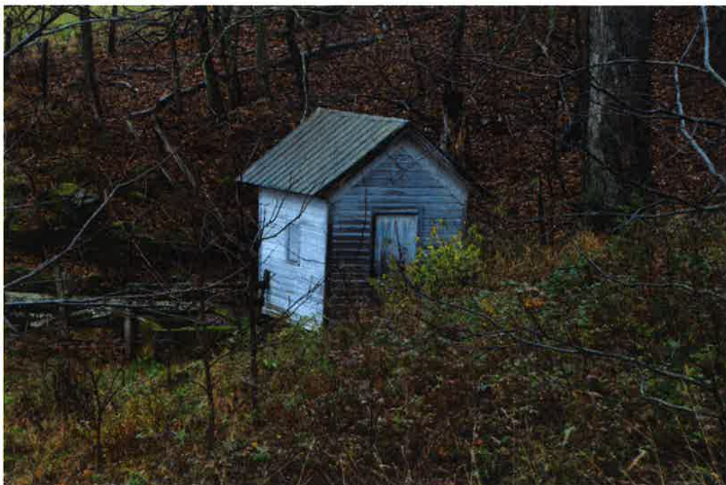
PH-0903, Well House, facing southeast.
