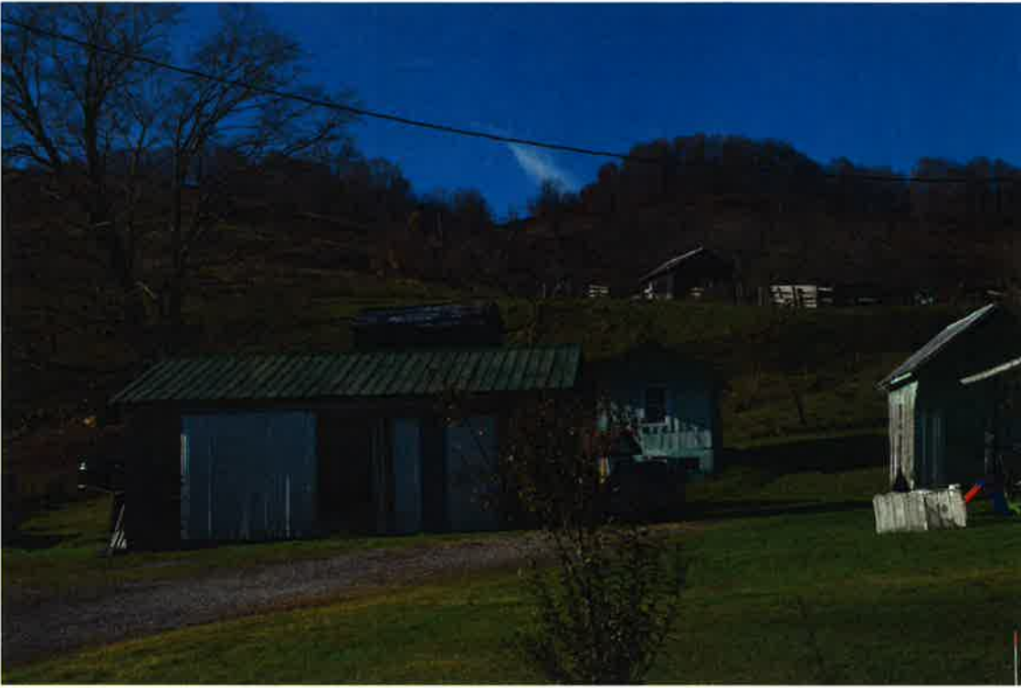
RD-0911, Shed 1, facing southwest.
