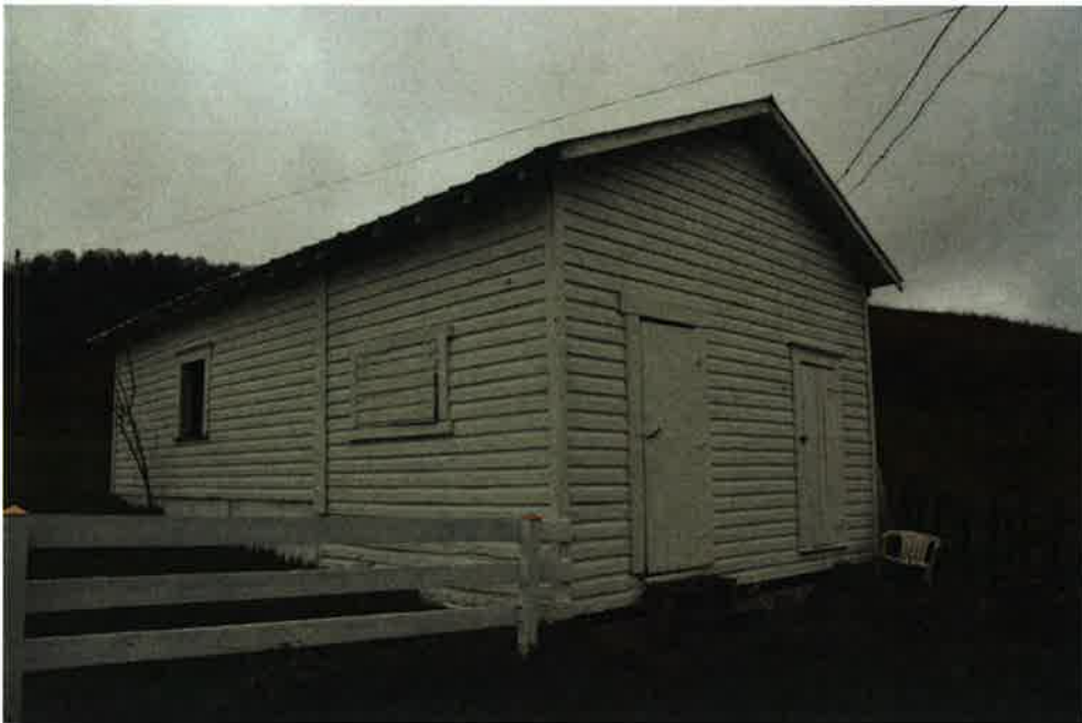
PH-0903, Outbuilding 1, facing north.
