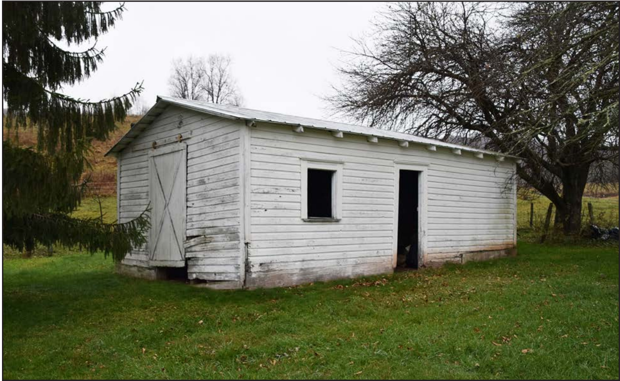
Photo 19. PH-0904, Outbuilding, facing northwest.
