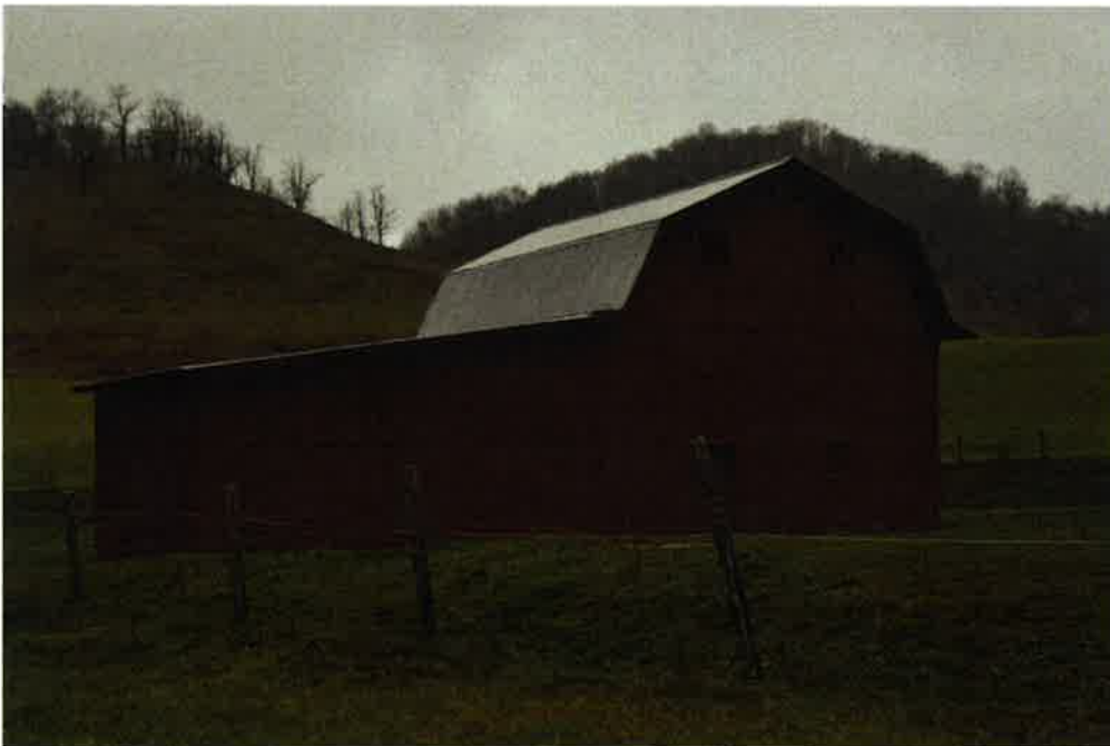
PH-0903, Barn 3, facing southwest.
