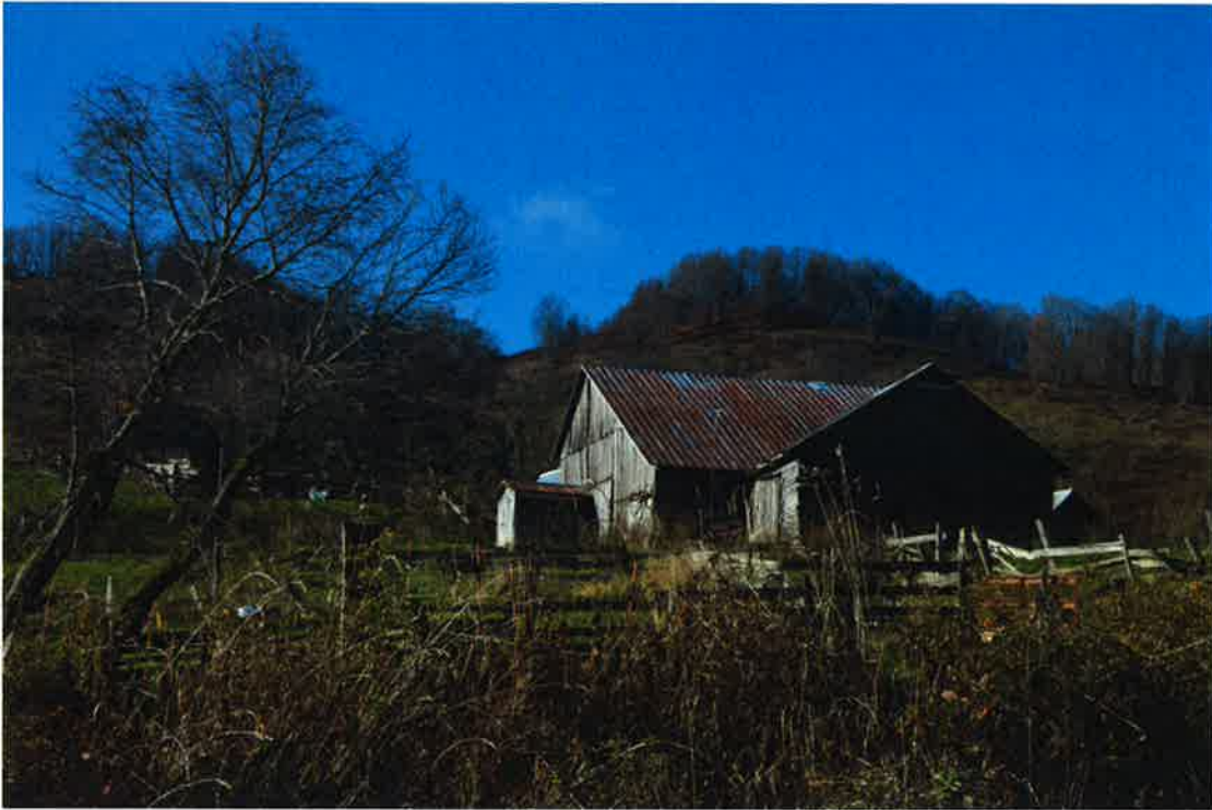
RD-0911, Barn 3 and Barn 4, facing west.
