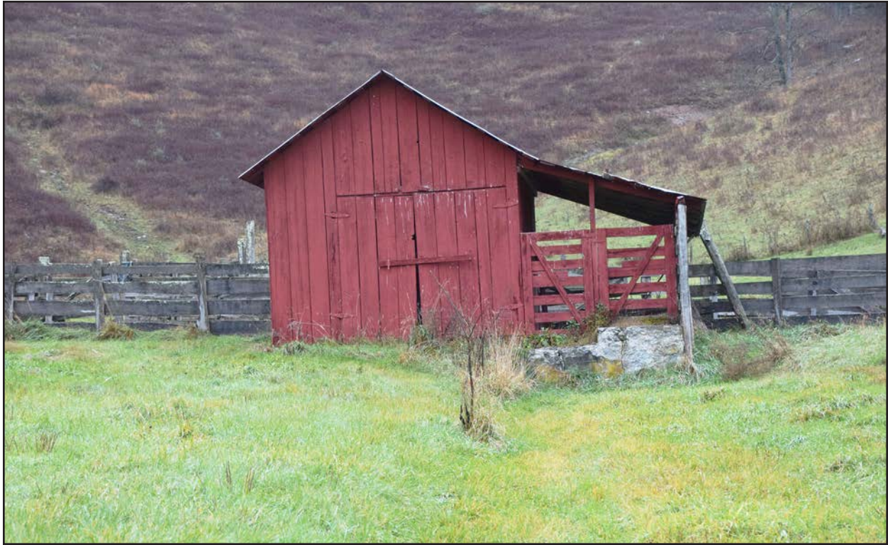
Photo 9. PH-0903, Barn 2, facing west.
