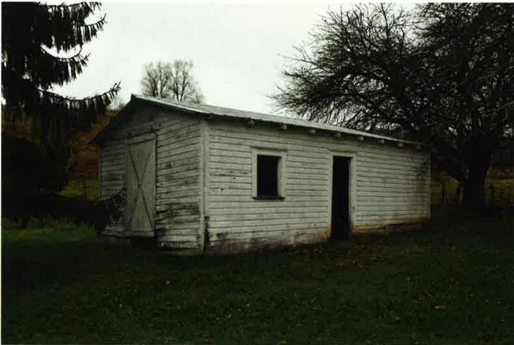
PH-0904, Outbuilding, facing northwest.
