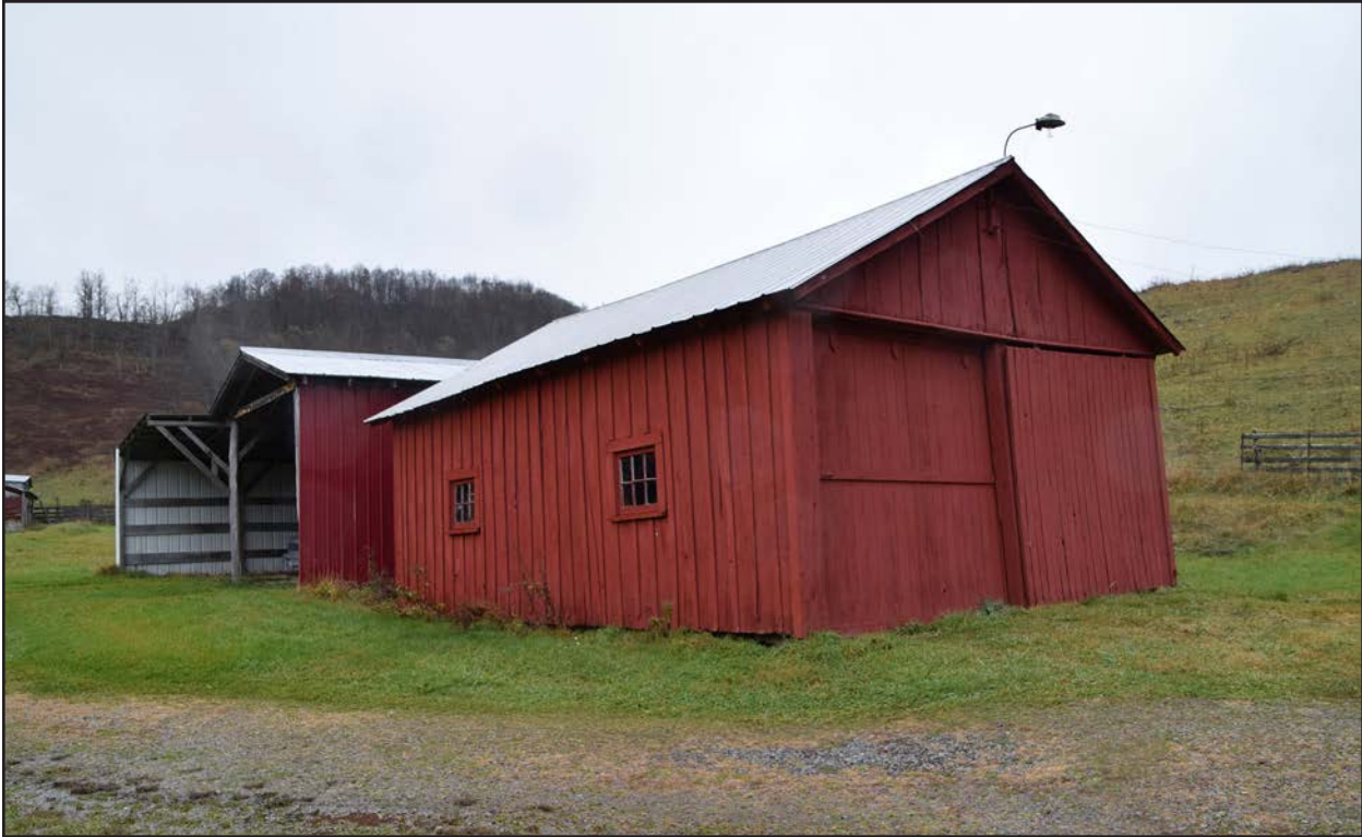
Photo 8. PH-0903, Barn 1 and Shed 5, facing northwest
