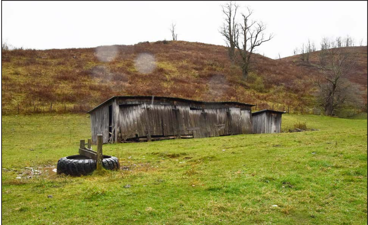
Photo 12. PH-0903, Shed 1 and 2, facing northwest.
