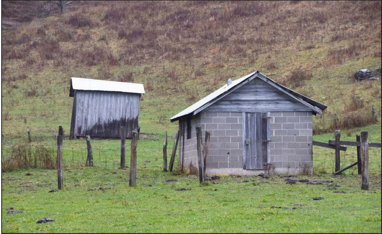
Photo 11. PH-0903, Outbuilding 2 and Shed 4, facing northwest.
