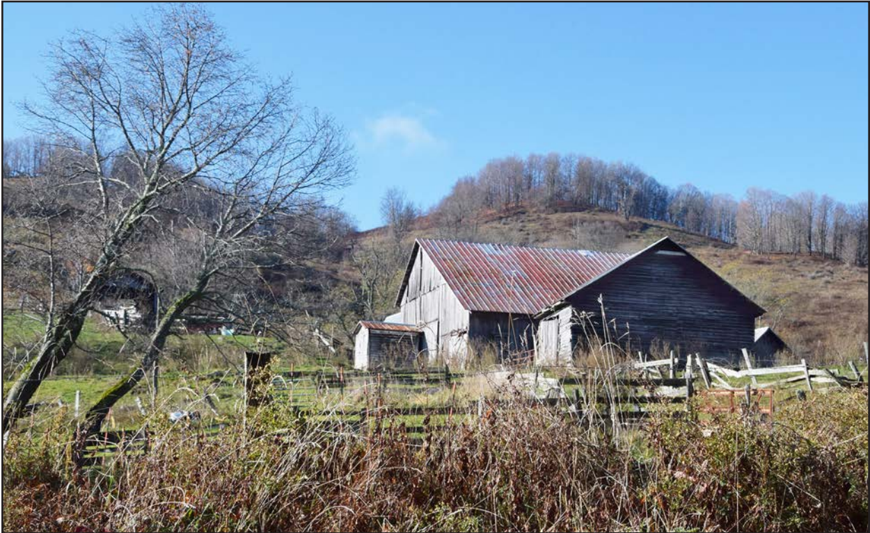
Photo 31. RD-0911, Barn 3 and Barn 4, facing west.
