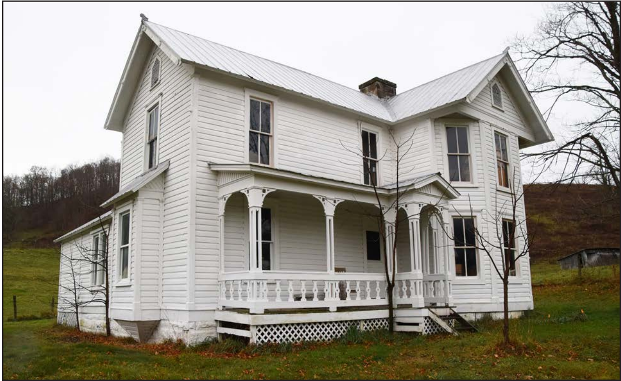
Photo 3. PH-0903, ca. 1890 house, facing west.
