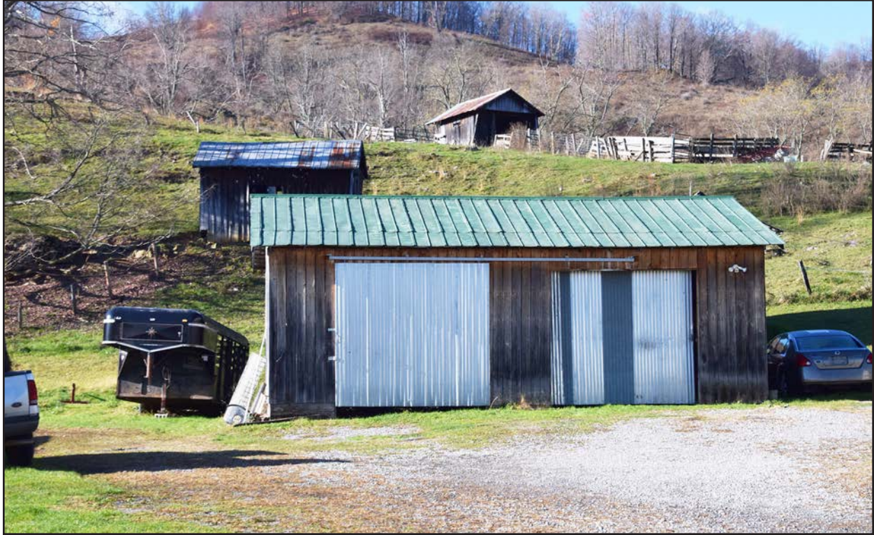
Photo 29. RD-0911, Garage, facing southwest.
