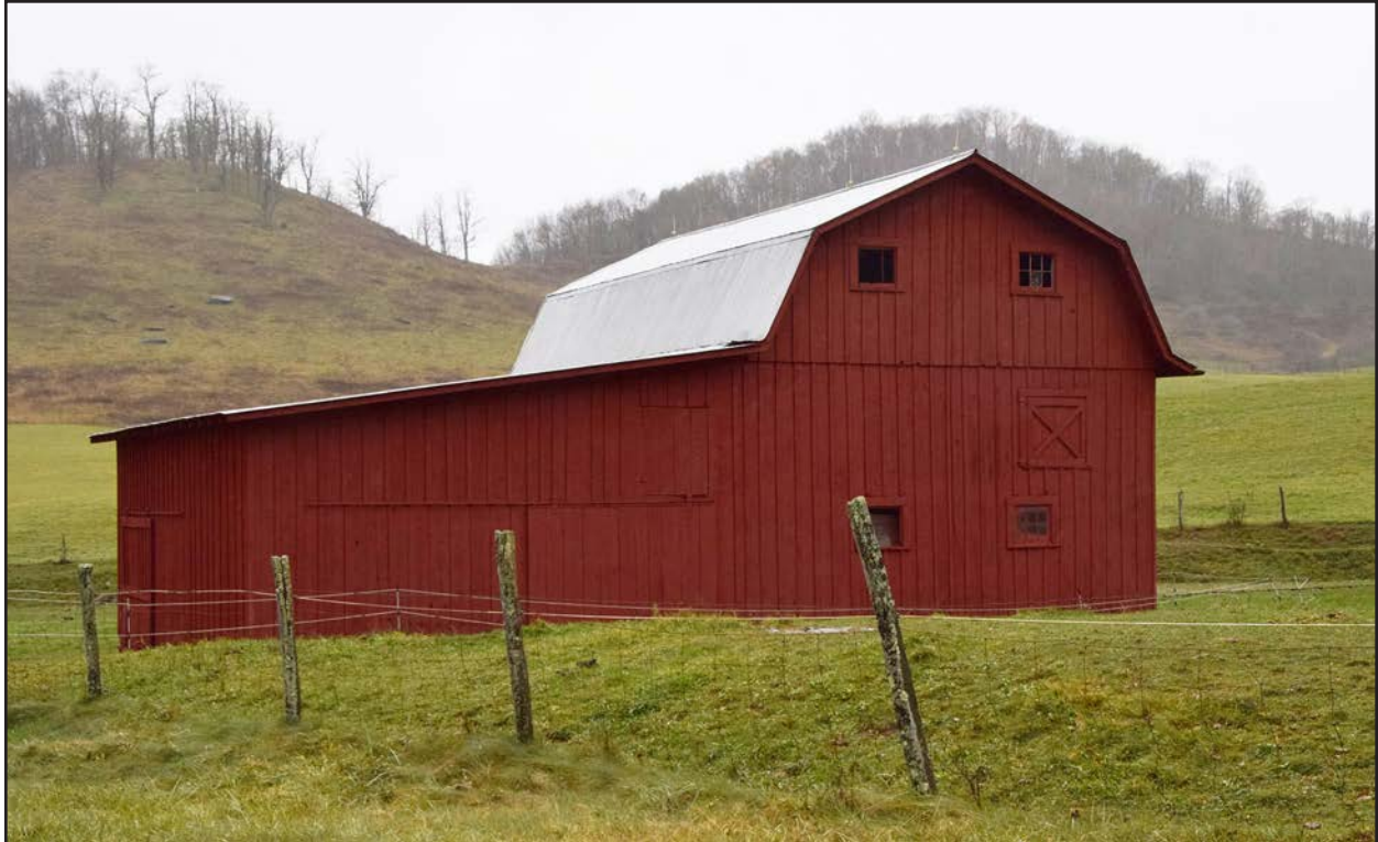
Photo 10. PH-0903, Barn 3, facing southwest.
