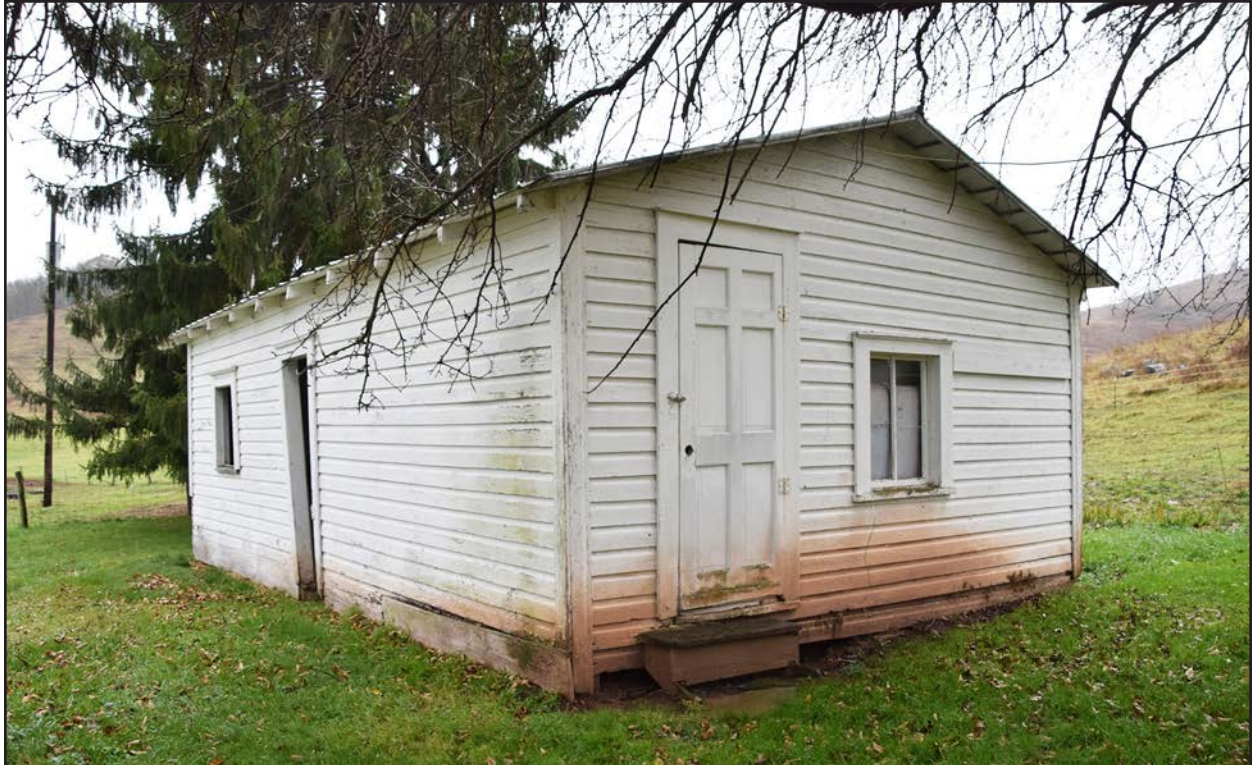
Photo 20. PH-0904, Outbuilding, facing southwest.
