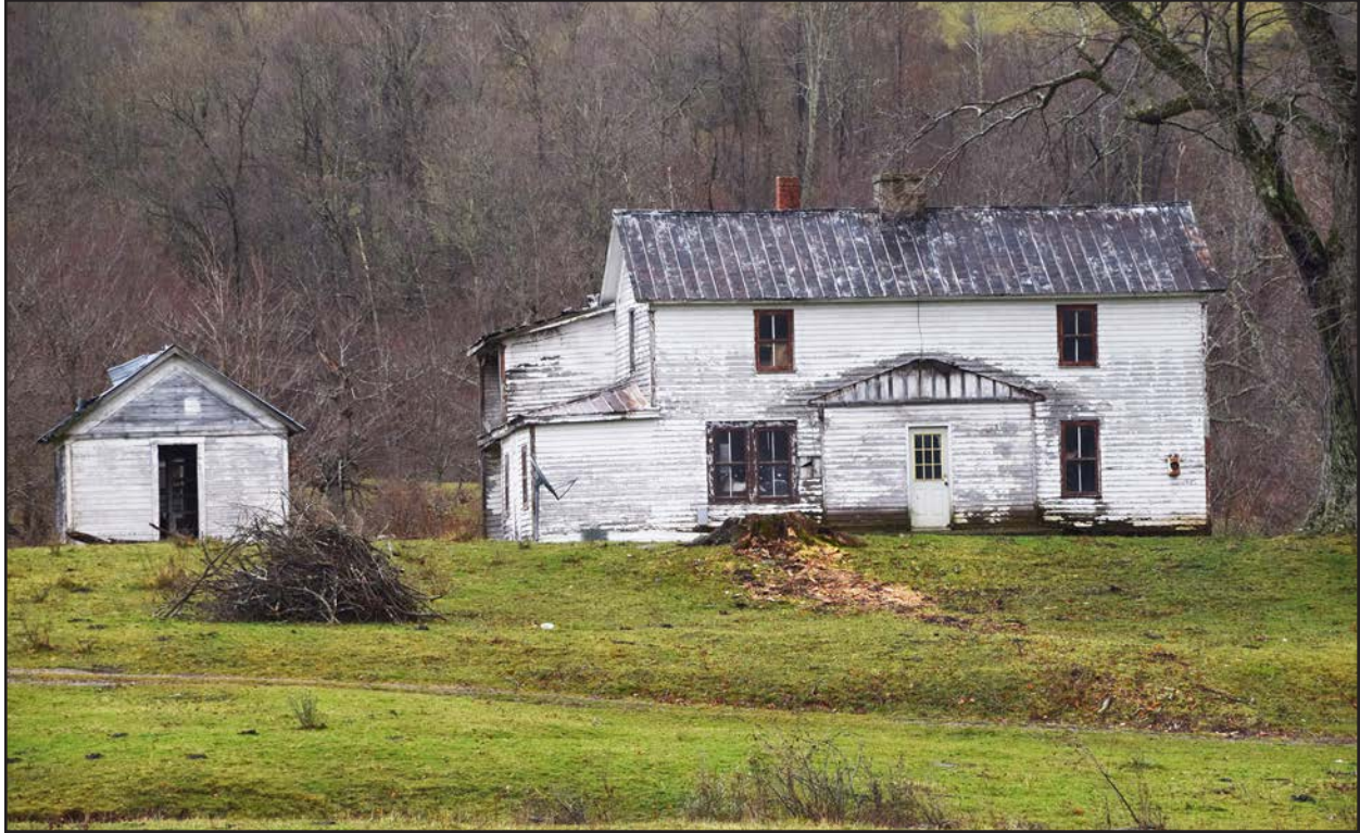
Photo 21. PH-0905, facing southwest.
