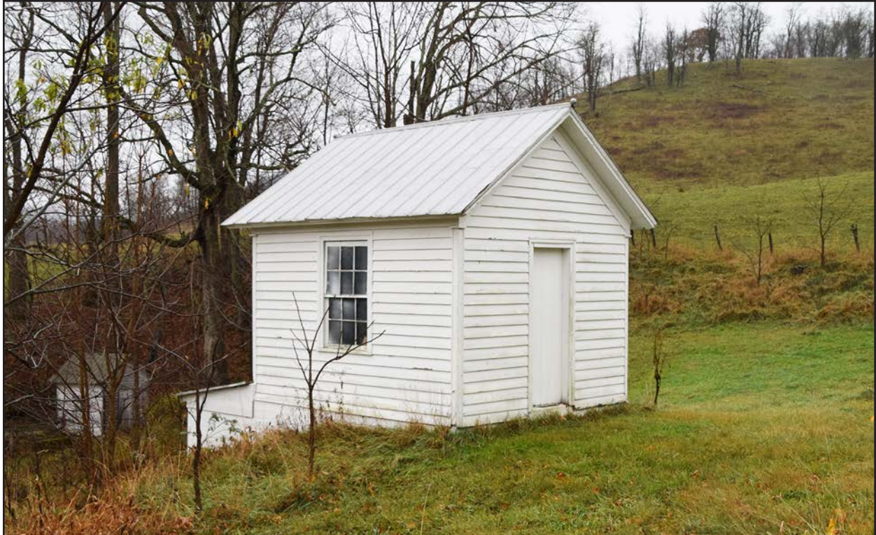
Photo 14. PH-0903, Root cellar, facing south.
