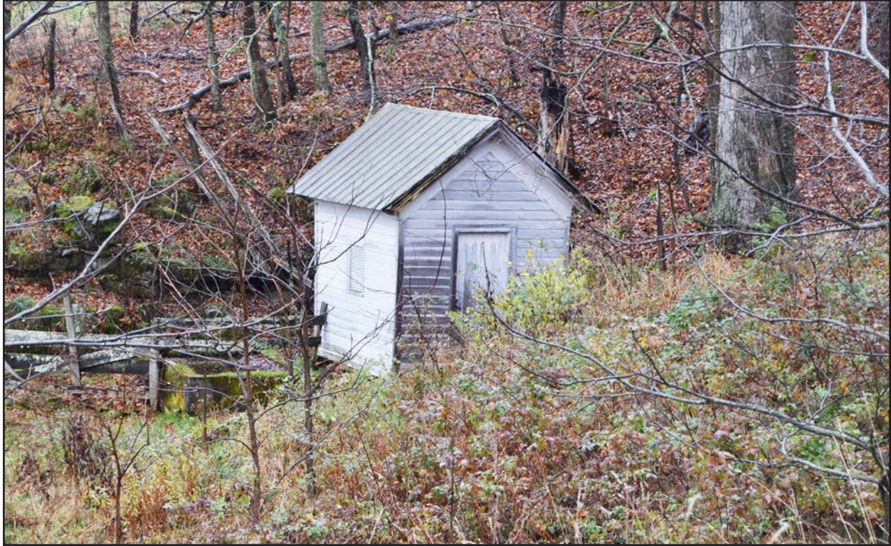
Photo 15. PH-0903, Well house, facing southeast
