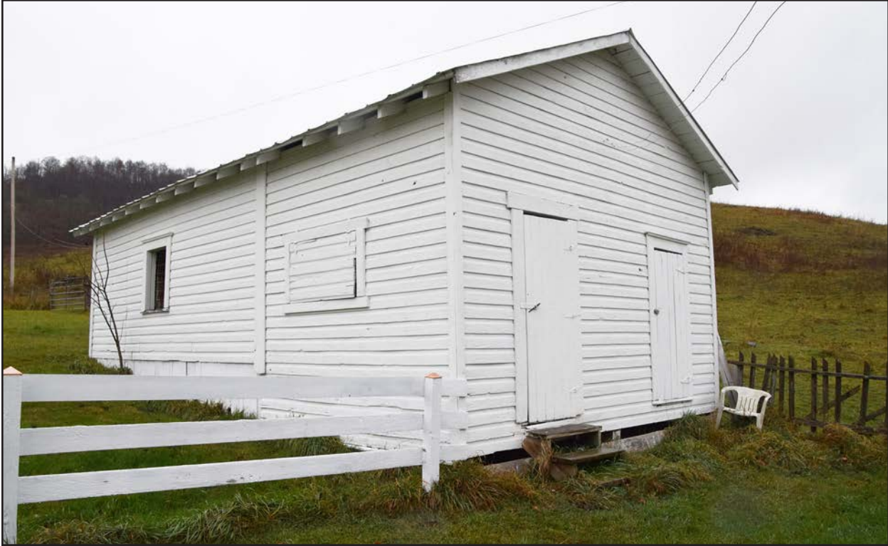
Photo 7. PH-0903, Outbuilding 1, facing north.
