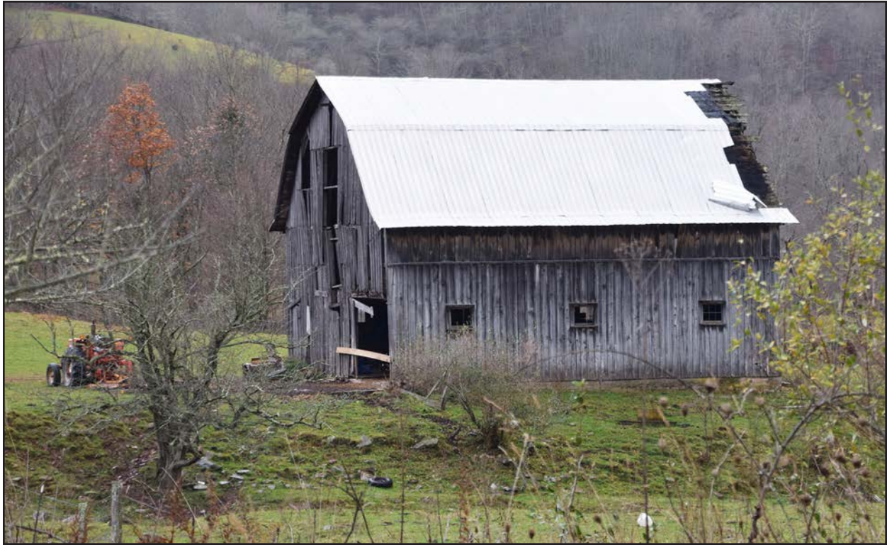
Photo 25. PH-0905, Barn, facing west.
