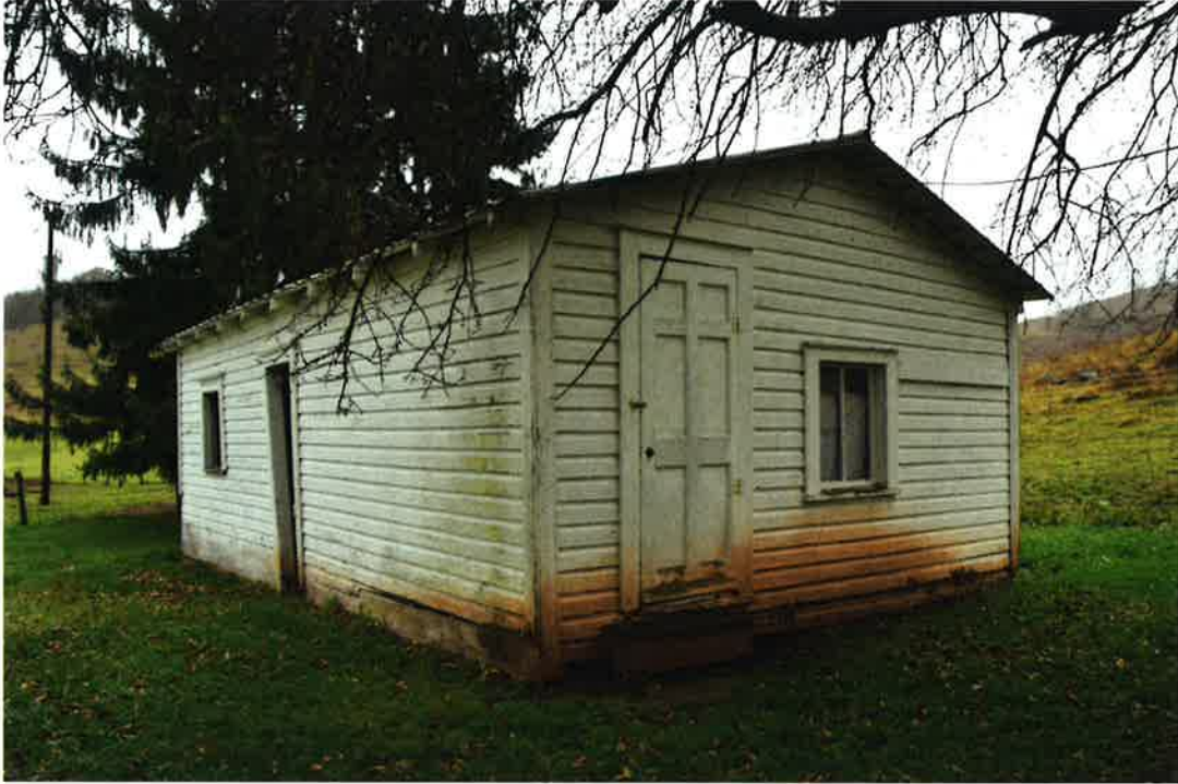
PH-0904, Outbuilding, facing southwest.
