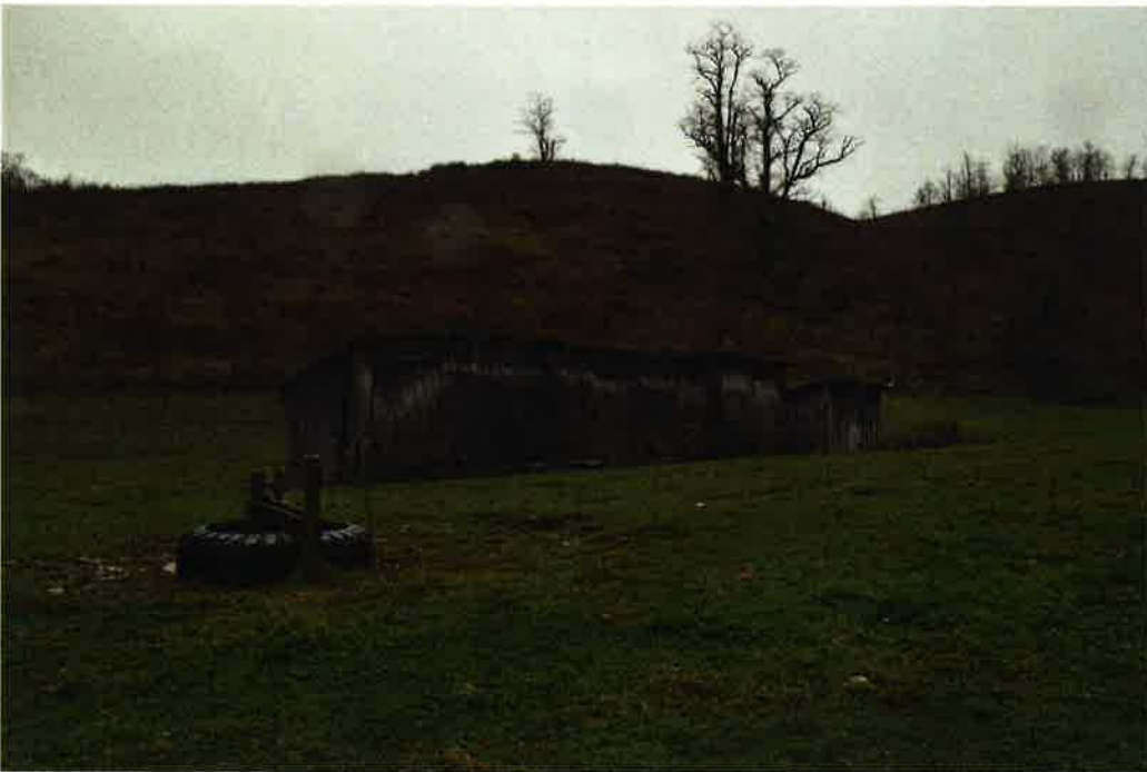
PH-0903, Shed 1 and 2, facing northwest.
