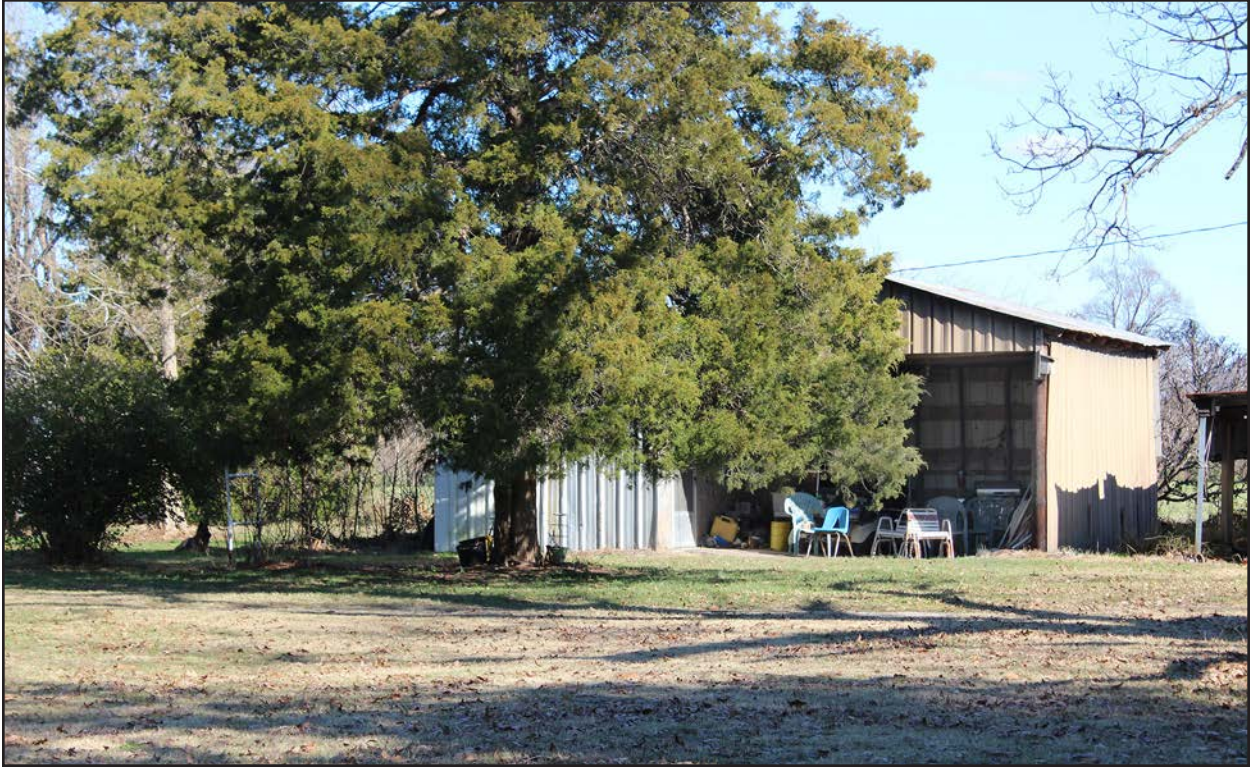
Photo 67. JT0957, storage structure, facing east-northeast.
