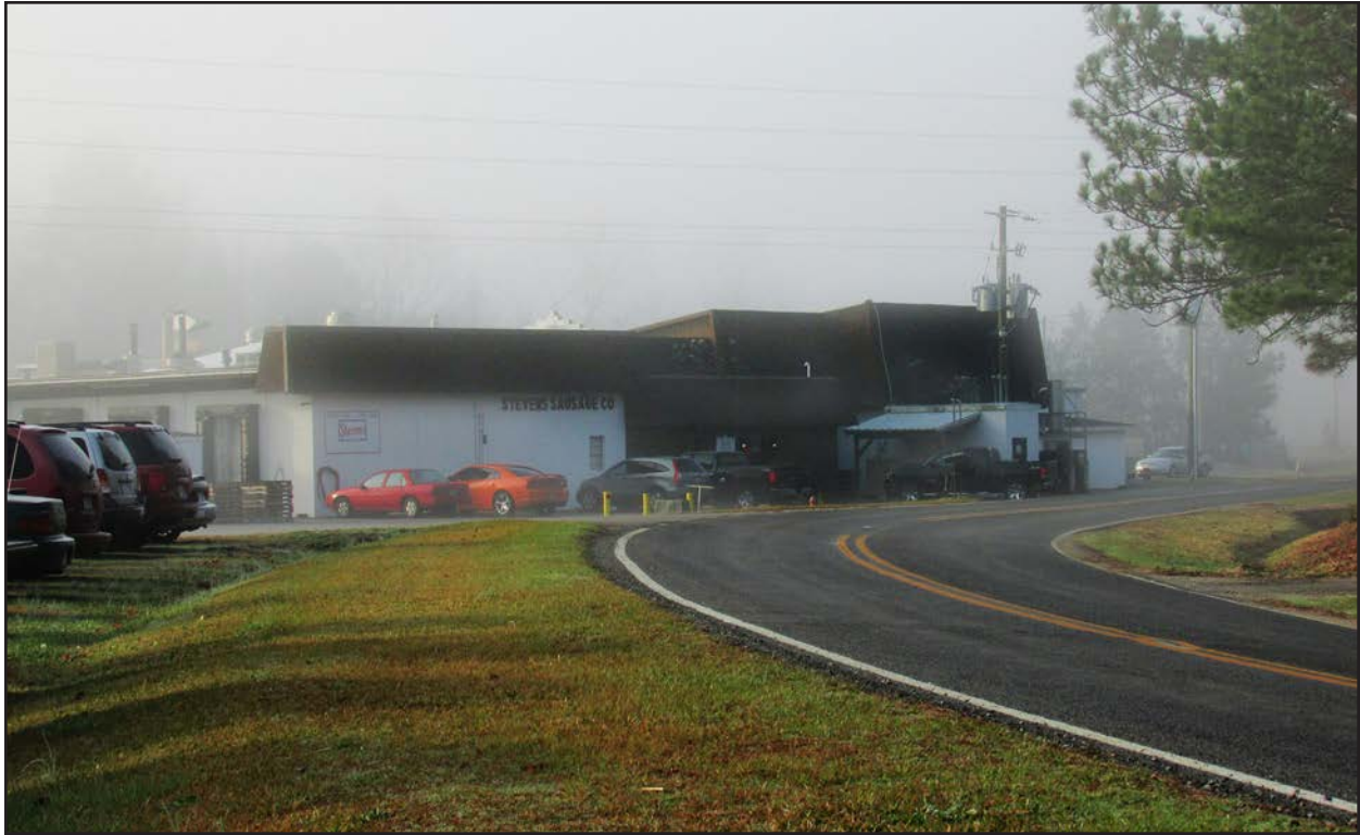
Photo 95. JT1921 (Stevens Sausage Company plant), facing south.
