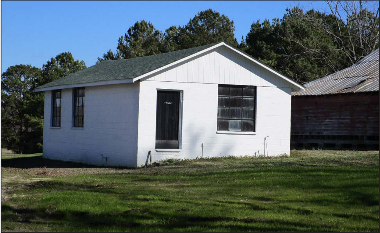
Photo 13. HX0021, milking barn, facing northeast.
