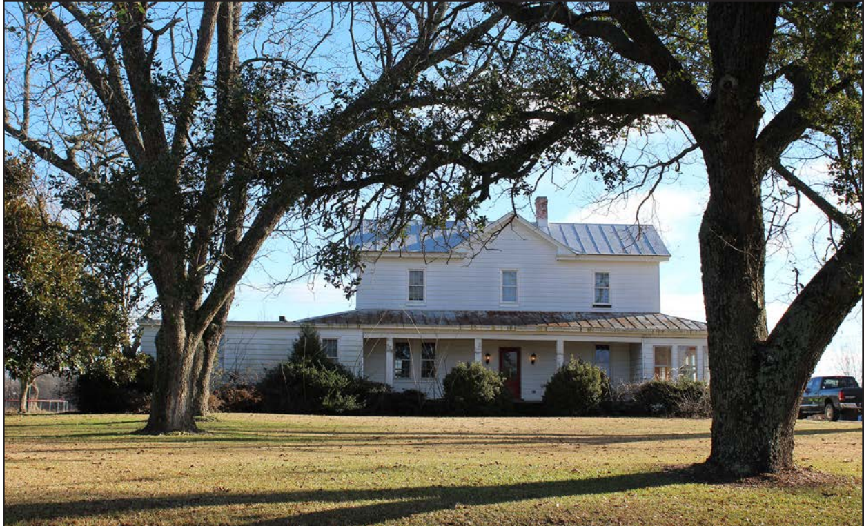
Photo 26. HX0227, main house, facing east.
