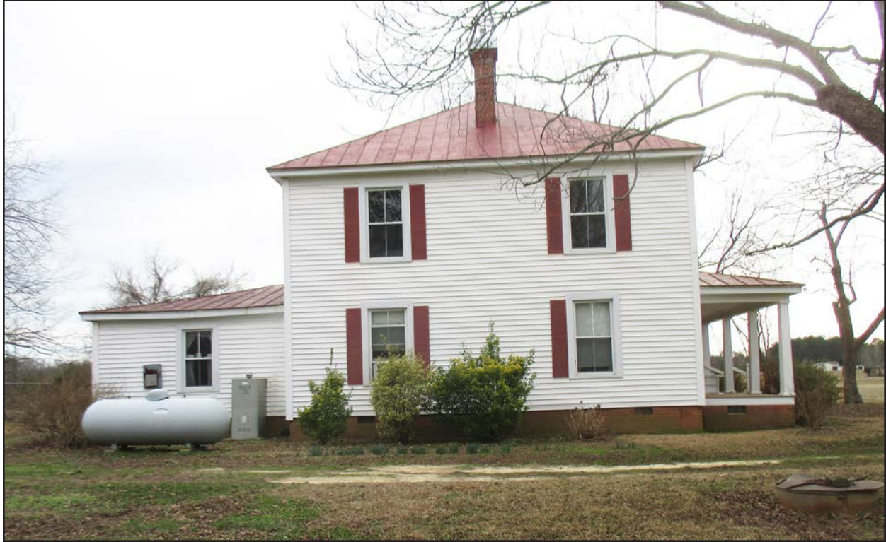
Photo 127. NS0650, house, facing south.
