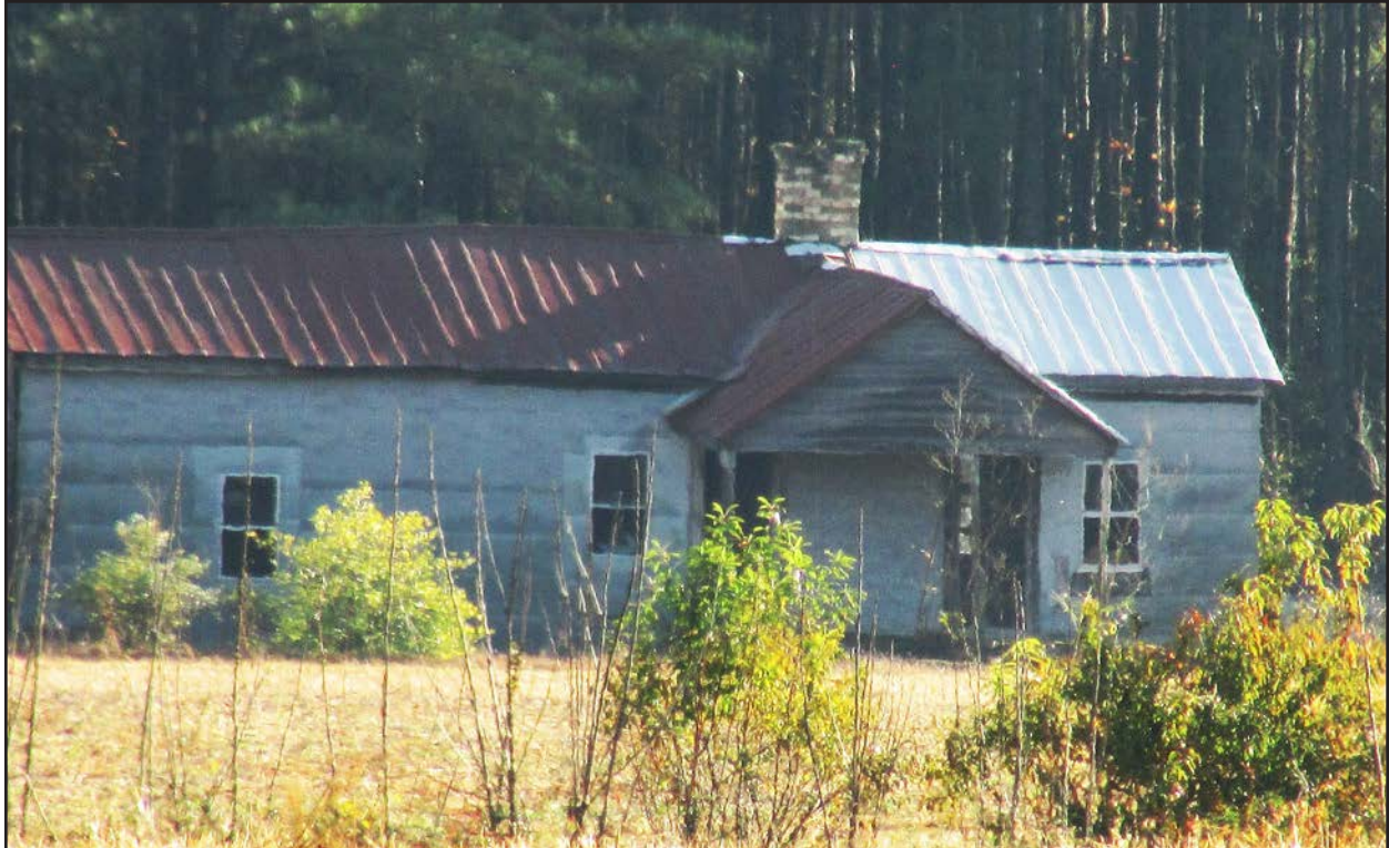
Photo 172. RB0680, house, porch detail.
