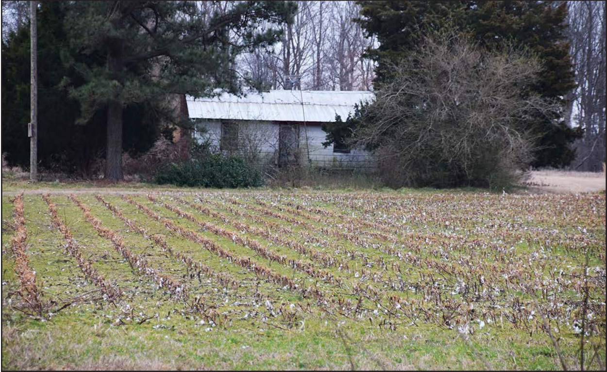
Photo 55. HX1590, facing south.
