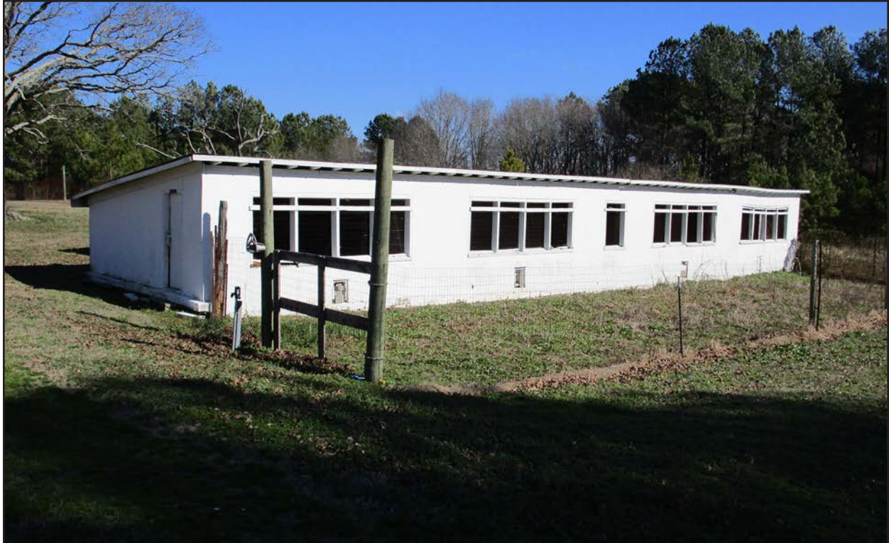
Photo 16. HX0021, chicken house, facing east.
