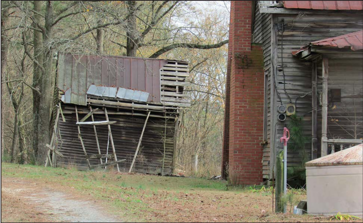
Photo 116. JT1937, accessory structure facing east.
