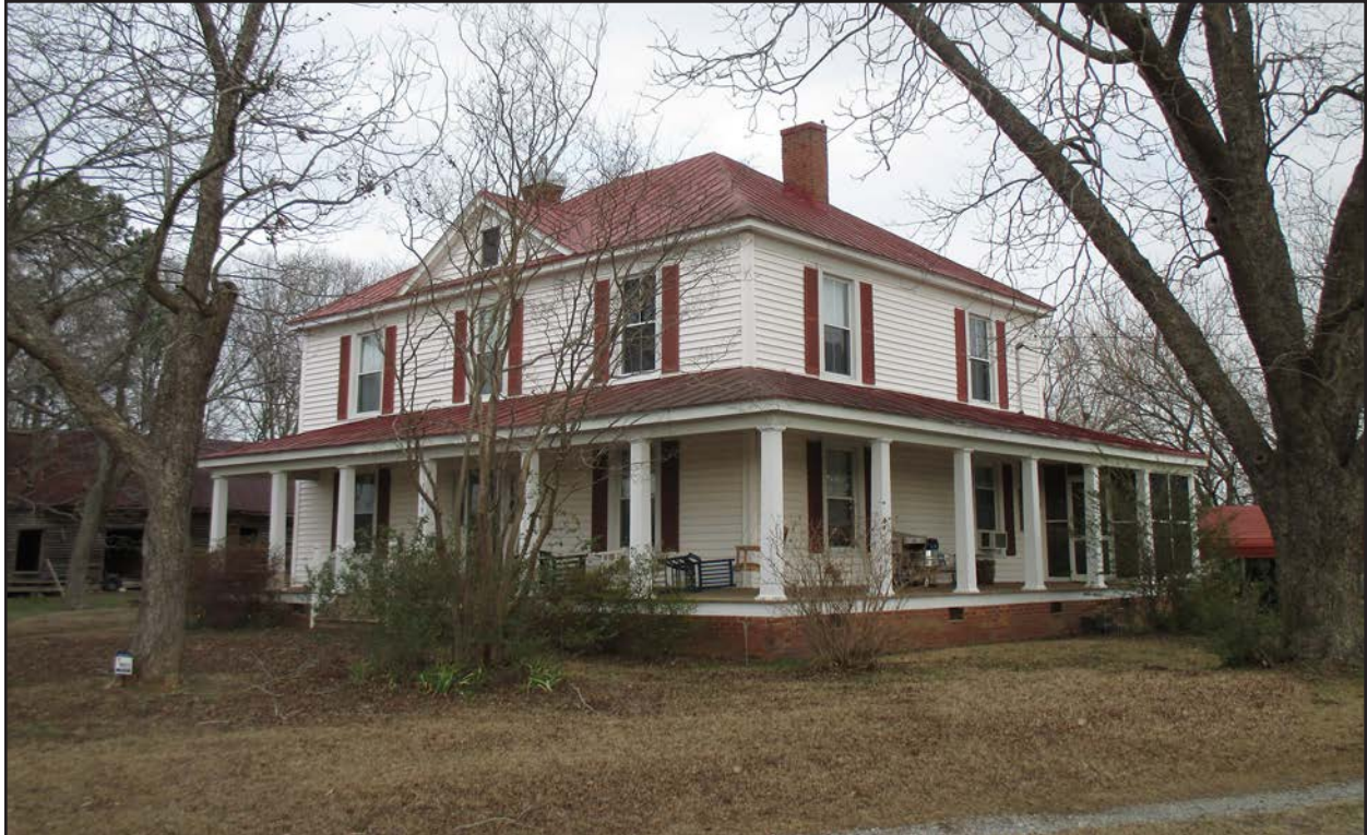
Photo 124. NS0650, house, facing northeast.
