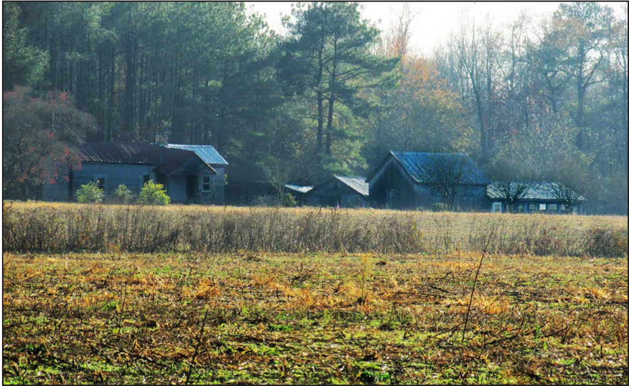
Photo 173. RB0680, agricultural outbuildings, facing south.
