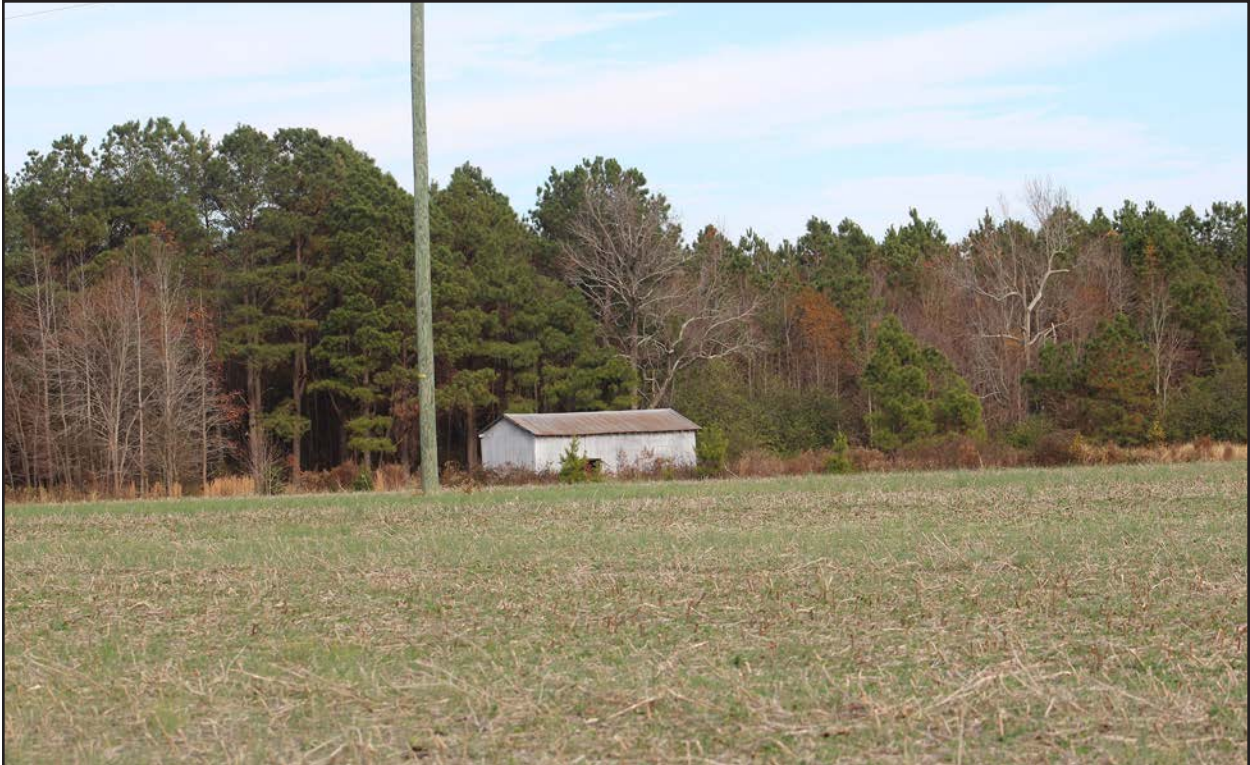
Photo 86. JT1913, storage structure, facing northeast.
