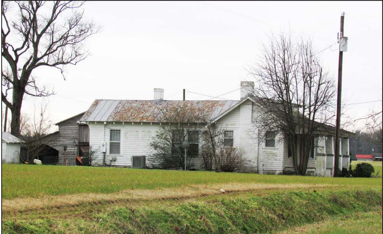
Photo 162. NS1517, dwelling, facing southwest.
