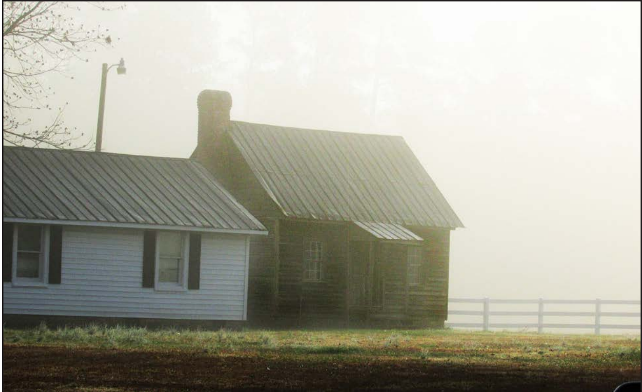
Photo 92. JT1920, log cabin, facing southeast.
