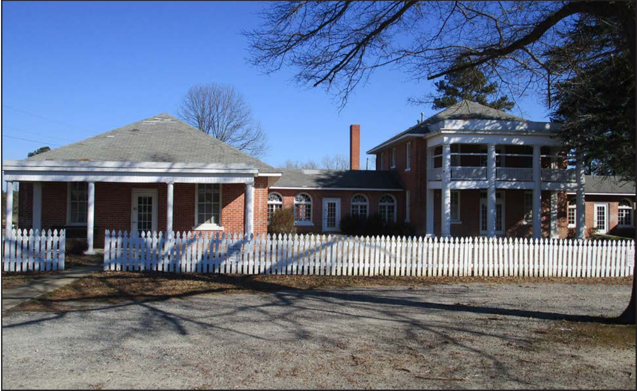
Photo 7. HX0021, facing northeast.
