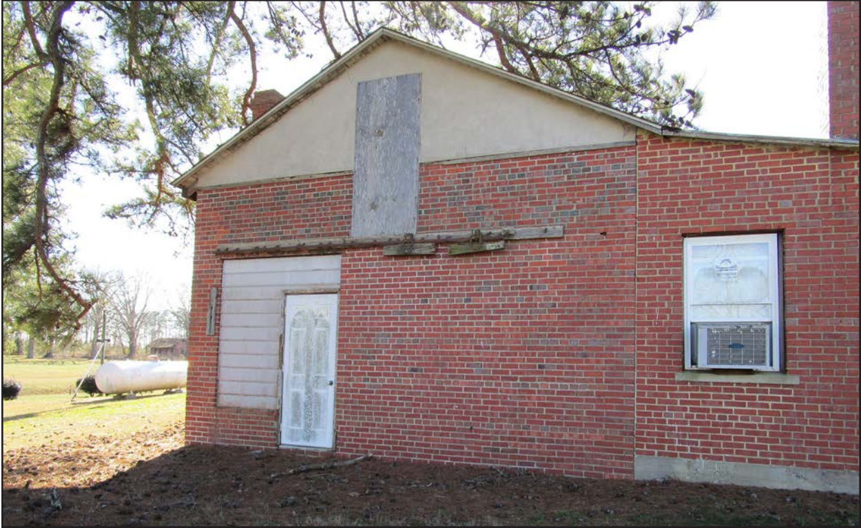
Photo 19. HX0021, barn door on smokehouse, facing south.
