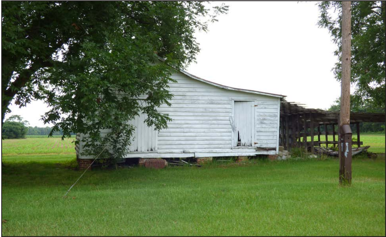
Photo 143. NS1493, agricultural outbuildings, facing north.
