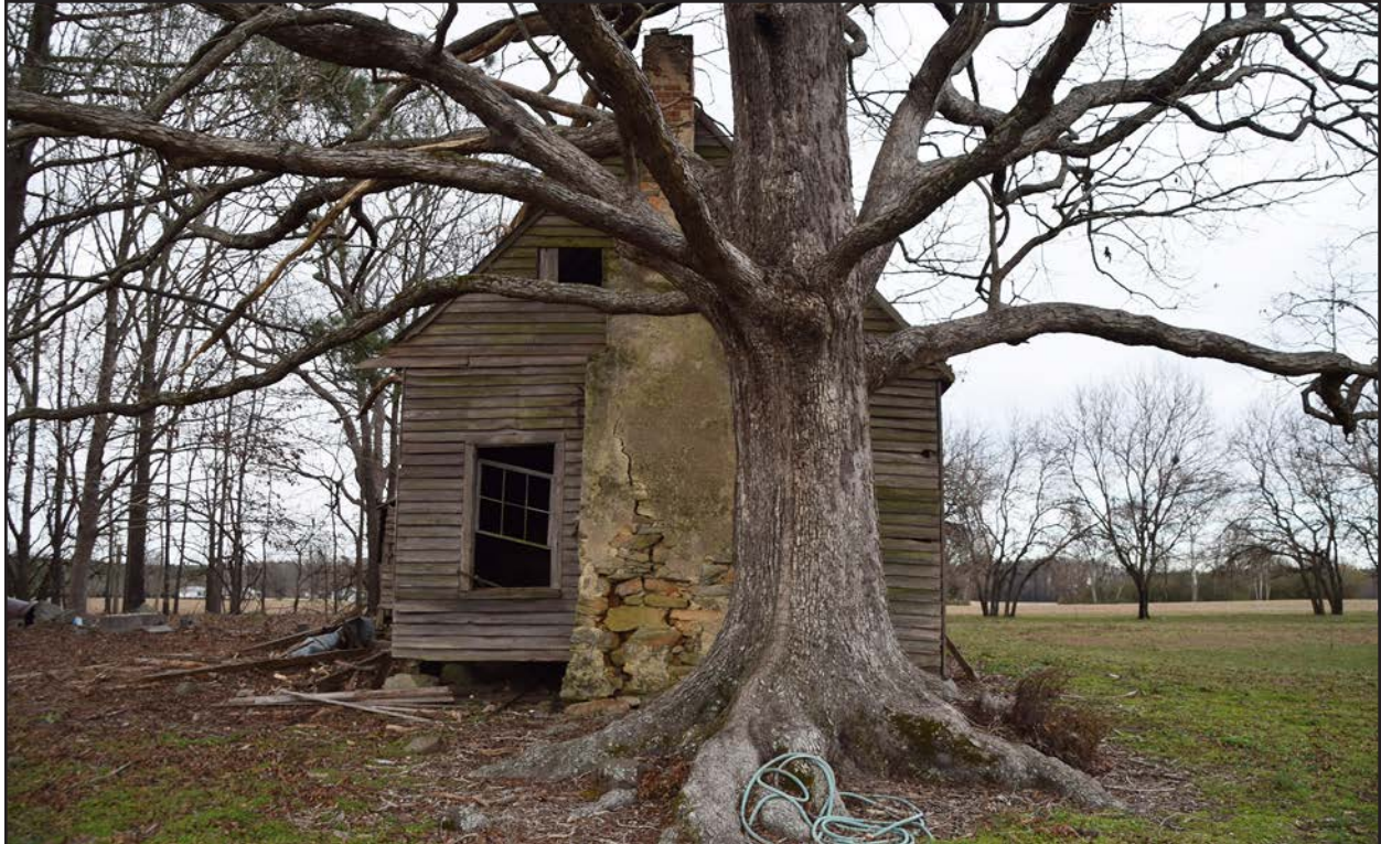
Photo 132. NS0650, cabin, facing east.
