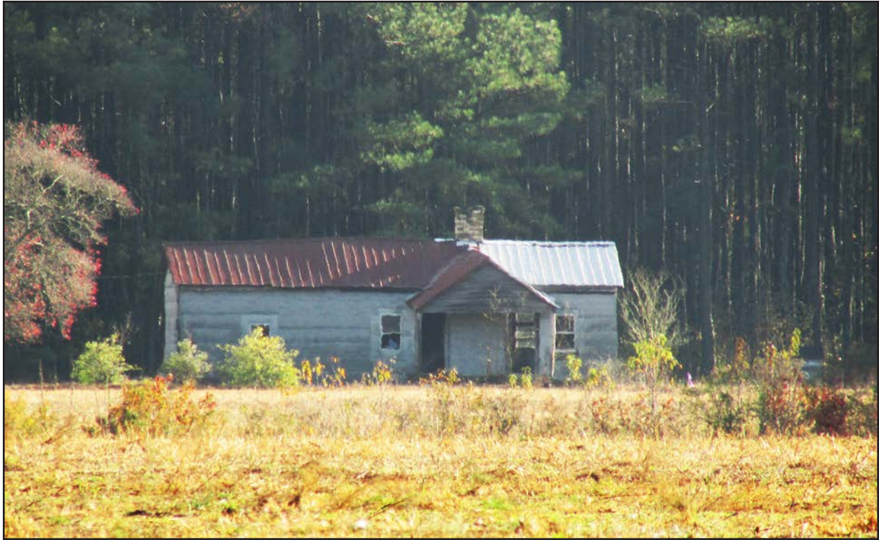
Photo 171. RB0680, house, facing southeast.
