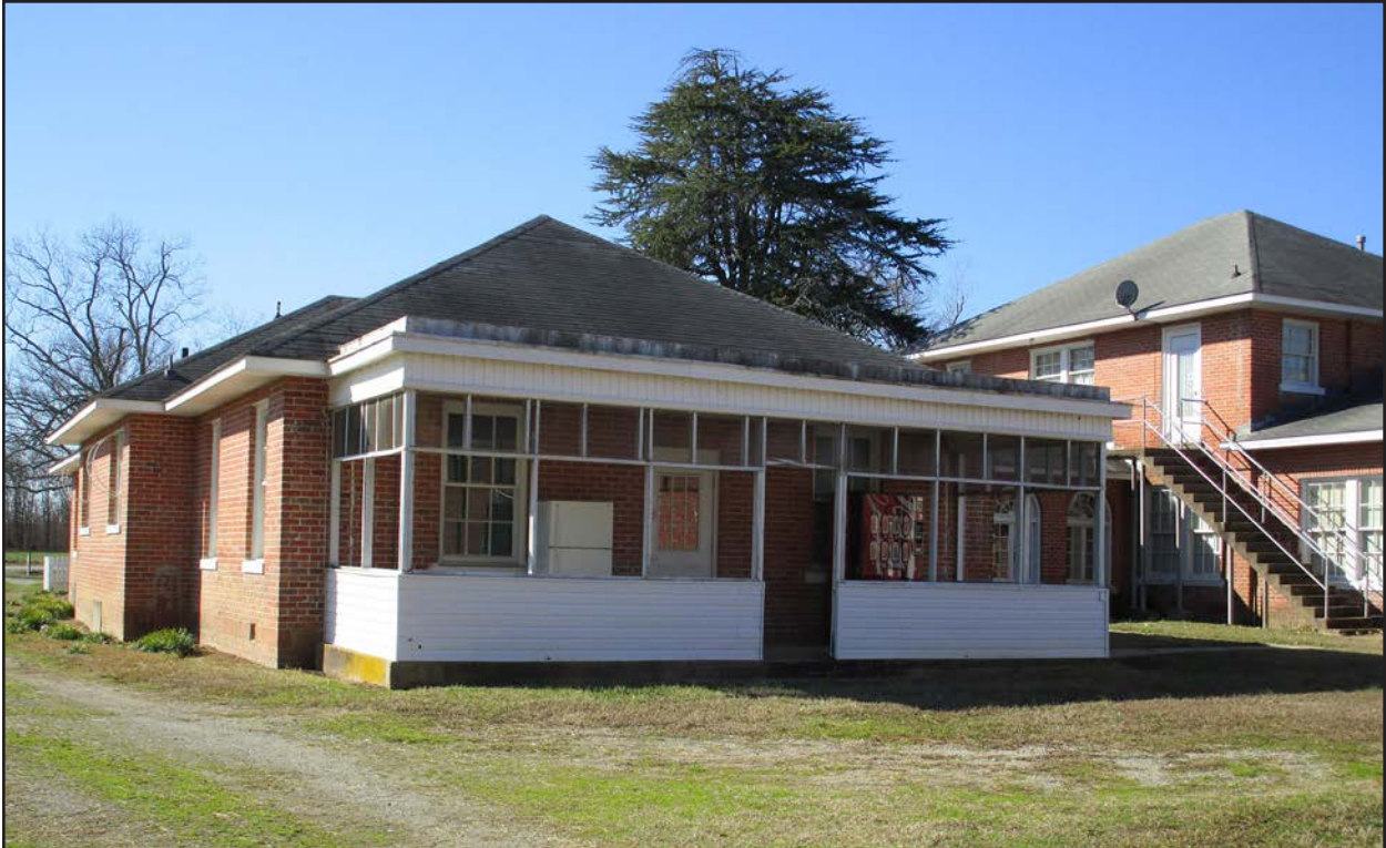
Photo 8. HX0021, facing southwest.
