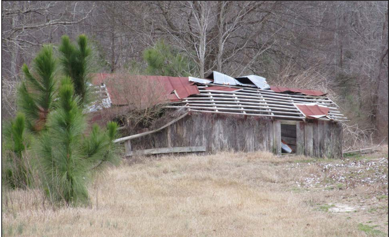
Photo 52. HX1581, storage structure, facing south.
