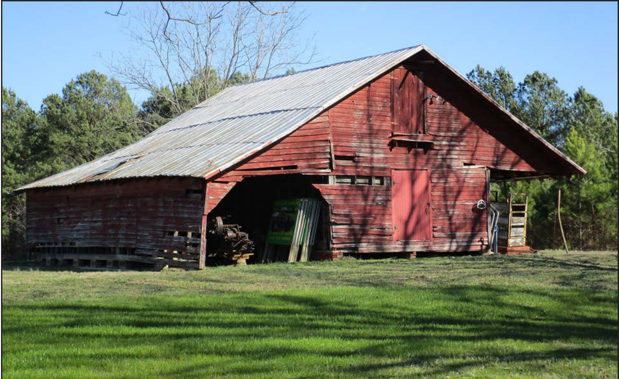
Photo 14. HX0021, corn and equipment barn, facing east-northeast.
