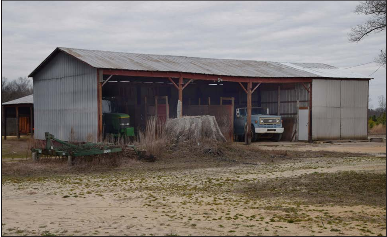
Photo 47. HX1581, garage, facing northeast.
