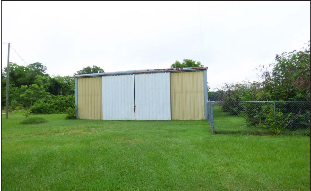
Photo 147. NS1493, metal workshop building, facing south.
