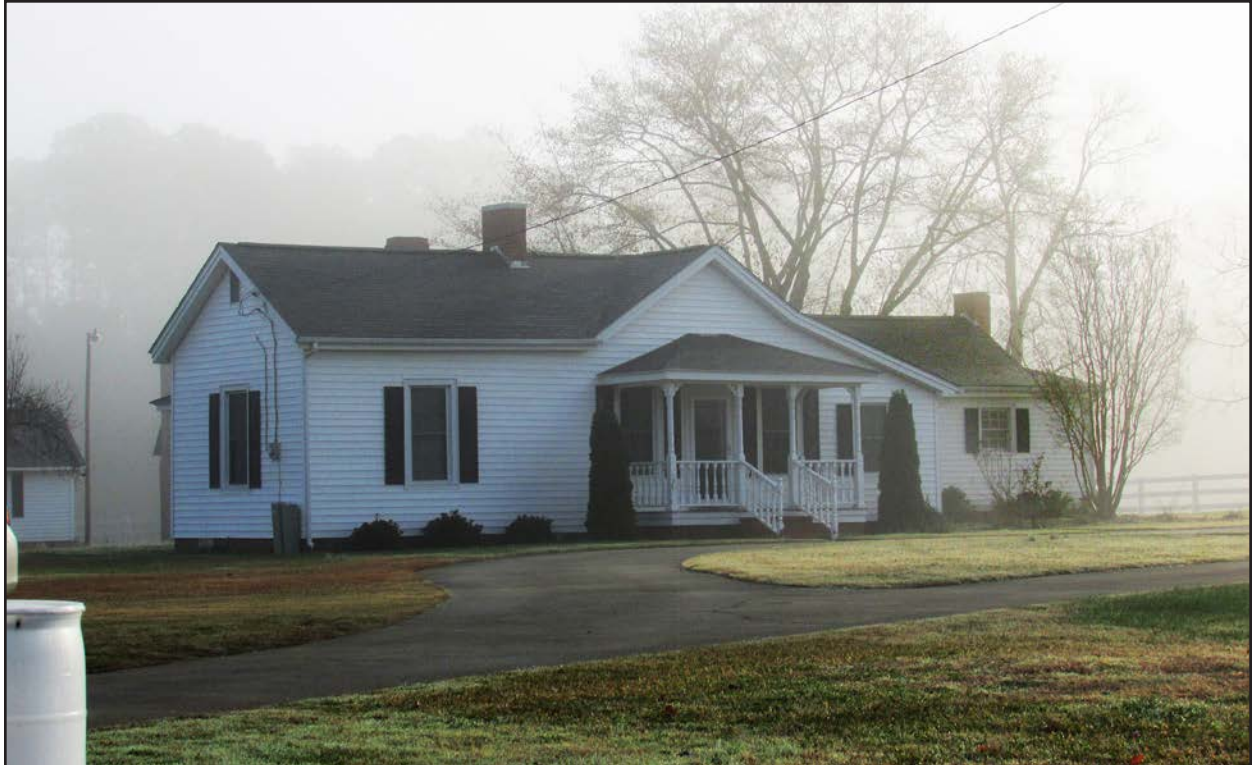
Photo 90. JT1920, facing east-southeast. Dove
