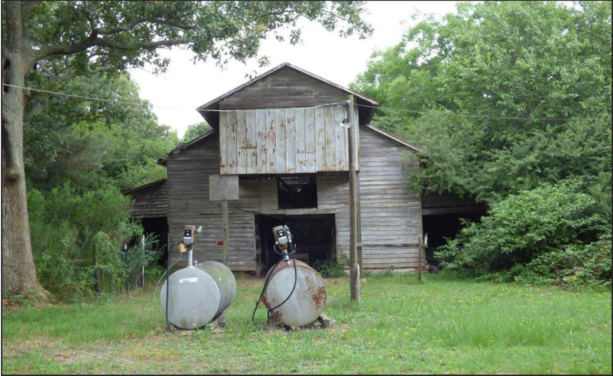
Photo 139. NS1493, hay barn, facing west.
