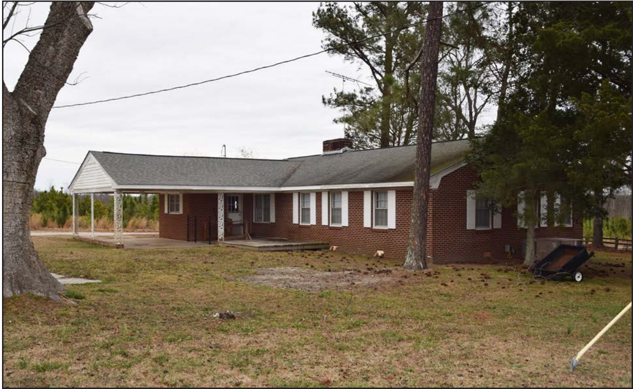
Photo 45. HX1581, facing northeast.
