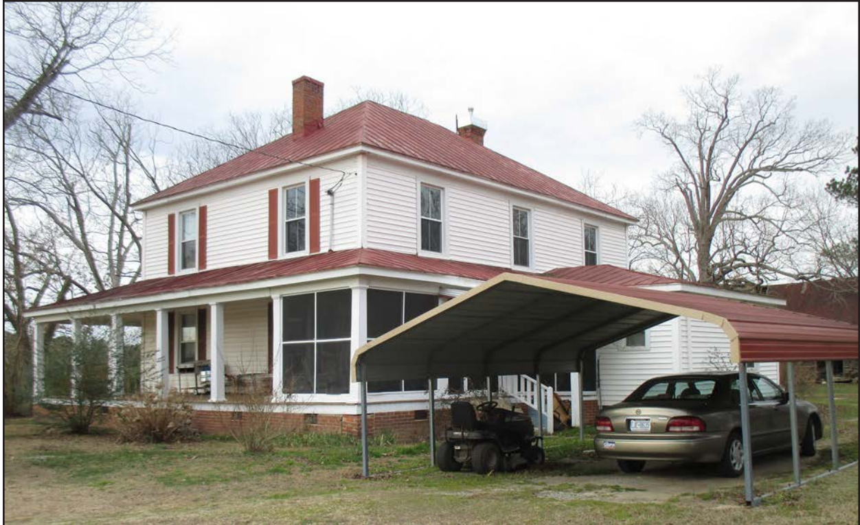
Photo 136. NS0650, carport, facing northwest.
