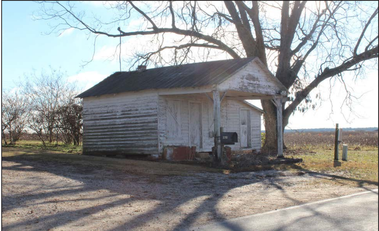
Photo 32. HX0227, rear accessory structure, facing southeast.
