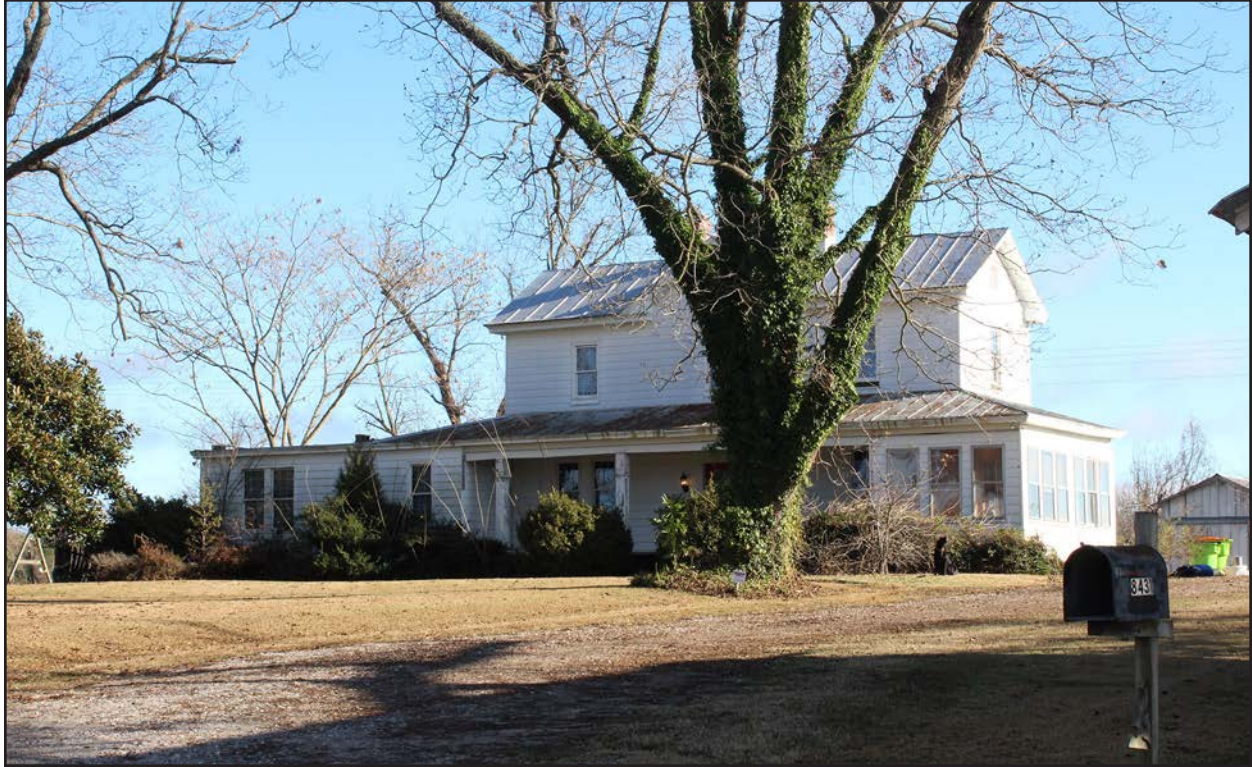
Photo 27. HX0227, main house, facing northeast.
