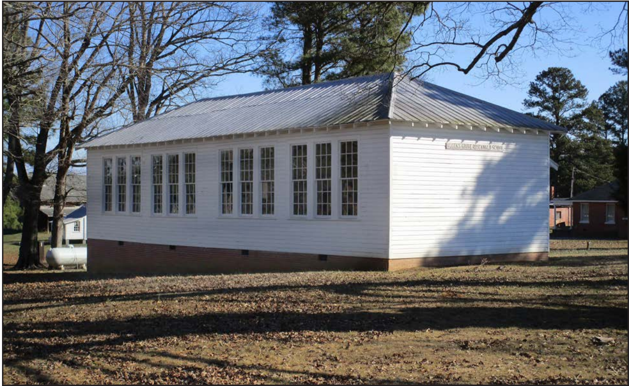
Photo 41. HX1556 (Allen Grove Rosenwald School), facing east.
