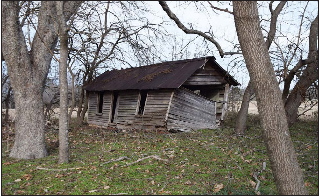
Photo 133. NS0650, summer kitchen, facing northeast
