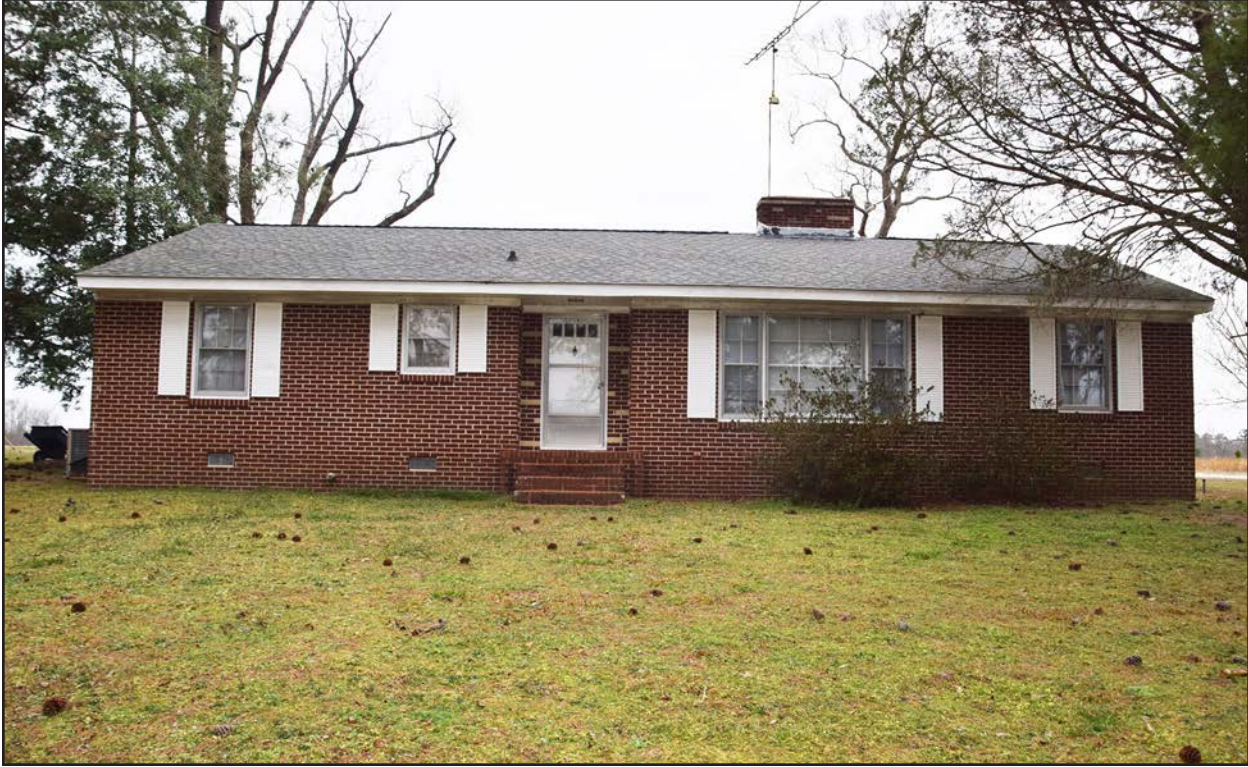
Photo 44. HX1581, facing north-northwest.
