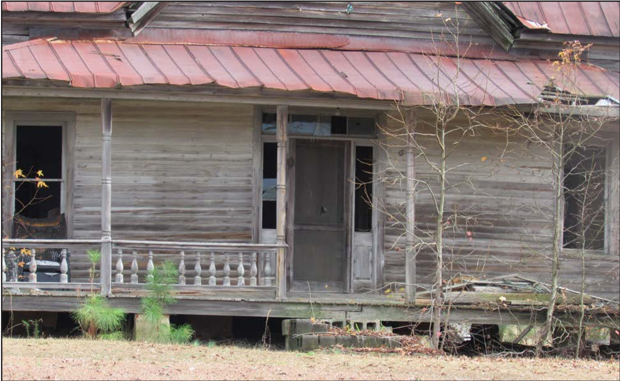
Photo 115. JT1937, main entrance facing east.
