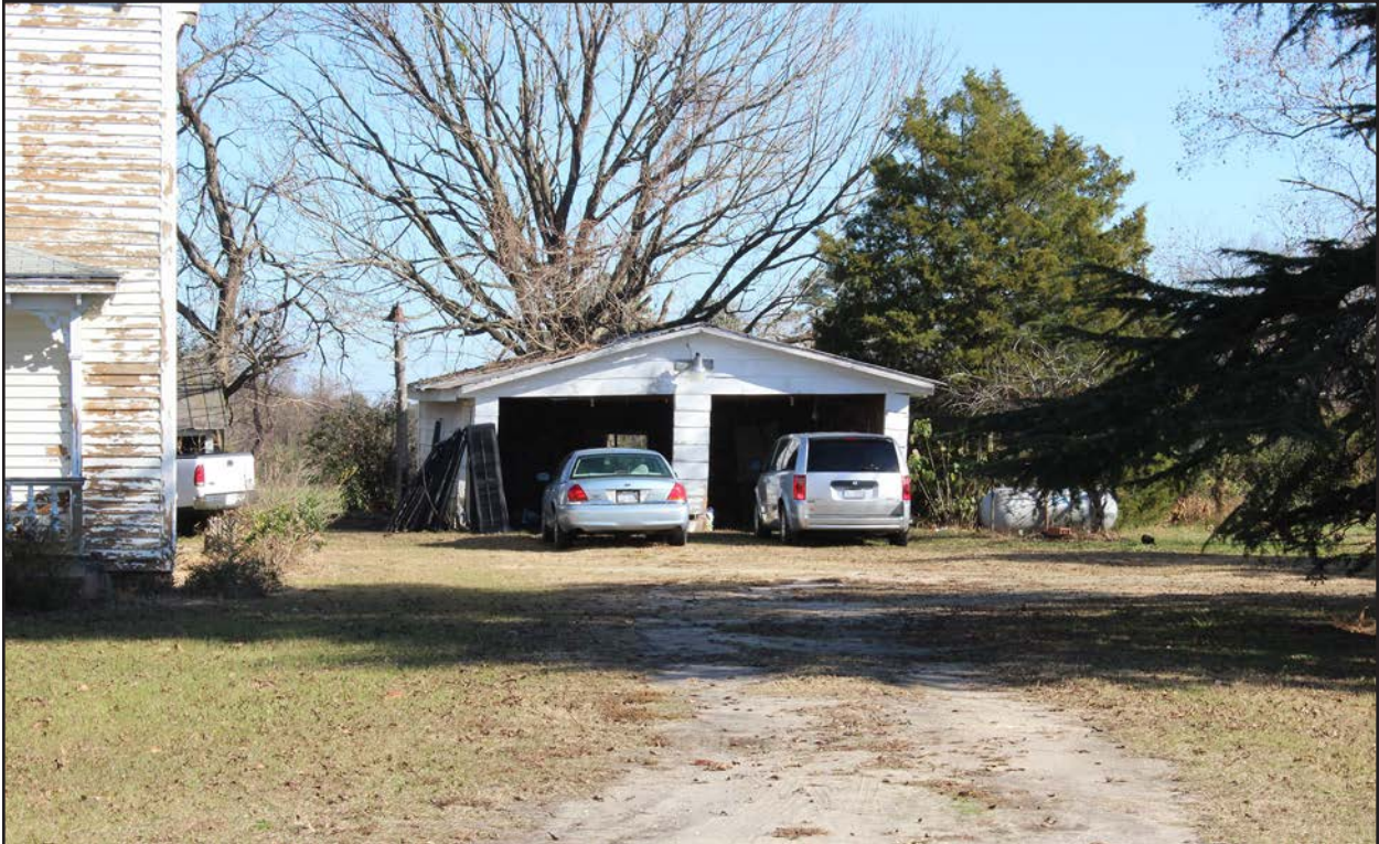
Photo 64. JT0957, garage, facing east.
