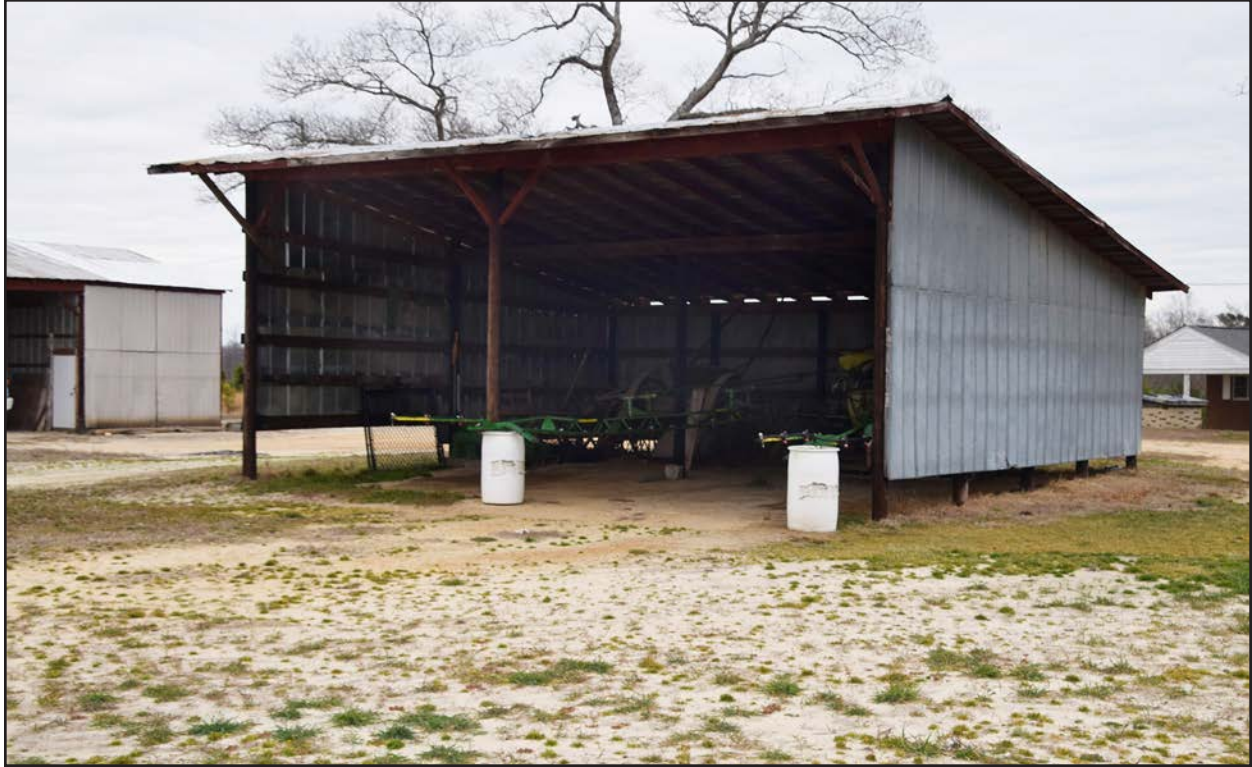
Photo 49. HX1581, equipment shelter, facing northeast.
