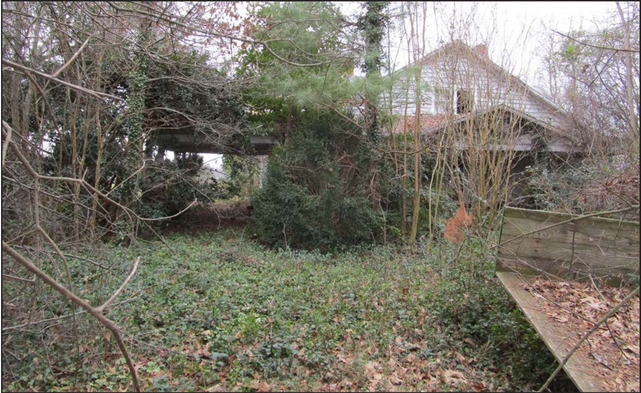
Photo 104. JT1935, facing south.
