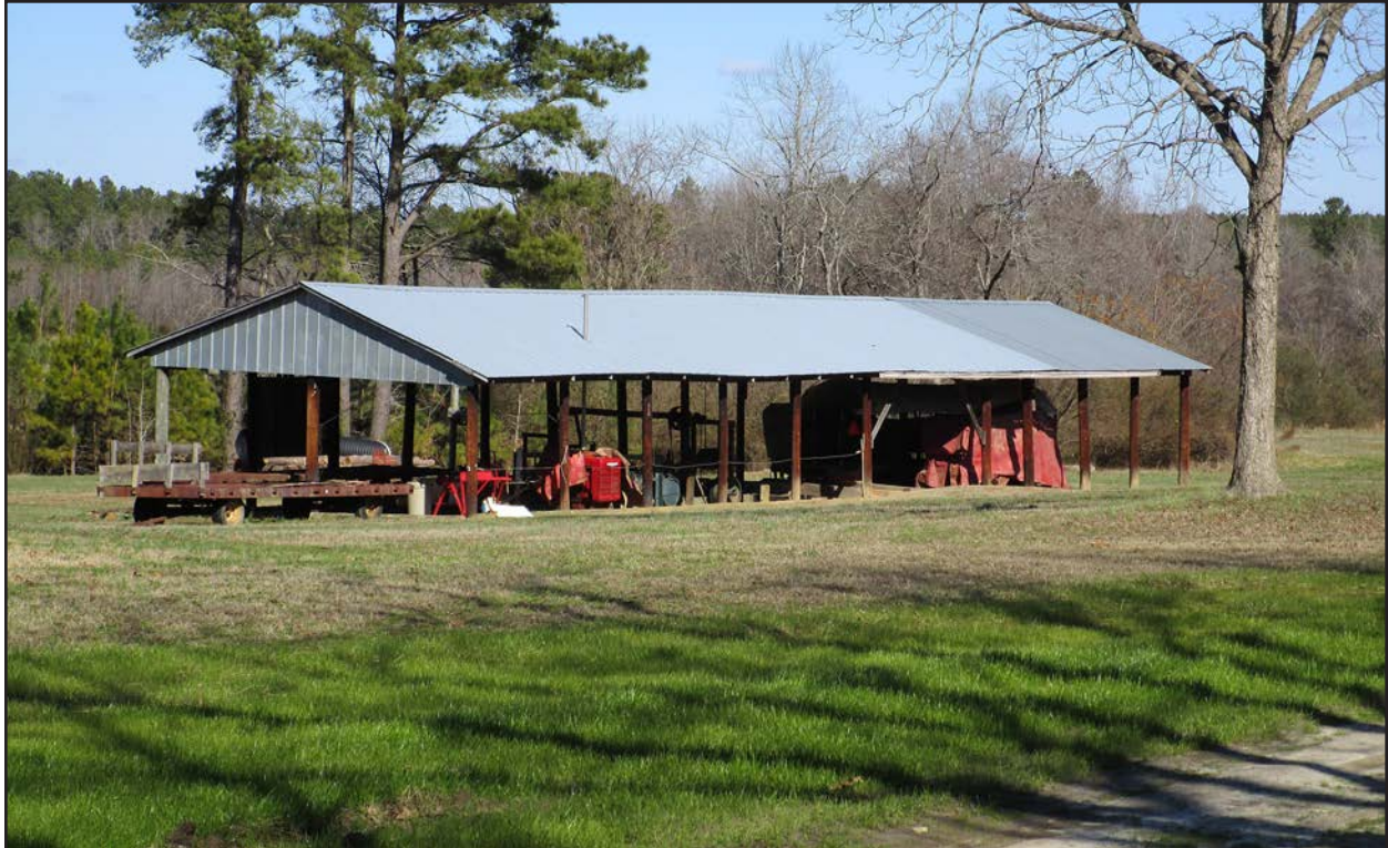
Photo 12. HX0021, equipment shed, facing north-northeast.
