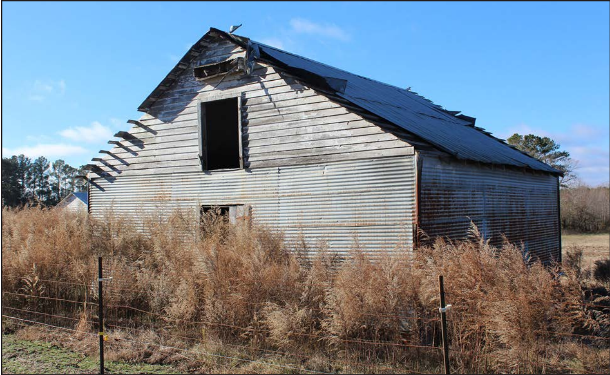
Photo 38. HX0229, facing southwest.
