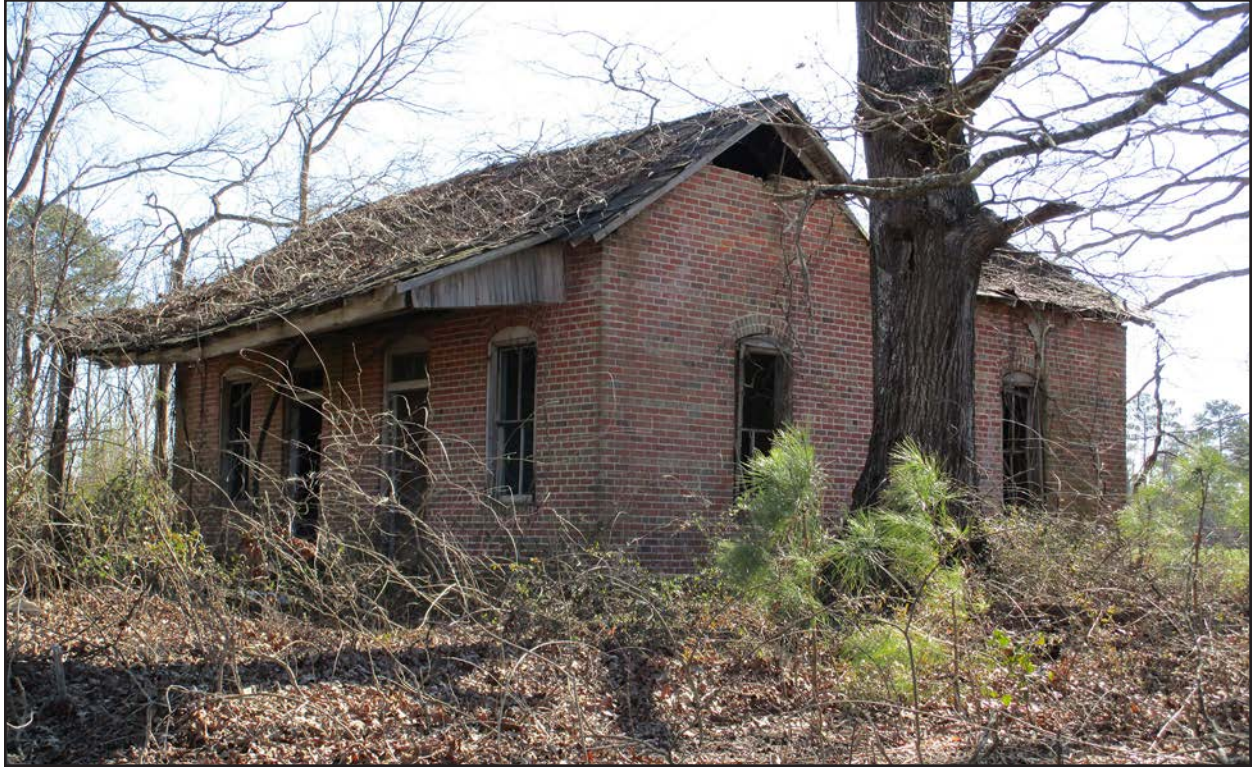
Photo 39. HX0354, facing south.
