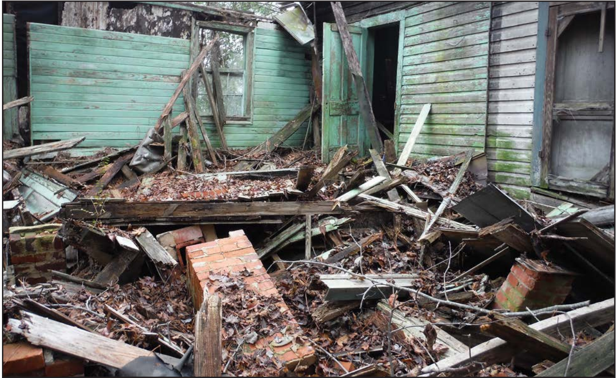
Photo 57. HX1597, dwelling, collapsed addition, facing south.
