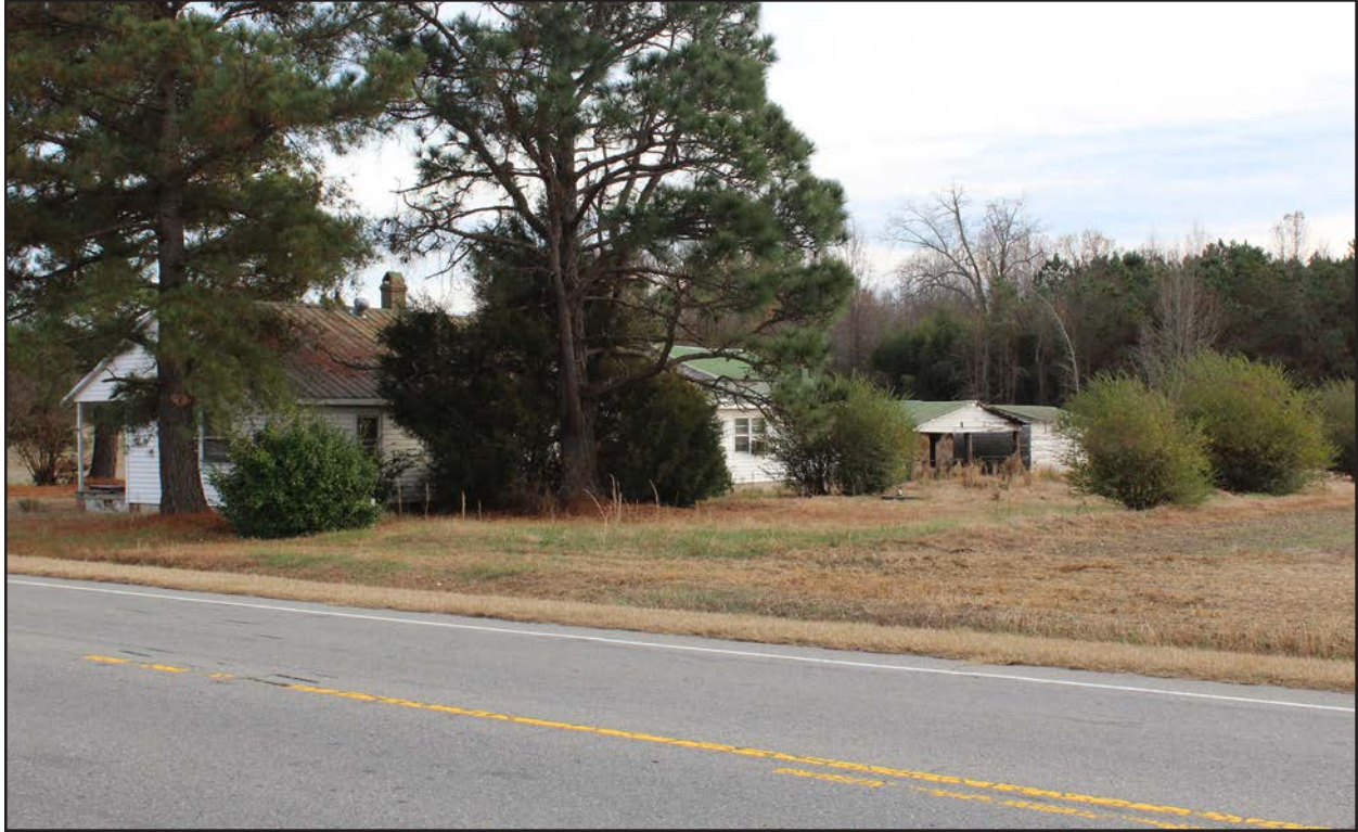
Photo 79. JT1864, house with rear wings, facing southeast.
