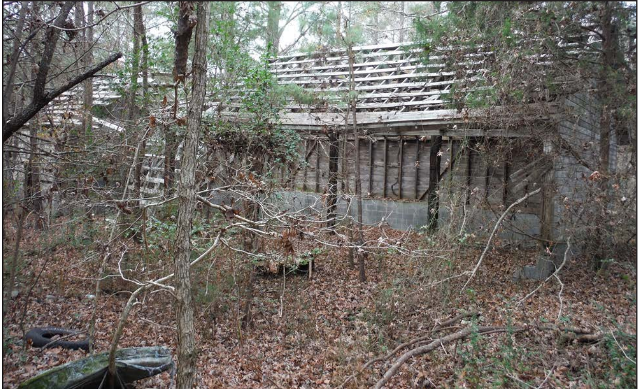
Photo 58. HX1597, barn, facing north.
