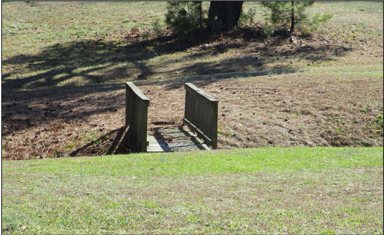
Photo 25. HX0021, wooden bridge, facing south-southeast.
