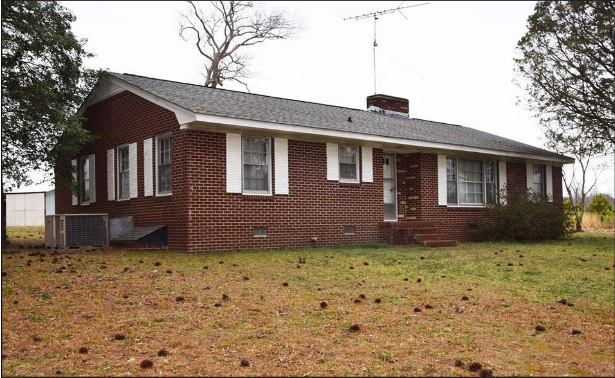
Photo 43. HX1581, facing north-northwest.
