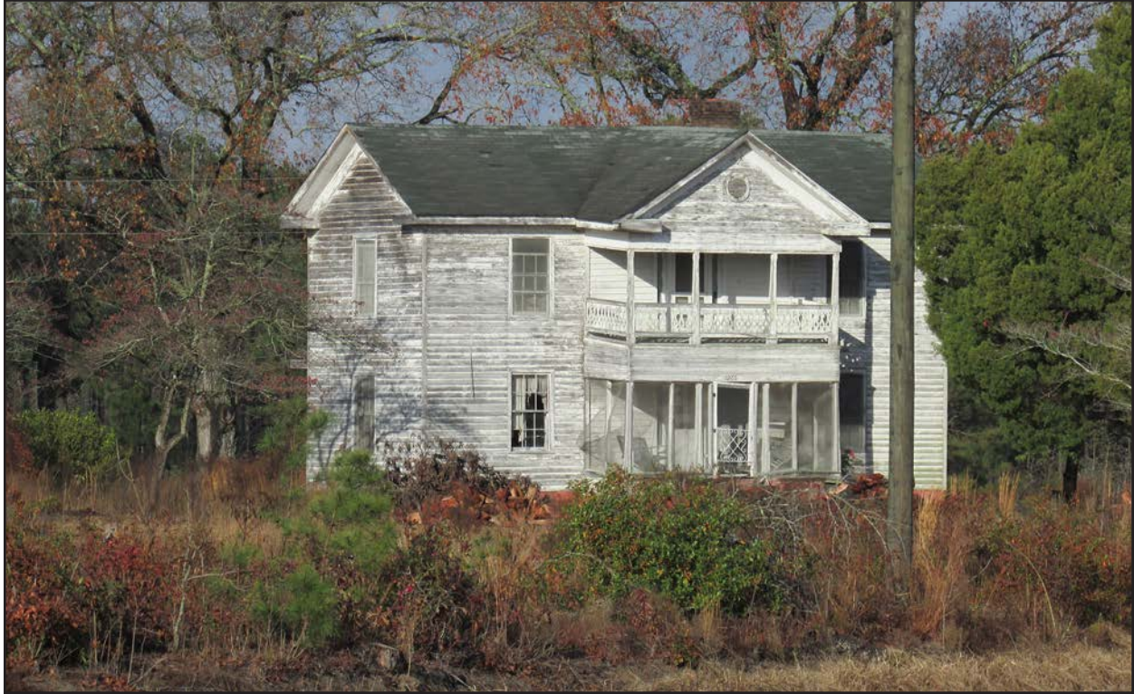
Photo 165. RB0678, house, facing northwest.
