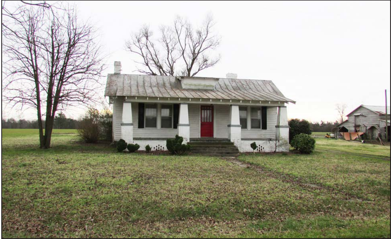
Photo 161. NS1517, dwelling, facing south-southeast.
