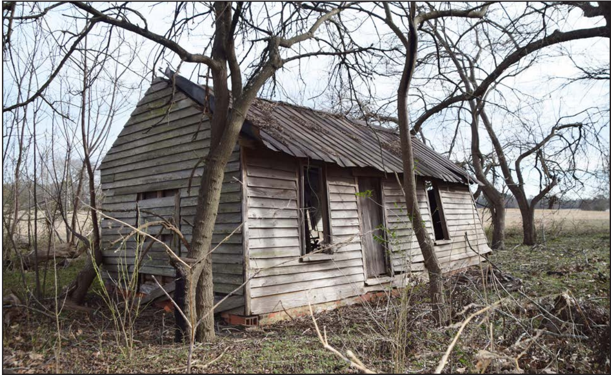
Photo 135. NS0650 summer kitchen, facing northeast.
