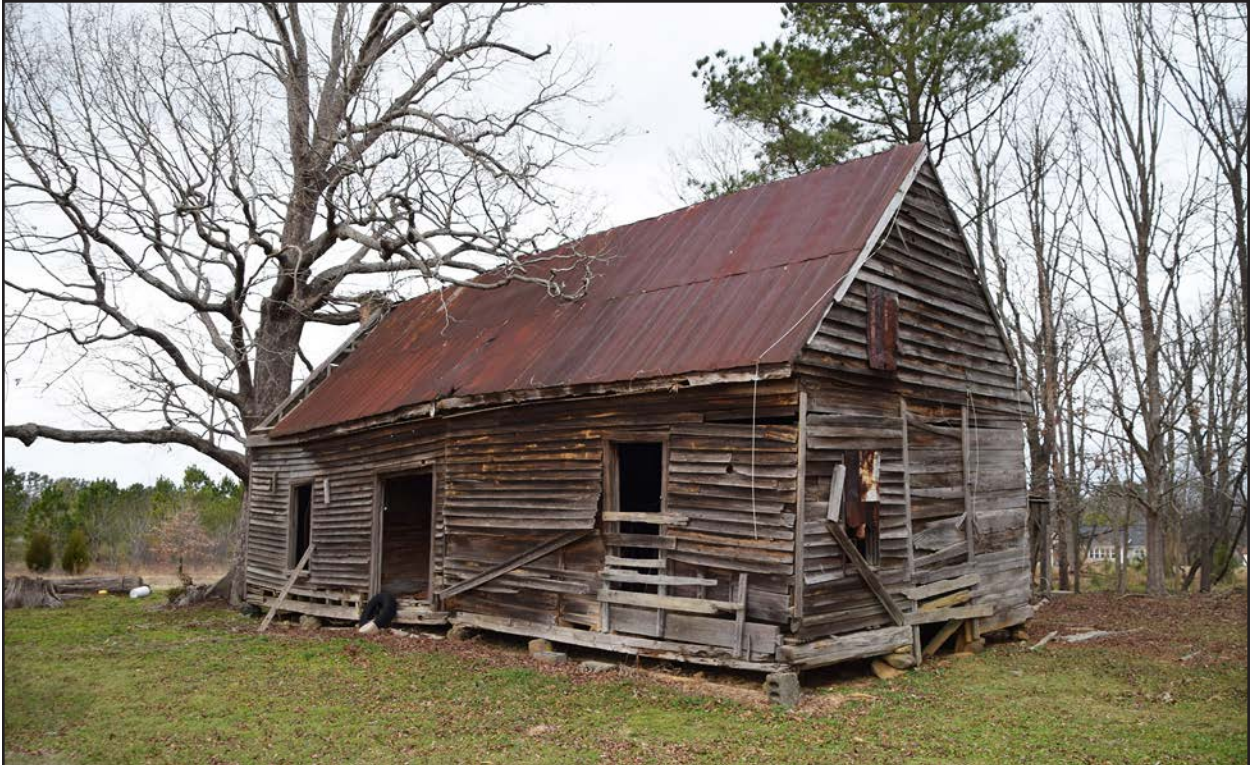
Photo 130. NS0650, cabin, facing northwest.
