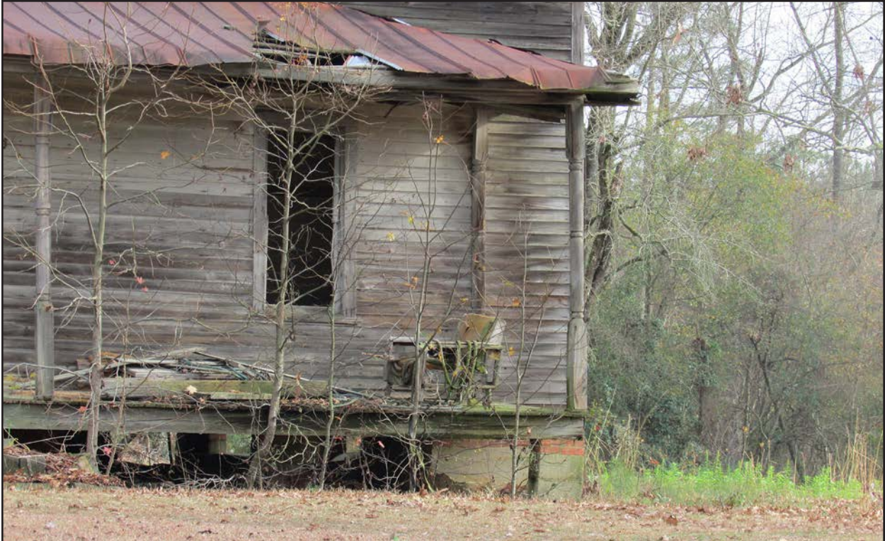
Photo 112. JT1937, foundation, facing southeast.
