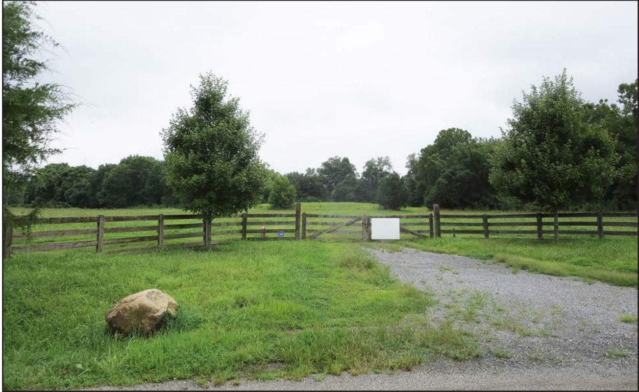
Figure 244. 062-5119, South Rockfish Valley Historic District from Glenthorpe Loop, view northwest.
