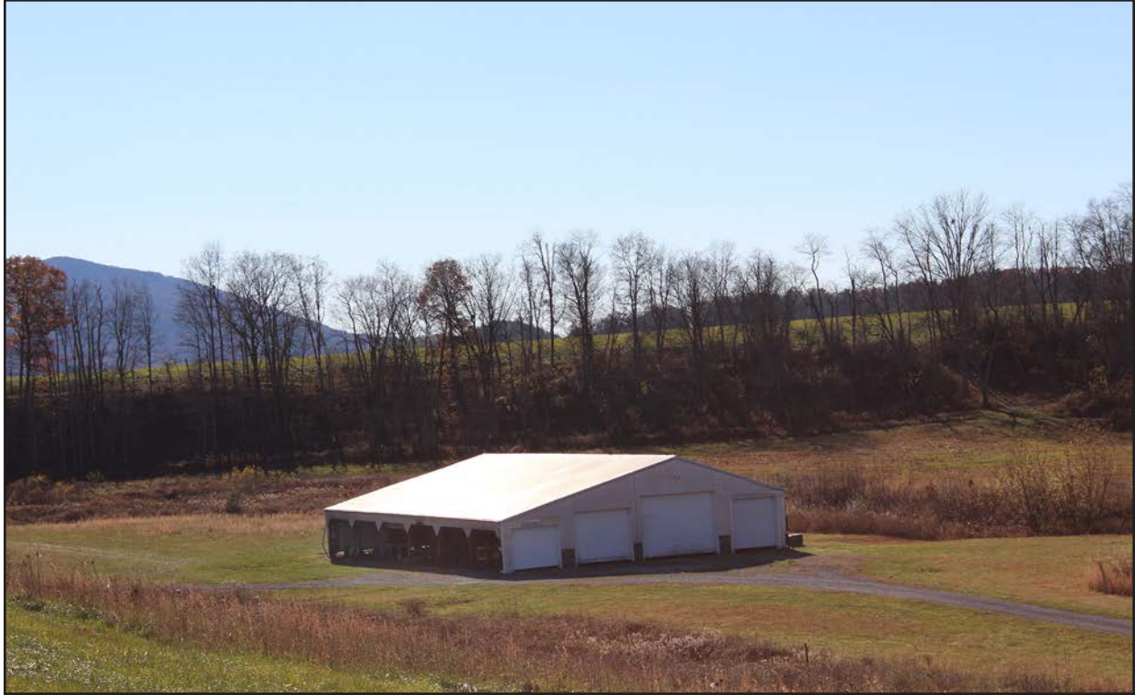
Figure 145. 008-0011, barn, view southwest
