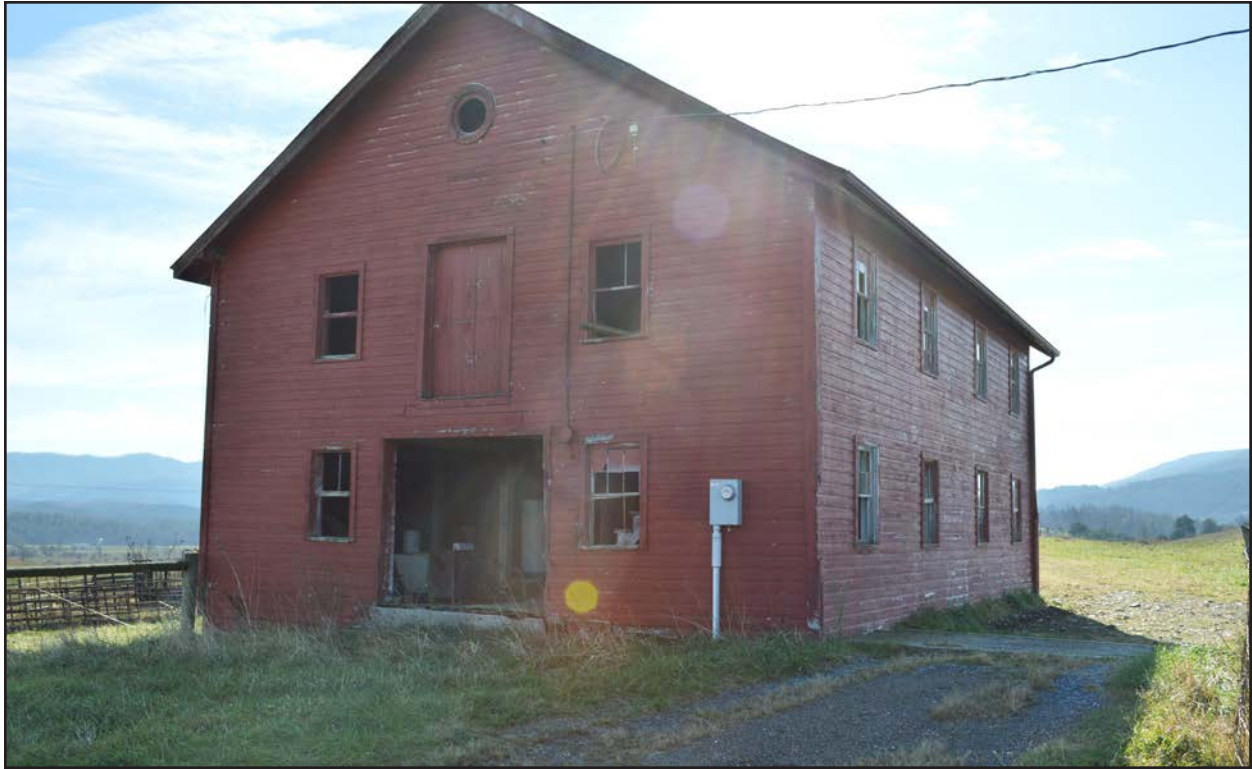
Figure 51. 007-0463, barn 1, view south.
