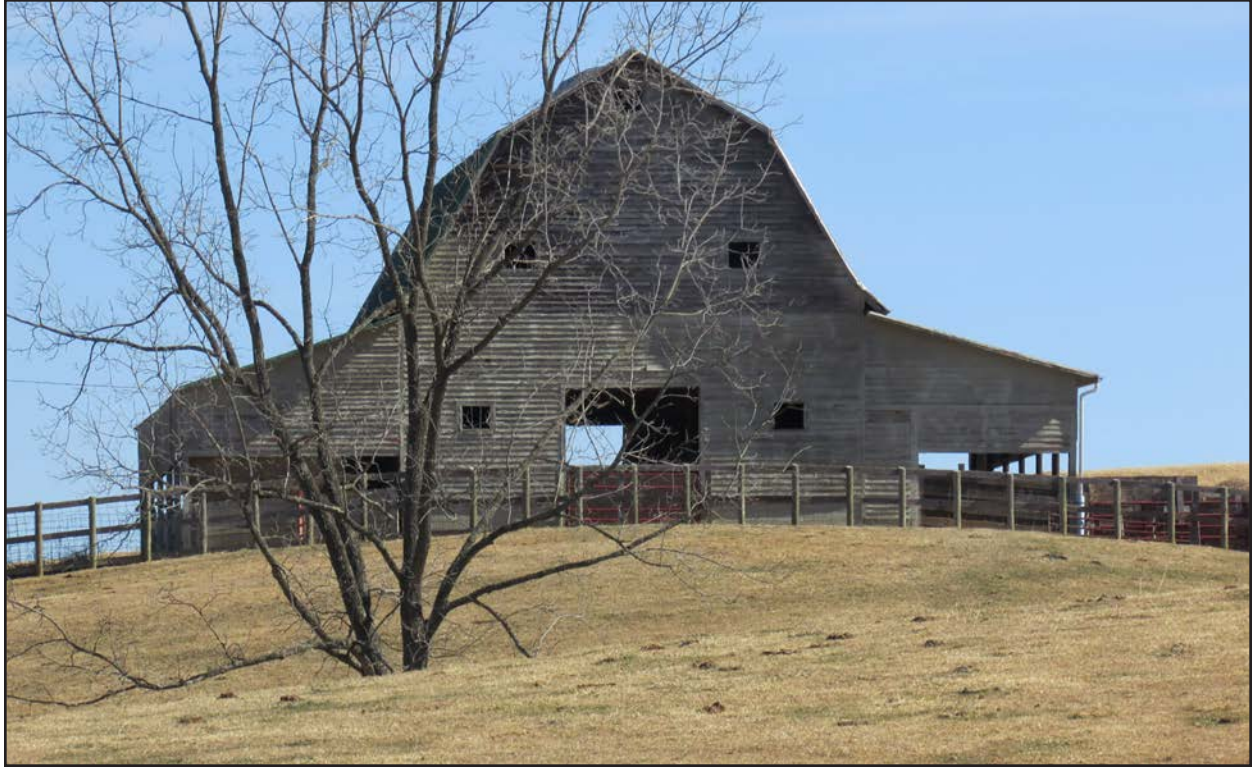
Figure 180. 014-5062, barn, view east.
