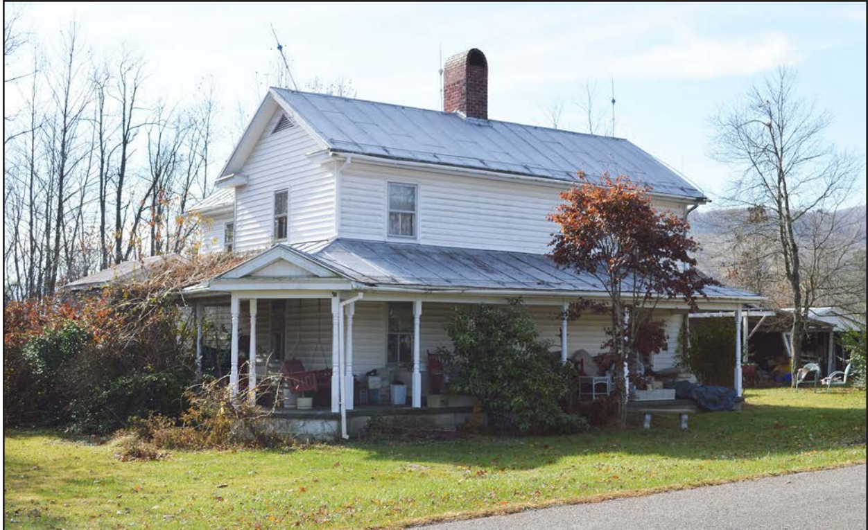
Figure 62. 007-0476, dwelling house, view southwest.
