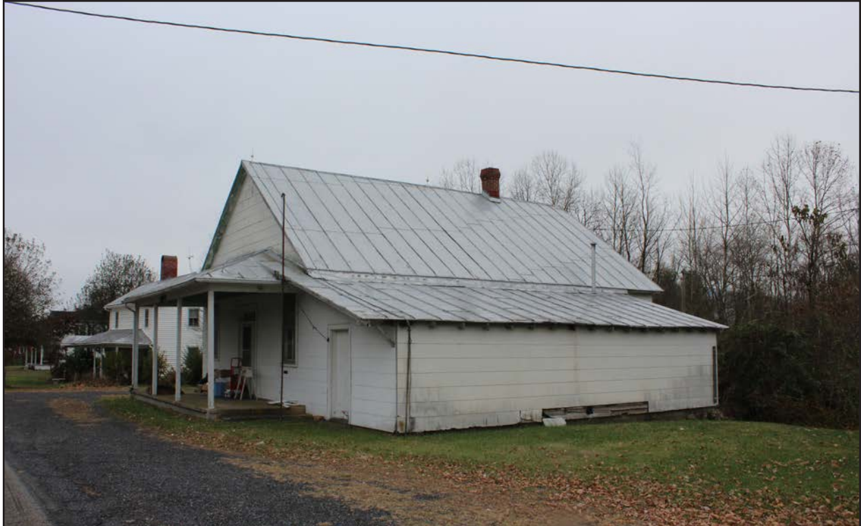
Figure 60. 007-0476, store, view southeast.
