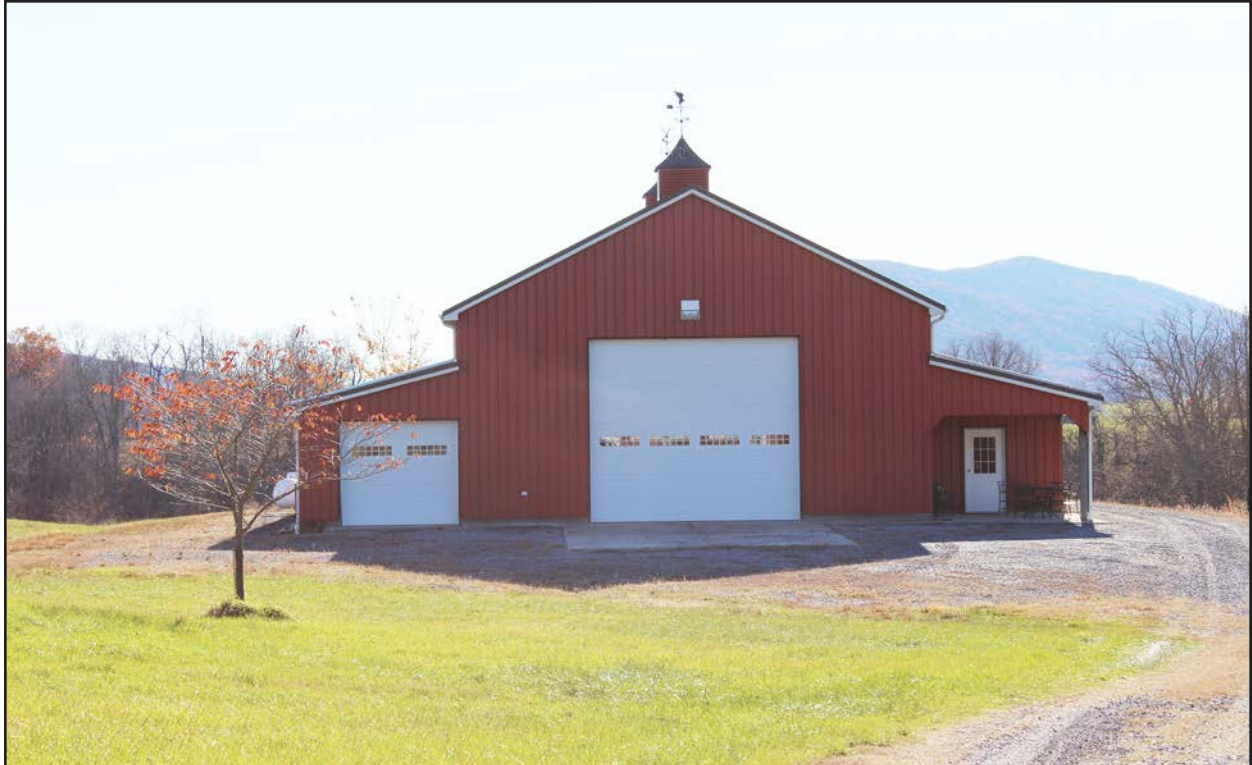
Figure 144. 008-0011, modern barn, view southwest.
