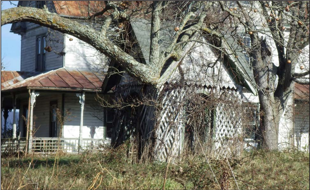
Figure 73. 007-0487, gazebo, view east.
