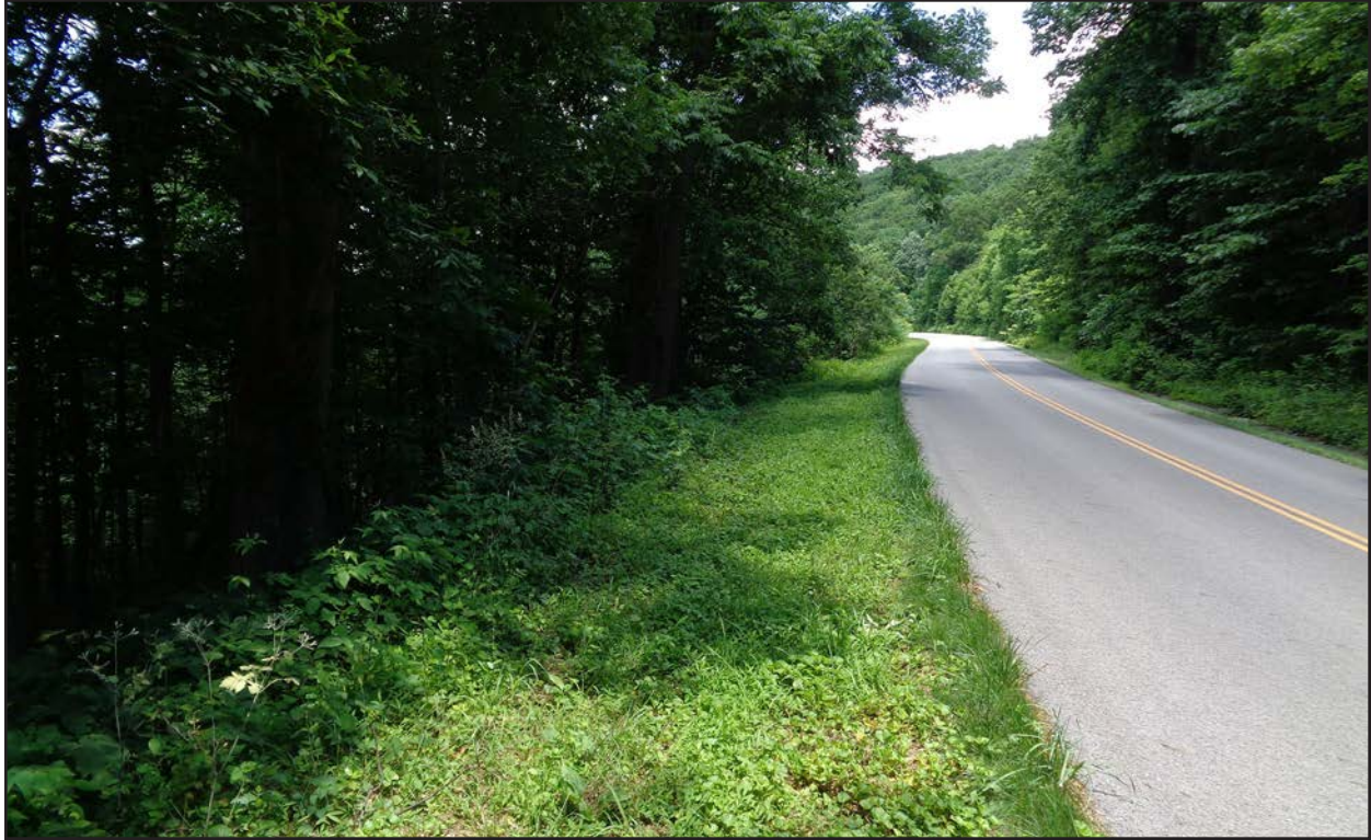
Figure 139. 080-5161, towards Project, view northeast
