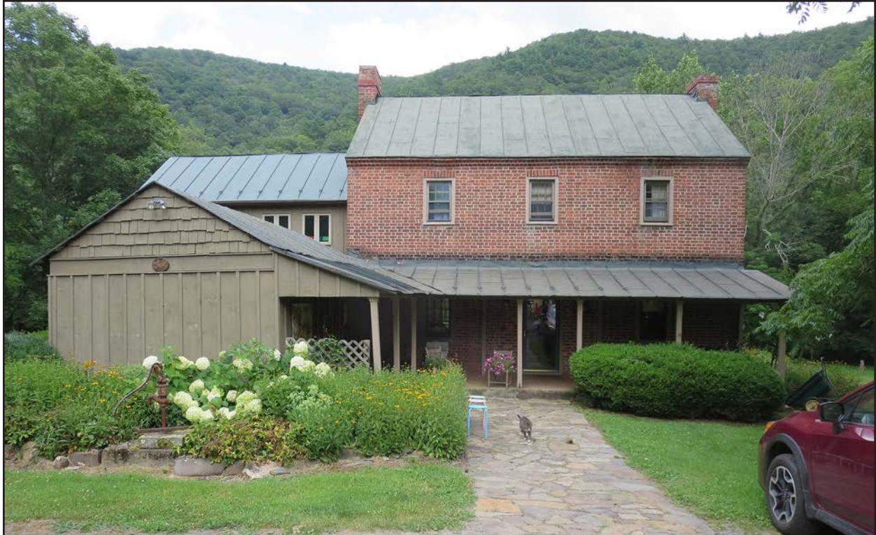
Figure 224. 045-0007, view of west elevation, view east.
