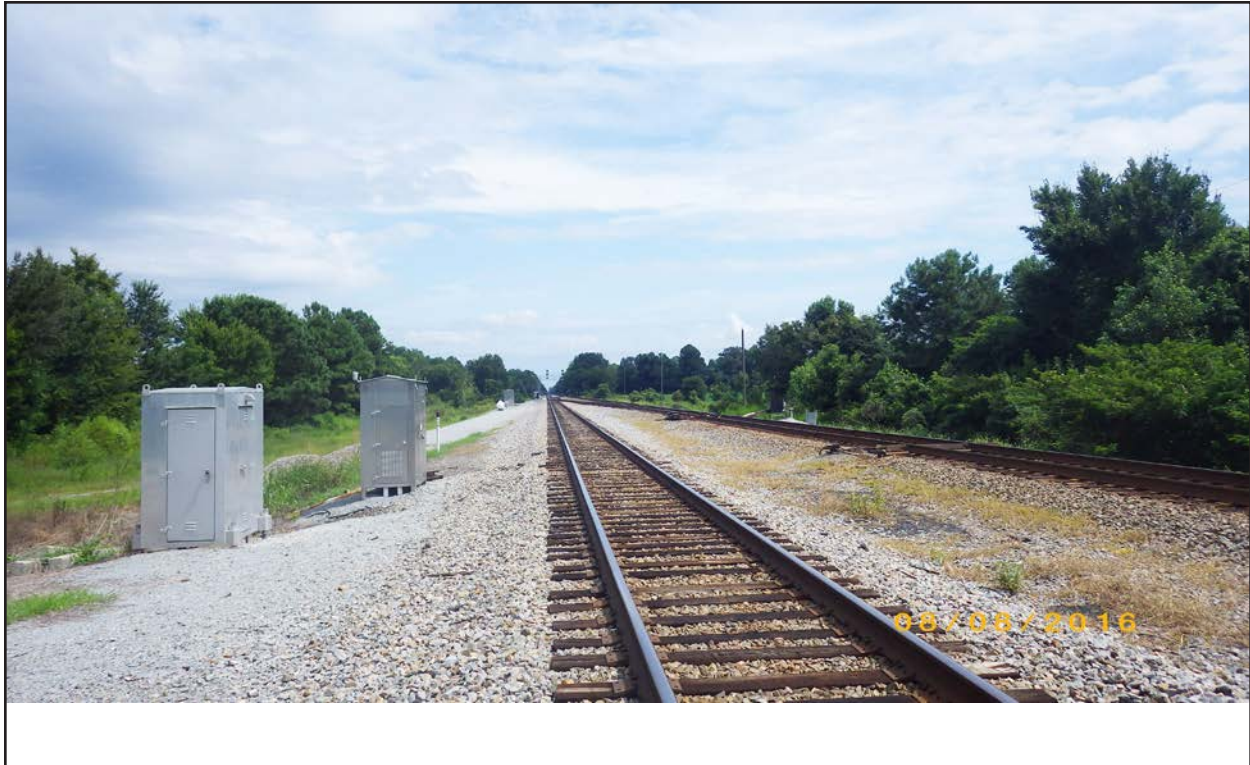
Figure 351. 091-5098, toward Project, view southeast
