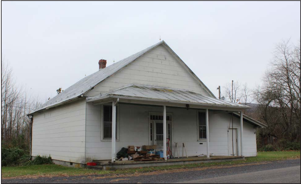
Figure 59. 007-0476, store, view southwest.
