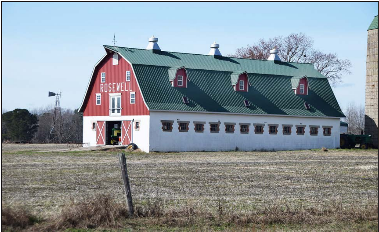
Figure 331. 087-5505, dairy barn, view northwest.
