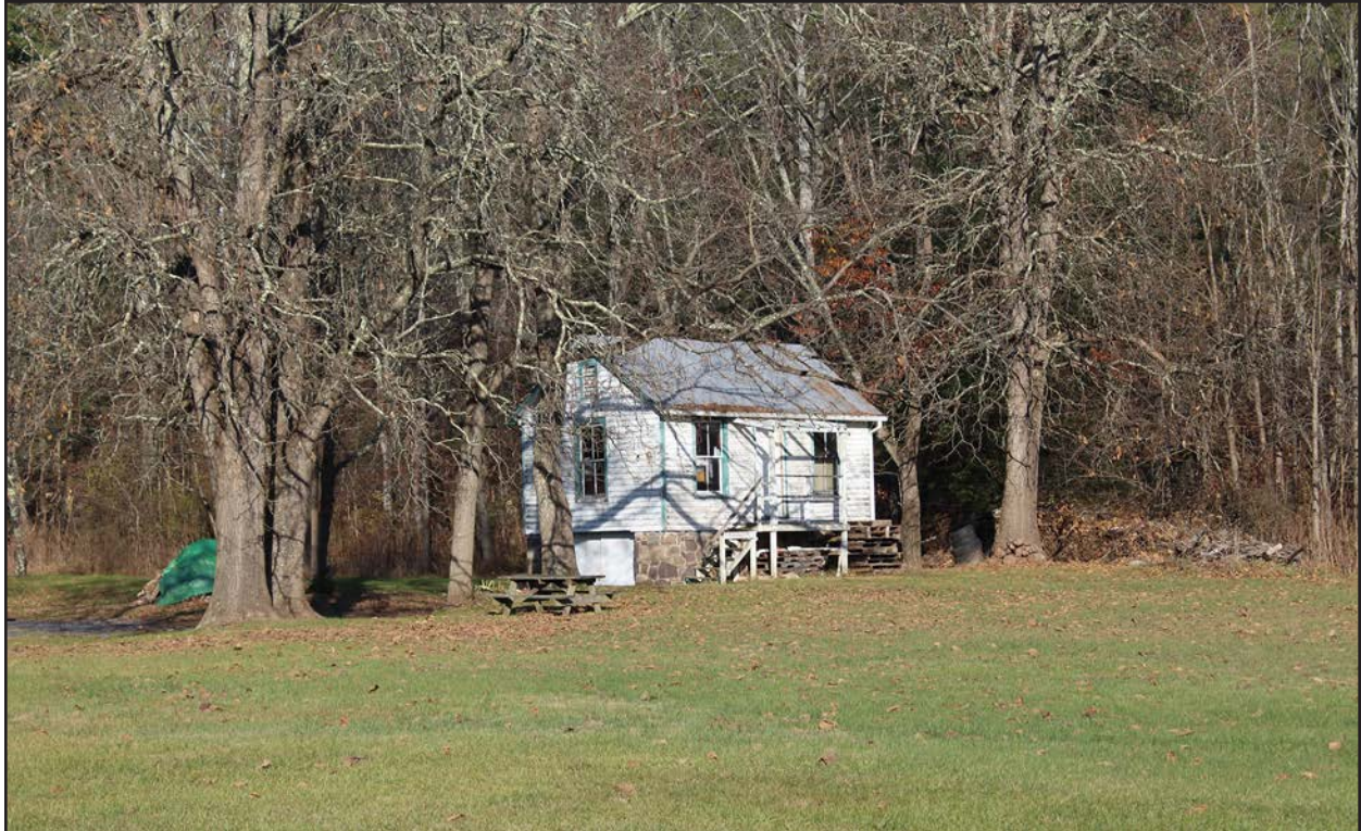
Figure 44. 007-0447, outbuilding 1, view southeast
