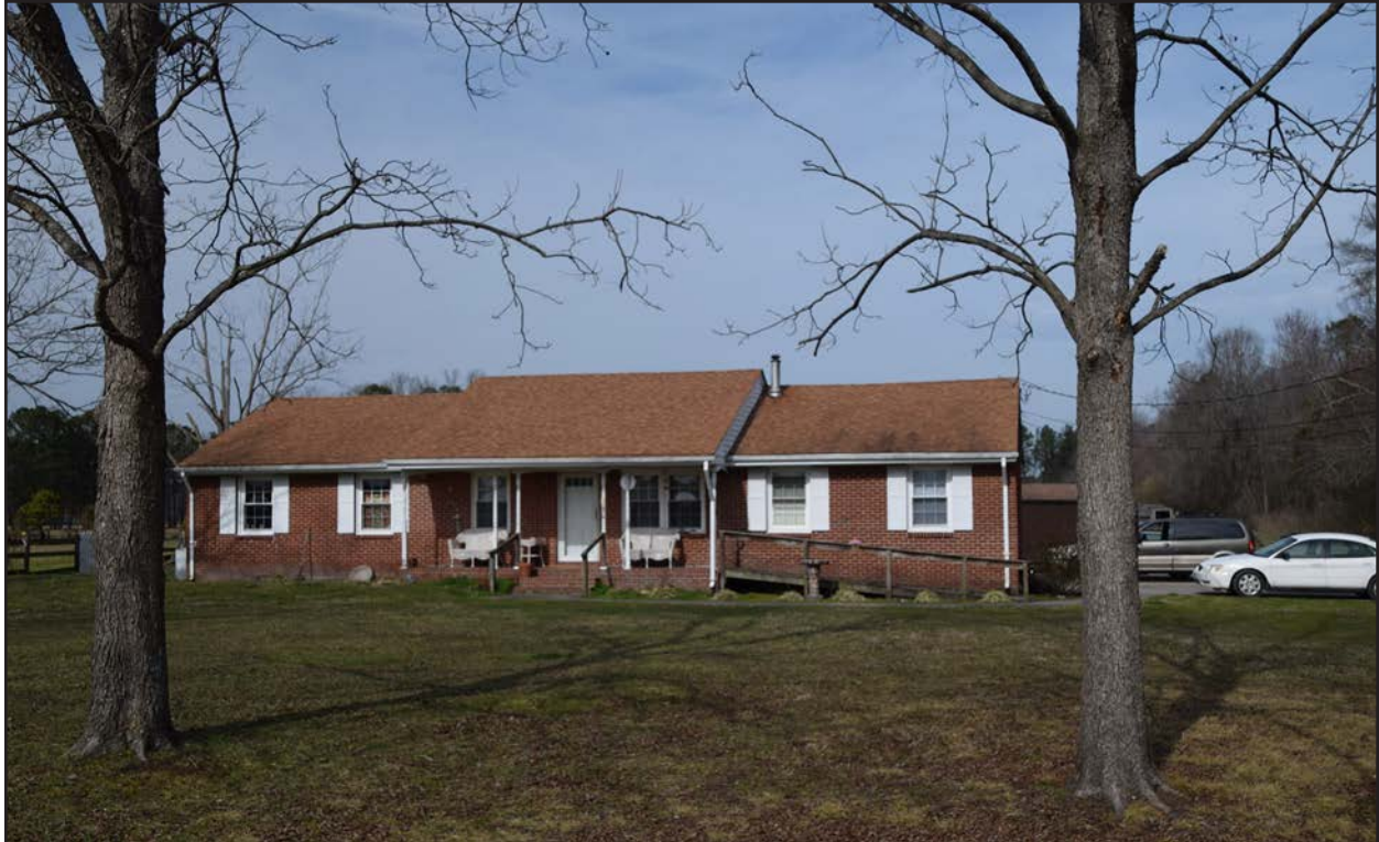
Figure 206. 131-5325-0064, residence, view north.
