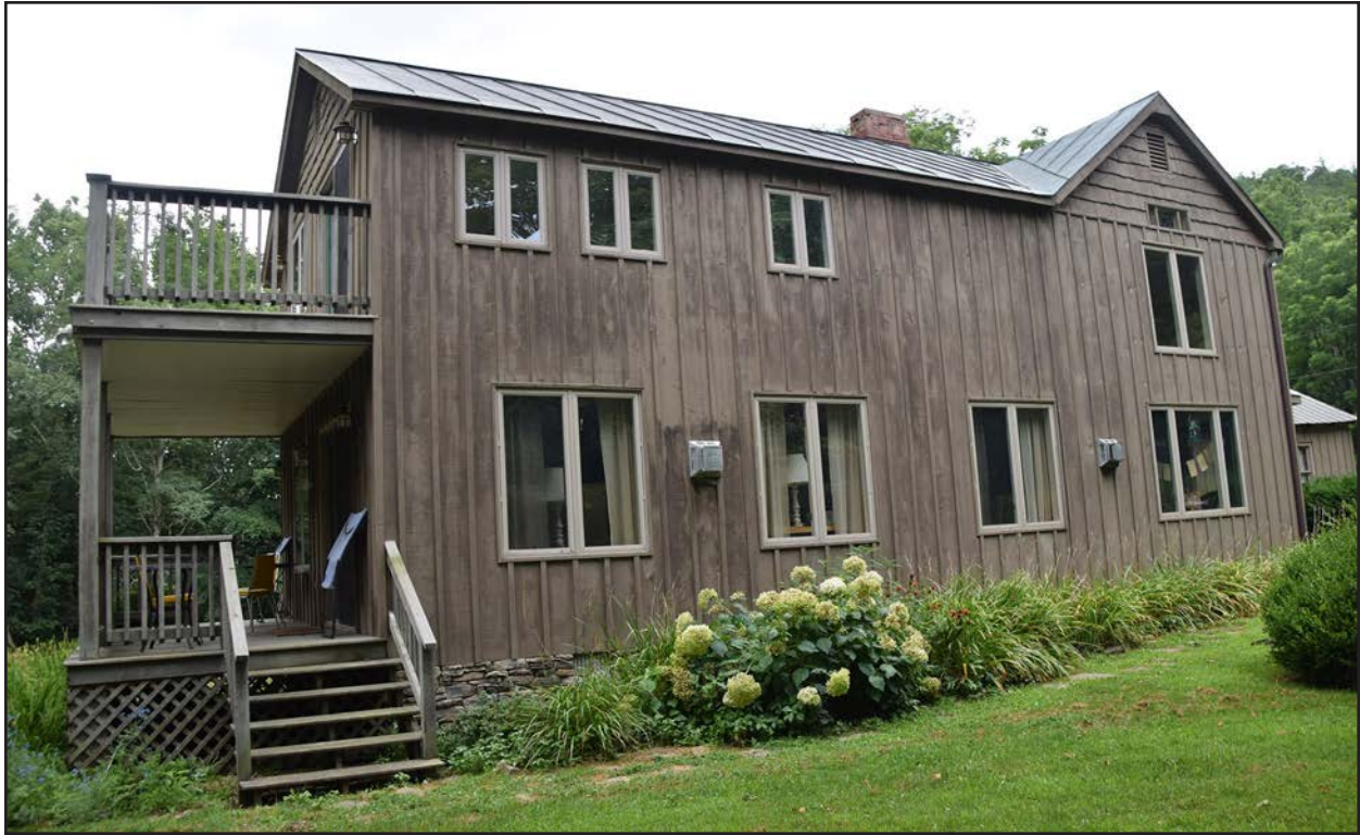
Figure 225. 045-0007, view of additions, view south.
