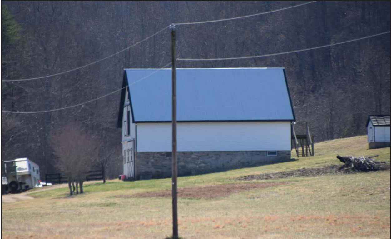
Figure 259. 062-5119-0113, barn, view south-southwest.
