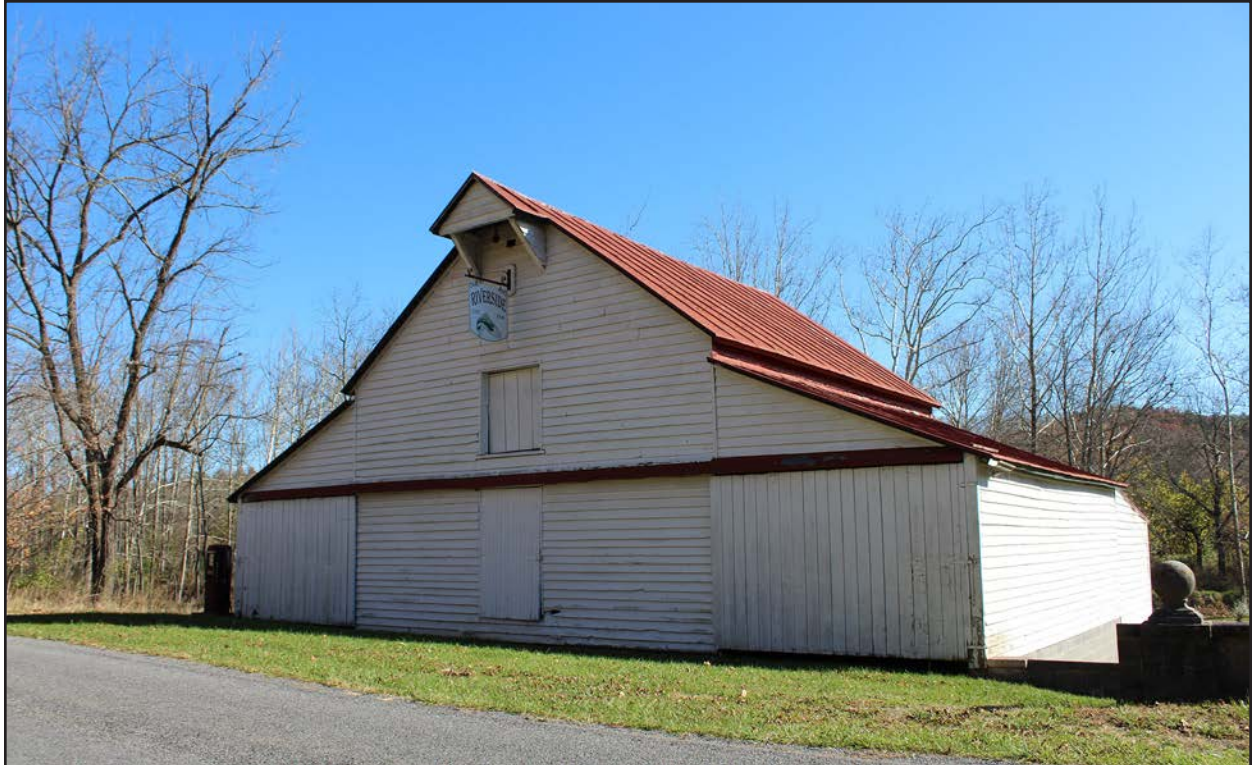
Figure 154. 008-0126, barn, view east.
