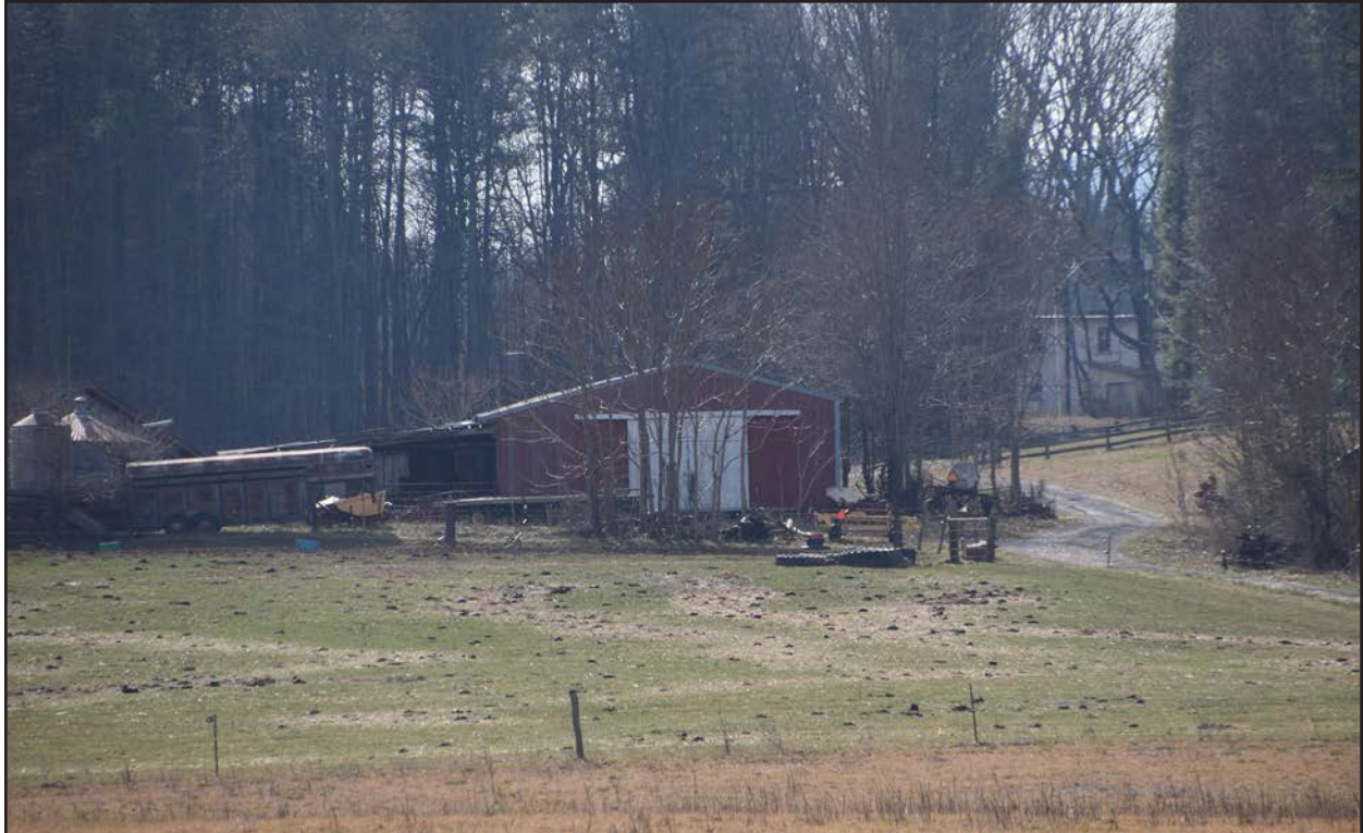
Figure 100. 007-5542, towards project, view west.
