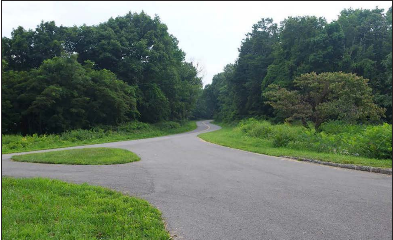
Figure 135. 080-5161, Blue Ridge Parkway Historic District, view south.
