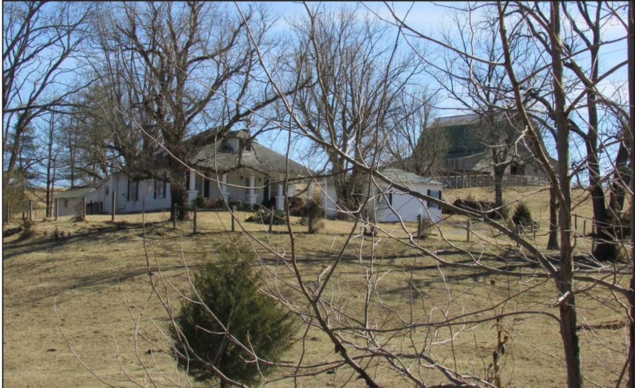
Figure 181. 014-5062, house and outbuildings, view southeast.
