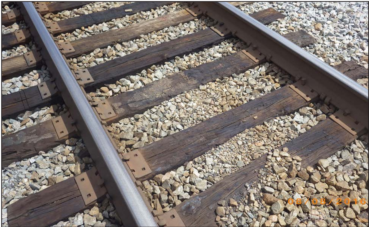
Figure 347. 091-5098, close up of rails, view southeast.
