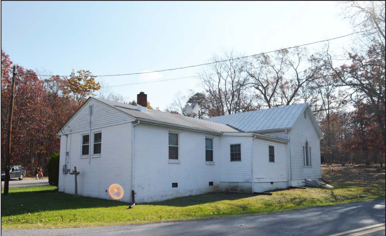
Figure 78. 007-0863, church, view southeast.
