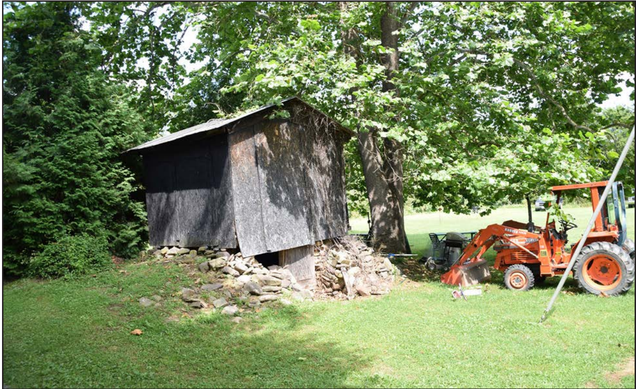
Figure 120. 007-5689, root cellar, view north-northeast.
