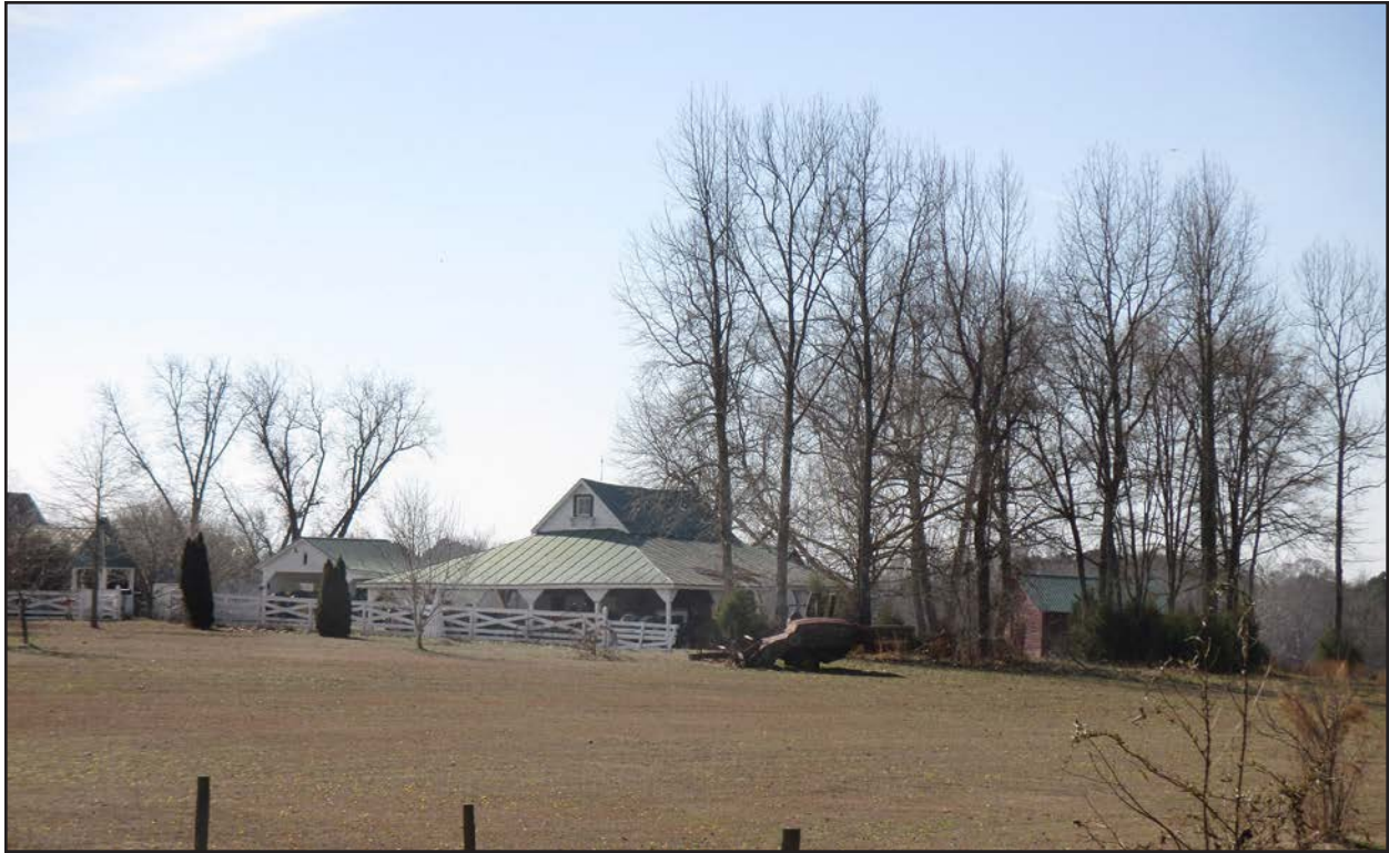
Figure 329. 087-5505, outbuilding, view southwest.
