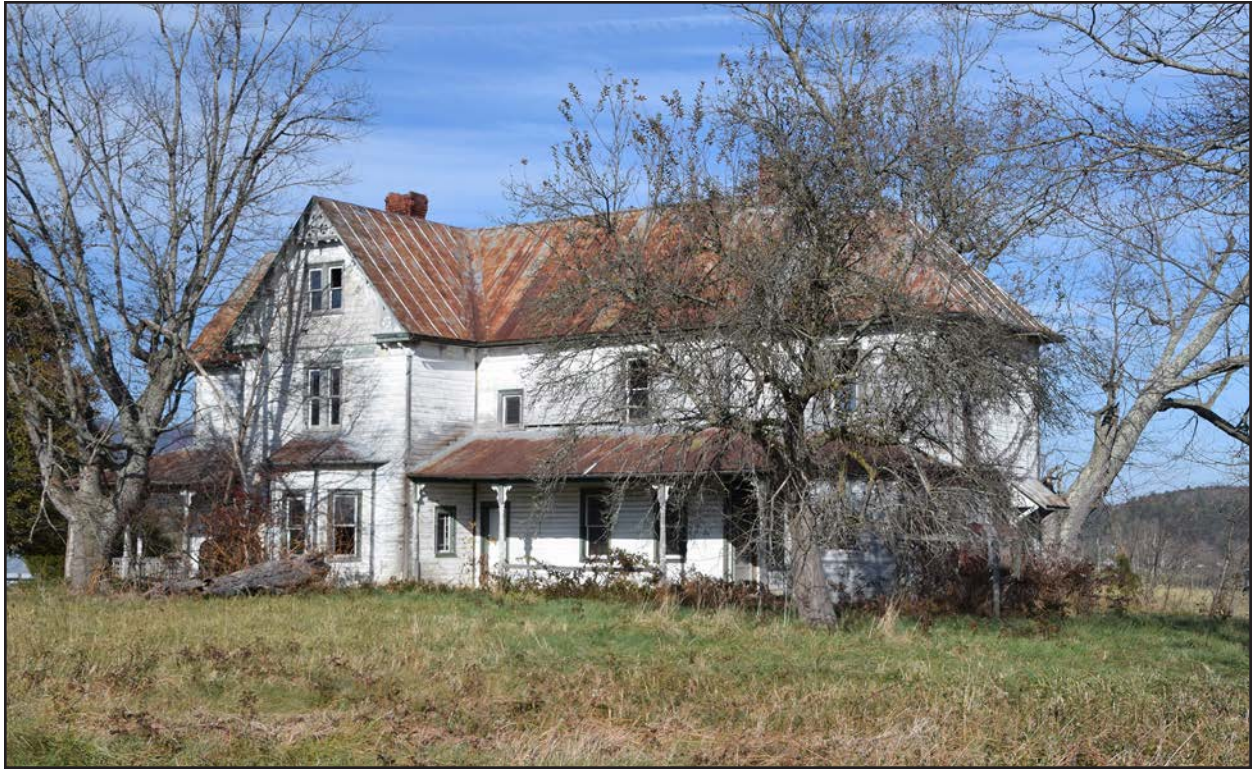
Figure 71. 007-0487, house, view east
