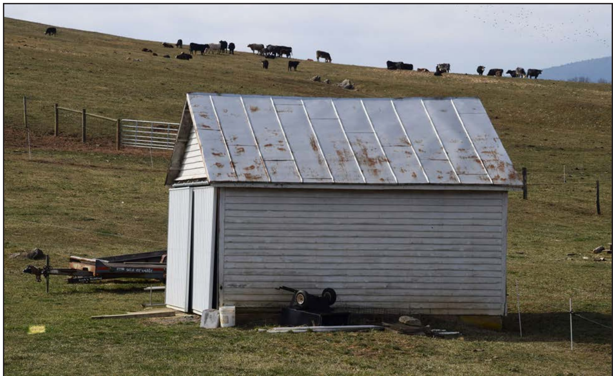
Figure 30. 007-0272, garage, view northwest.
