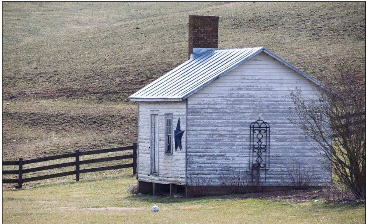
Figure 29. 007-0272, wash house, view southwest.
