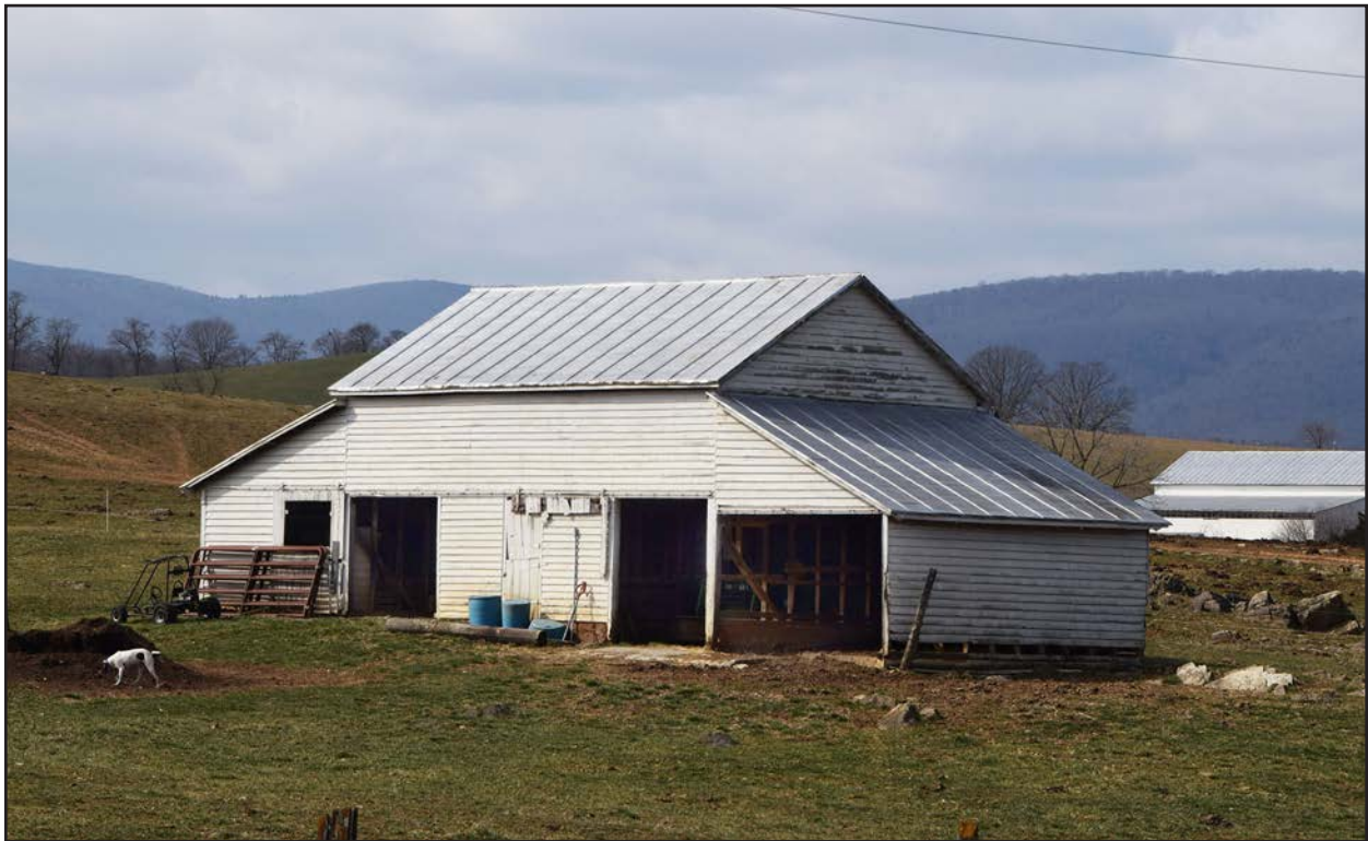
Figure 31. 007-0272, barn, view southwest.
