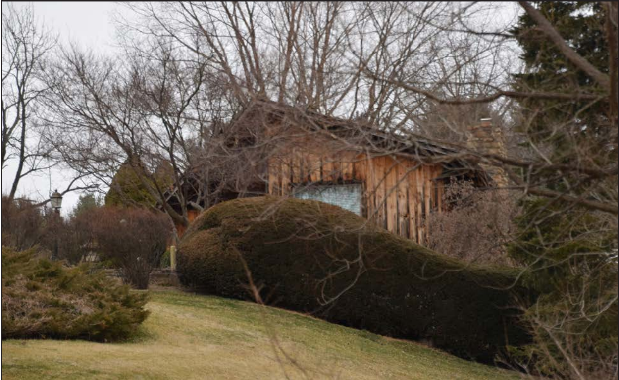
Figure 37. 007-0442, secondary dwelling, view north.
