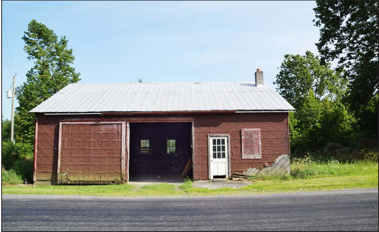
Figure 18. 007-0103, workshop, view south.
