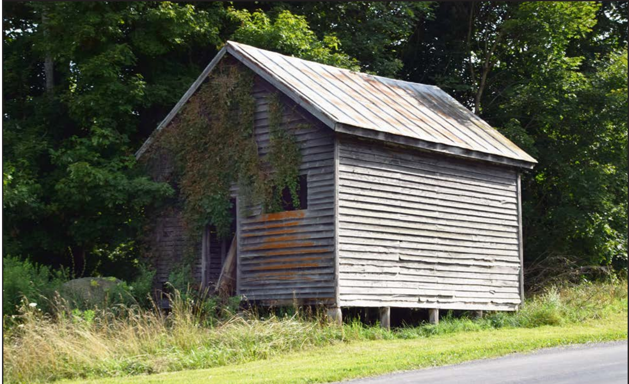
Figure 19. 007-0103, barn, view southwest
