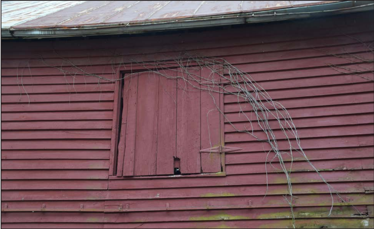
Figure 46. 008-5068, granary and livestock barn, window detail, facing east.
