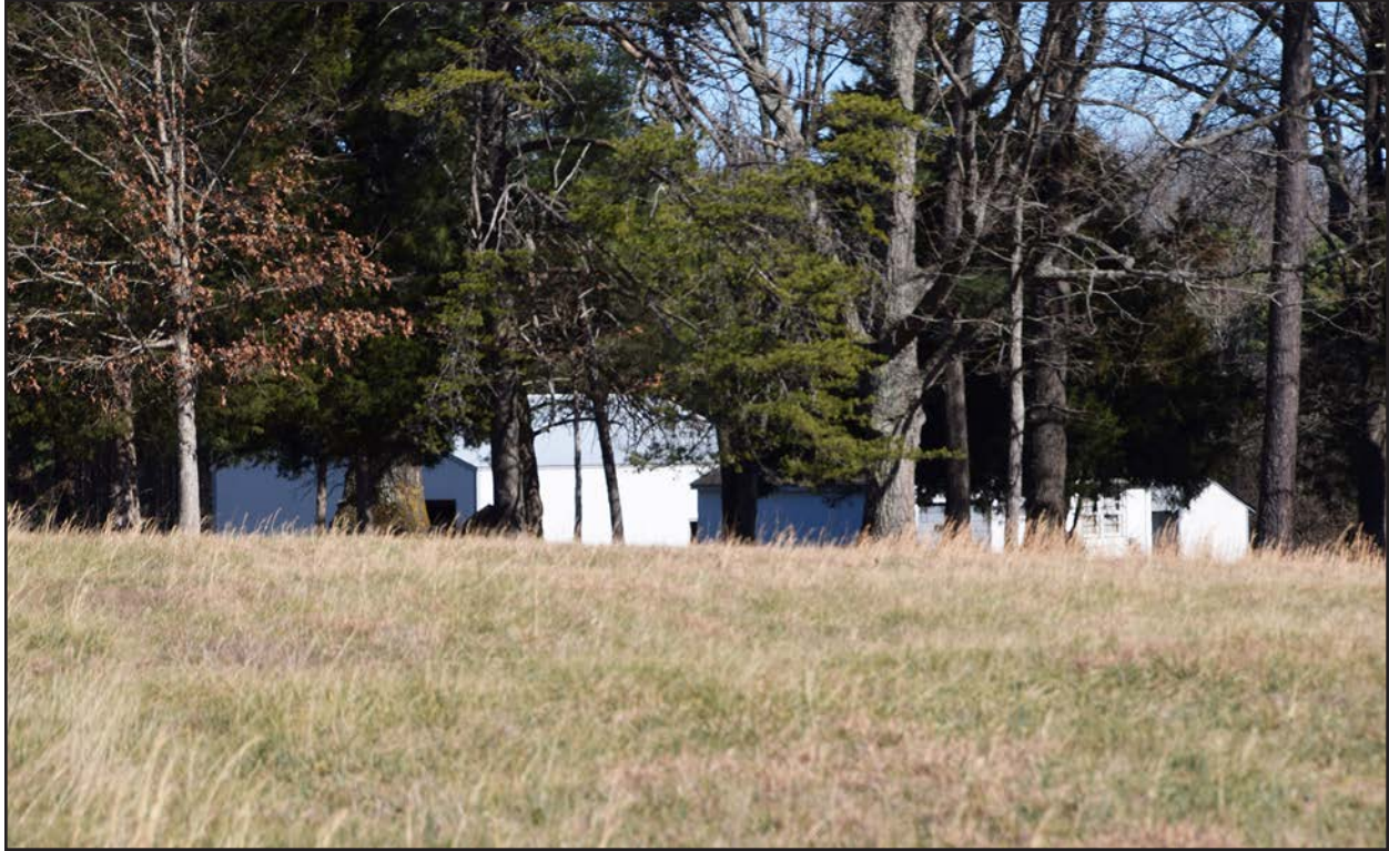
Figure 65. 014-5065, outbuildings, facing east.
