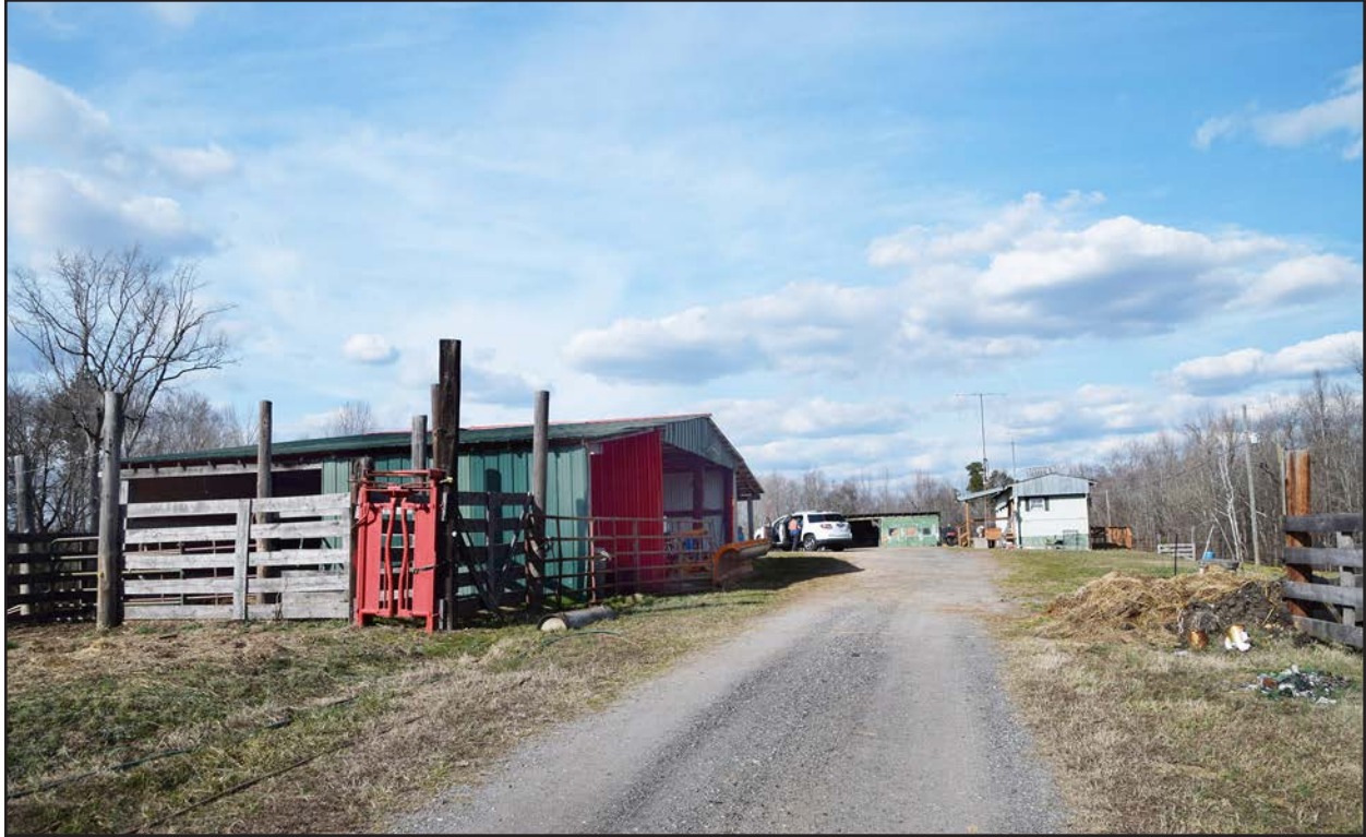
Figure 61. 012-5191, modular home and outbuildings, facing north.
