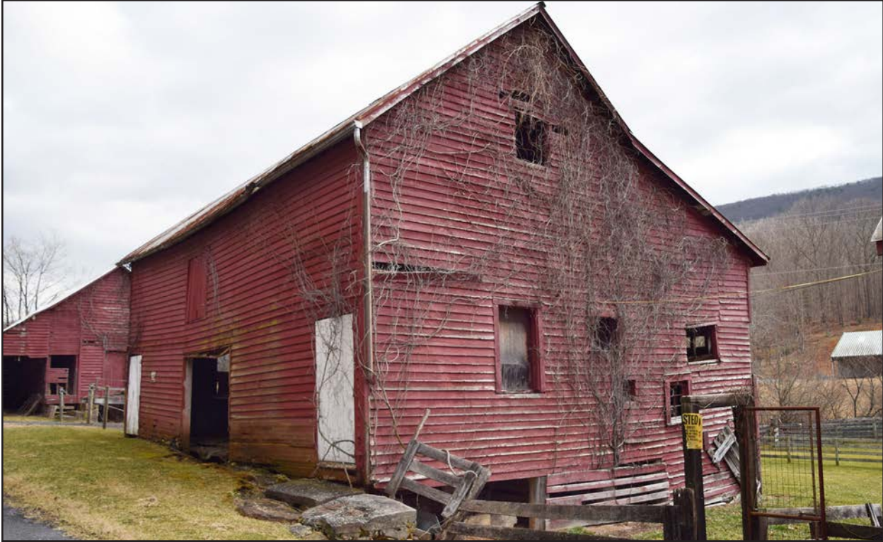
Figure 45. 008-5068, granary and livestock barn, side detail, facing northeast.
