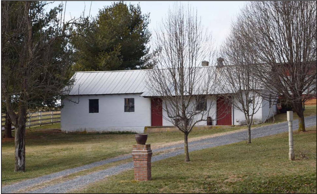
Figure 25. 007-5584, concrete block building detail, facing northwest.
