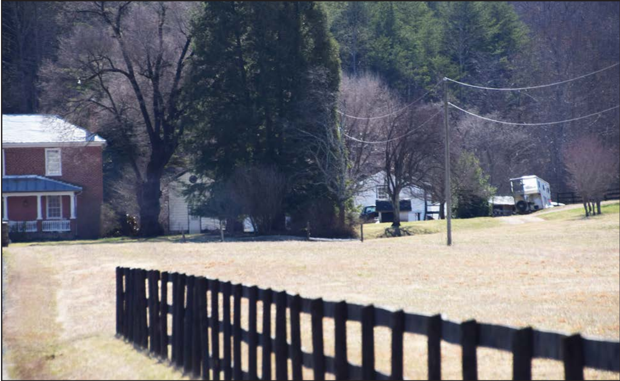
Figure 84. 062-5119-0113, accessory structures, facing south.
