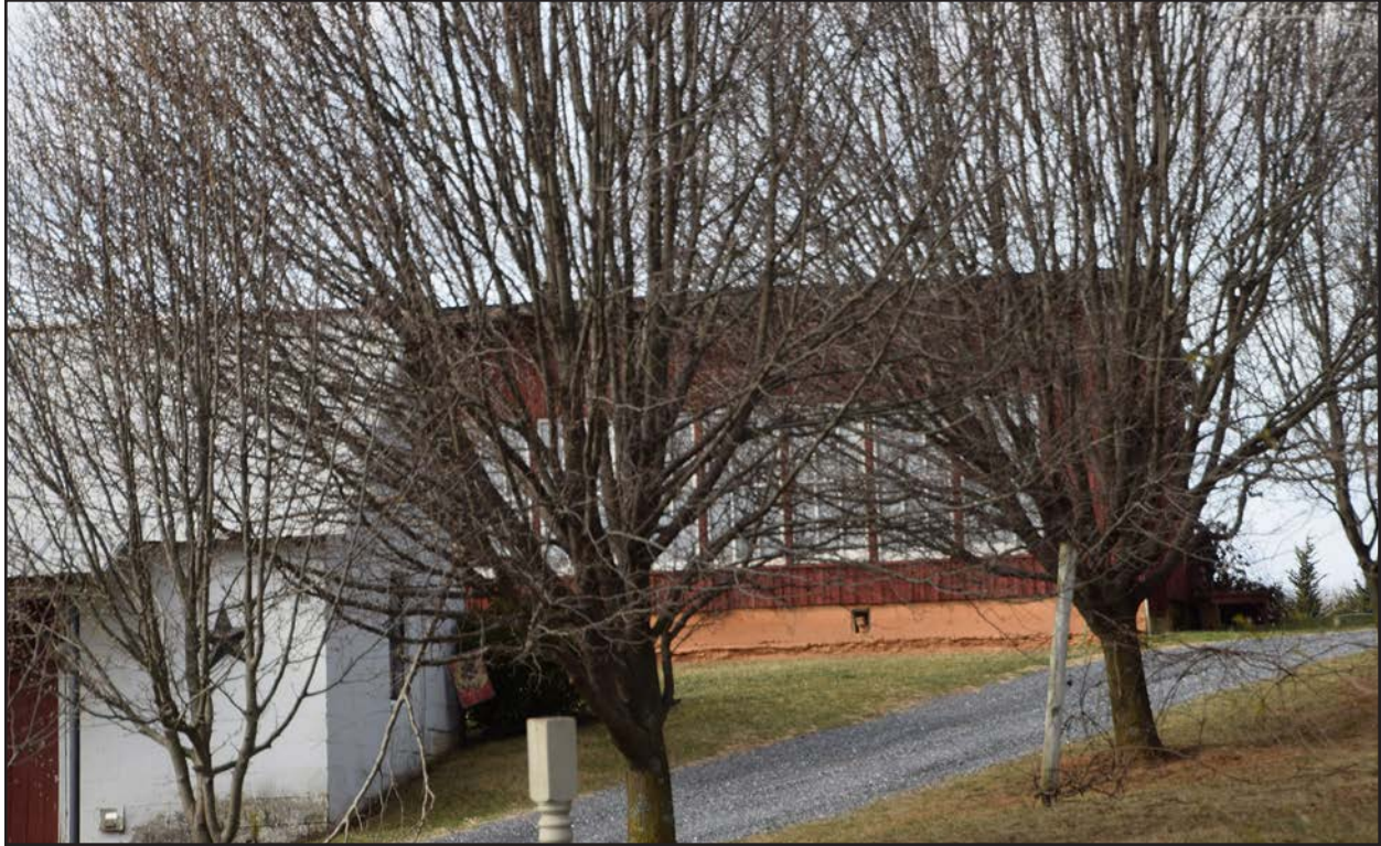
Figure 27. 007-5584, shed detail, facing northwest.
