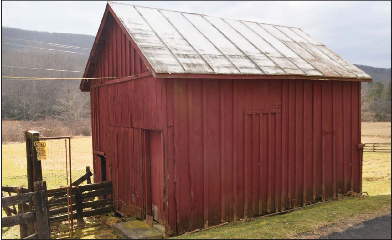
Figure 49. 008-5068, small livestock barn, facing southeast.
