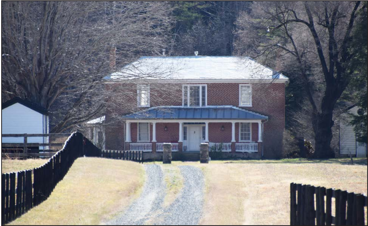
Figure 81. 062-5119-0113, house, facing south.
