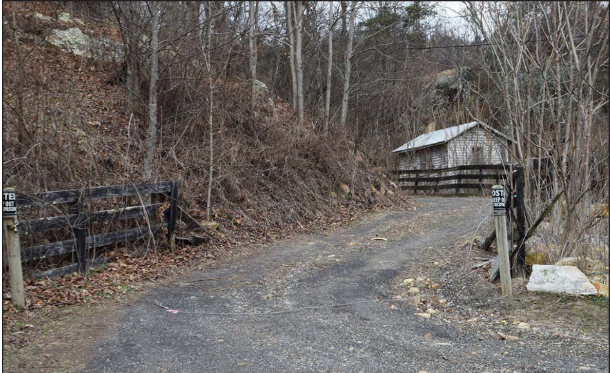
Figure 42. 008-5068, outbuildings, detail, facing northwest.
