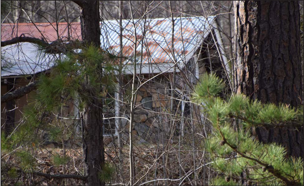
Figure 18. 007-5556, northeast addition, facing west.
