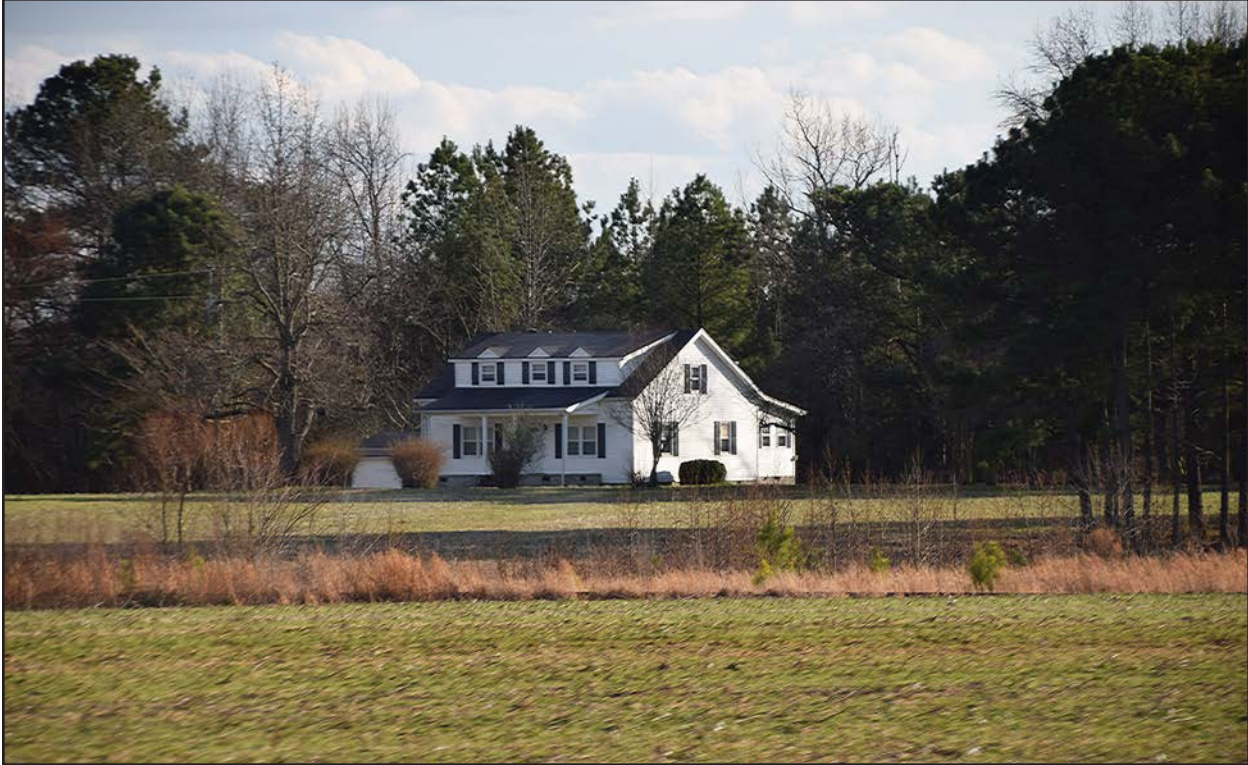
Figure 56. 012-5188, dwelling, facing southeast.
