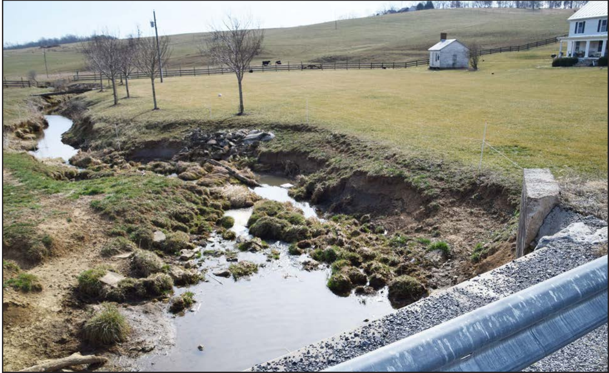
Figure 13. 007-1163, bridge, facing north.
