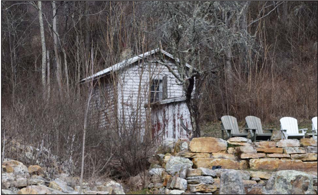
Figure 41. 008-5068, outbuildings, detail, facing northwest.
