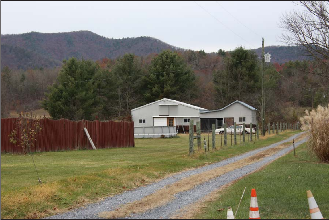
Figure 167. 007-5733, modern metal barn, facing north.
