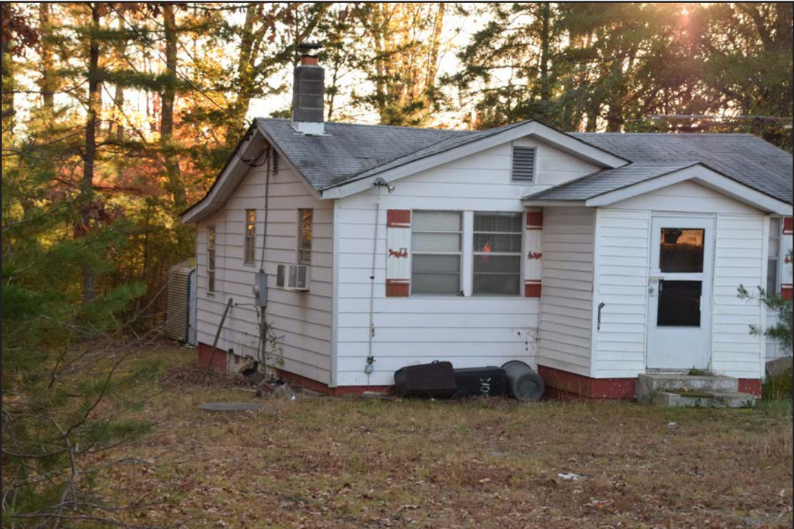
Figure 236. 026-5256, house and shed, facing southwest.
