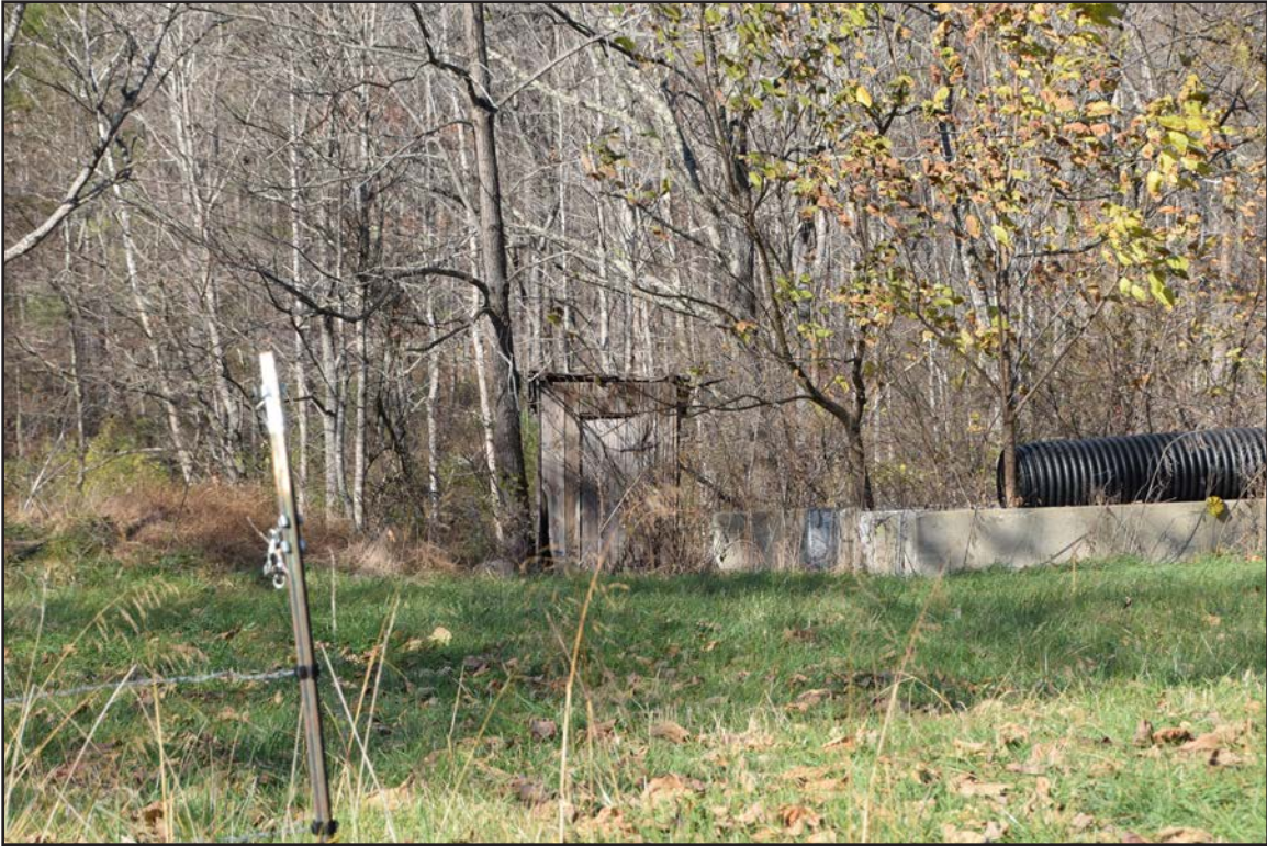
Figure 71. 007-5710, outhouse, facing northwest.
