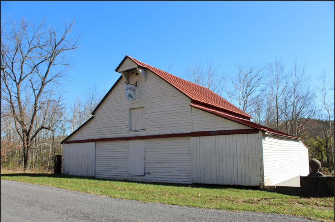
Figure 204. 008-0126, barn, facing east.
