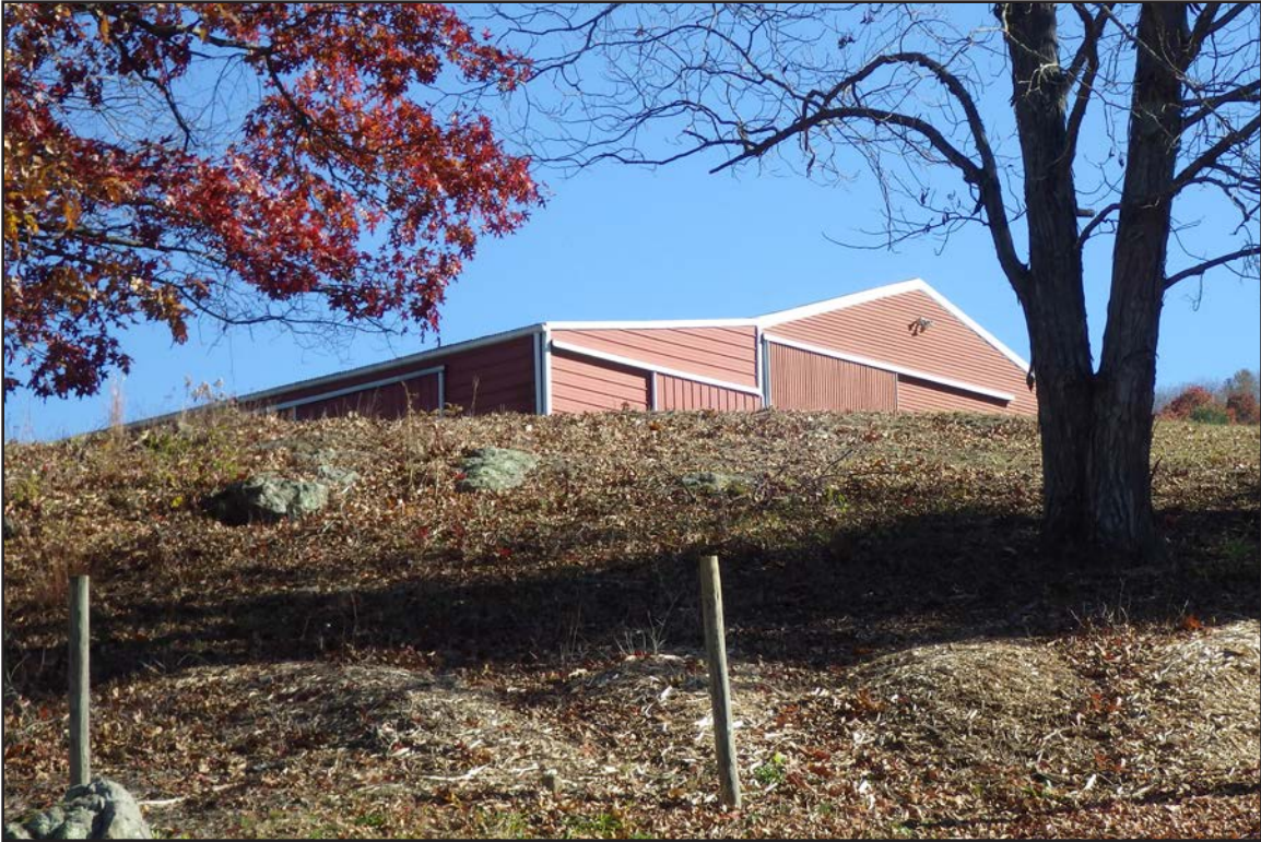
Figure 101. 007-5716, barn, facing east.
