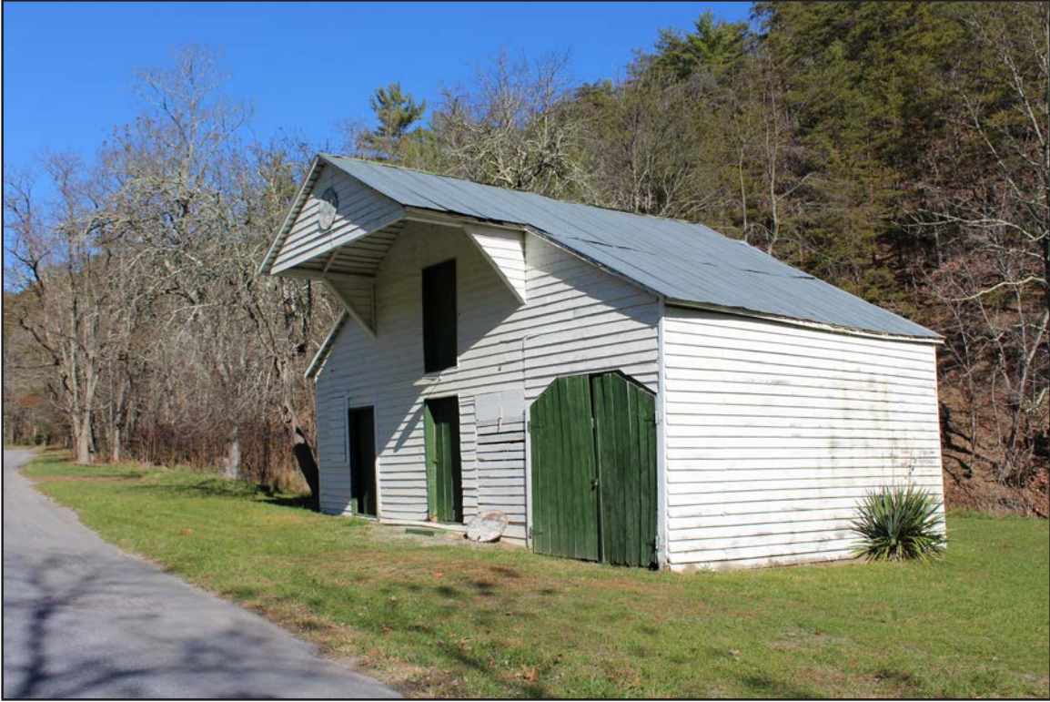
Figure 213. 008-5065, barn, facing north.
