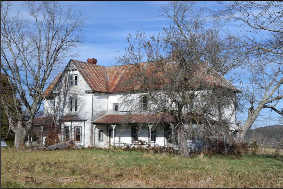
Figure 25. 007-0487, house, facing east.
