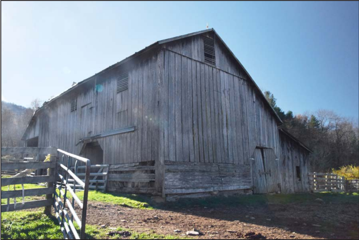
Figure 67. 007-5709, barn, facing south-southeast.
