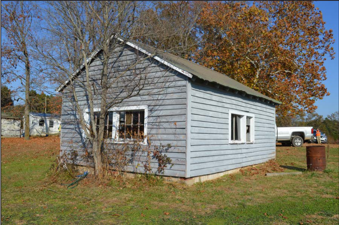
Figure 228. 014-5085, ca. 1930 outbuilding, facing northeast.
