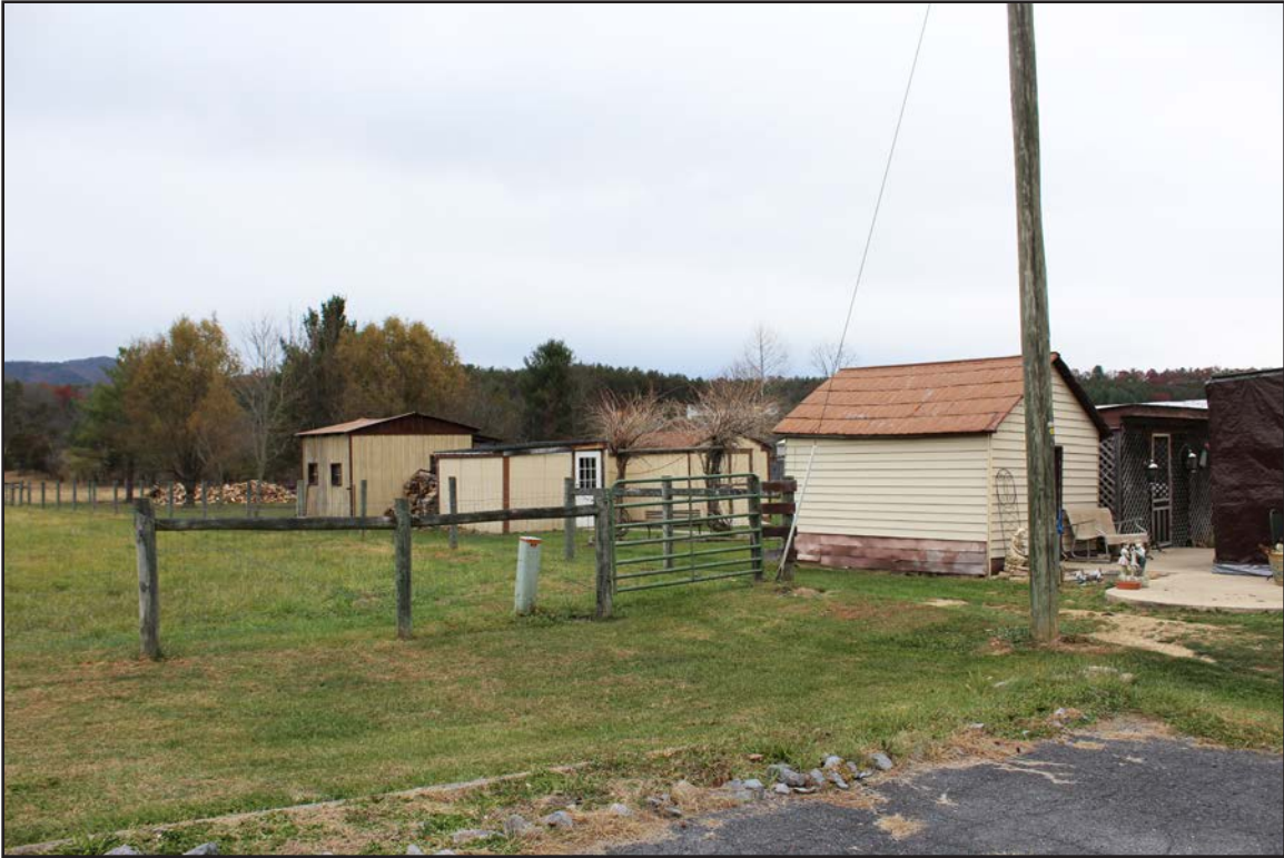
Figure 31. 007-0490, sheds, facing northeast.
