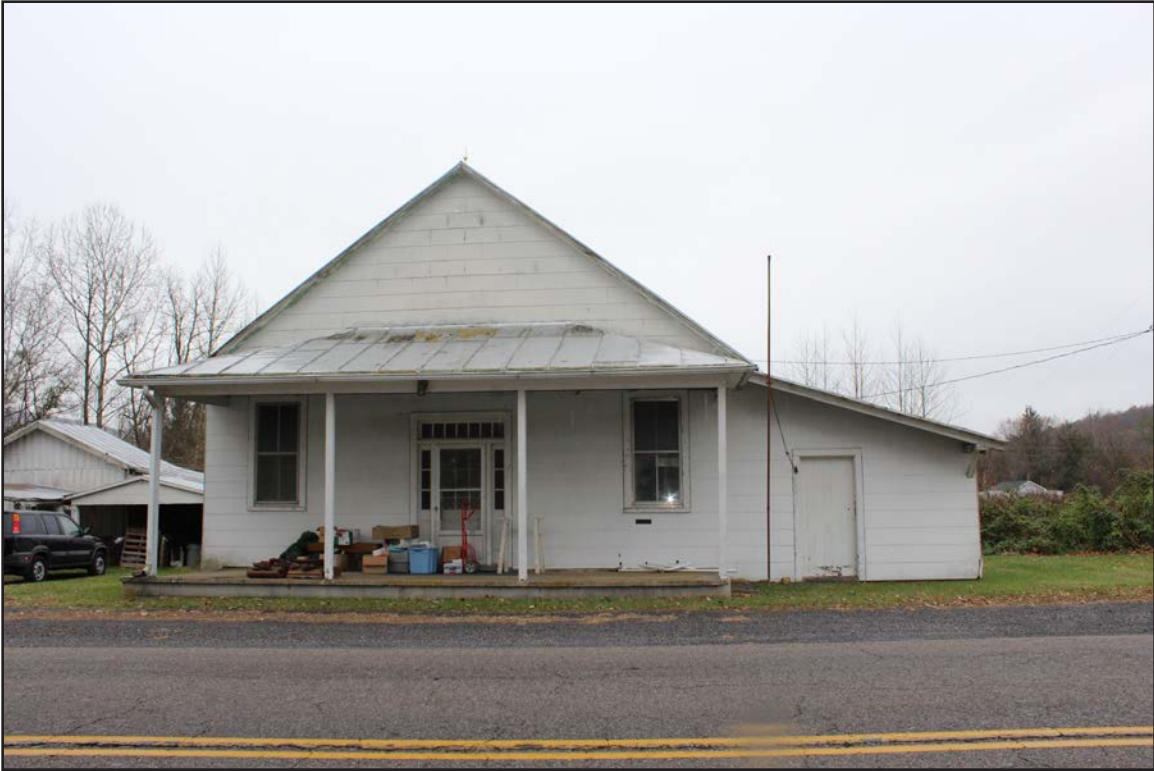
Figure 15. 007-0476, store, facing south.
