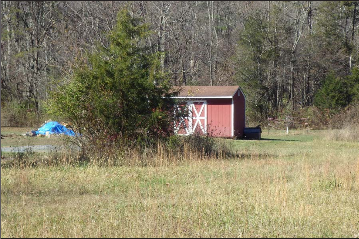
Figure 110. 007-5718, shed, facing northwest.
