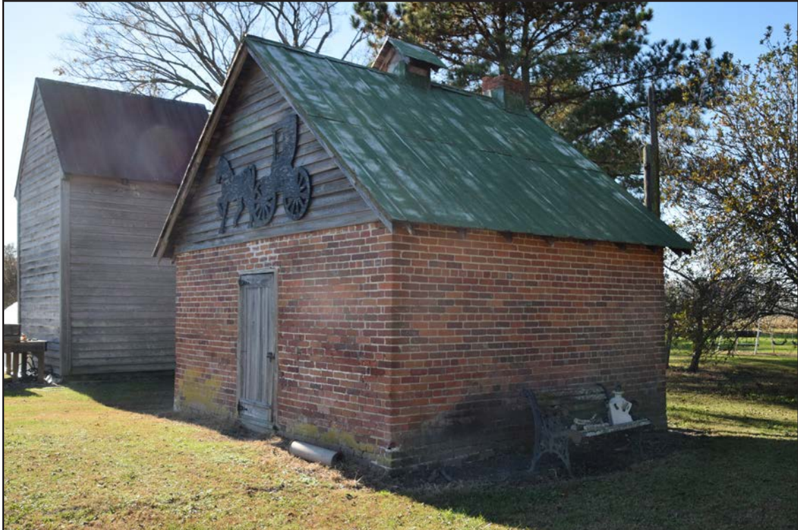
Figure 268. 133-0101, potato house, facing west.
