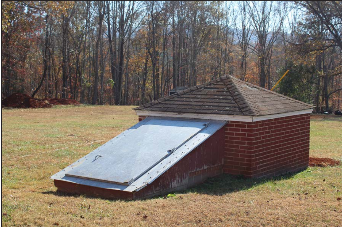
Figure 254. 062-5229, well house, facing southeast.
