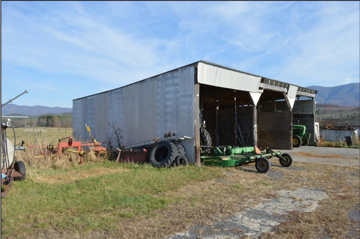
Figure 90. 007-5714, shed, facing east.
