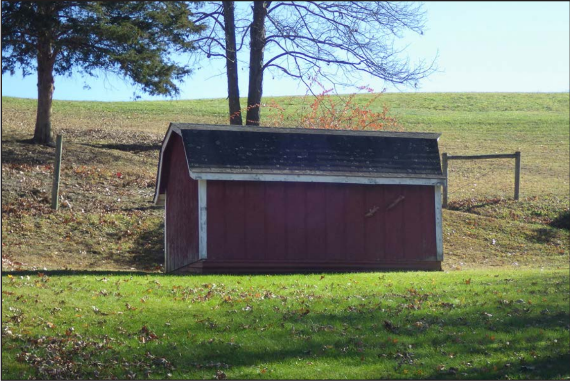
Figure 100. 007-5716, shed, facing southeast.
