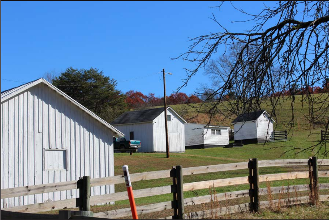
Figure 219. 008-5066, outbuildings, facing east.
