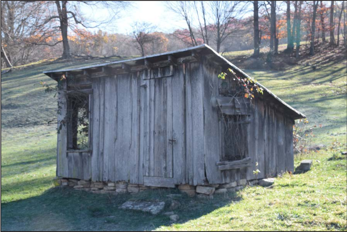
Figure 63. 007-5709, Outbuilding 2, facing southeast.
