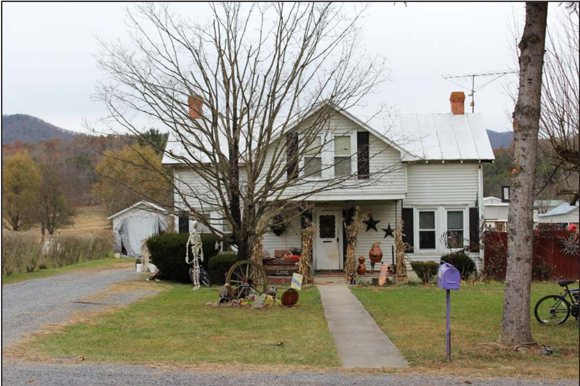
Figure 164. 007-5733, house, facing north-northwest.
