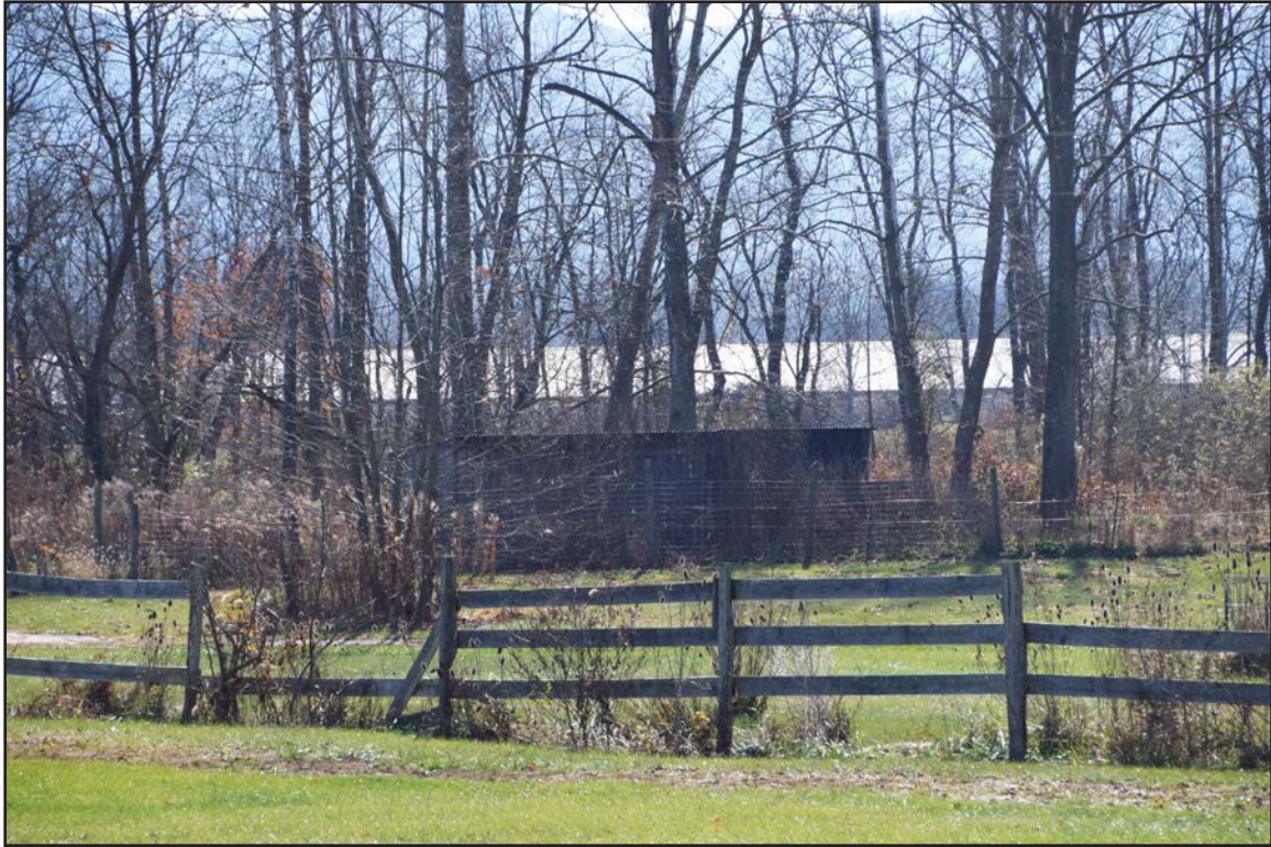
Figure 13. 007-0467, chicken house, facing southwest.
