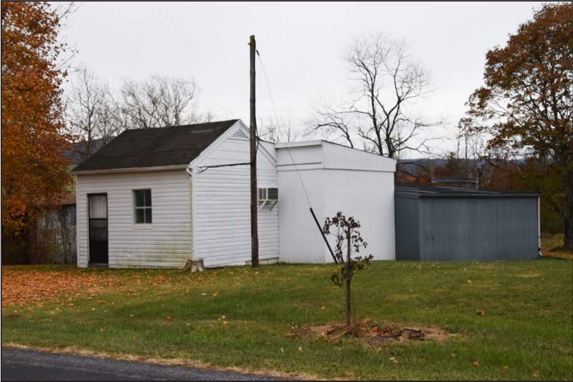
Figure 121. 007-5721, building, facing southwest.
