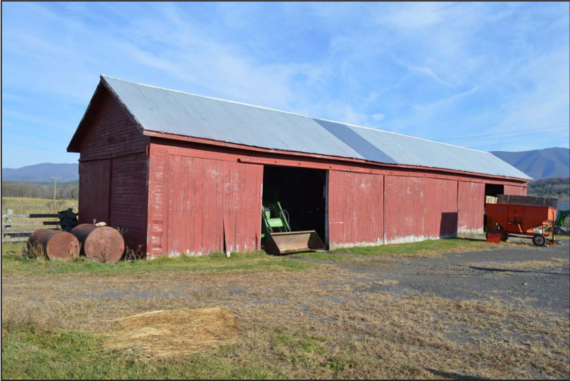
Figure 89. 007-5714, barn, facing east.
