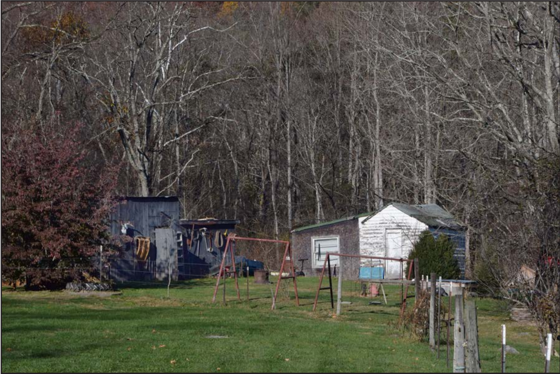
Figure 83. 007-5712 Shed 2 and Shed 3, facing west.
