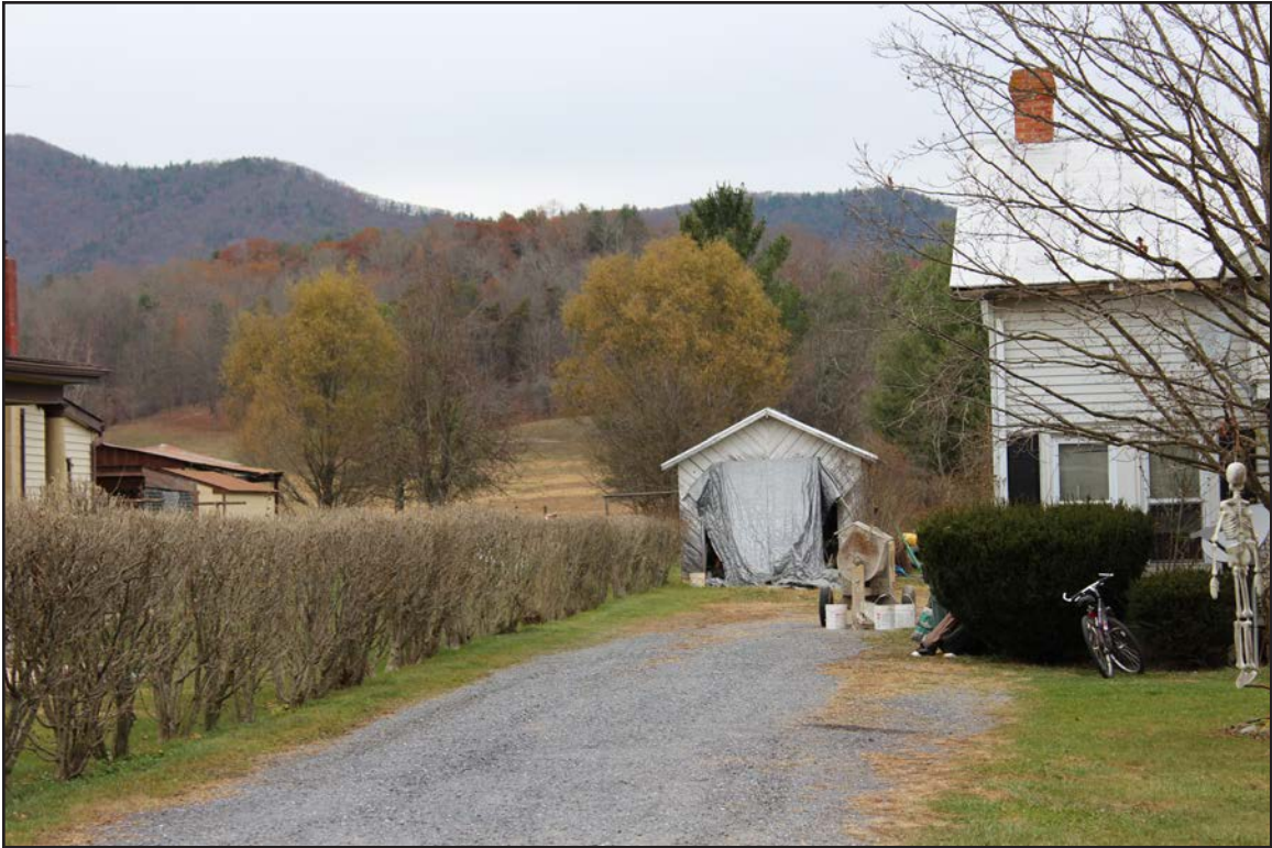
Figure 163. 007-5733, garage, facing north.
