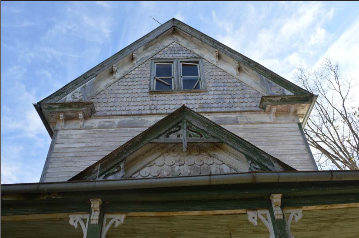
Figure 26. 007-0487, gable details on house, facing southeast.
