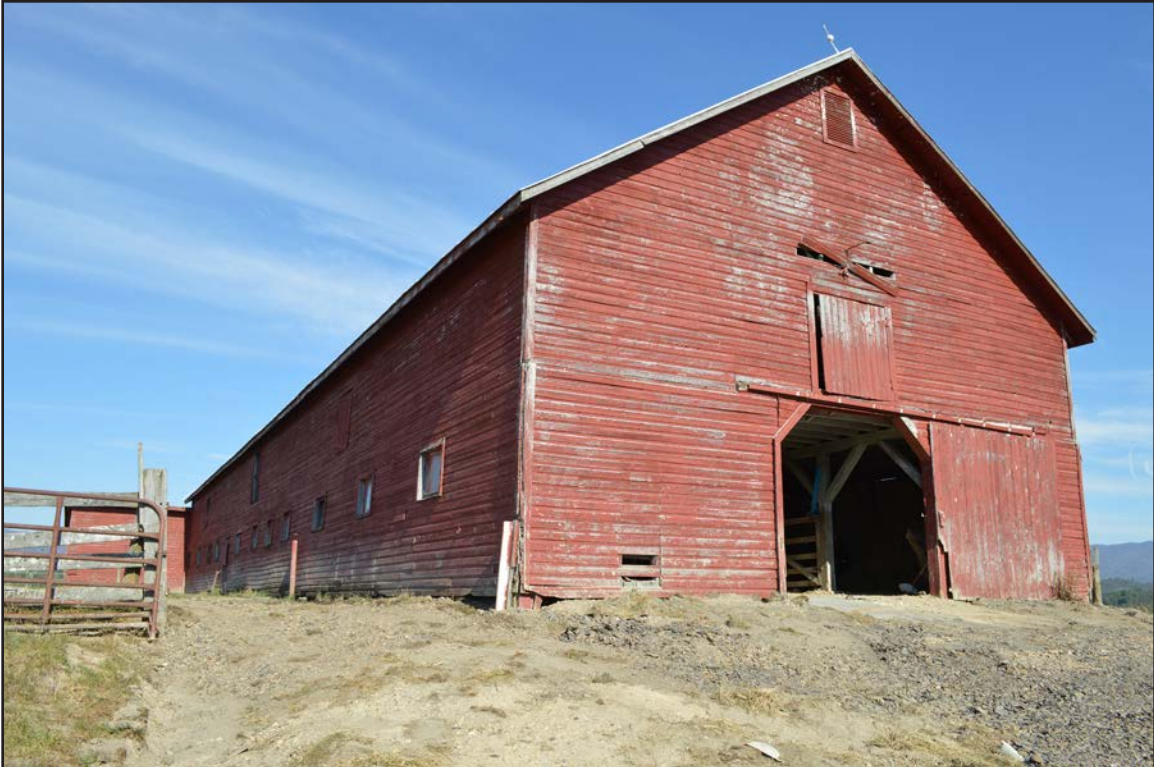
Figure 8. 007-0463, Barn 2, facing northeast.
