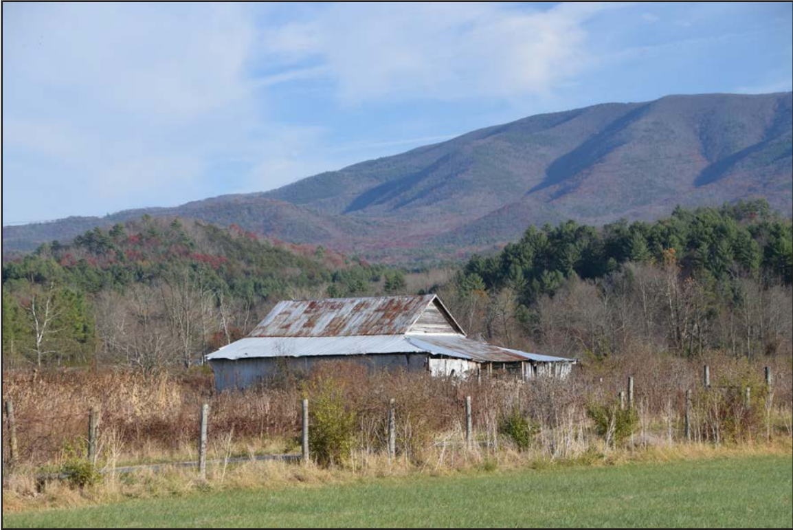
Figure 147. 007-5728, barn, facing east.
