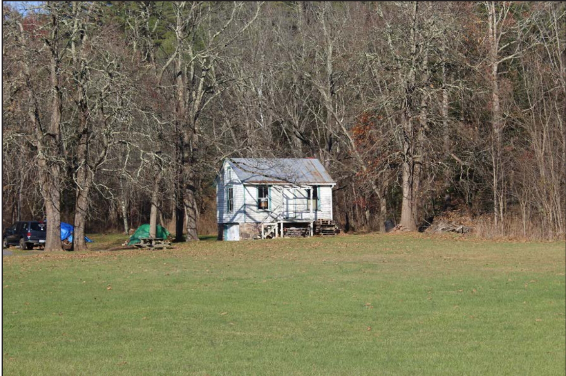
Figure 4. 007-0447. Outbuilding 1, facing southeast.
