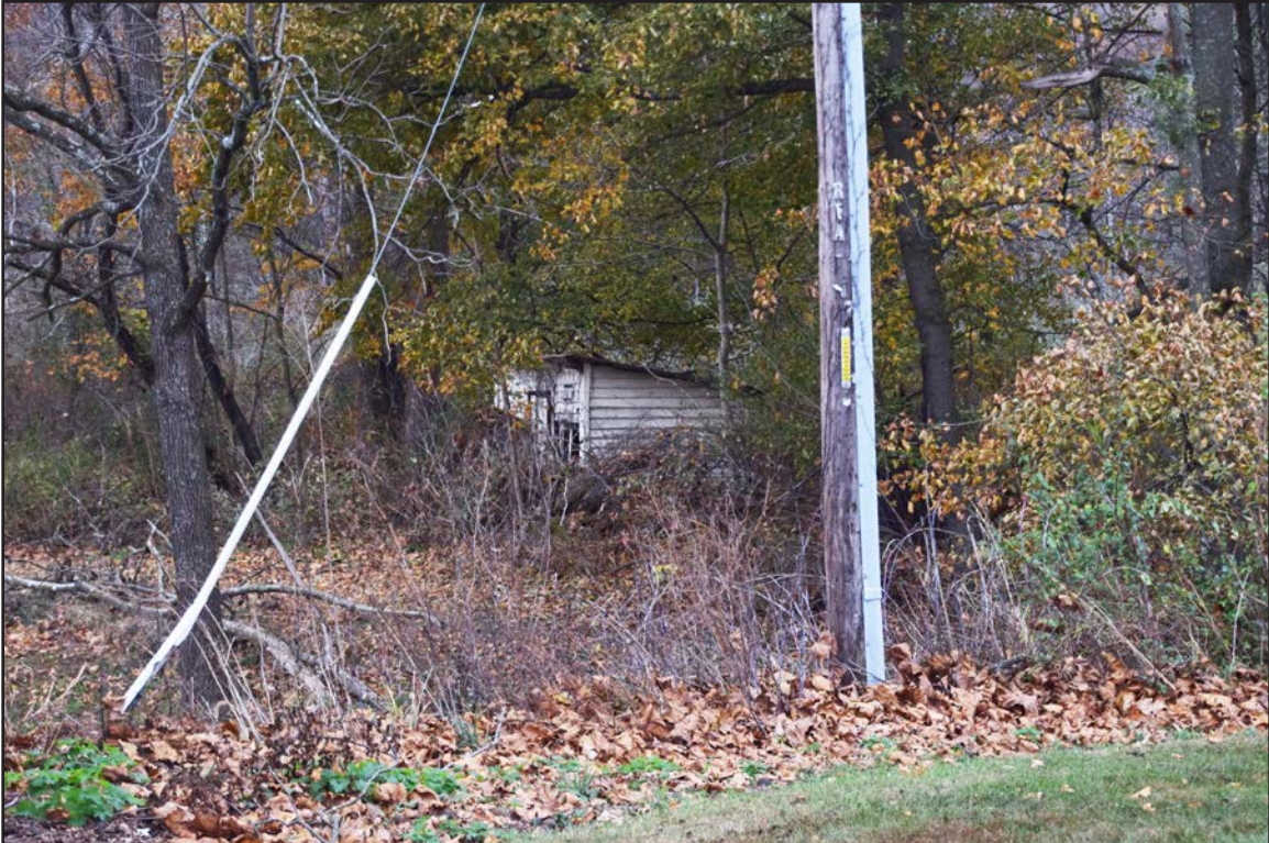
Figure 118. 007-5720, facing south by southwest.
