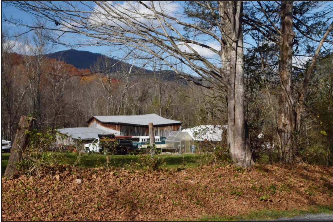
Figure 75. 007-5711, carport, barn, and Outbuilding 3, facing northeast.
