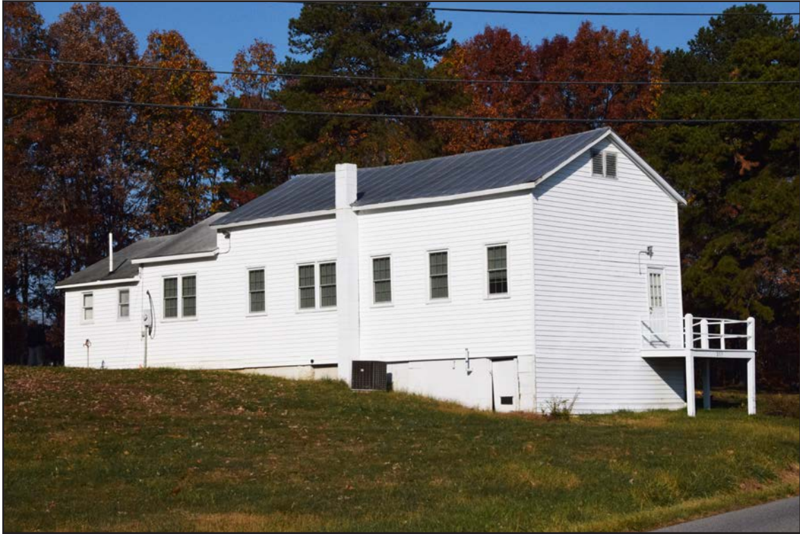
Figure 149. 007-5729, church, facing northwest.
