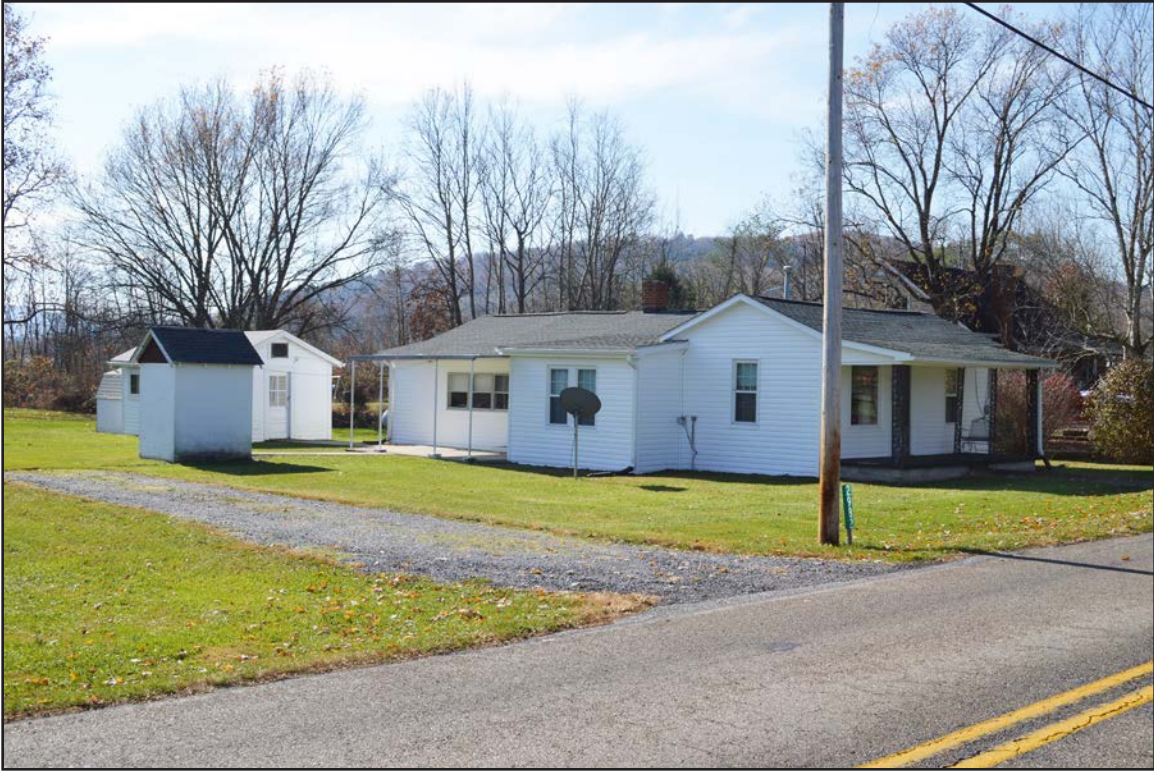
Figure 42. 007-5704, house and outbuildings, facing southwest.
