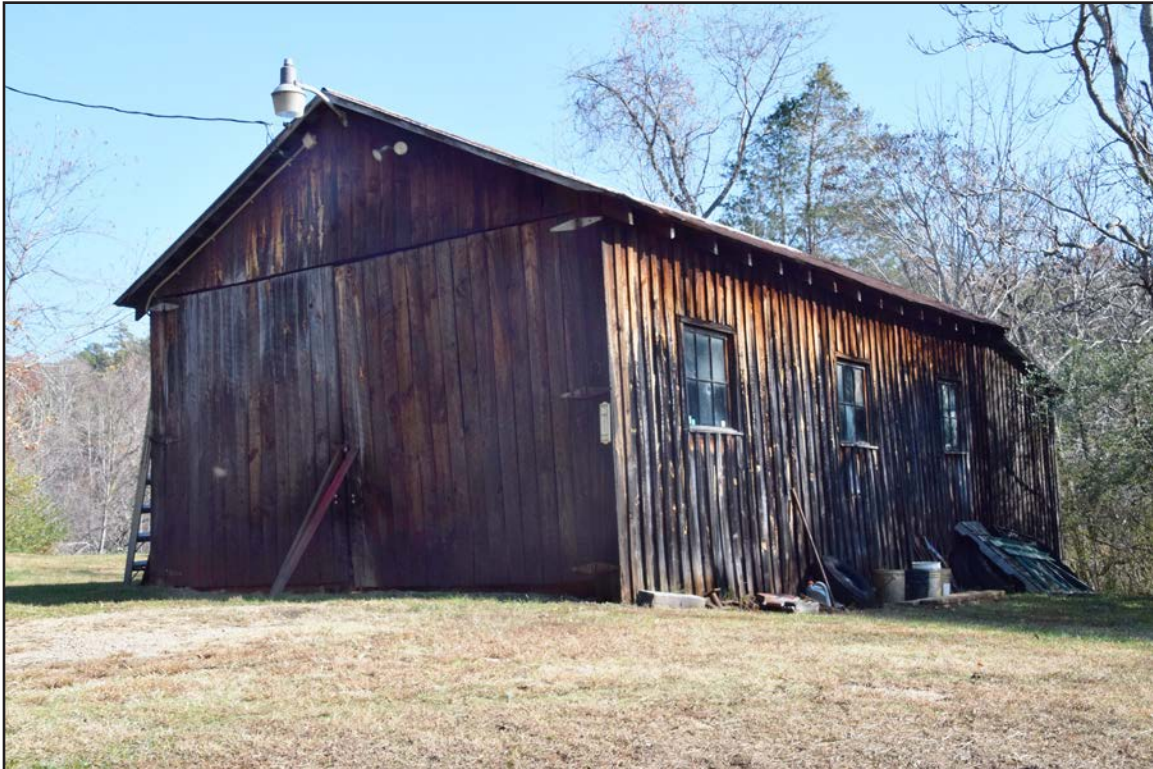
Figure 248. 062-5223, garage, facing southeast.
