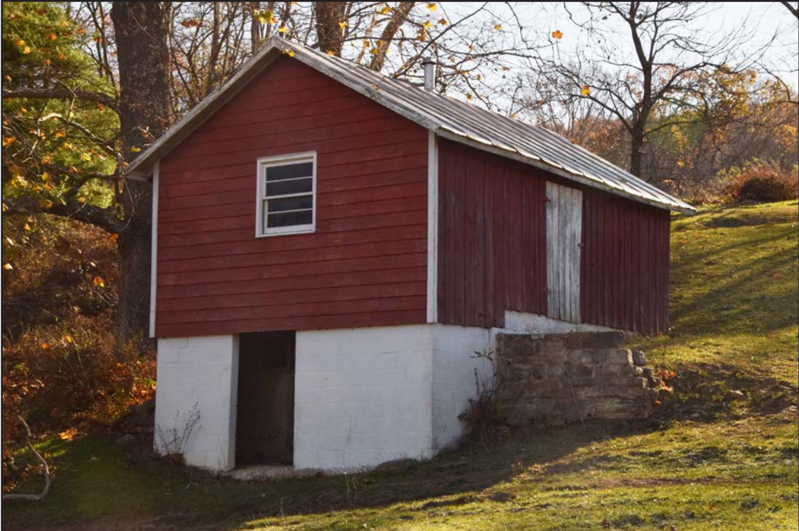
Figure 62. 007-5709, Outbuilding 1, facing southeast.
