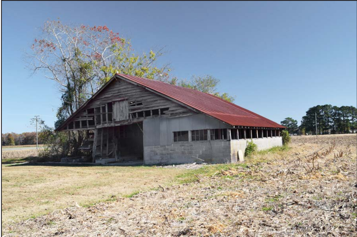
Figure 276. 133-5443, barn, facing east.
