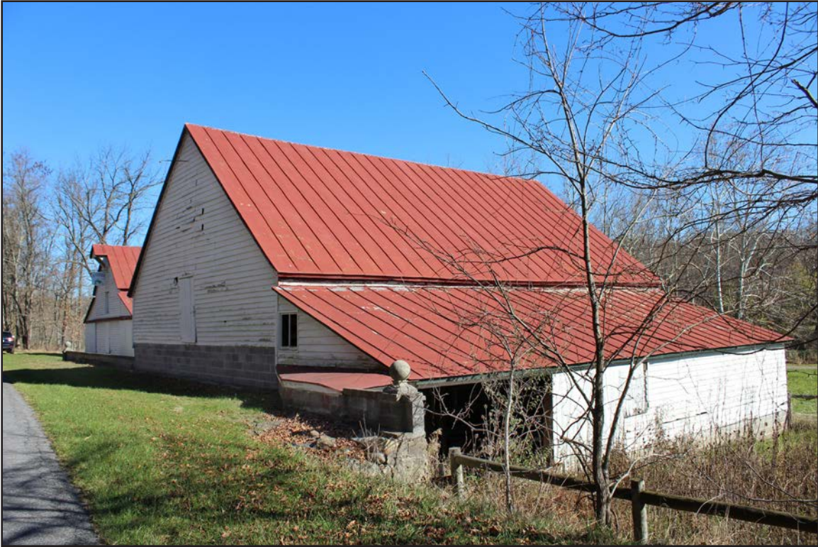
Figure 205. 008-0126, barn, facing northeast.
