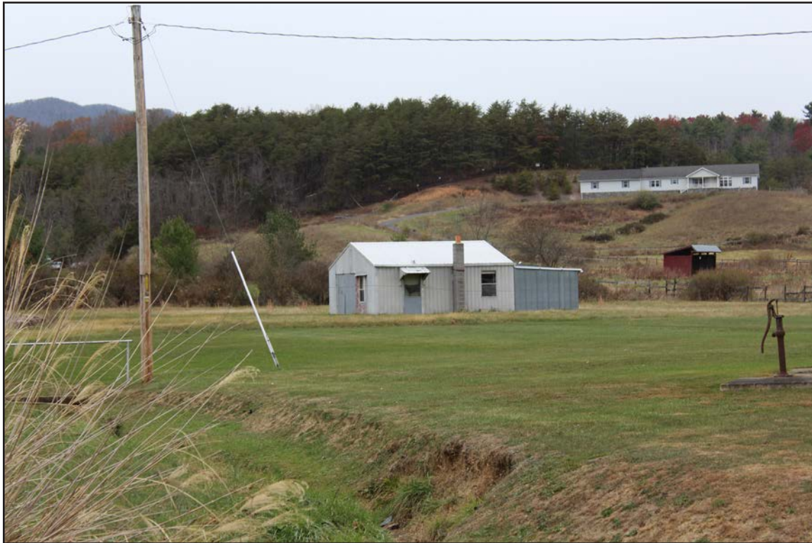
Figure 177. 007-5736, outbuilding, facing northeast.
