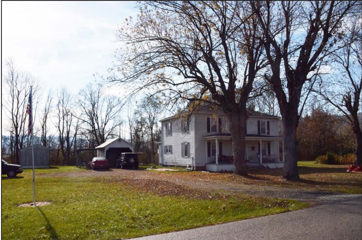
Figure 136. 007-5725, house and outbuildings, facing southwest.
