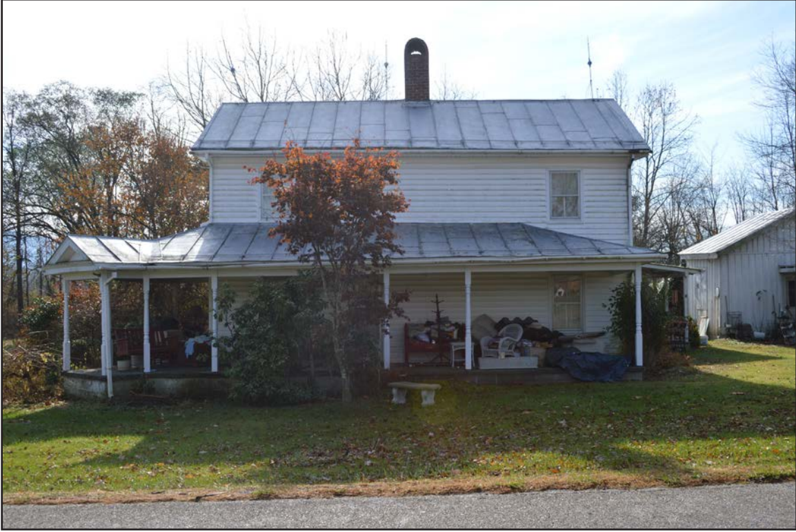
Figure 20. 007-0476, dwelling house, facing south-southwest.
