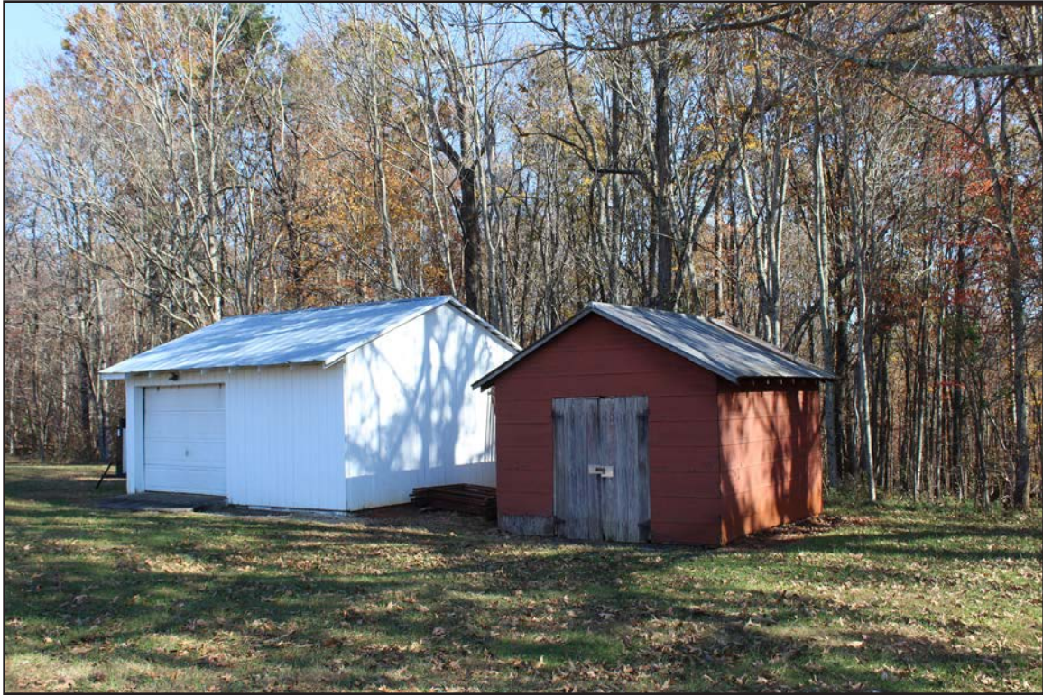
Figure 253. 062-5229, Shed 1 and Shed 2, facing northeast.
