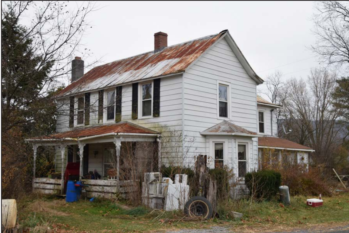
Figure 130. 007-5724, house, facing east.
