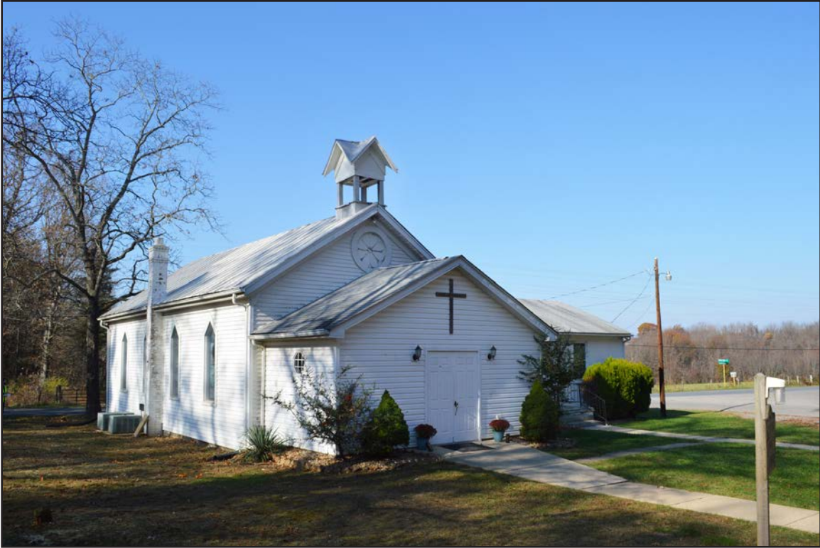
Figure 34. 007-0863, church, facing southwest.
