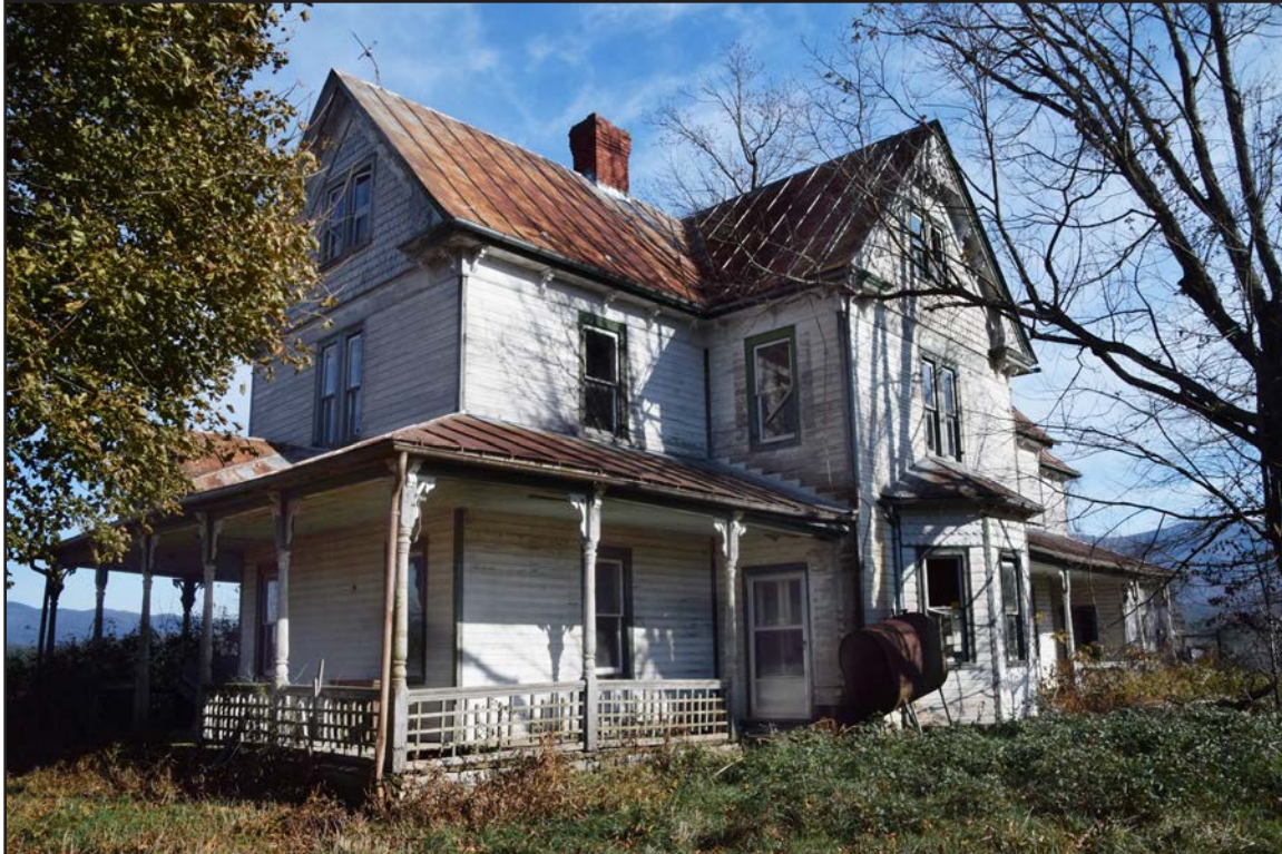
Figure 24. 007-0487, house, facing north.
