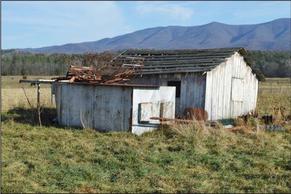
Figure 91. 007-5714, shed, facing southeast.
