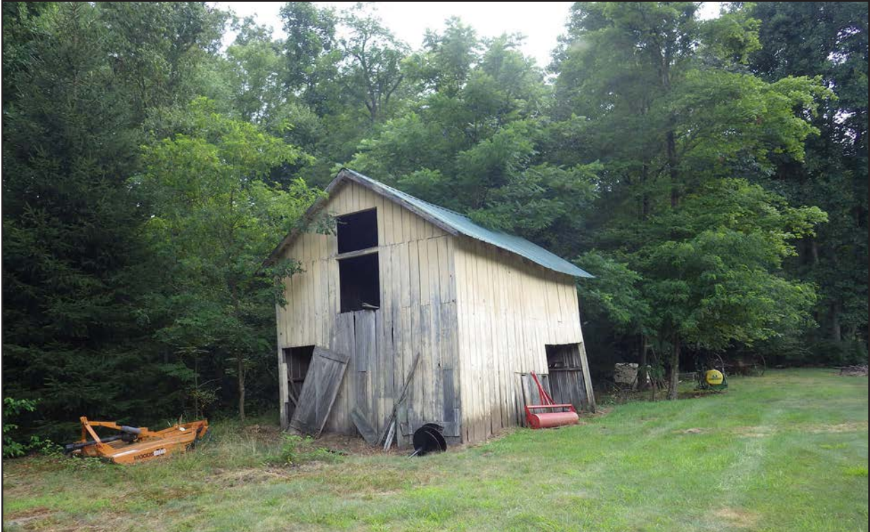
Figure 130. 008-5053, barn, facing west-southwest.
