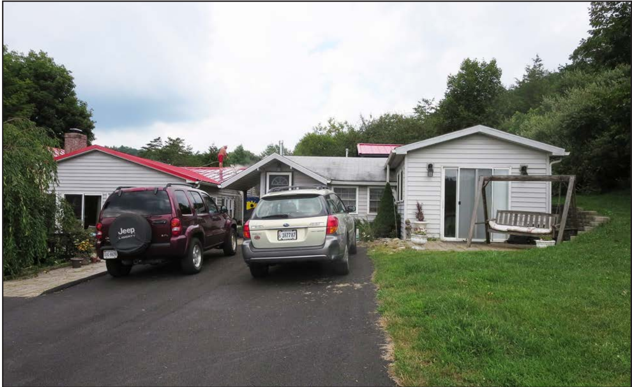
Figure 101. 007-5693, accessory building, facing northwest.
