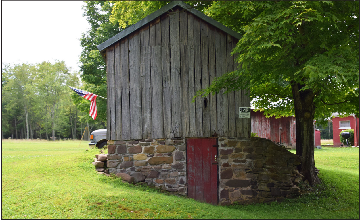
Figure 77. 007-5688, root cellar, facing south.
