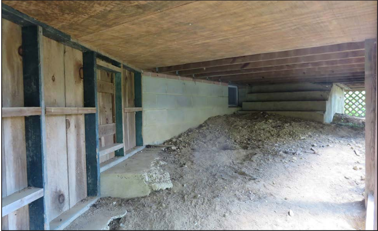
Figure 155. 008-5062, beneath front porch, facing south.
