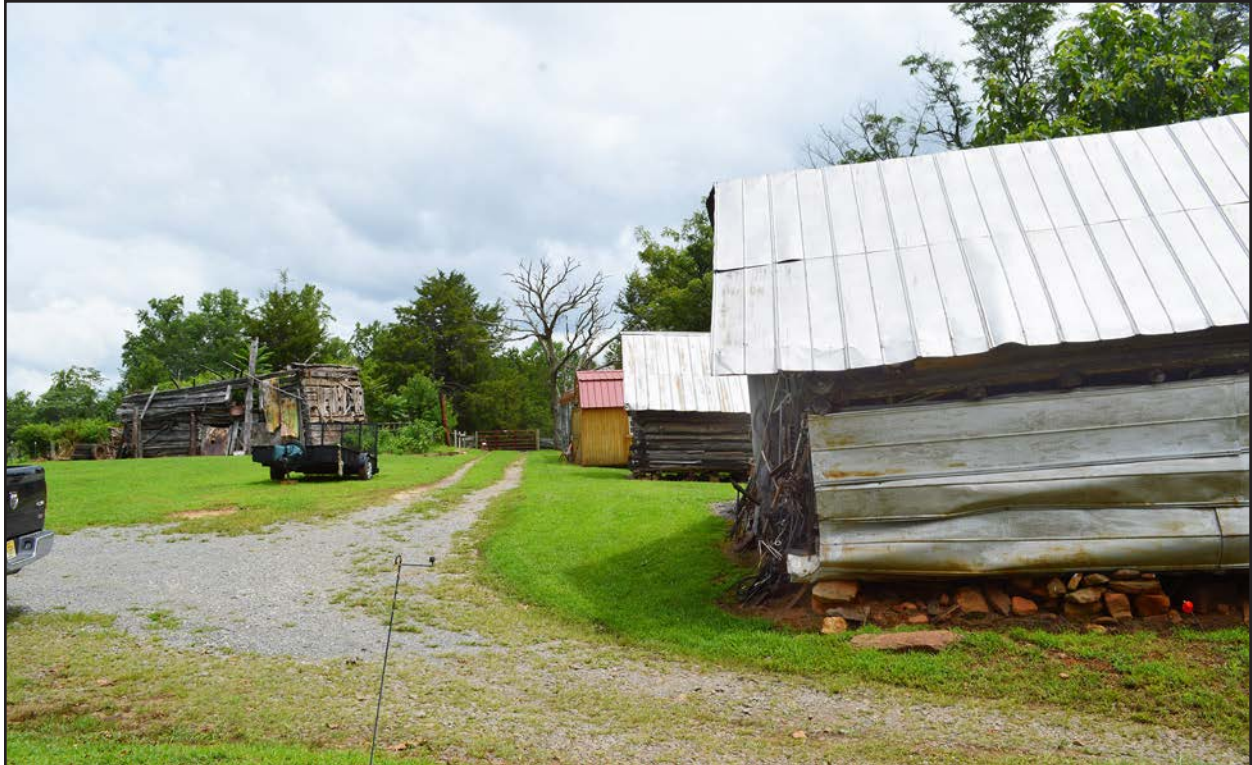
Figure 232. 062-5222, overview of outbuildings northeast of house, facing northeast.
