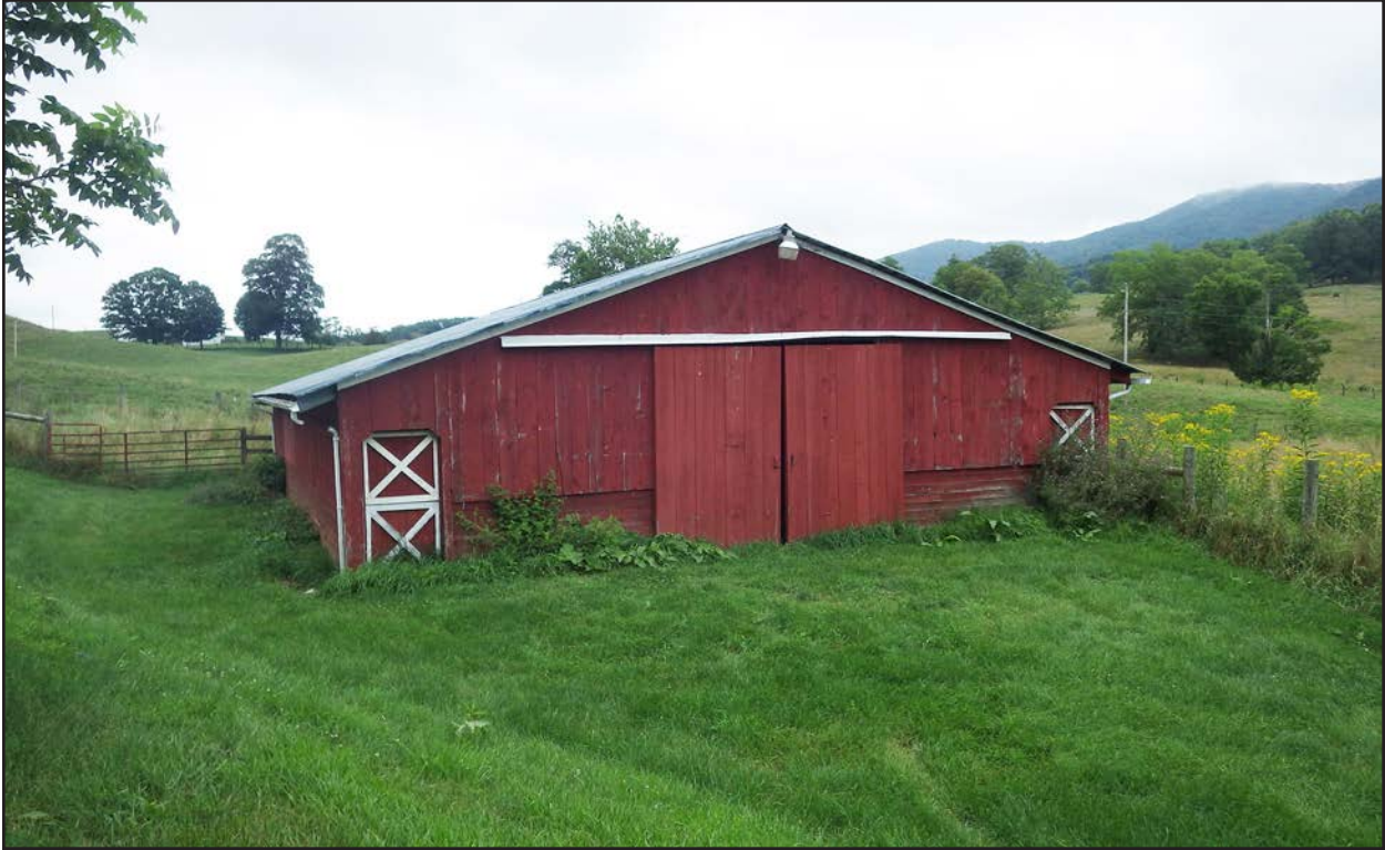
Figure 177. 045-0055, barn 3, facing east.
