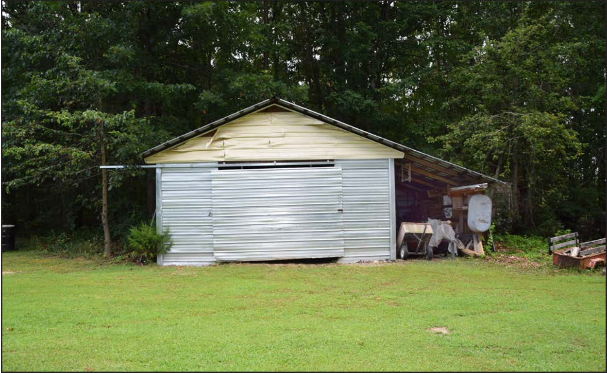
Figure 45. 007-5569, shed, view south.
