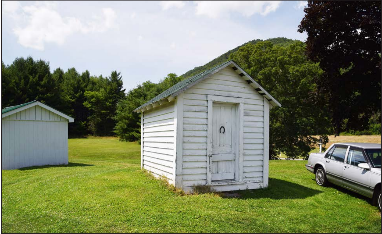
Figure 203. 045-5081, shed 1, facing northwest.
