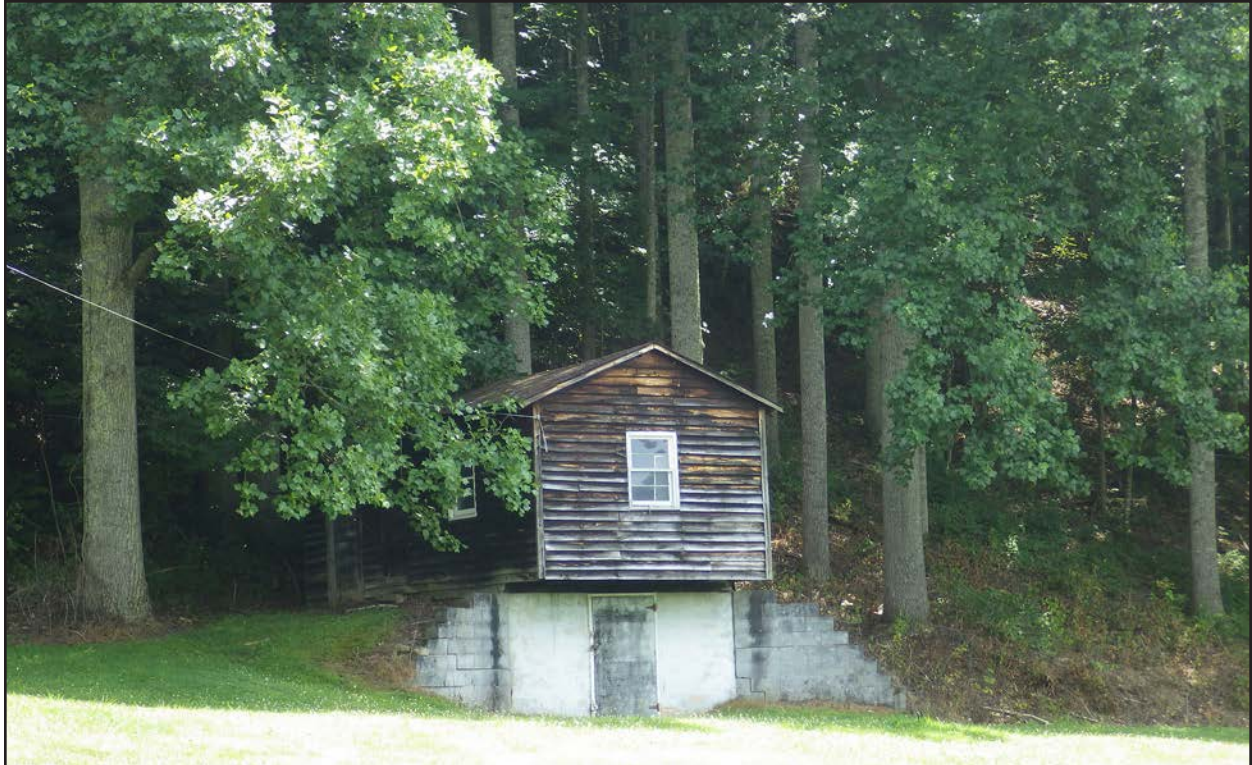
Figure 58. 007-5683, root cellar, facing south.
