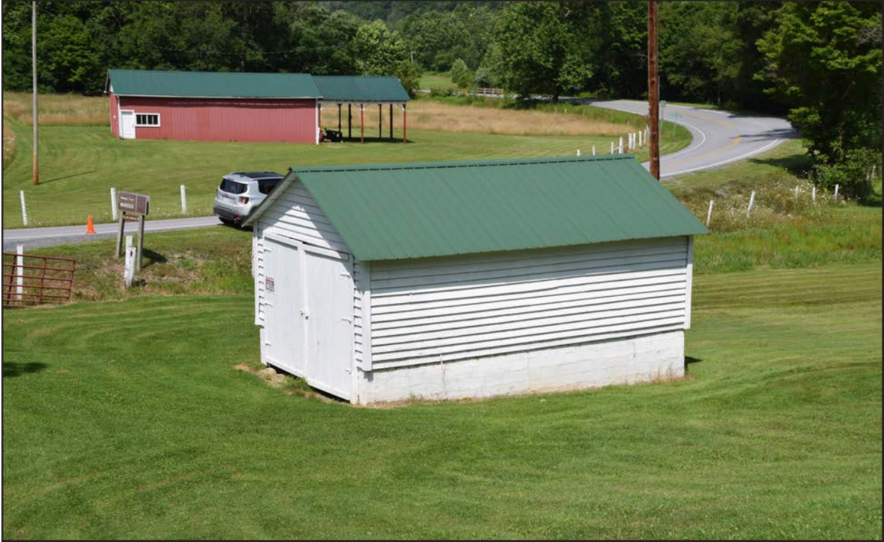
Figure 205. 045-5081, shed 3, facing east.
