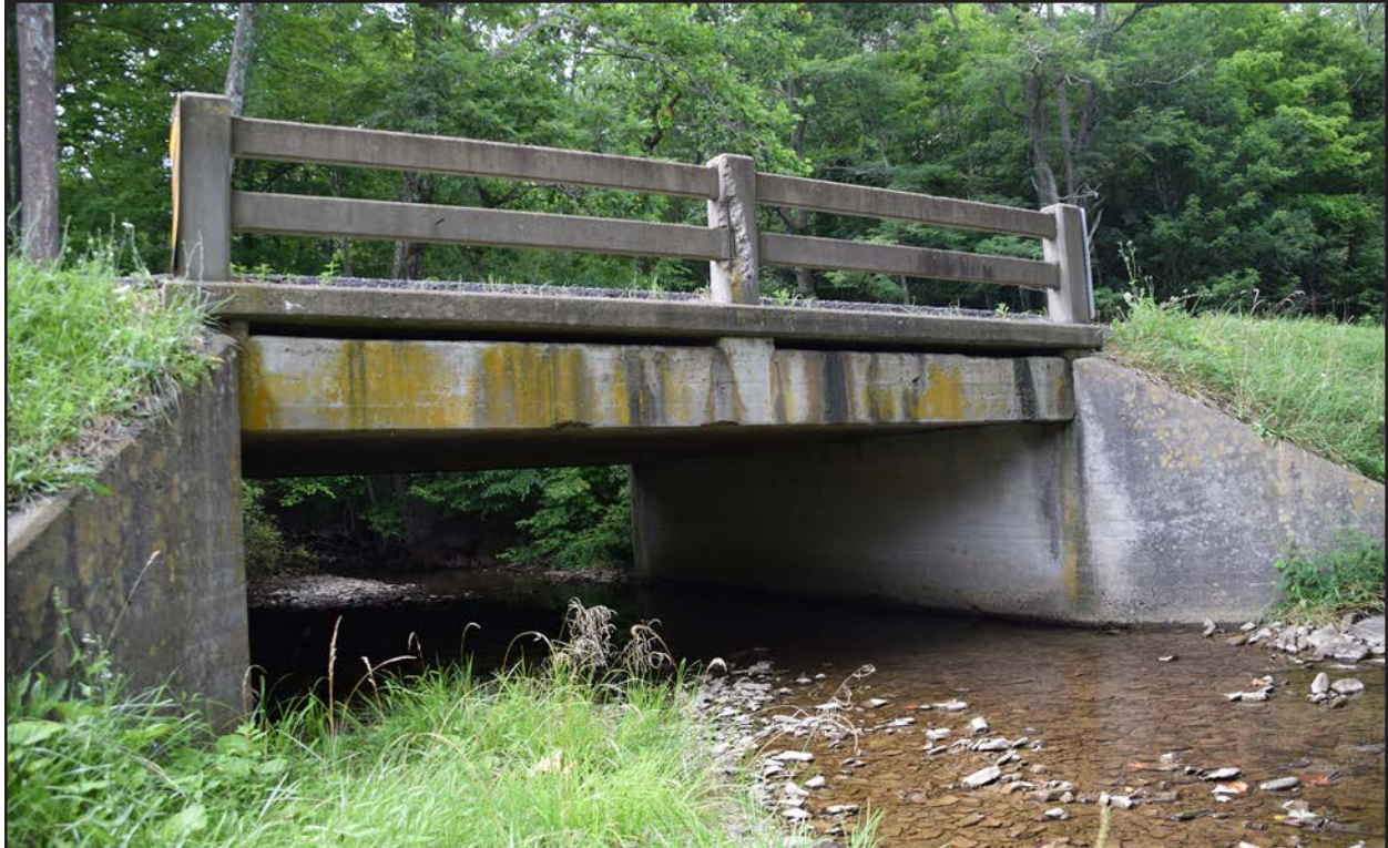
Figure 186. 045-5013, view of bridge, facing northwest.
