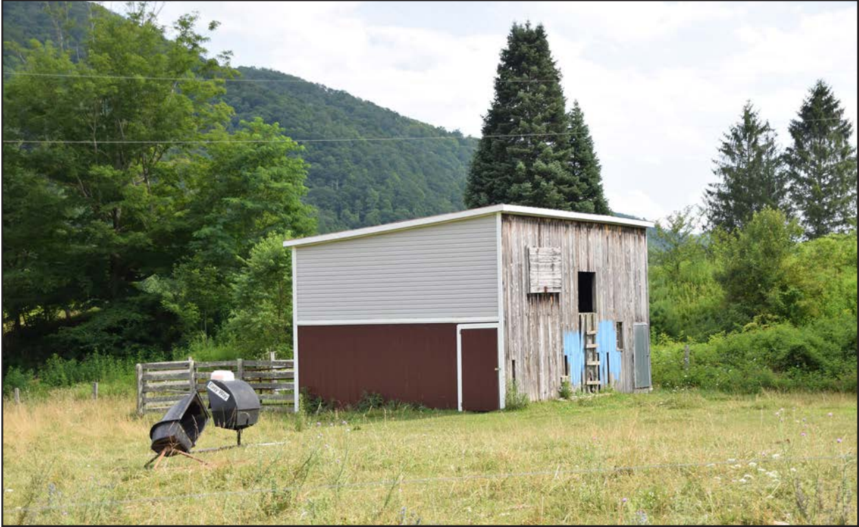
Figure 215. 045-5084, view of barn, facing east.
