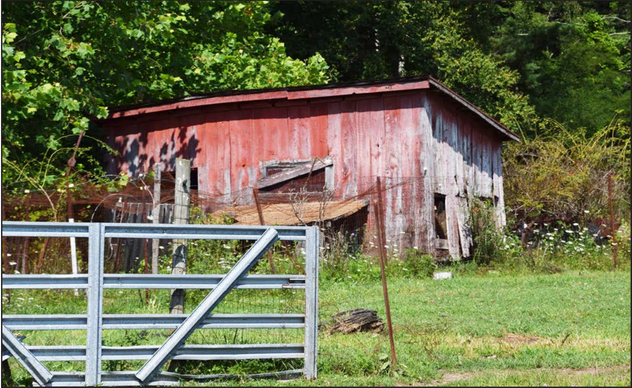
Figure 89. 007-5691, shed 3, facing northwest.
