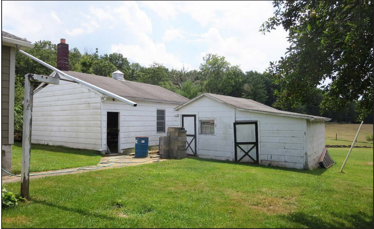
Figure 139. 008-5056, garage and accessory building, facing south.
