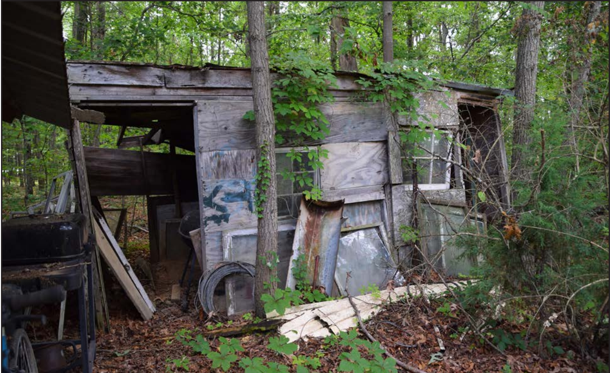
Figure 46. 007-5569, outbuilding, view south.
