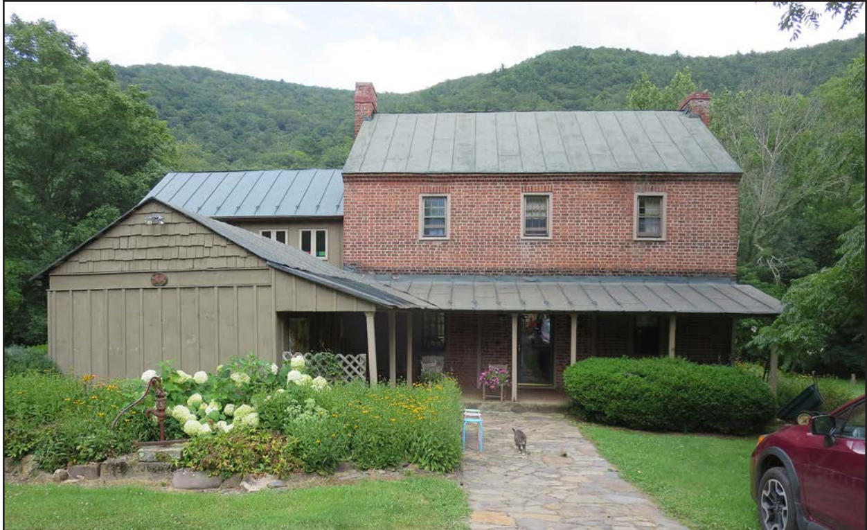
Figure 166. 045-0007, view of west elevation, facing east.
