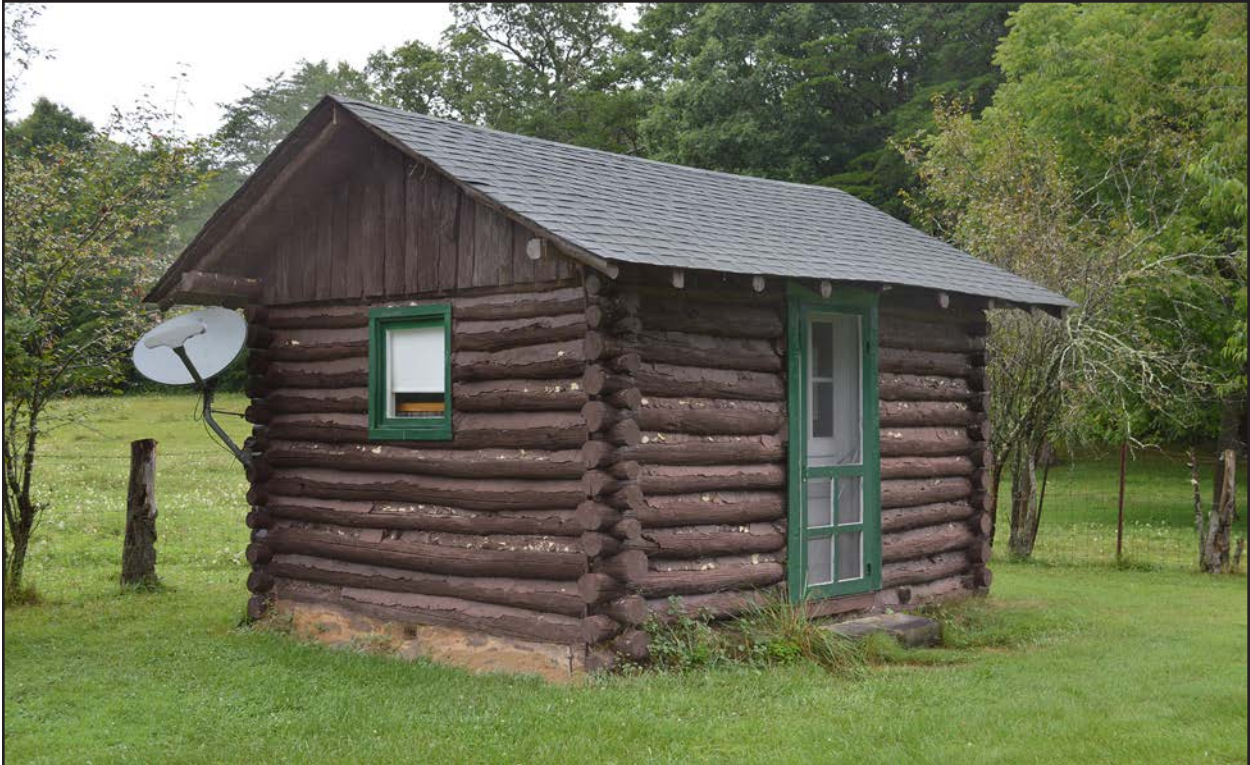
Figure 124. 007-5699 log cabin, facing north.
