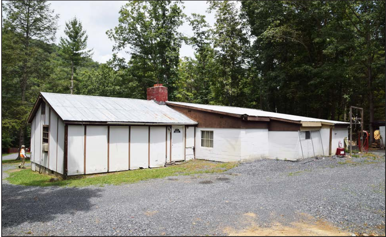
Figure 141. 008-5058, rear of house, facing northeast.
