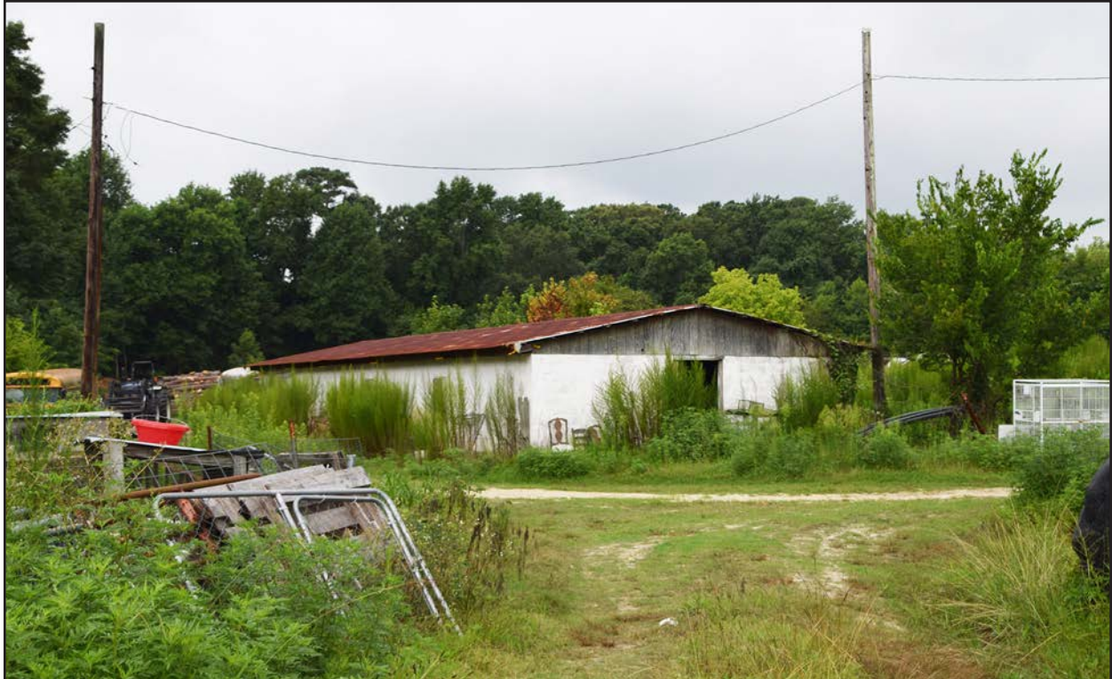
Figure 242. 133-0215 historic barn 1, facing southeast.
