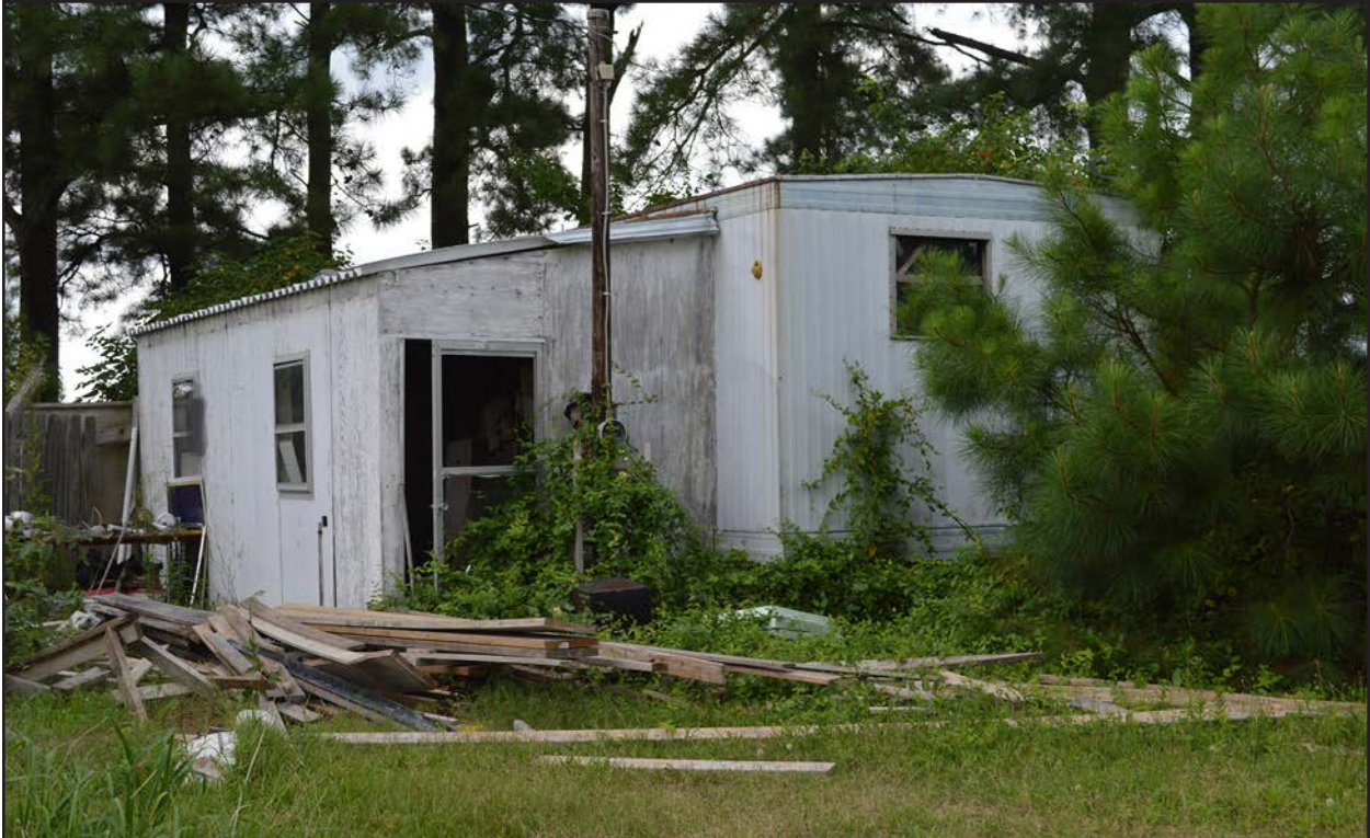
Figure 256. 133-5444, mobile home facing west.
