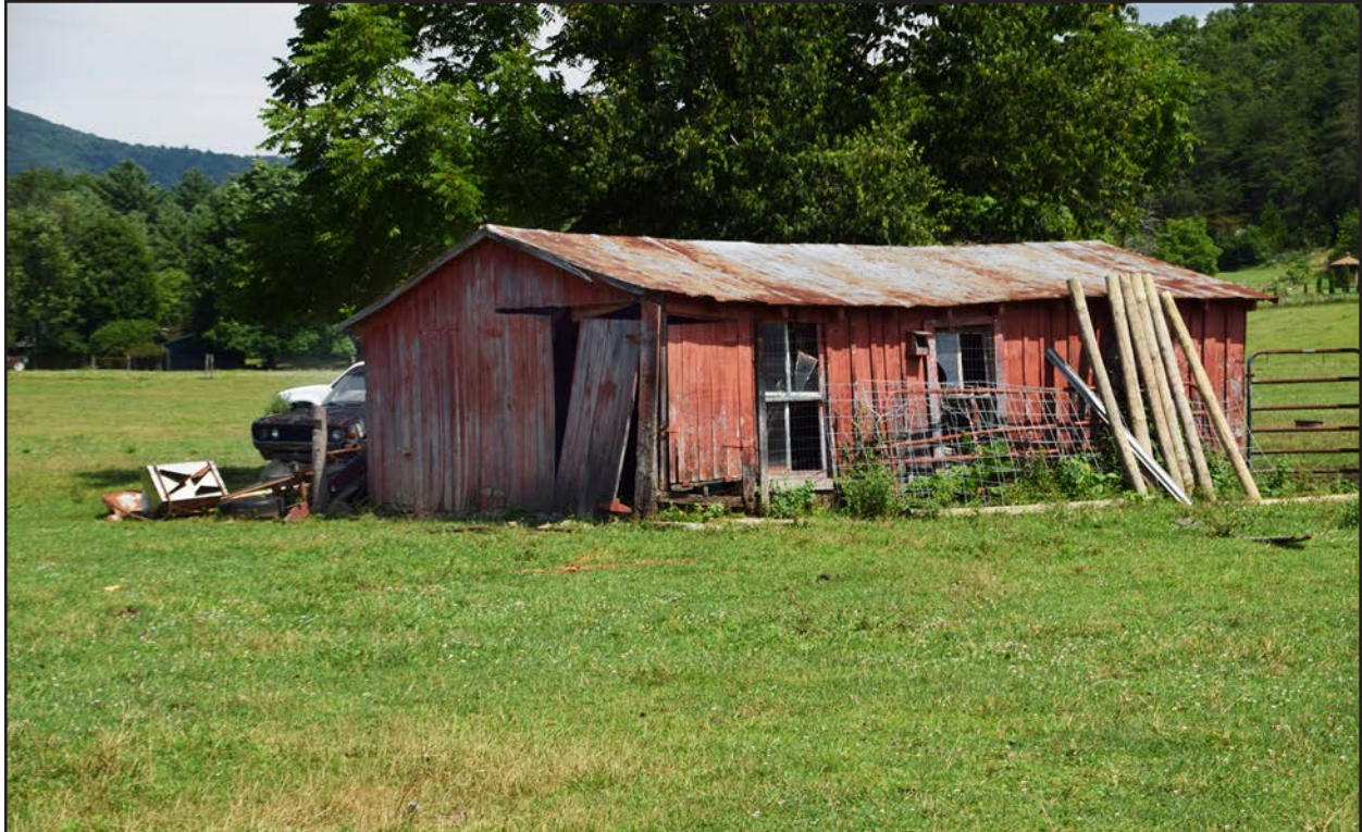
Figure 88. 007-5691, shed 2, facing northeast.
