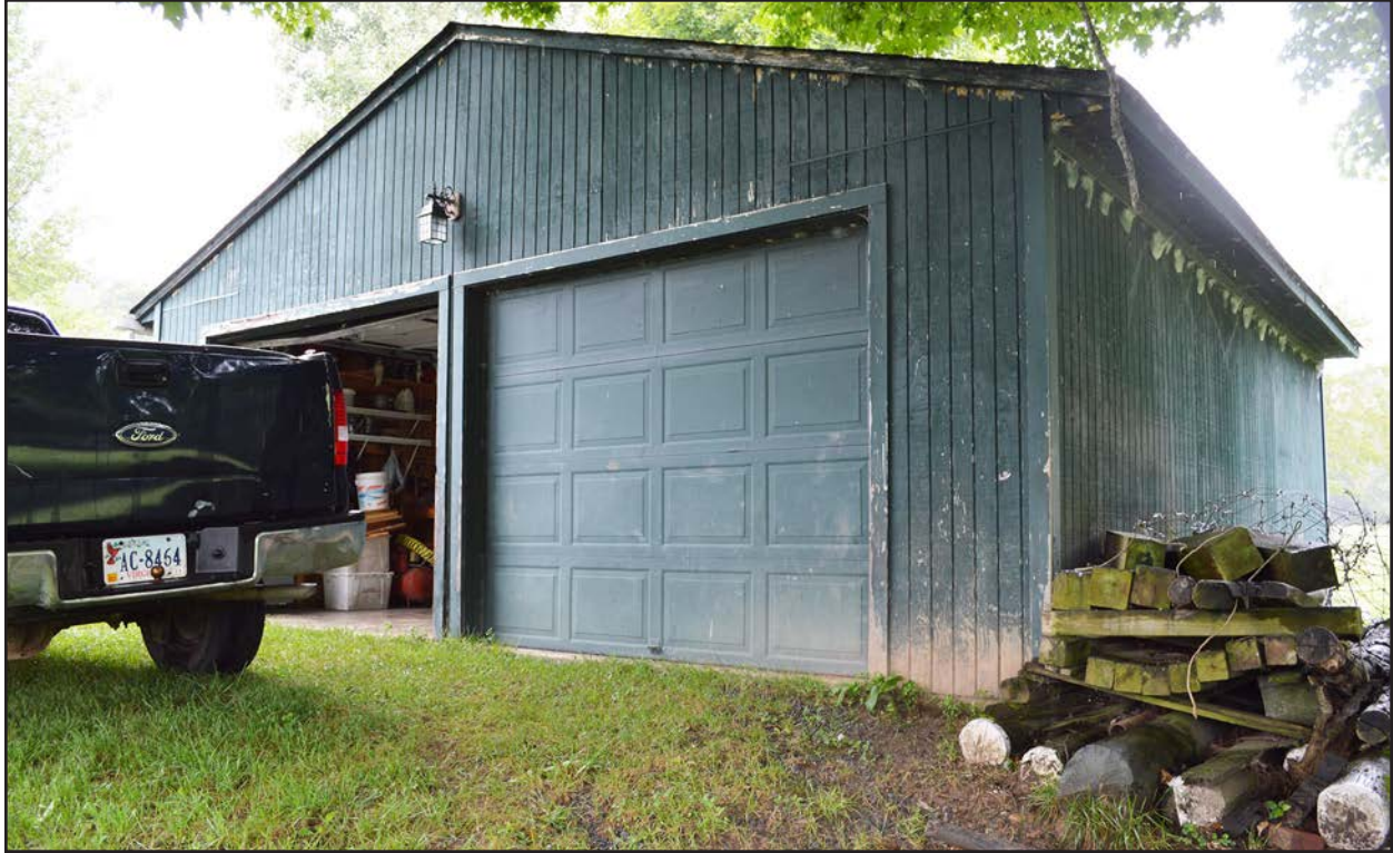
Figure 127. 007-5699 garage, facing southwest.
