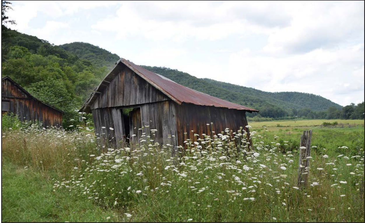
Figure 211. 045-5082, shed facing north.
