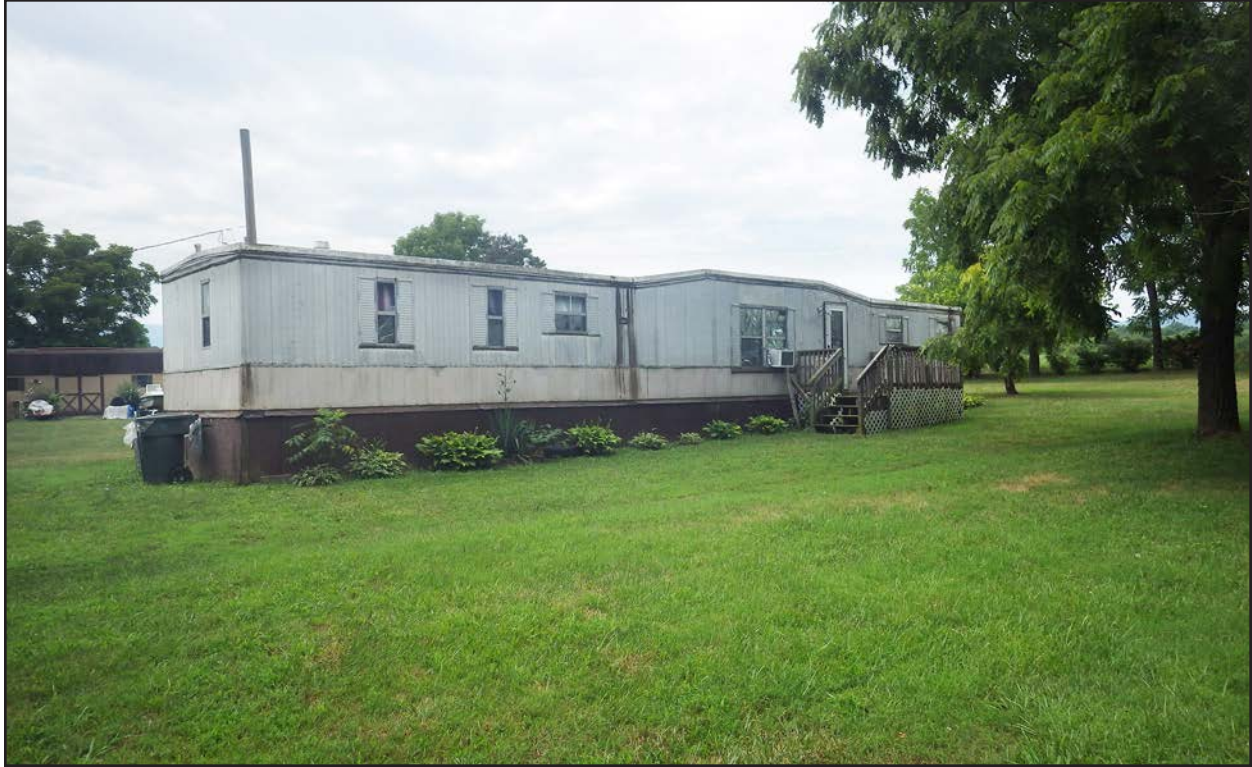
Figure 119. 007-5698, modular home, facing southwest.
