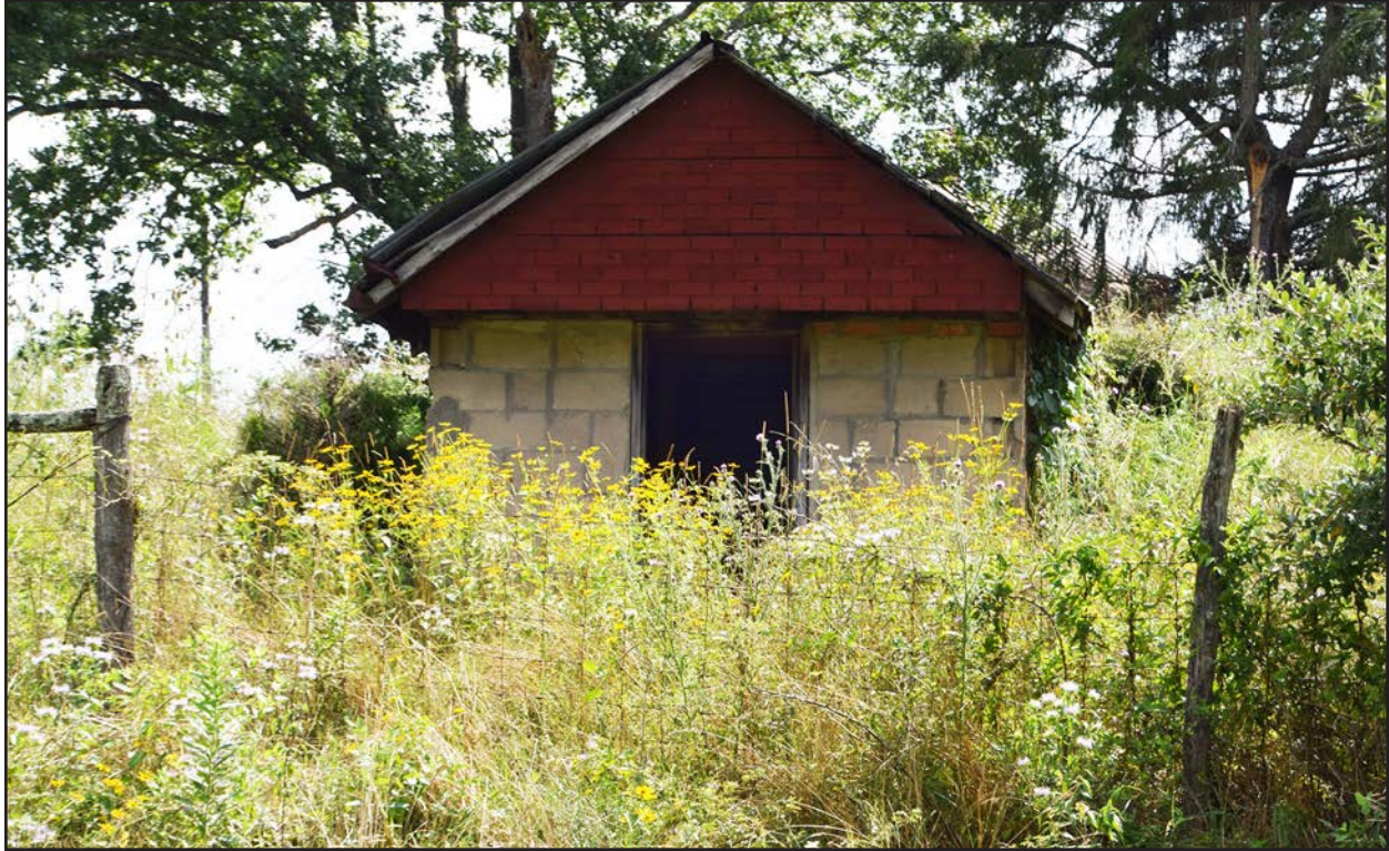
Figure 39. 007-0480, root cellar, facing east.
