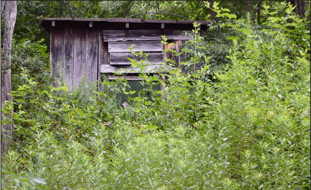
Figure 28. 007-0457, shed 1, facing east. 28
