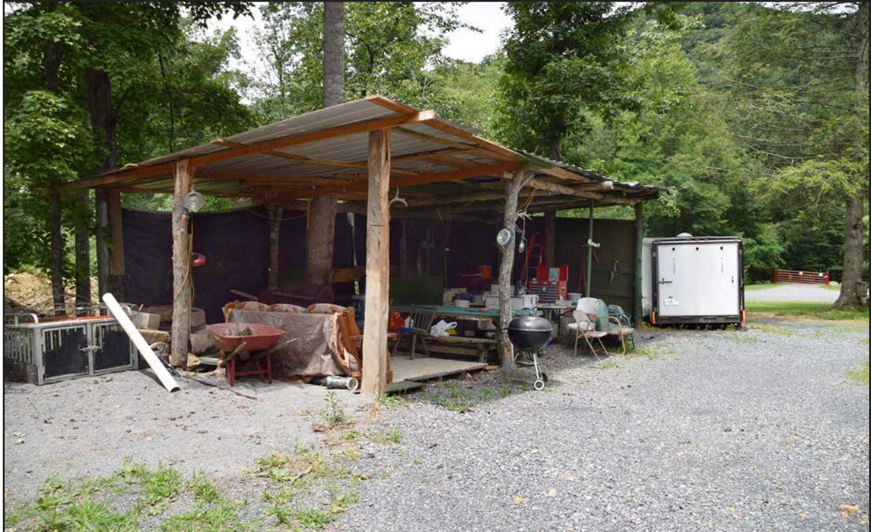
Figure 142. 008-5058, three bay shed carried by dressed tree posts, facing north.
