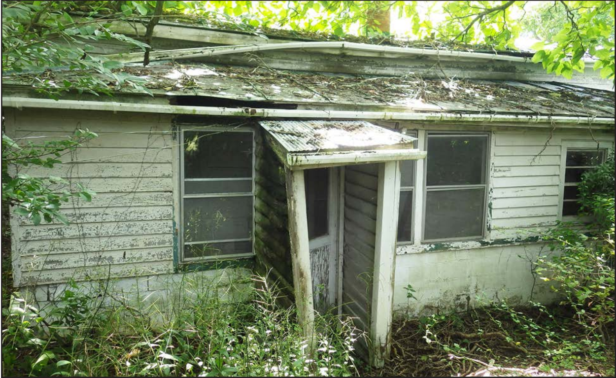
Figure 97. 007-5692, rear shed addition, facing south.
