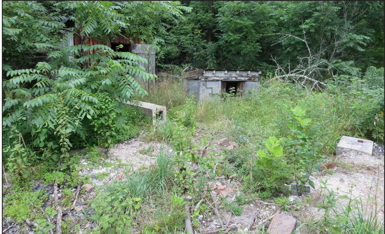
Figure 194. 045-5079, ruins showing concrete masonry unit chimney, facing east.
