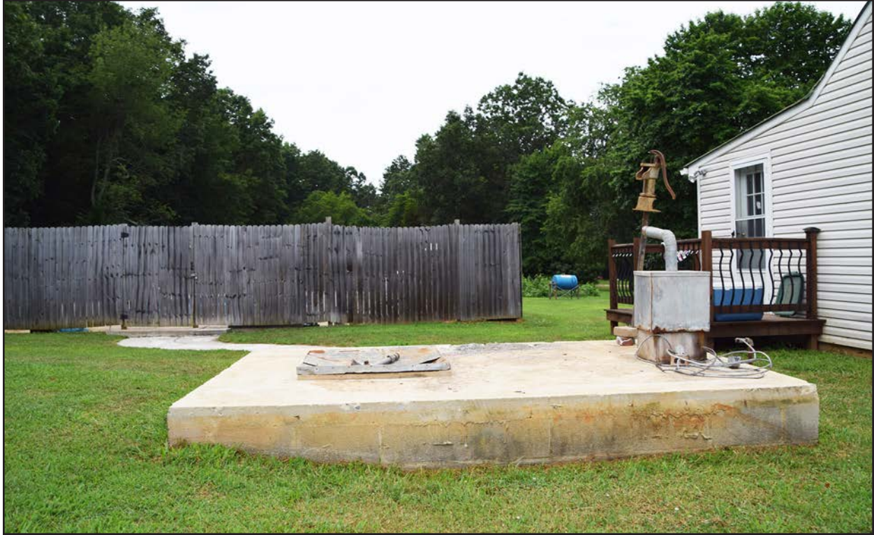
Figure 43. 007-5569, well pad, view east.
