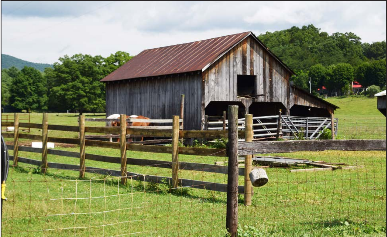
Figure 92. 007-5691, barn 1, facing northeast.
