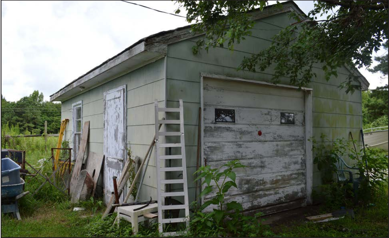
Figure 255. 133-5444, garage, facing southeast.
