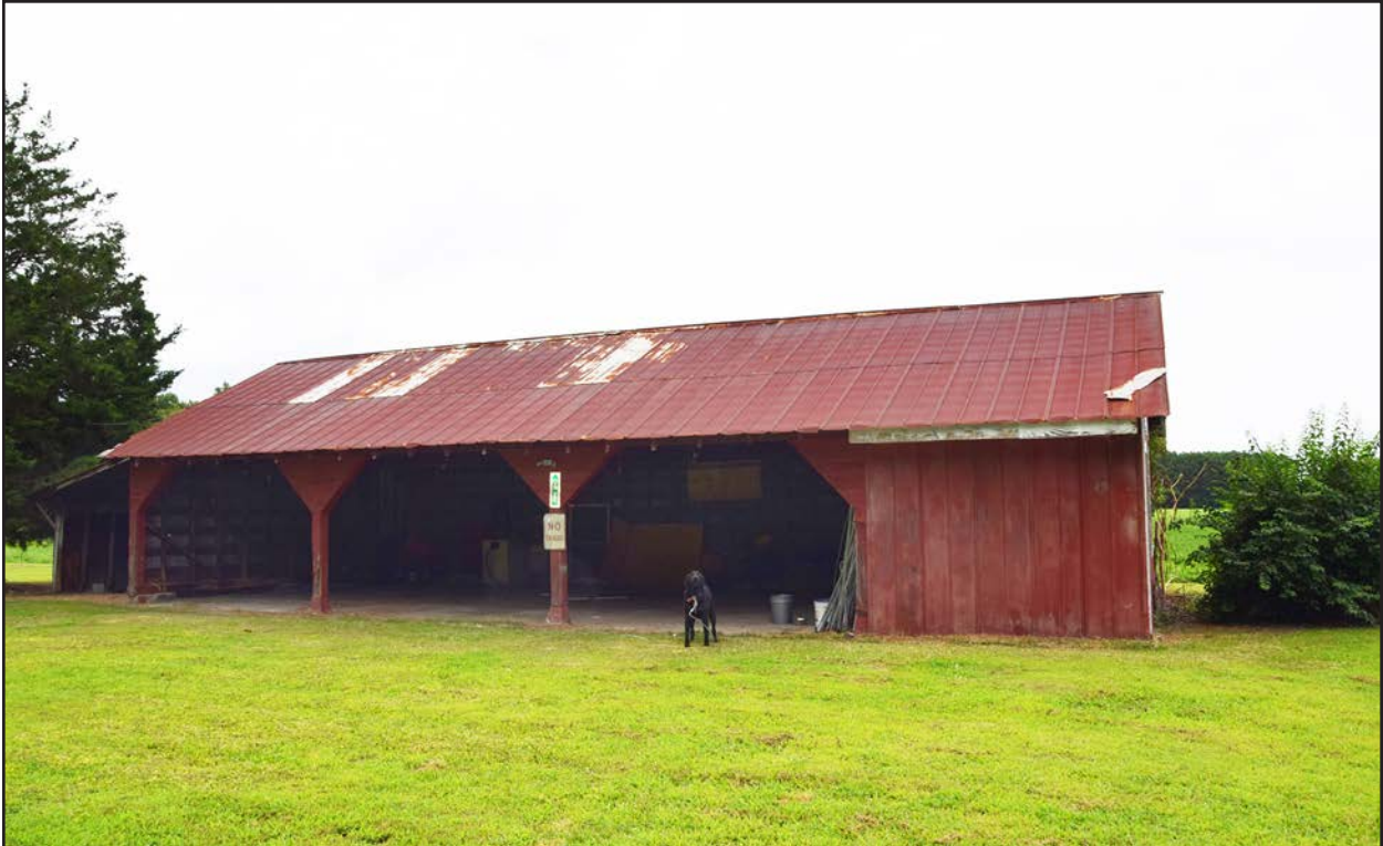
Figure 238. 133-0209 barn, facing north.
