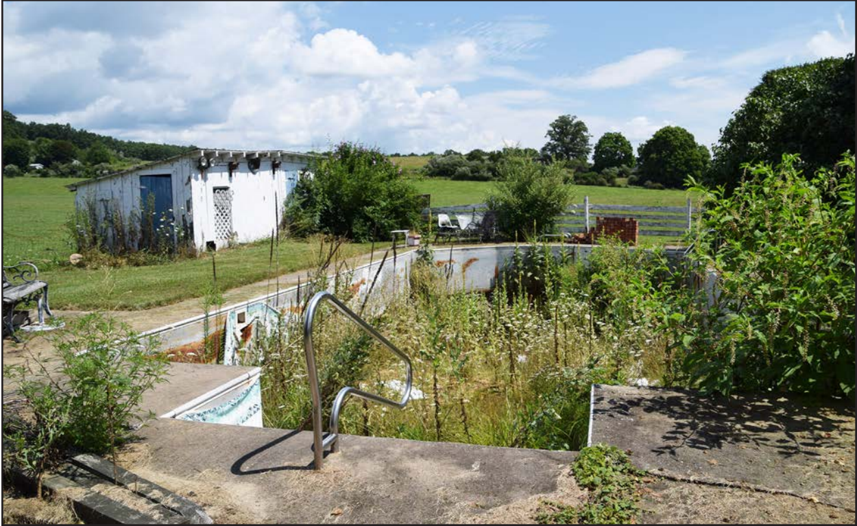
Figure 91. 007-5691, shed 5, facing northeast.
