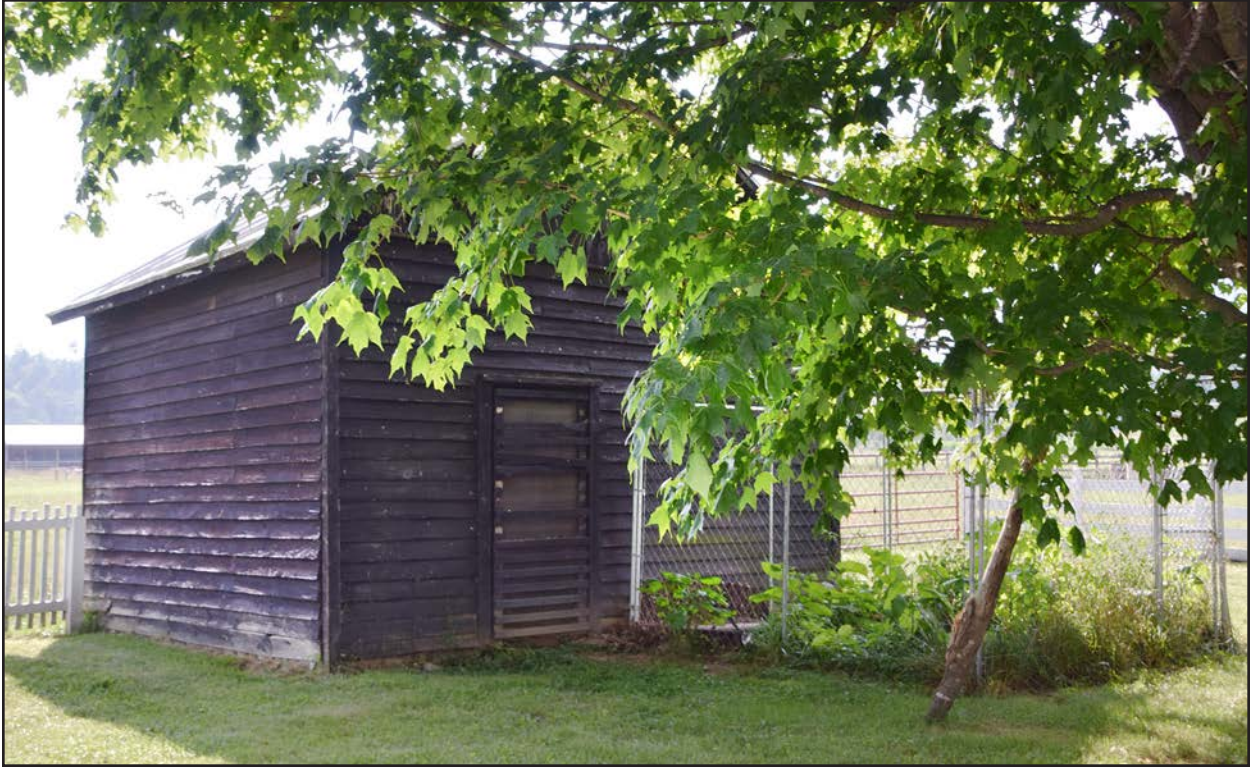
Figure 7. 007-0103, shed, facing northwest.
