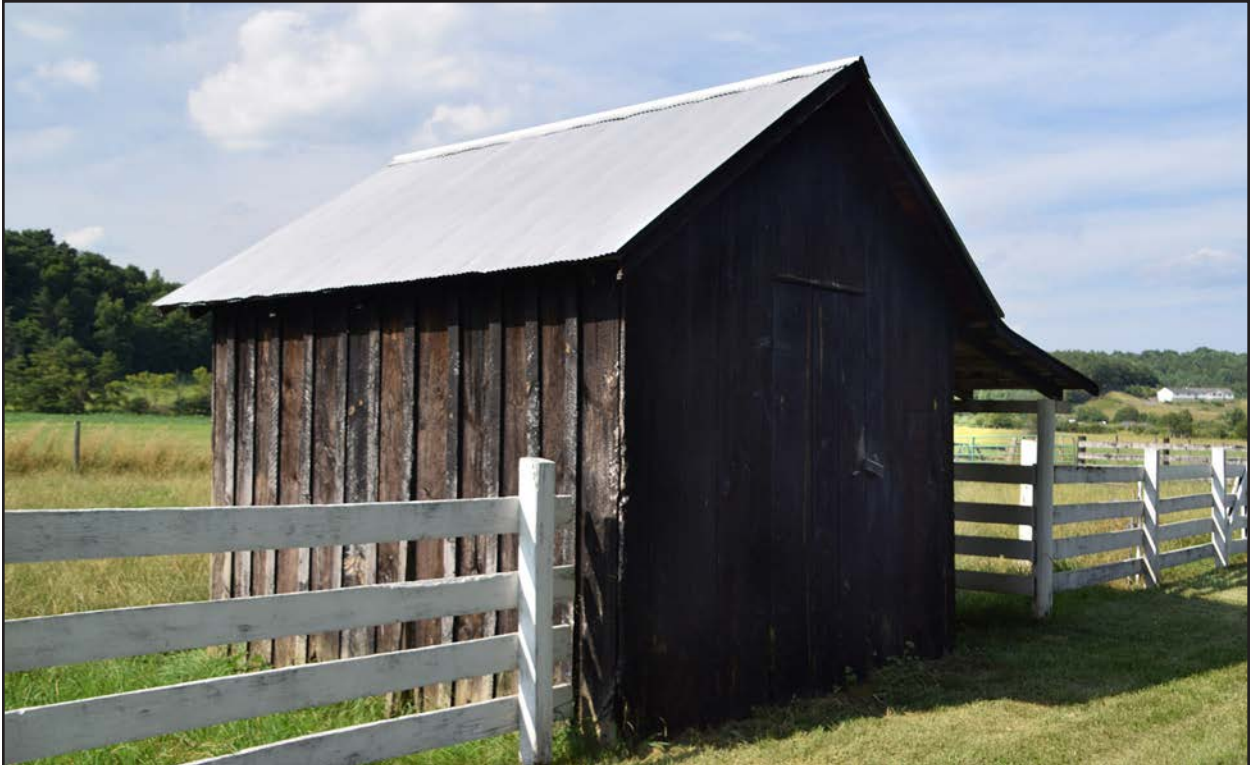
Figure 8. 007-0103, shed, facing northeast.
