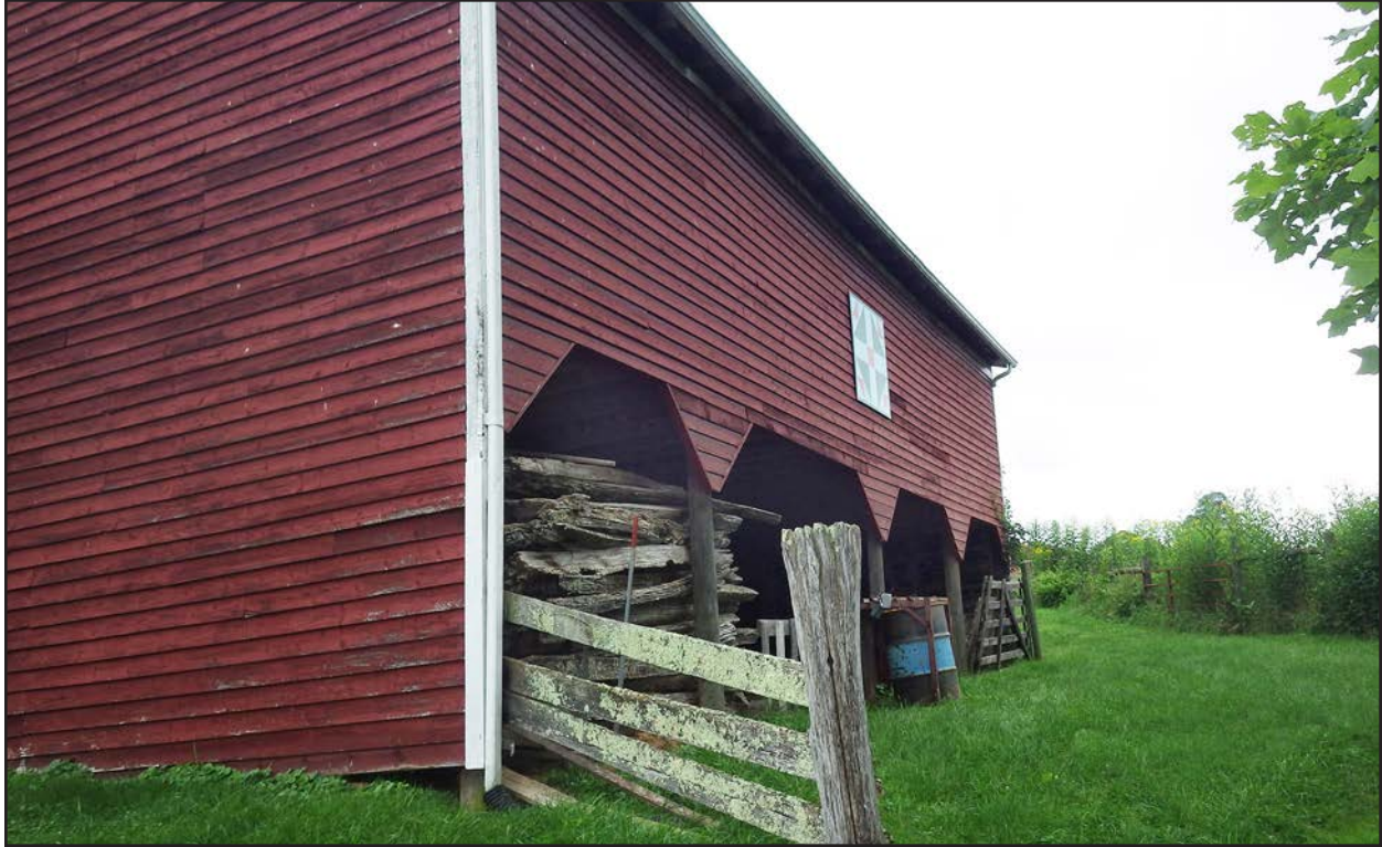
Figure 175. 045-0055, barn 1, facing north-northwest.
