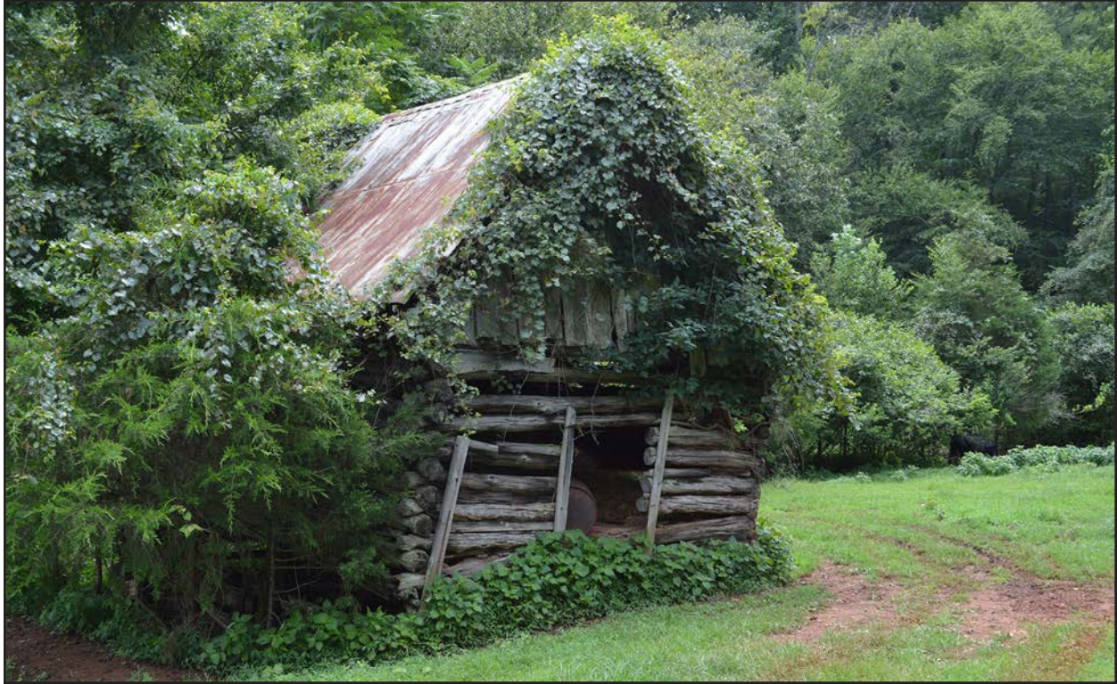
Figure 229. 062-5221, log barn 1, facing south.
