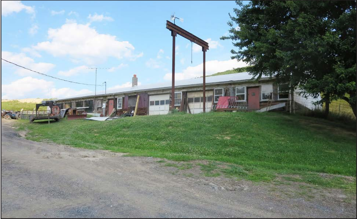
Figure 159. 008-5063, turkey house, facing east.
