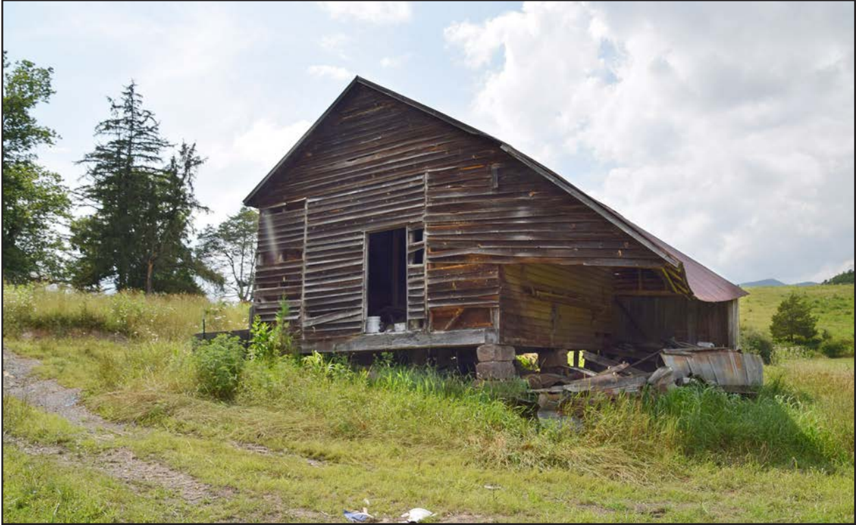
Figure 37. 007-0480, shed 2, facing northwest.
