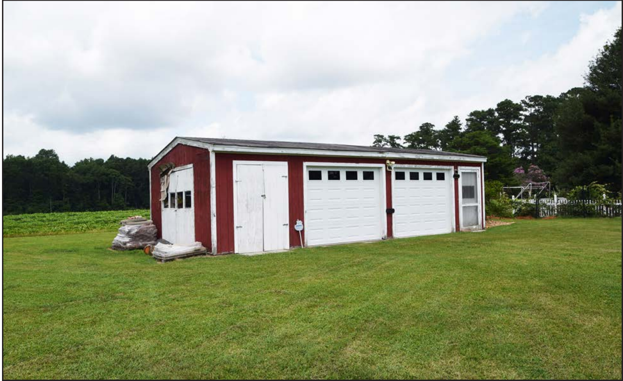
Figure 293. 133-5575, shed, facing northeast.
