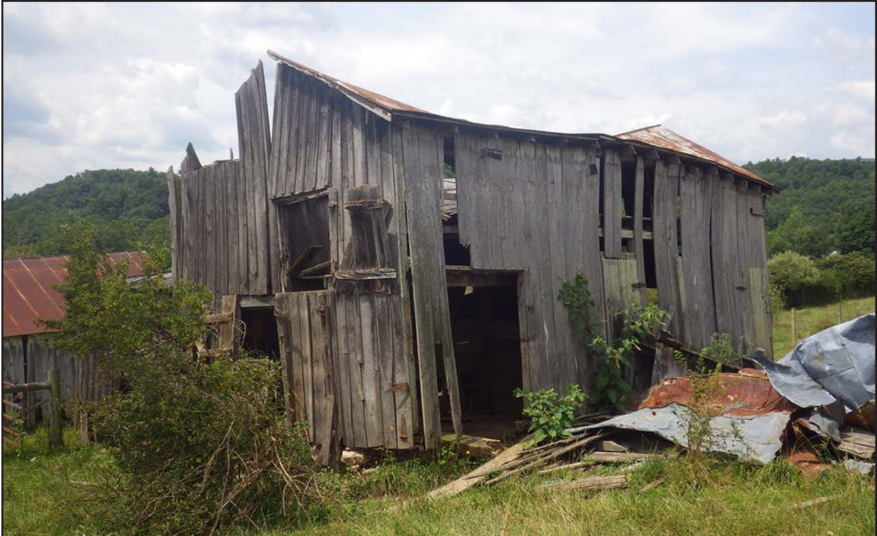
Figure 98. 007-5692, barns, facing south.
