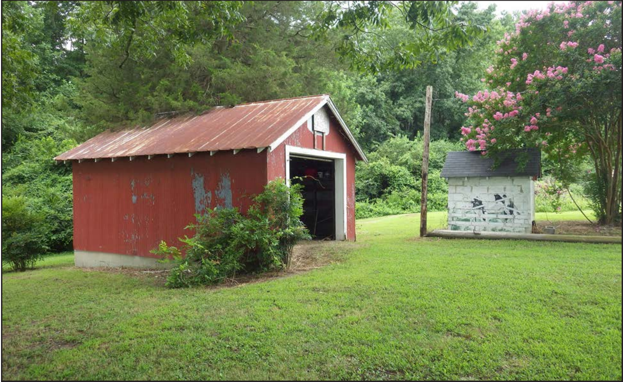
Figure 237. 133-0209, garage and pump house, facing west.
