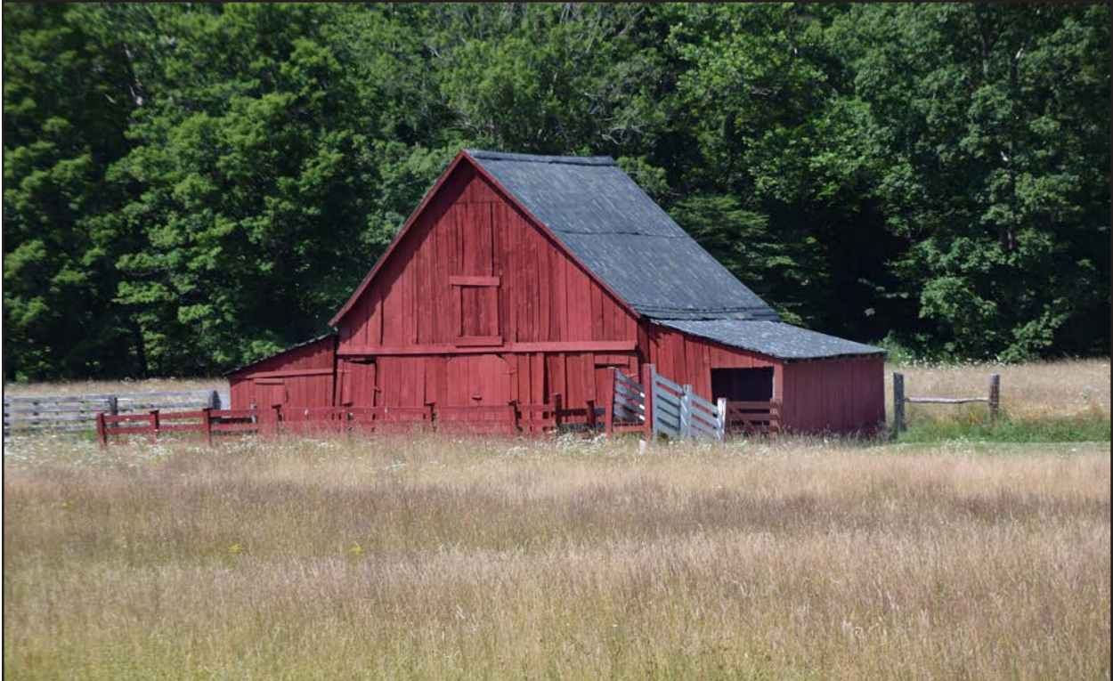
Figure 206. 045-5081, barn, facing northeast.
