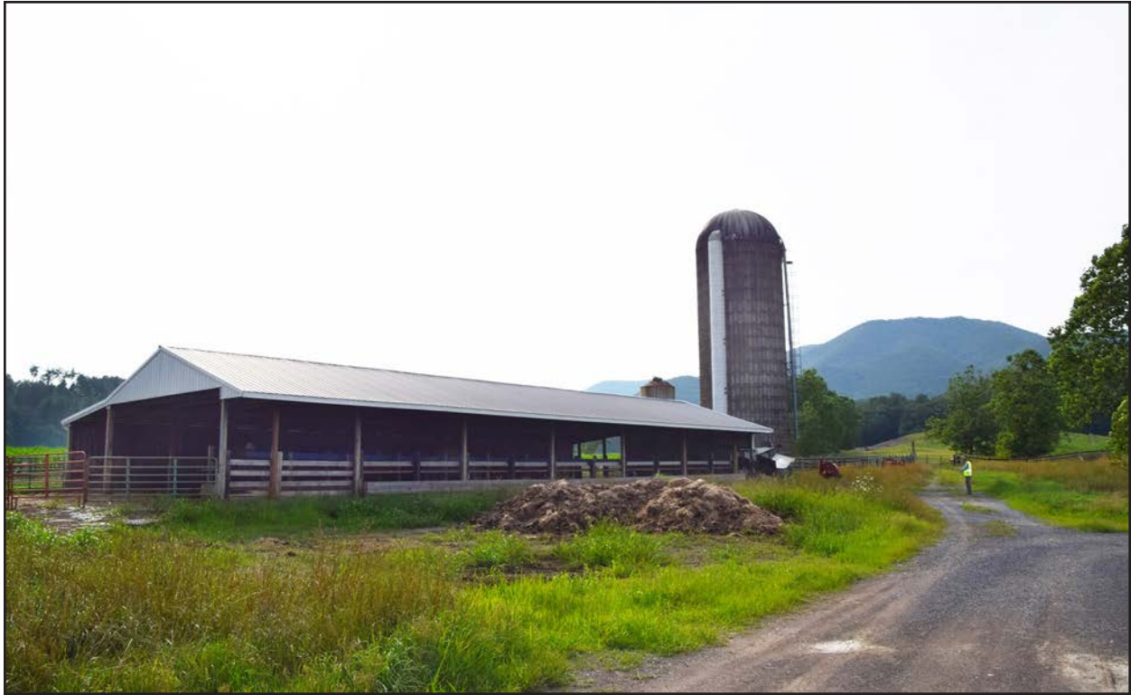
Figure 15. 007-0103, barn, facing north-northwest.
