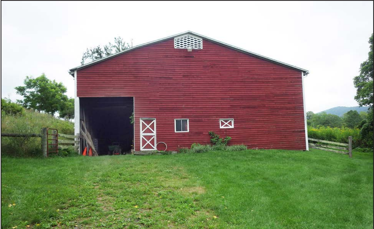
Figure 174. 045-0055, barn 1, facing northeast.
