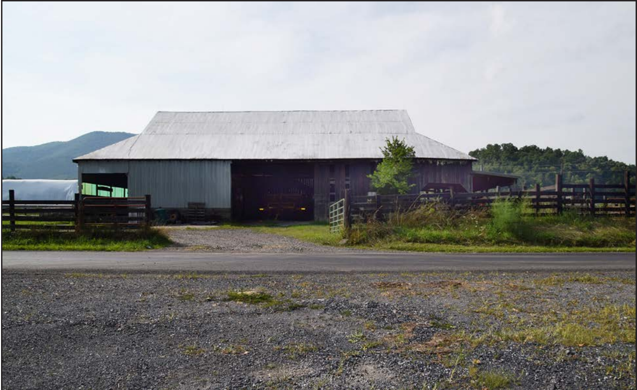
Figure 12. 007-0103, barn, facing north.
