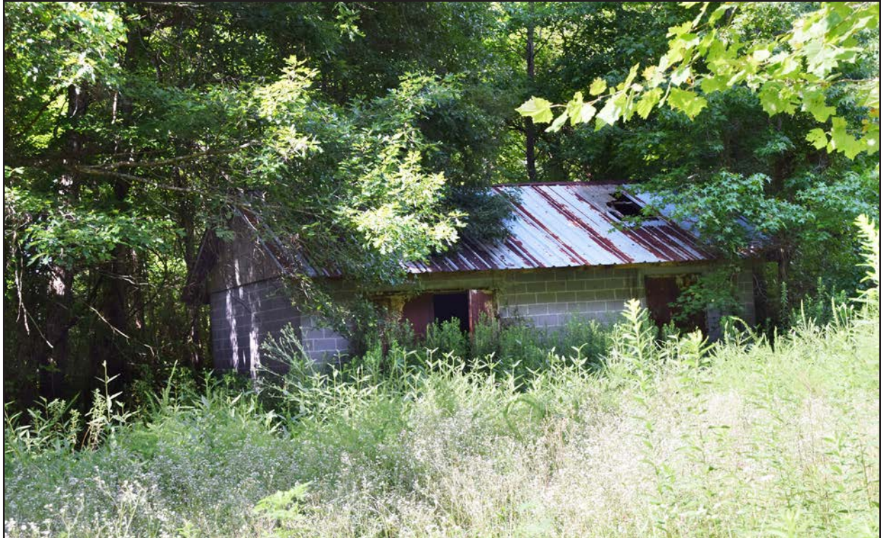
Figure 278. 133-5572, storage structure, facing northeast.
