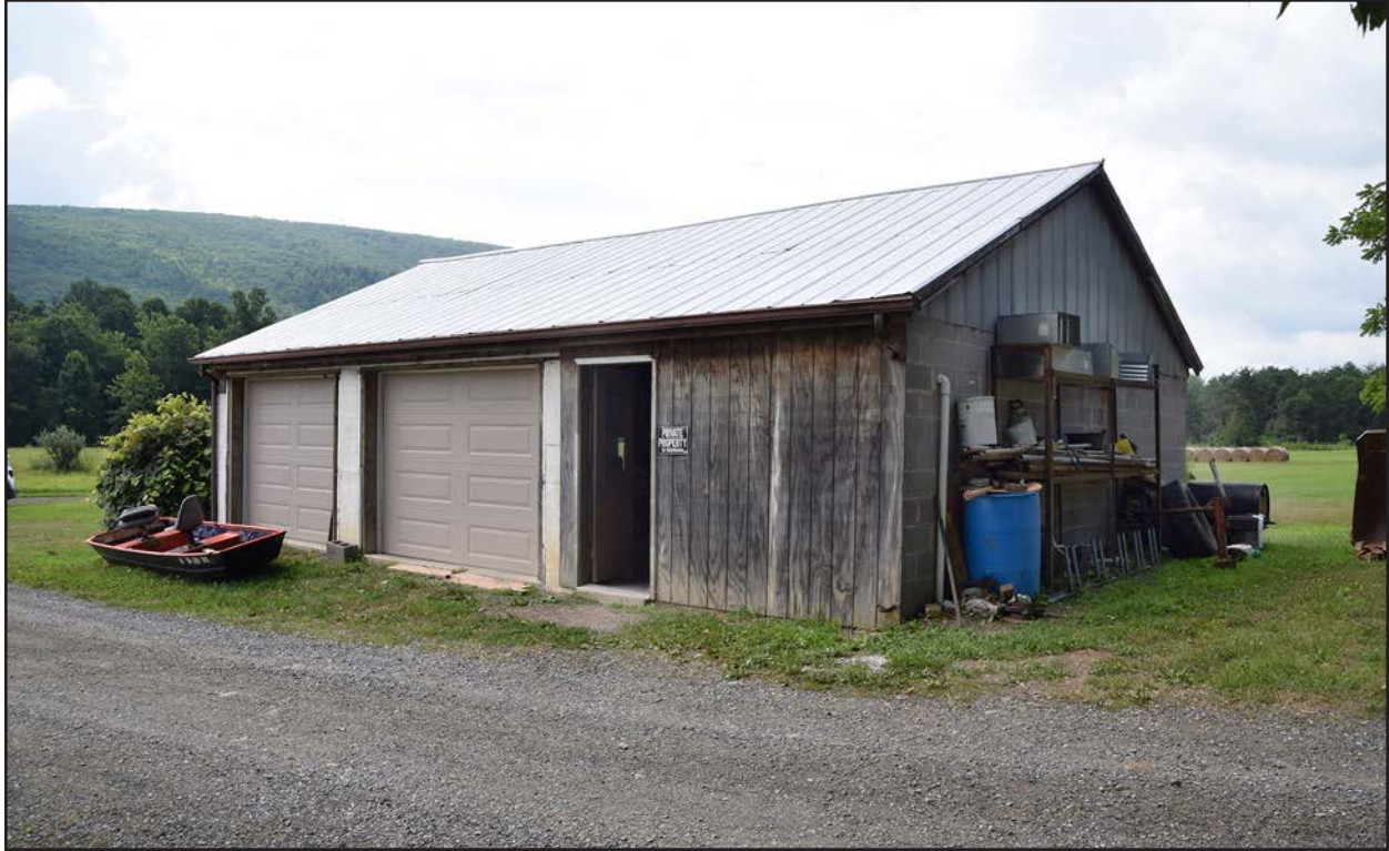
Figure 51. 007-5682, storage building, facing south.
