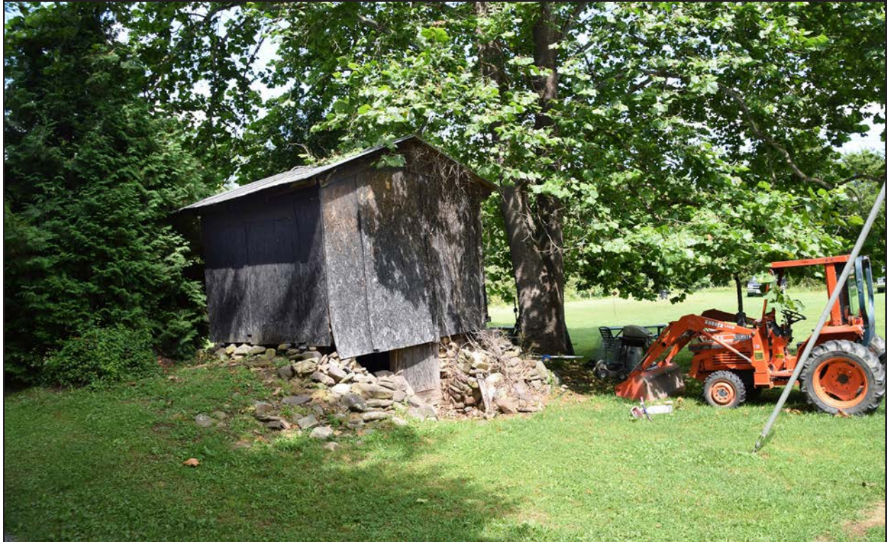
Figure 80. 007-5689 root cellar, facing north-northeast.
