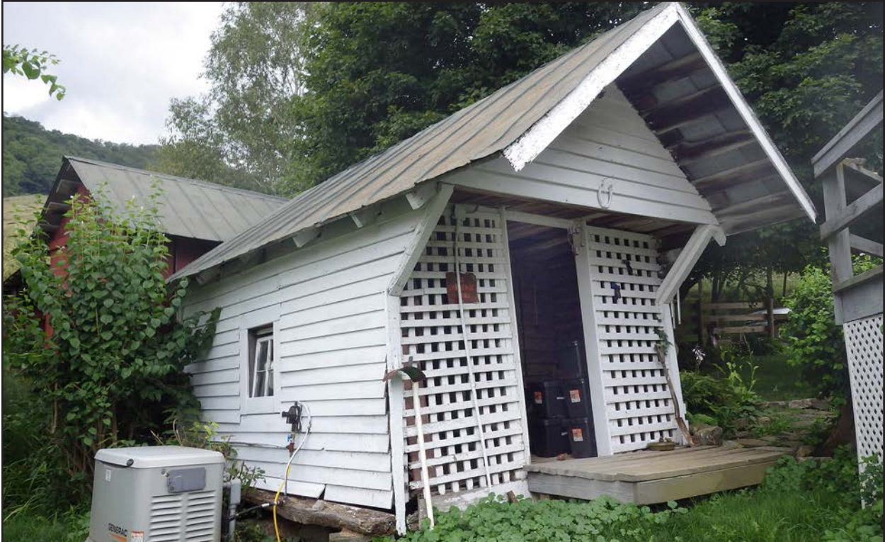
Figure 180. 045-0055, shed 1, facing north.
