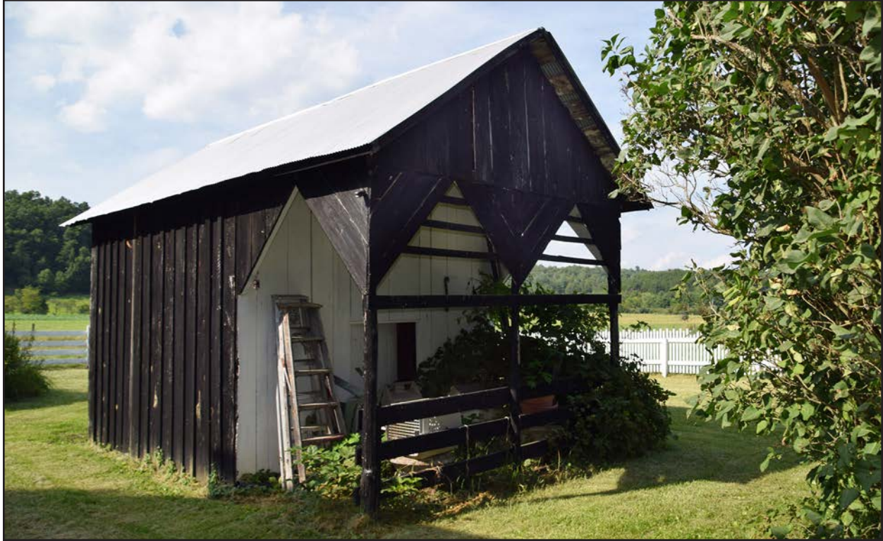
Figure 9. 007-0103, shed, facing northeast.
