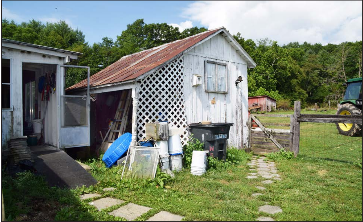
Figure 87. 007-5691, shed 1, facing northwest.
