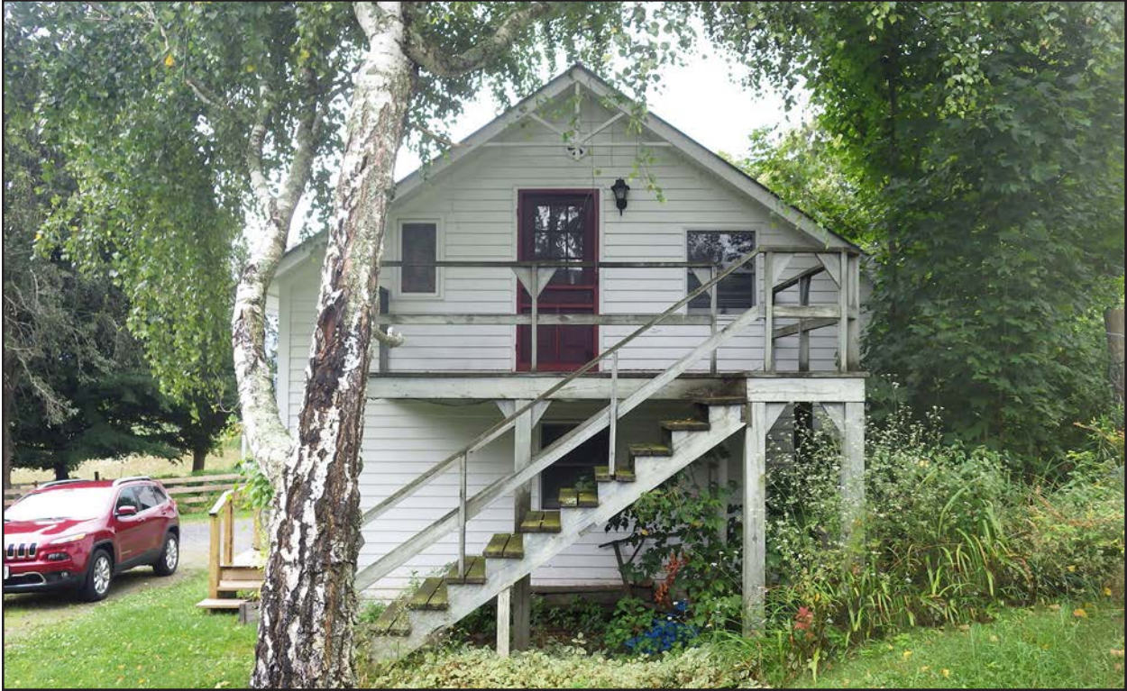
Figure 179. 045-0055, garage, facing southwest.
