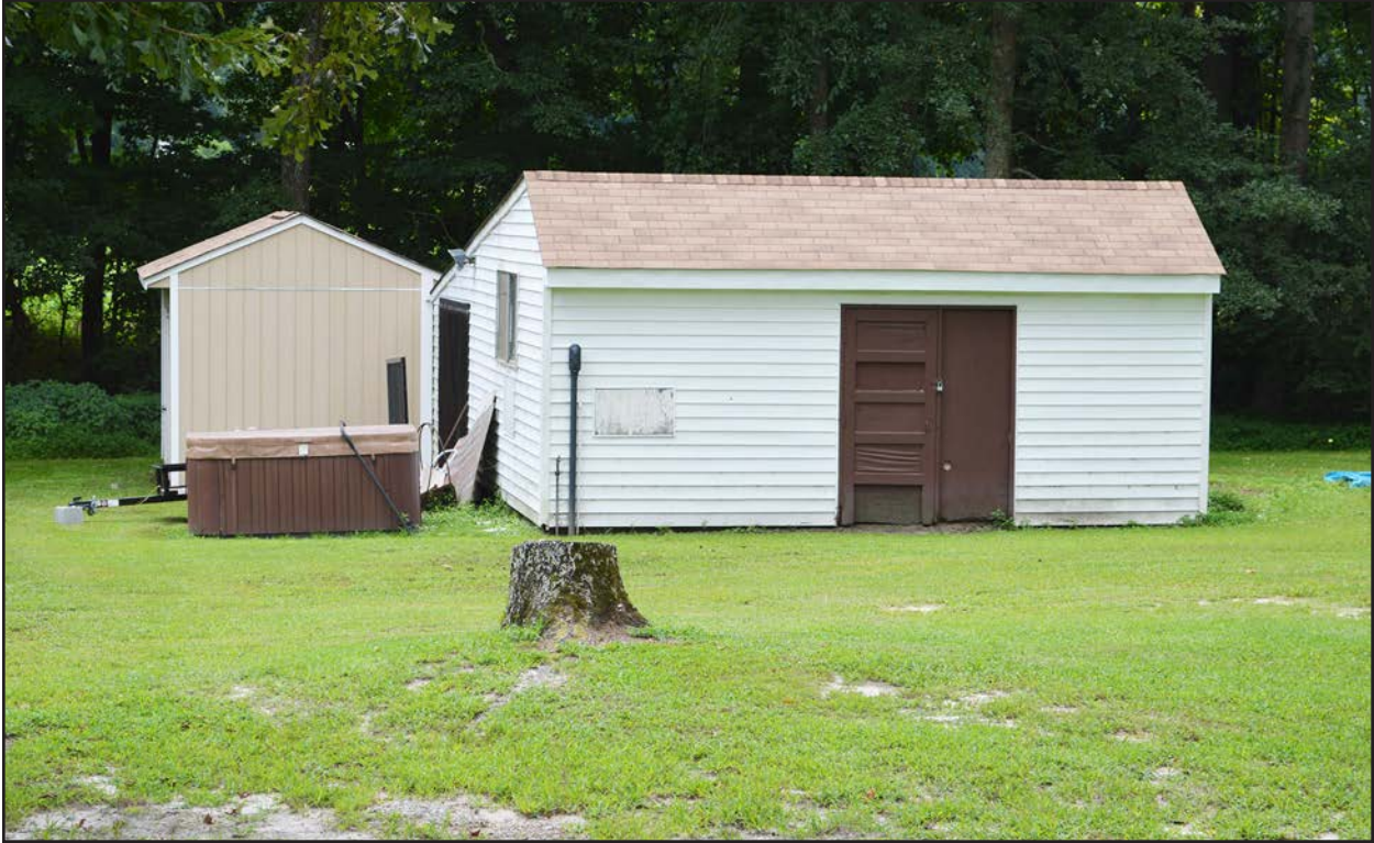
Figure 285. 133-5574, storage shed, facing south.
