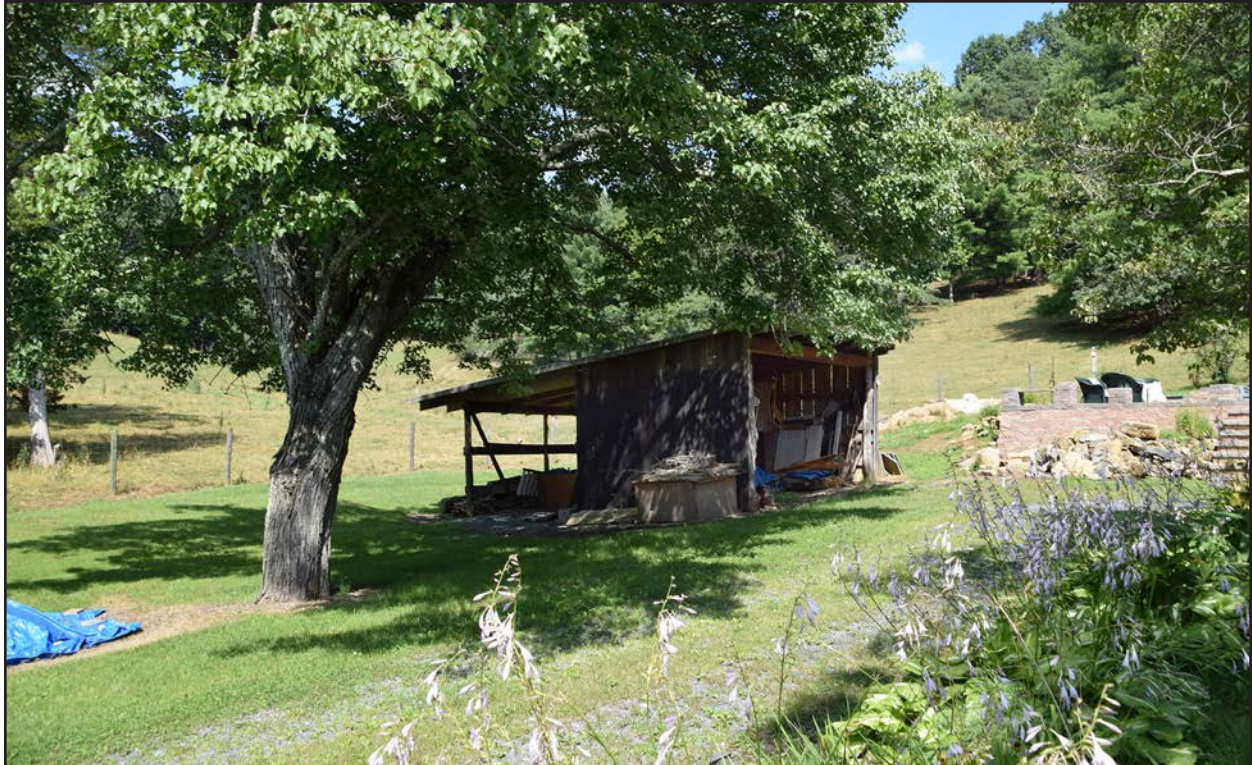
Figure 156. 008-5062, one bay shed, facing east.
