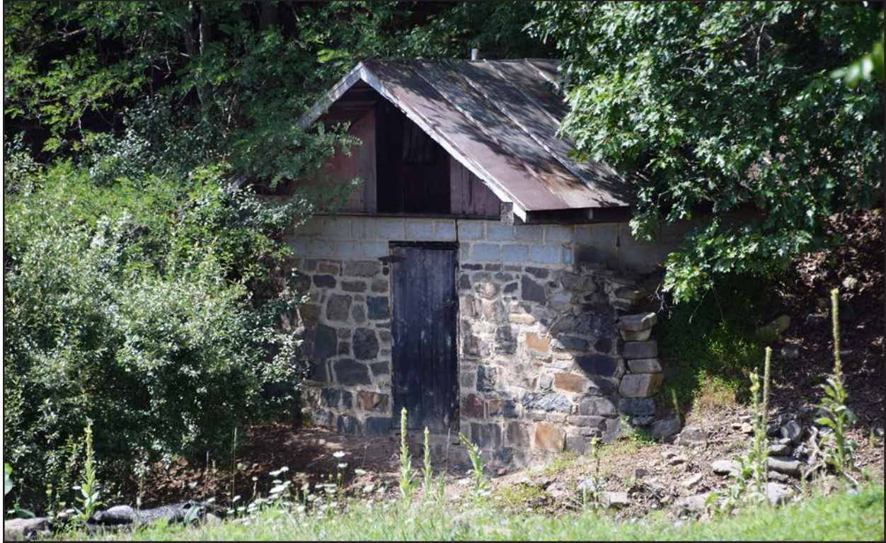
Figure 95. 007-5691, root cellar, facing southwest.
