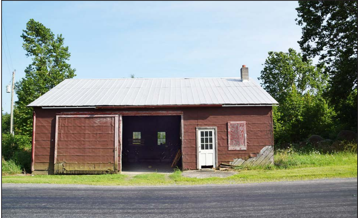
Figure 10. 007-0103, workshop, facing south.
