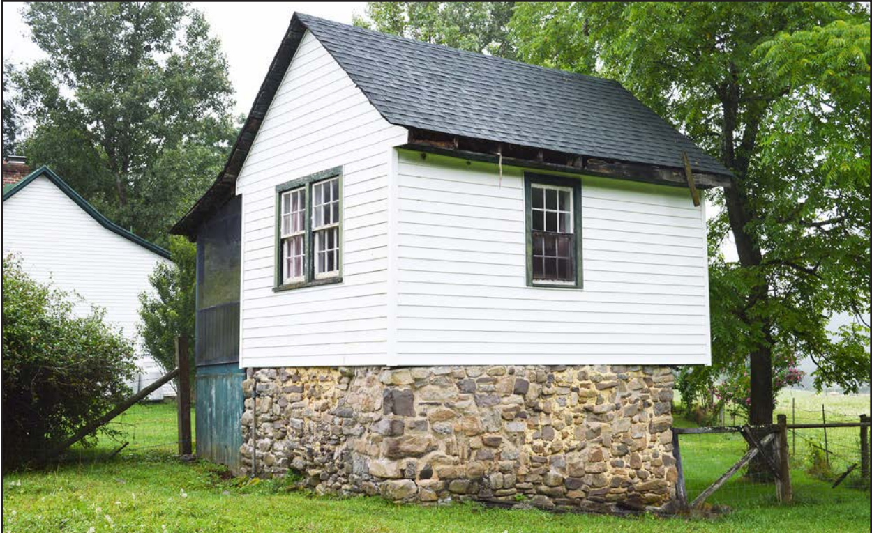
Figure 126. 007-5699 root cellar, facing east.
