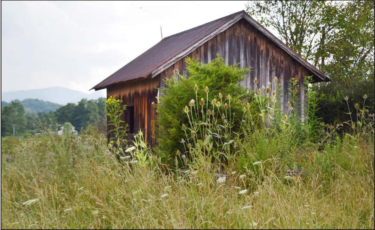
Figure 35. 007-0480, shed 1, facing east.
