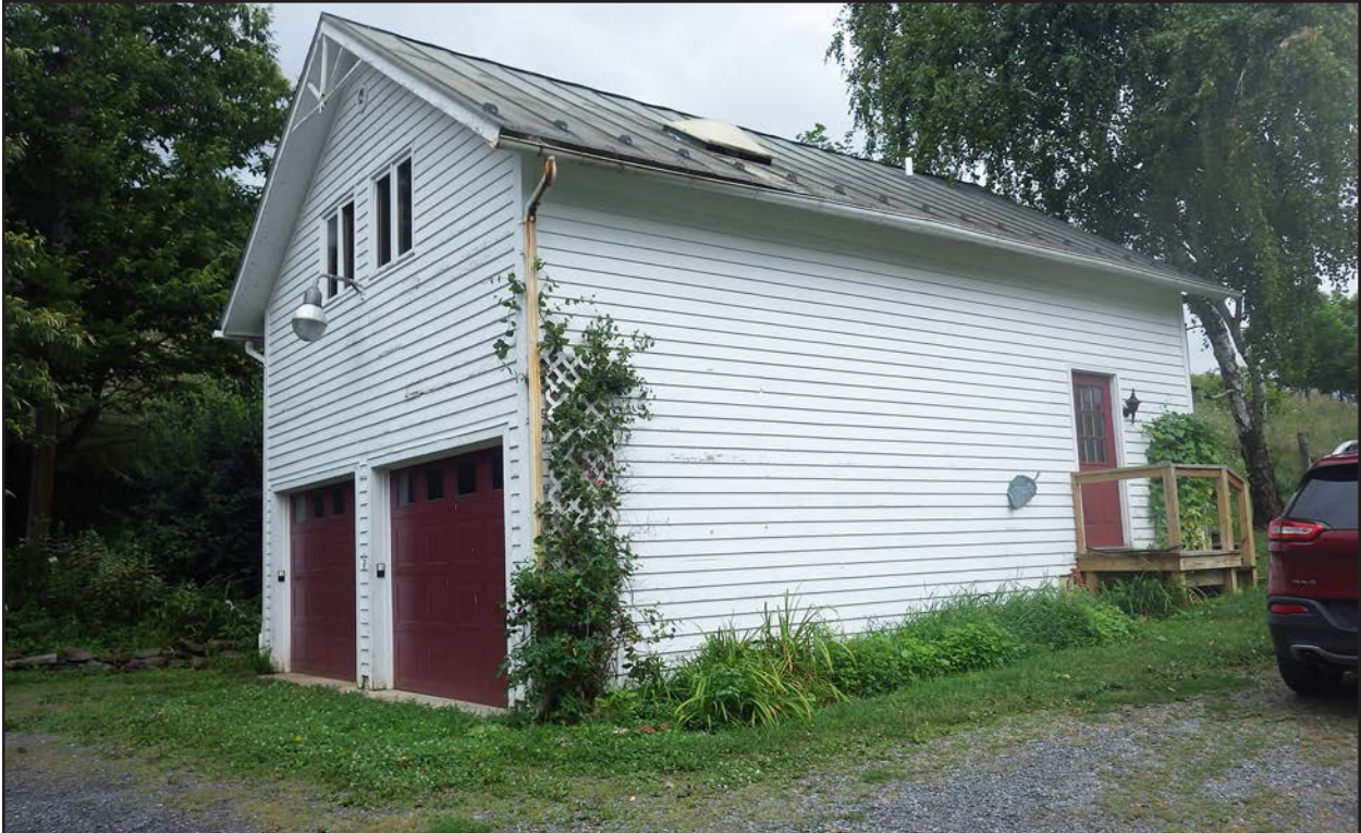
Figure 178. 045-0055, garage, facing north.
