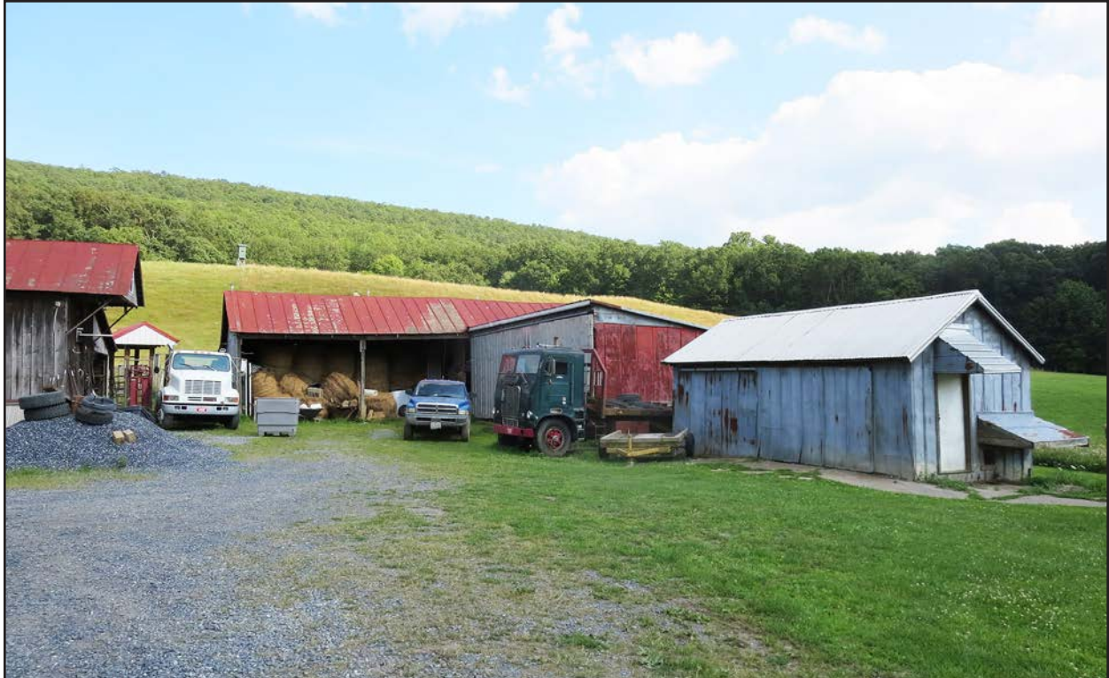
Figure 158. 008-5063, oldest outbuildings, facing southeast.
