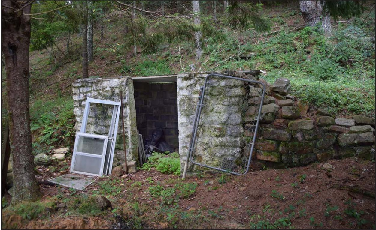
Figure 145. 008-5059, root cellar, facing south.
