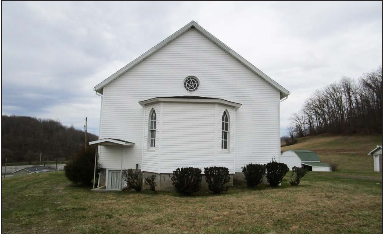
Photo 48. UP-0113, Gothic Revival Church, facing west.
