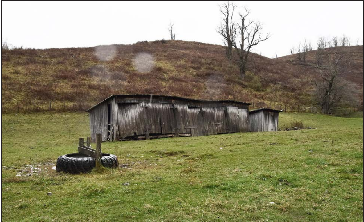
Photo 40. PH-0903, Shed 1 and 2, facing northwest.
