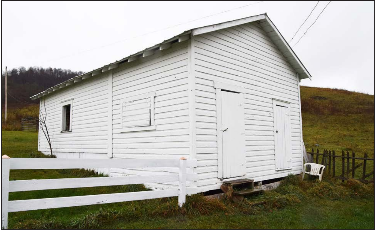
Photo 35. PH-0903, Outbuilding 1, facing north.
