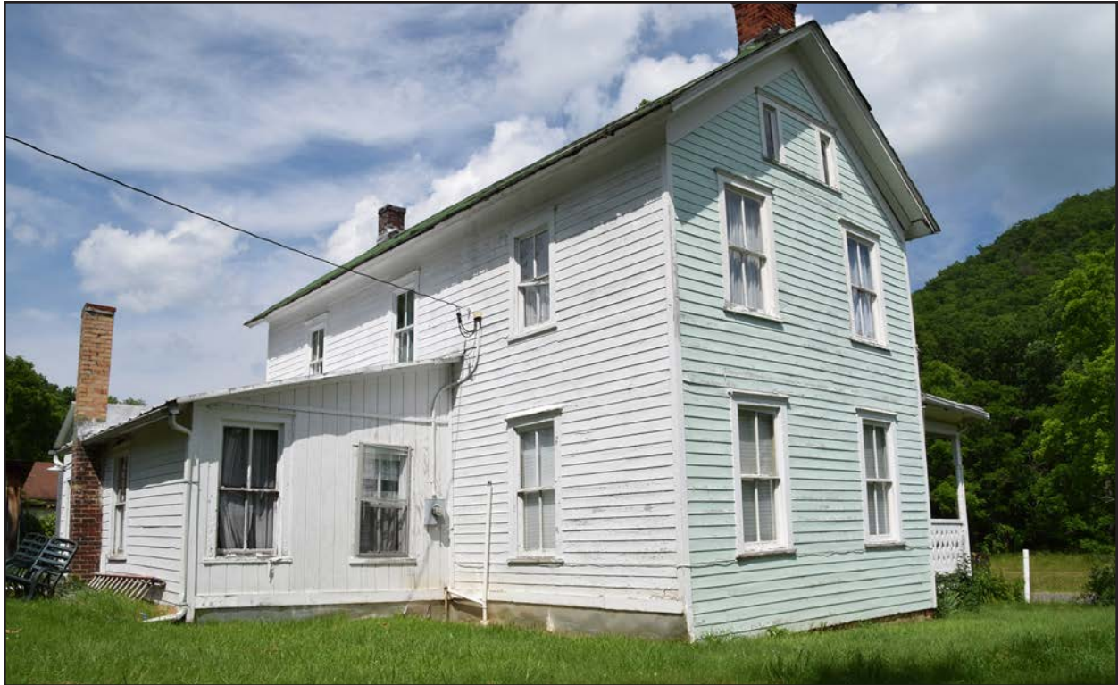
Photo 25. PH-0471, northwest and southwest elevations, facing east.
