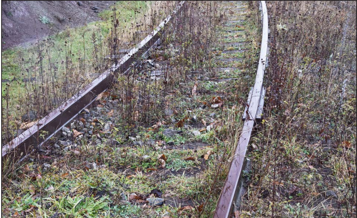
Photo 30. PH-0902, pulp and paper railroad, facing southeast.
