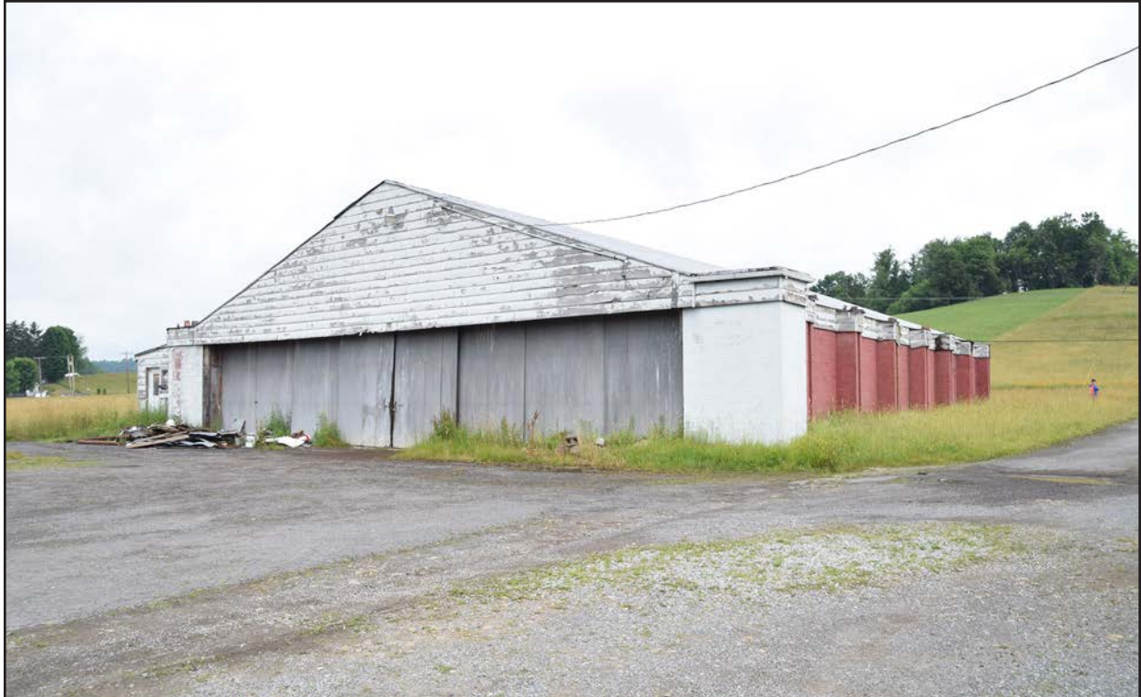
Photo 52. UP-0830, masonry hangar, facing north.
