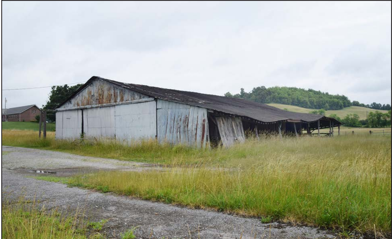
Photo 54. UP-0830, machine shop, facing northeast.
