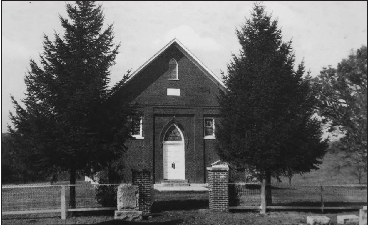
Photo 6. LE-0004, view of east façade of church in 1954, facing west.
