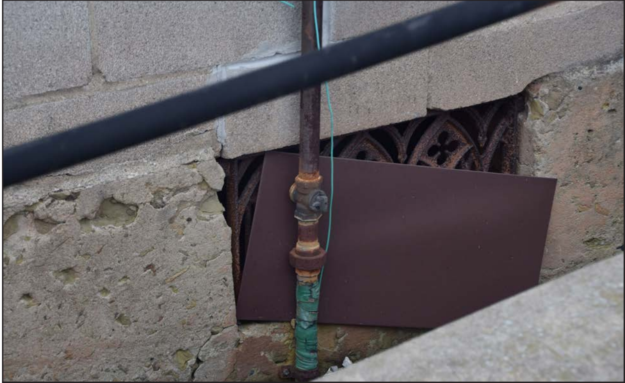
Photo 49. UP-0113, Gothic Revival Church, foundation detail, facing north.
