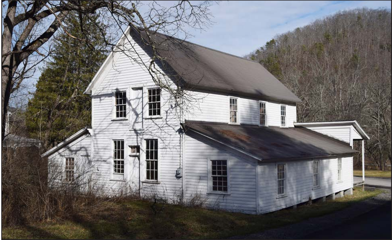
Photo 19. PH-0037-65, store, facing east.
