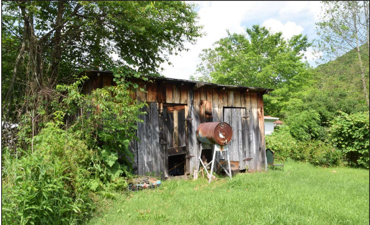
Photo 26. PH-0471, storage structure, facing east.
