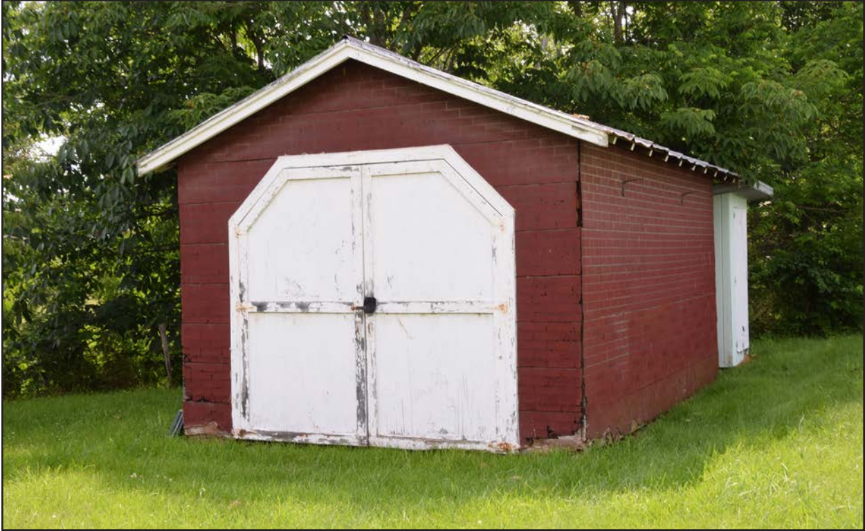
Photo 27. PH-0471, accessory structure, facing northwest.
