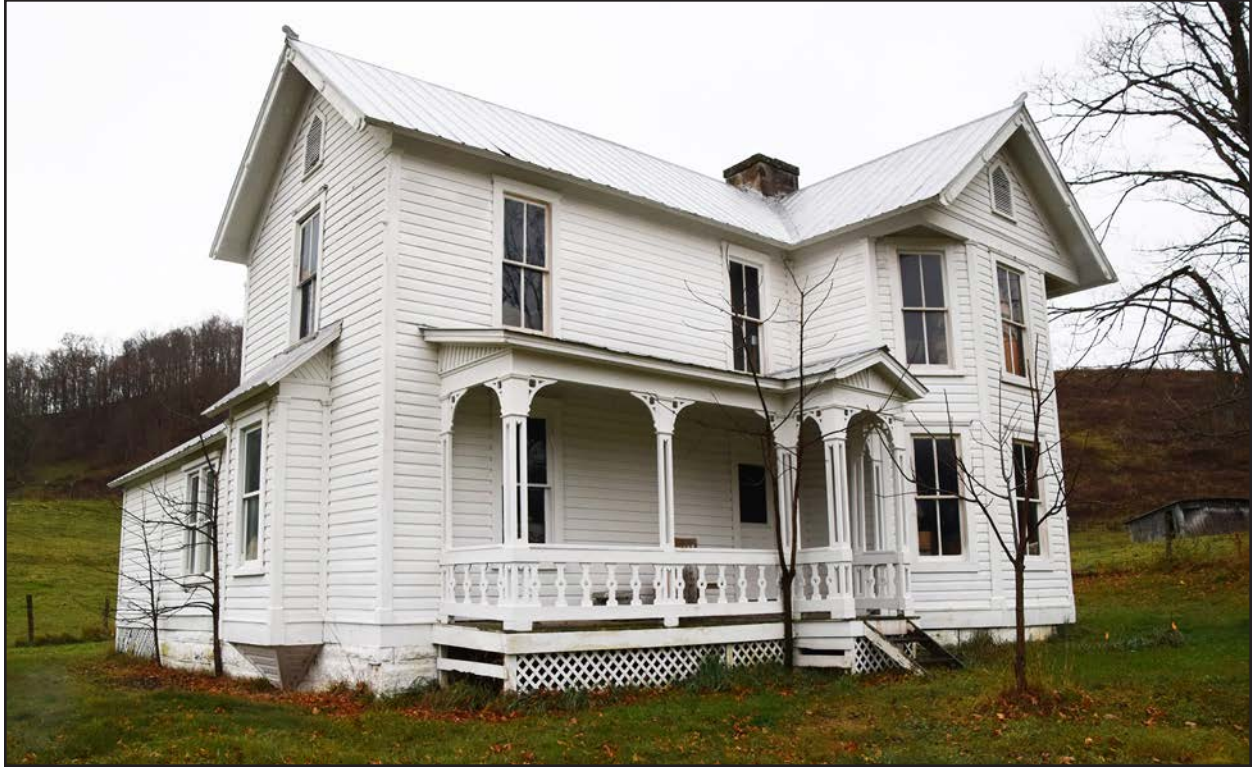
Photo 31. PH-0903, ca. 1890 house, facing west.
