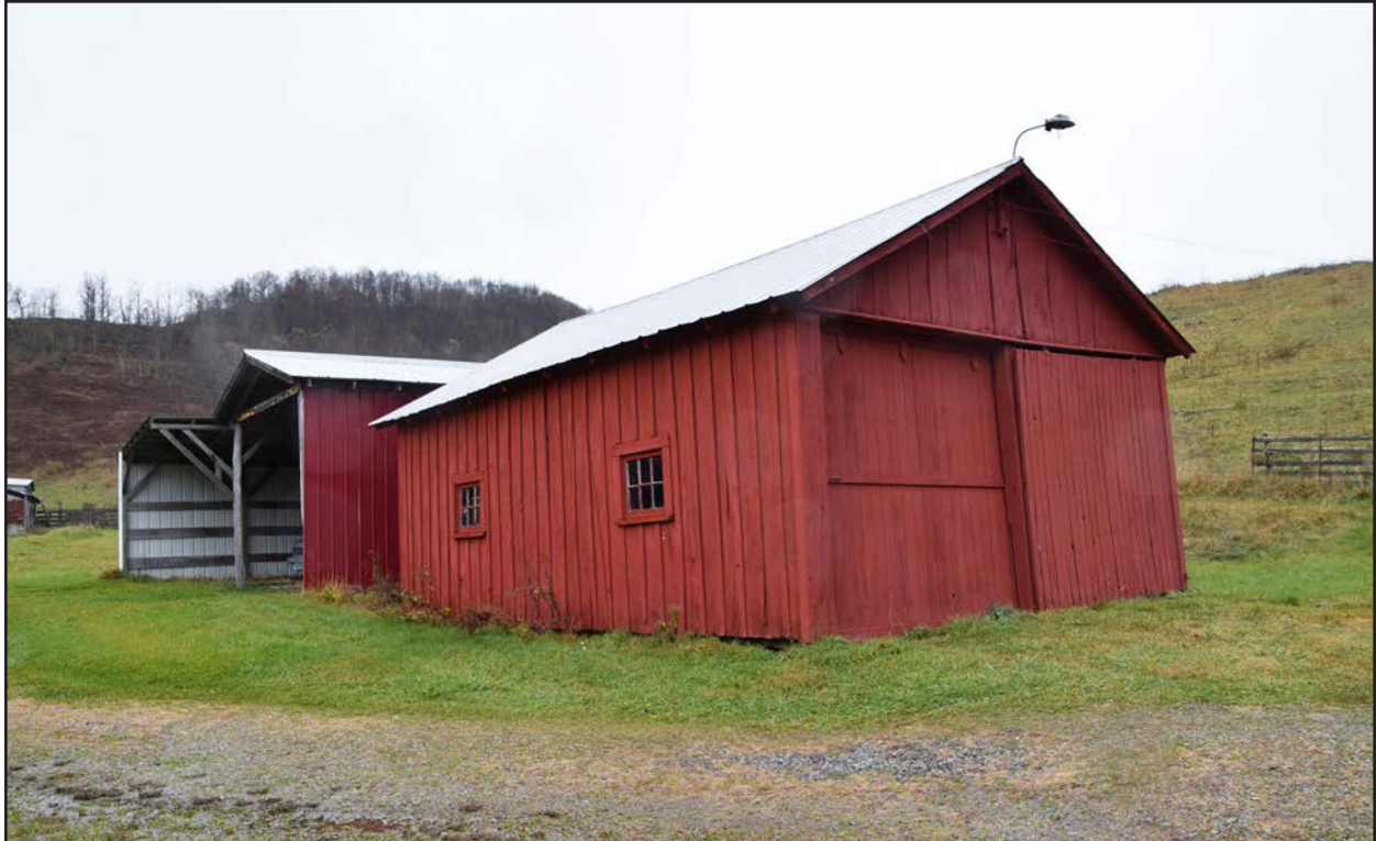
Photo 36. PH-0903, Barn 1 and Shed 5, facing northwest.
