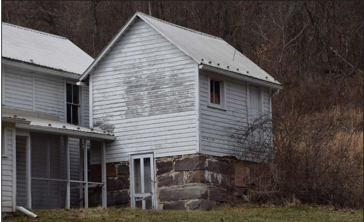
Photo 14. PH-0037-64 smokehouse/root cellar, facing northwest.
