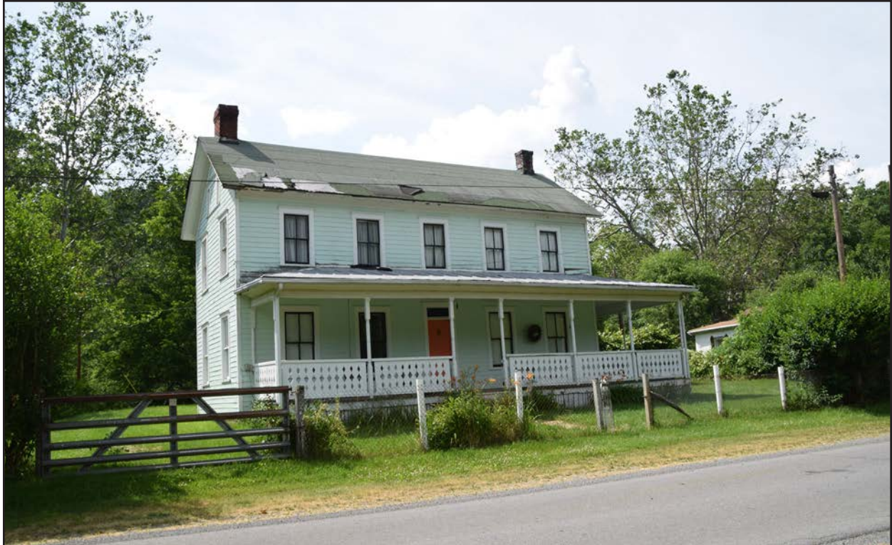
Photo 24. PH-0471, southwest elevation, facing north.
