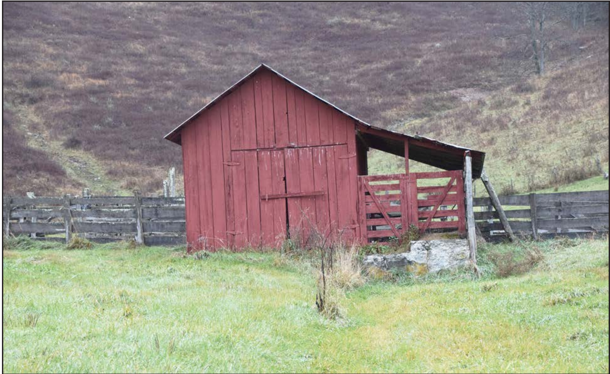
Photo 37. PH-0903, Barn 2, facing west.
