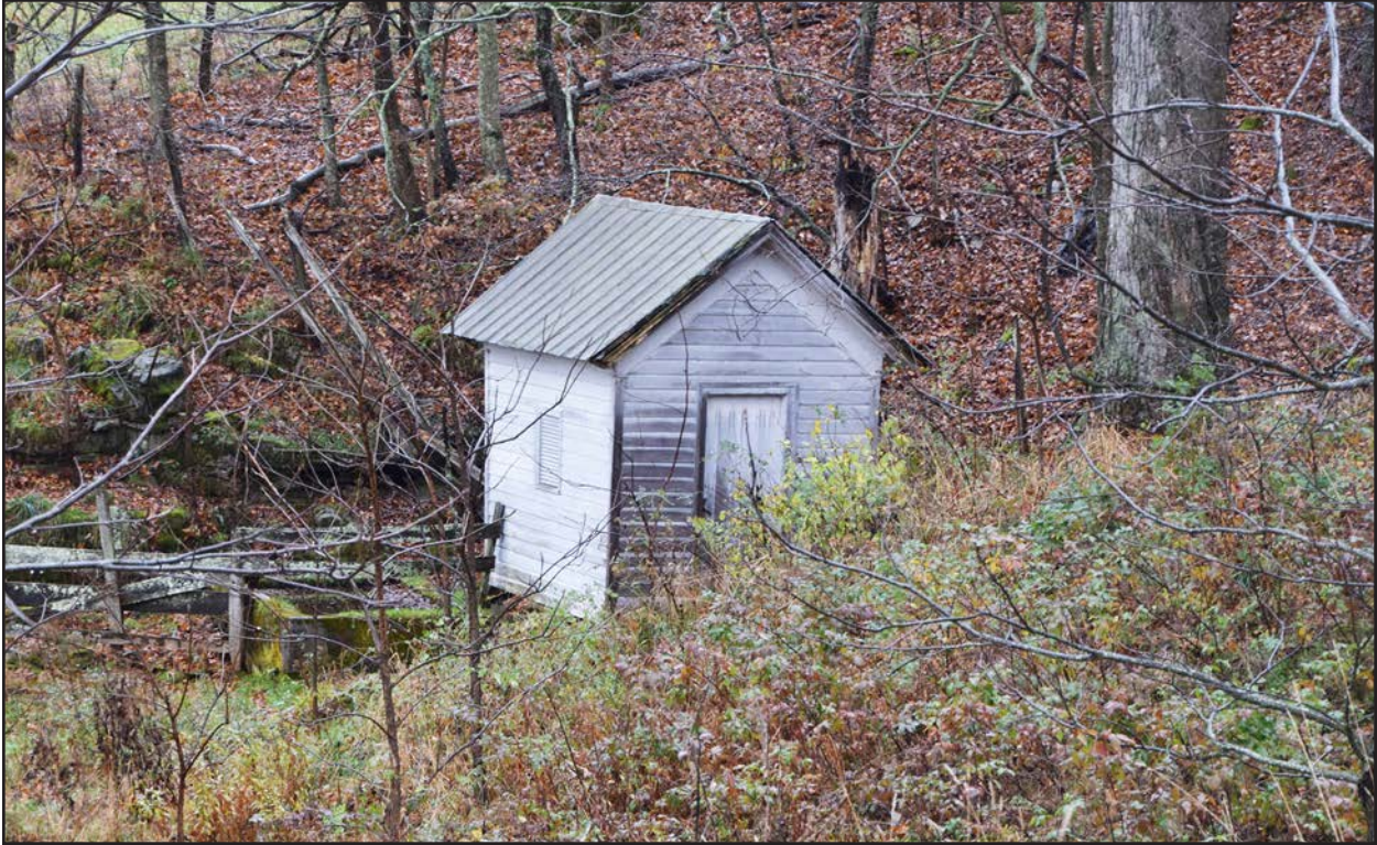
Photo 43. PH-0903, Well house, facing southeast.
