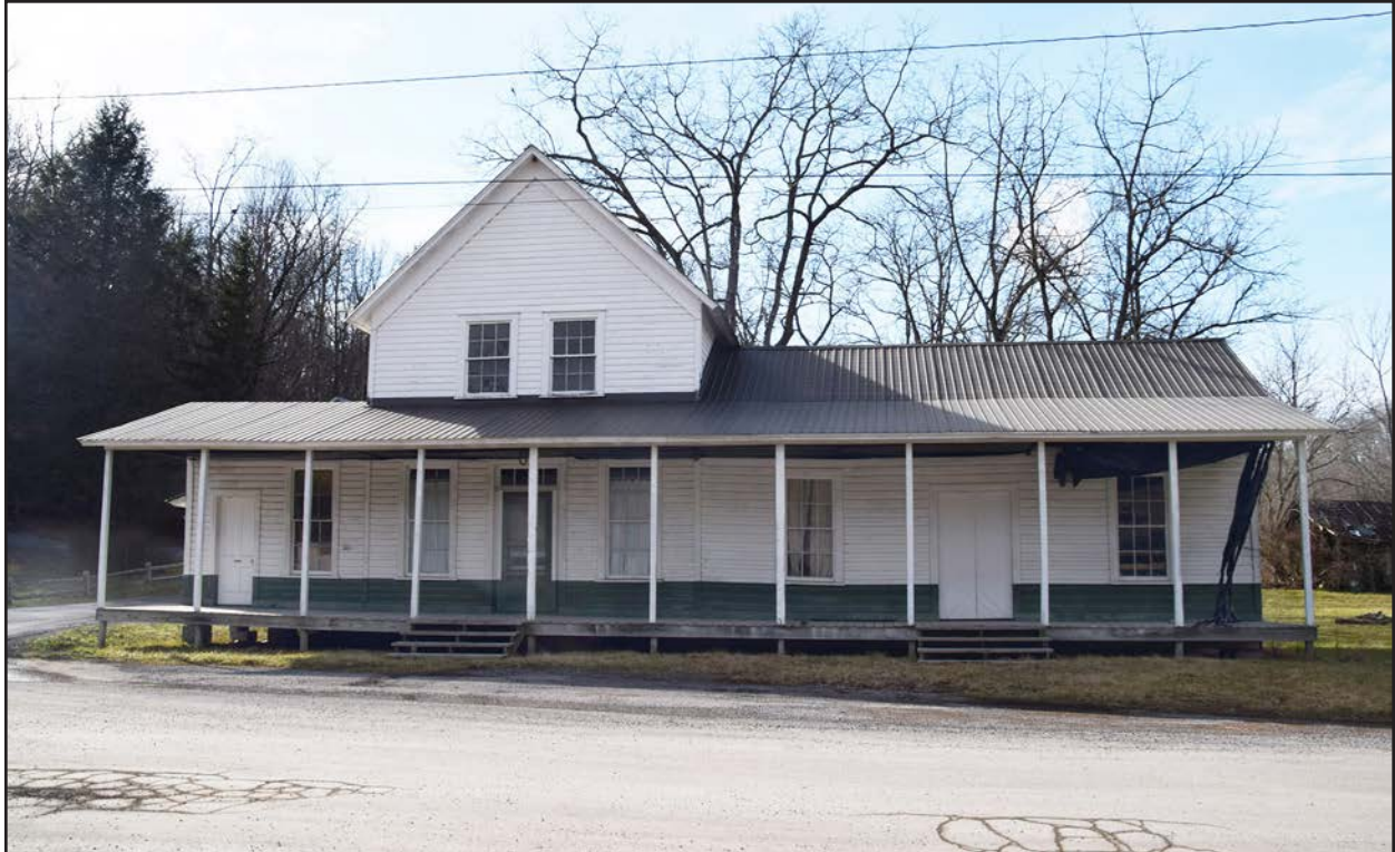
Photo 18. PH-0037-65, store, facing west.
