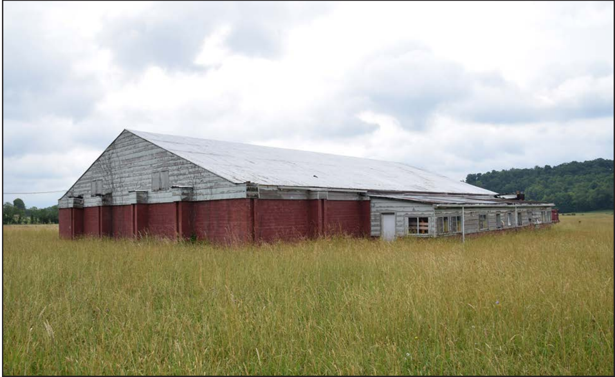
Photo 53. UP-0830, masonry hangar, facing southeast.
