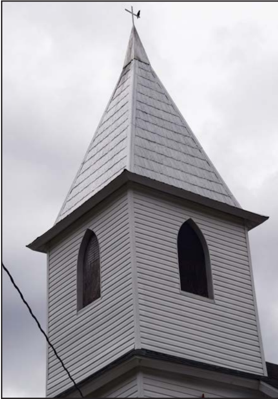
Photo 45. UP-0113, Gothic Revival Church, bell tower, facing northeast.
