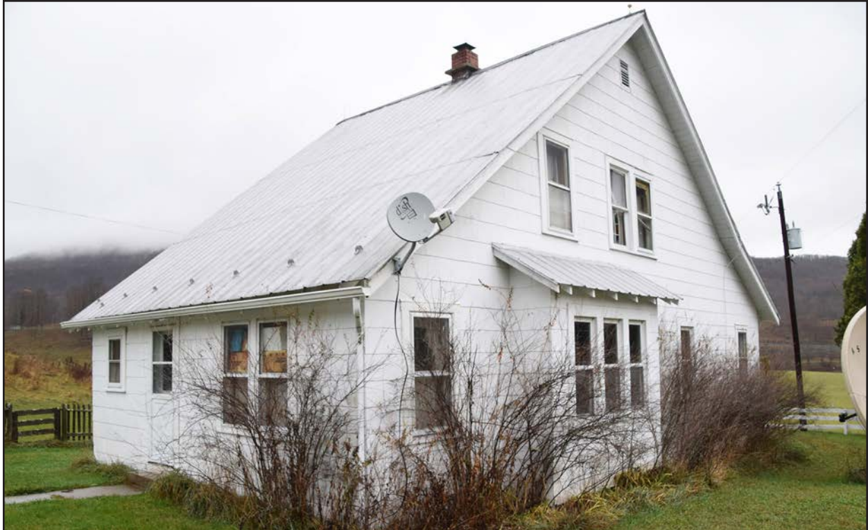
Photo 34. PH-0903, ca. 1940s house, facing east.
