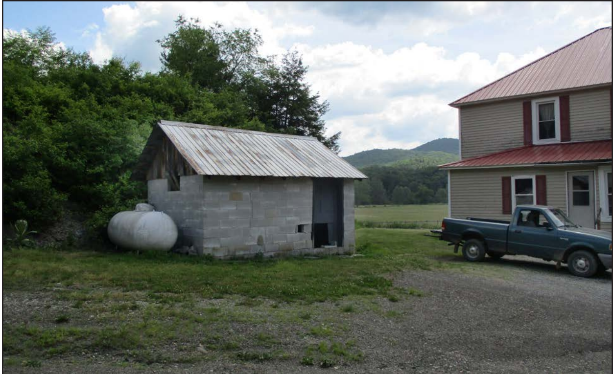
Photo 28. PH-0954, shed, facing east
