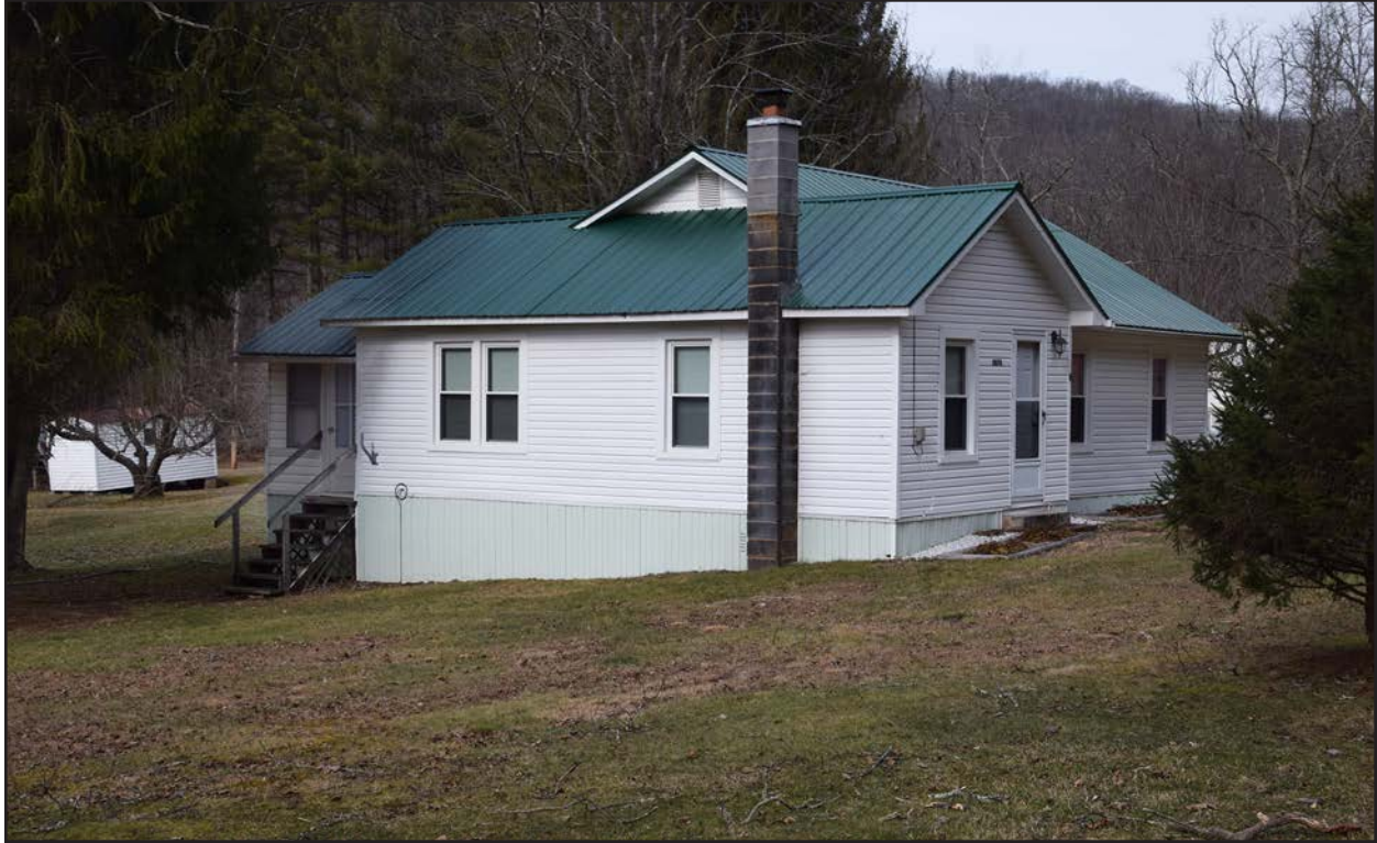
Photo 23. PH-0490, facing north.
