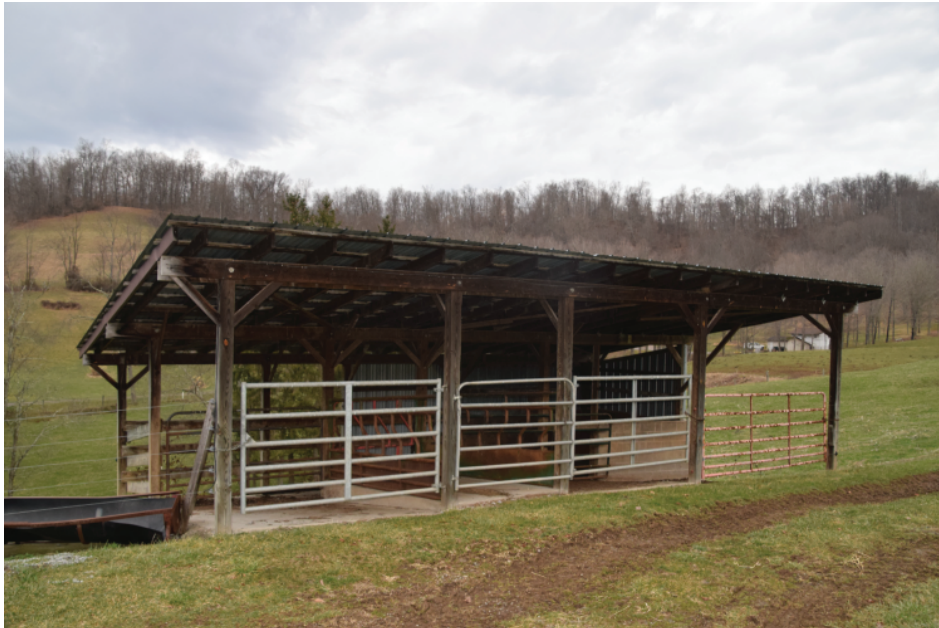
UP-0818, Shed, facing west.
