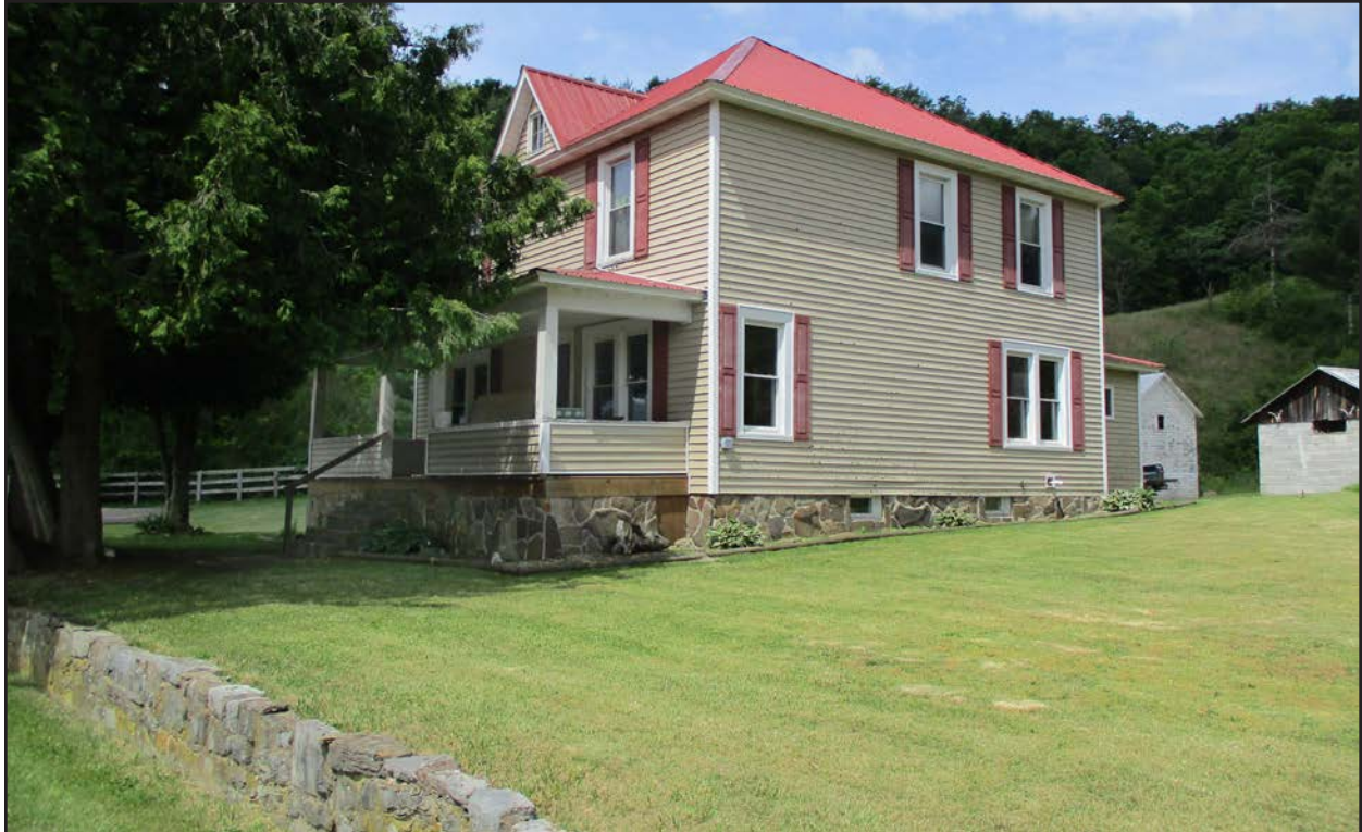
Photo 26. PH-0954, dwelling, facing west.
