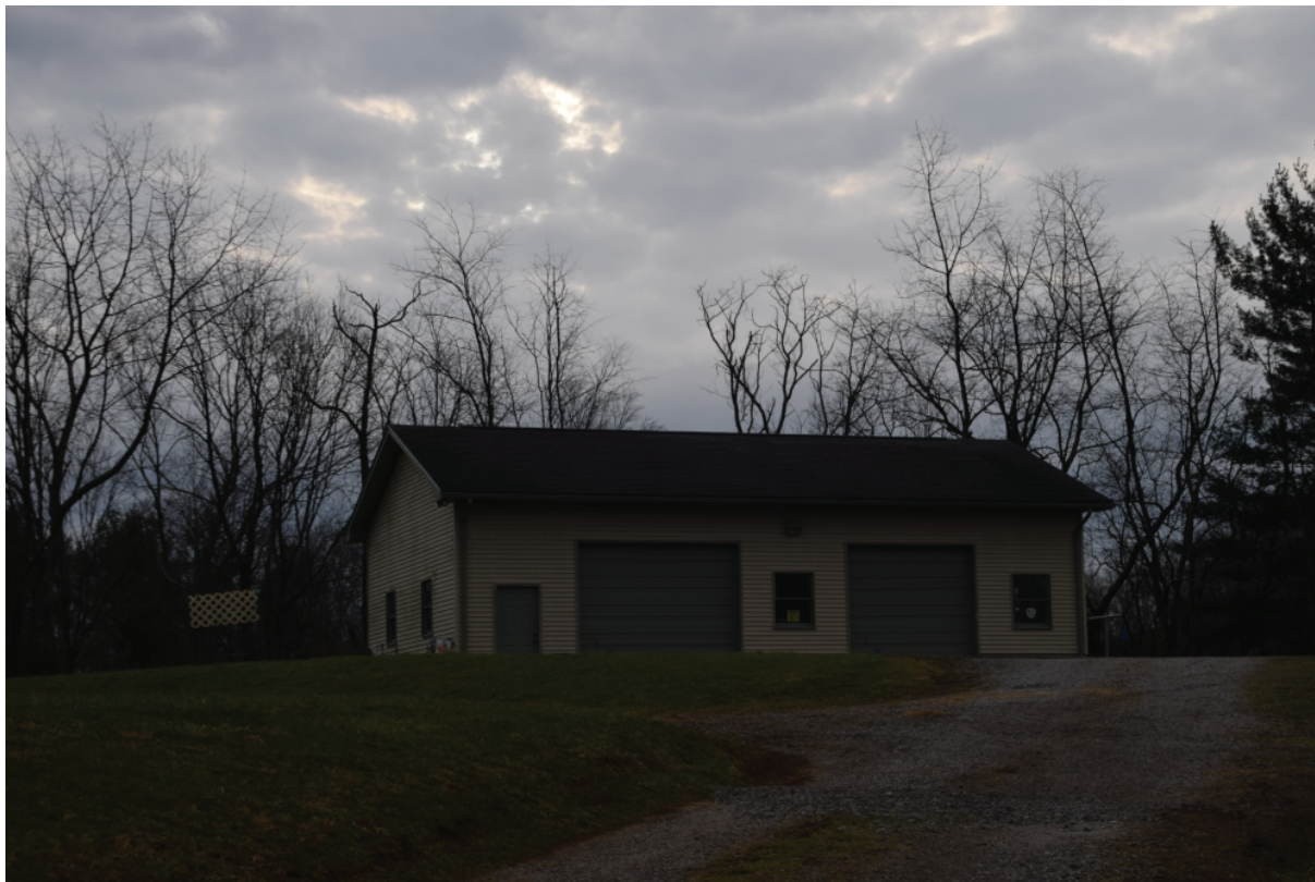
UP-0818, Garage, facing east.
