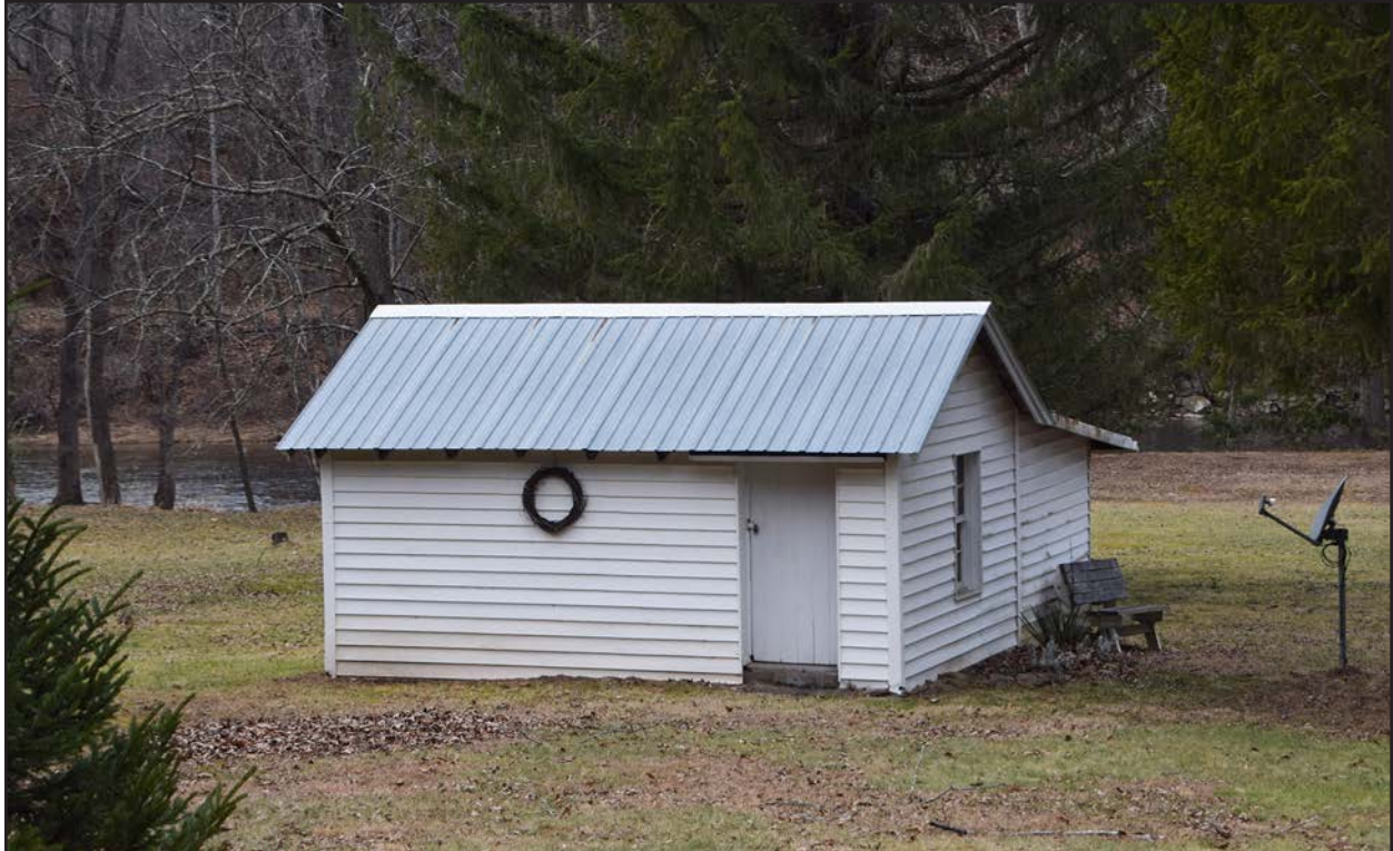
Photo 24. PH-0490, facing northwest.
