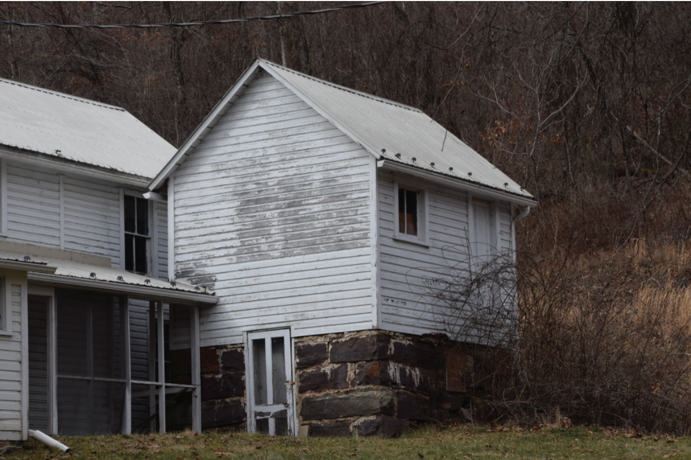
PH-0037-64, smokehouse/root cellar, facing northwest.
