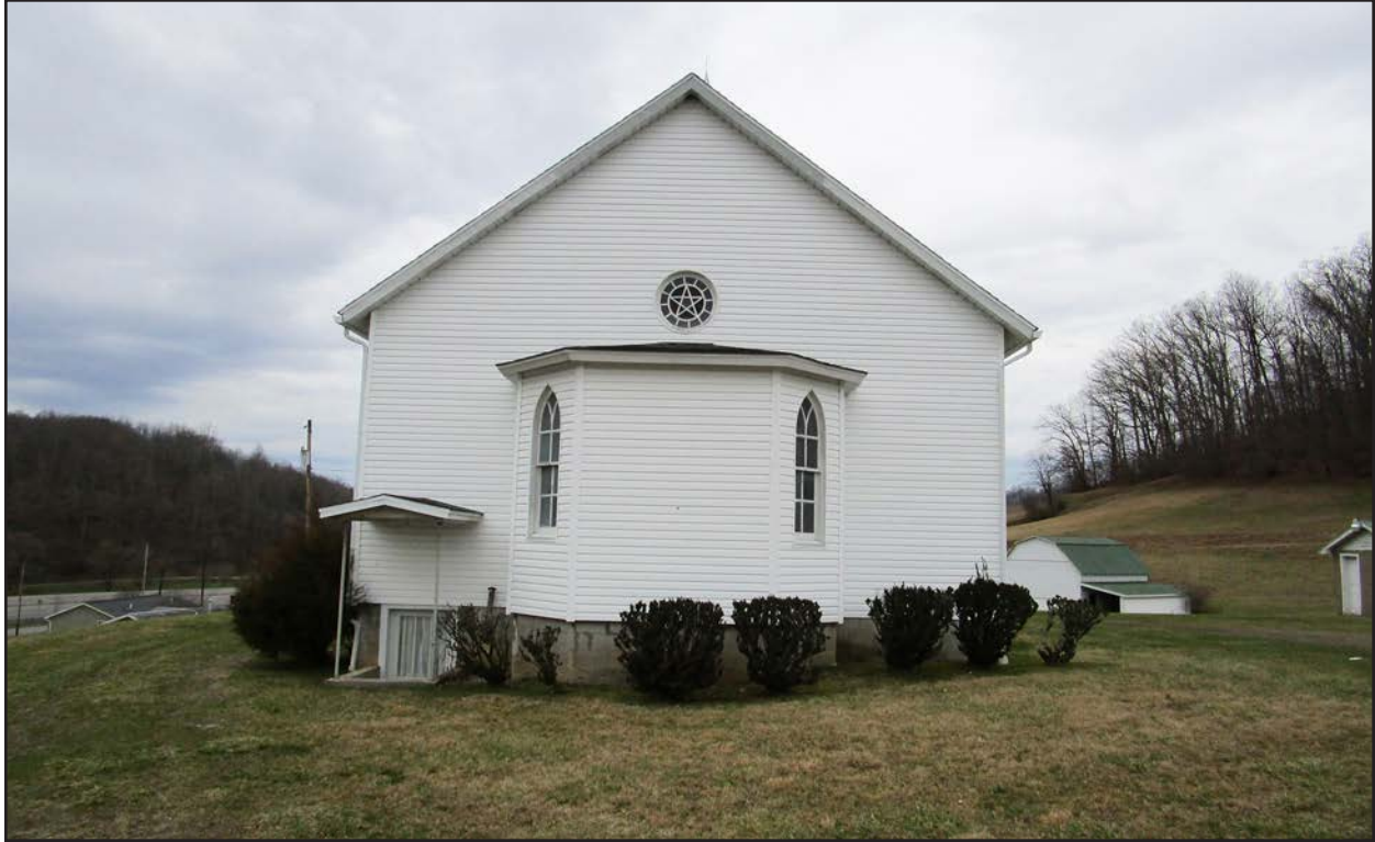
Photo 41. UP-0113, Gothic Revival Church, facing west.
