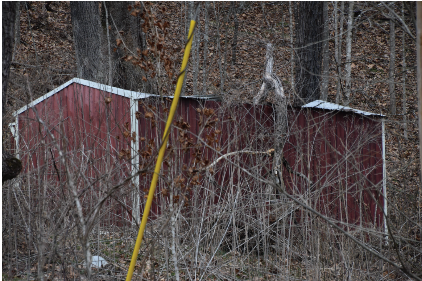
PH-0037-64, shed, facing north.
