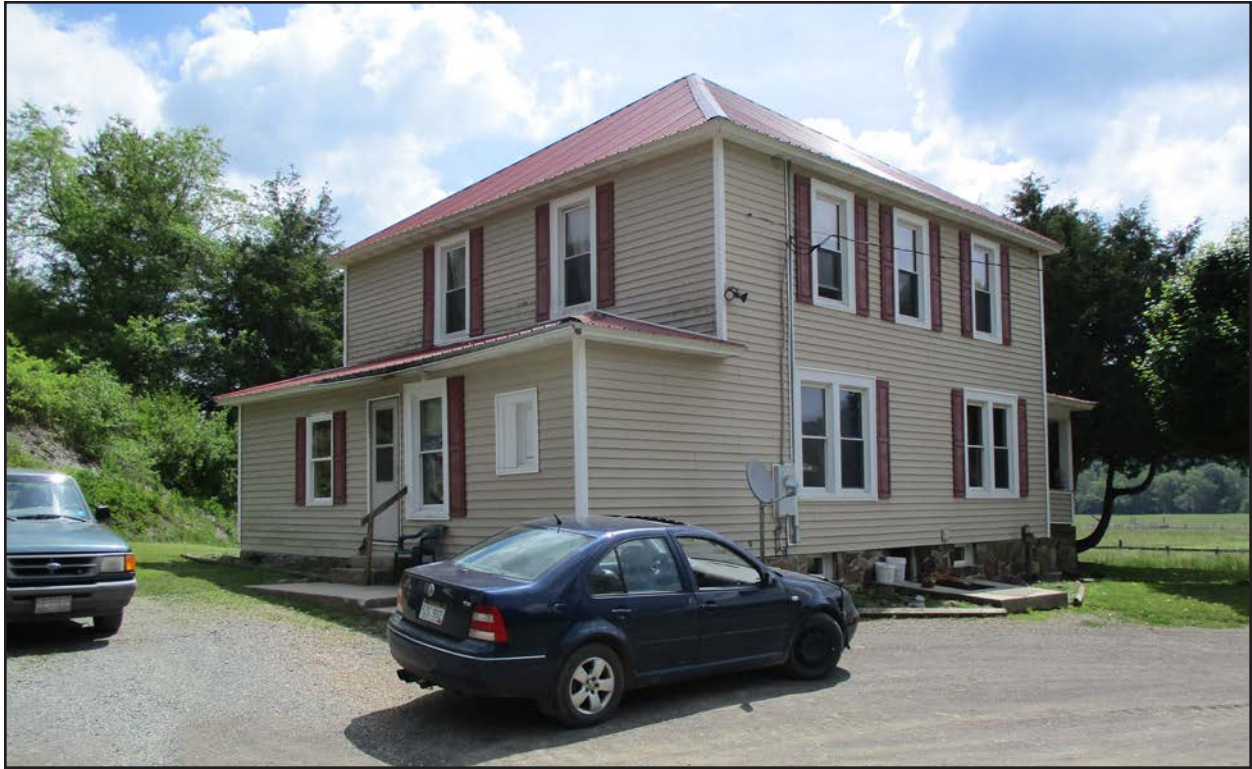
Photo 27. PH-0954, dwelling, facing east.
