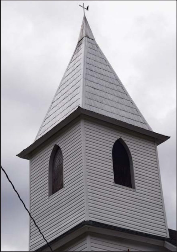
Photo 38. UP-0113, Gothic Revival Church, bell tower, facing northeast.
