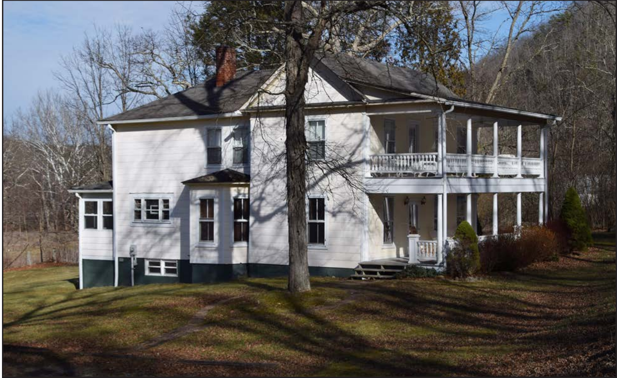
Photo 13. PH-0462, facing northeast.
