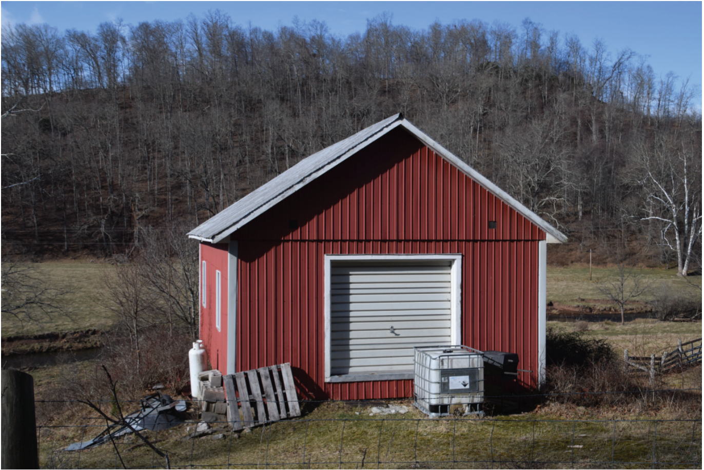
PH-0462, shed, facing north.
