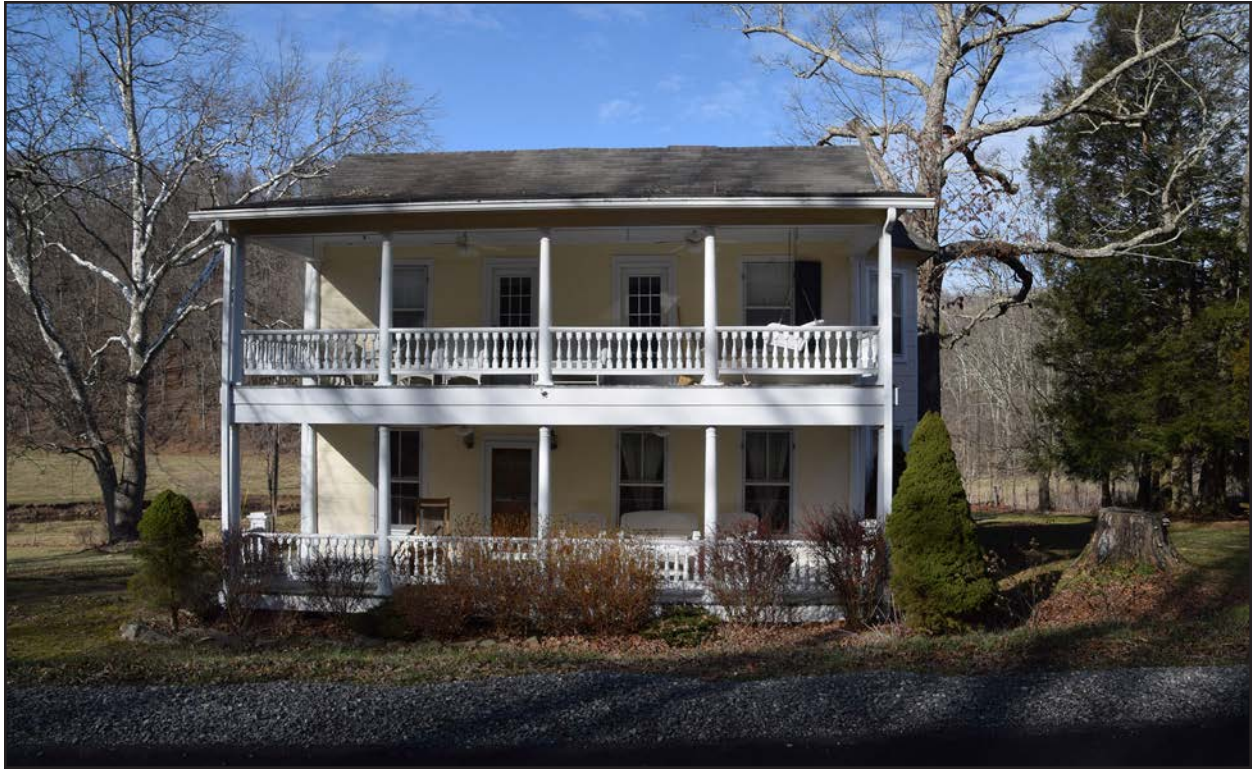
Photo 11. PH-0462, facing north.
