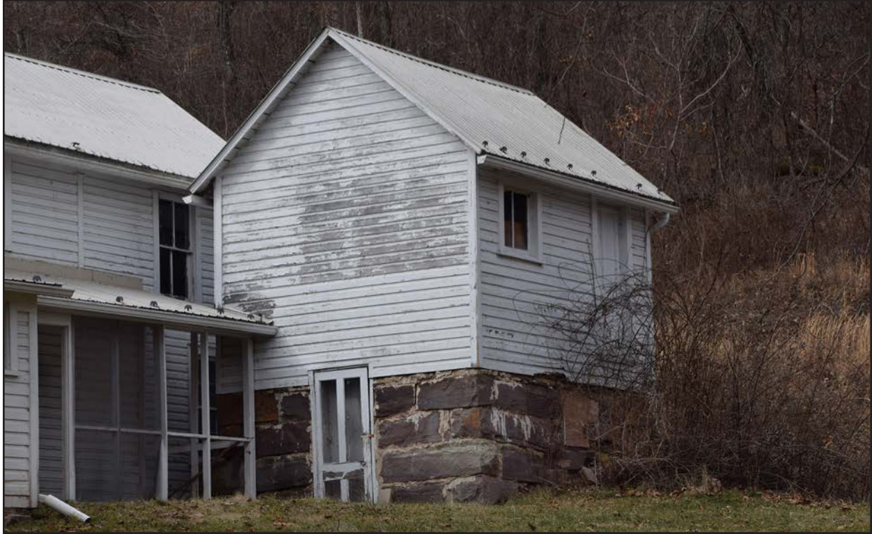
Photo 3. PH-0037-64 smokehouse/root cellar, facing northwest.
