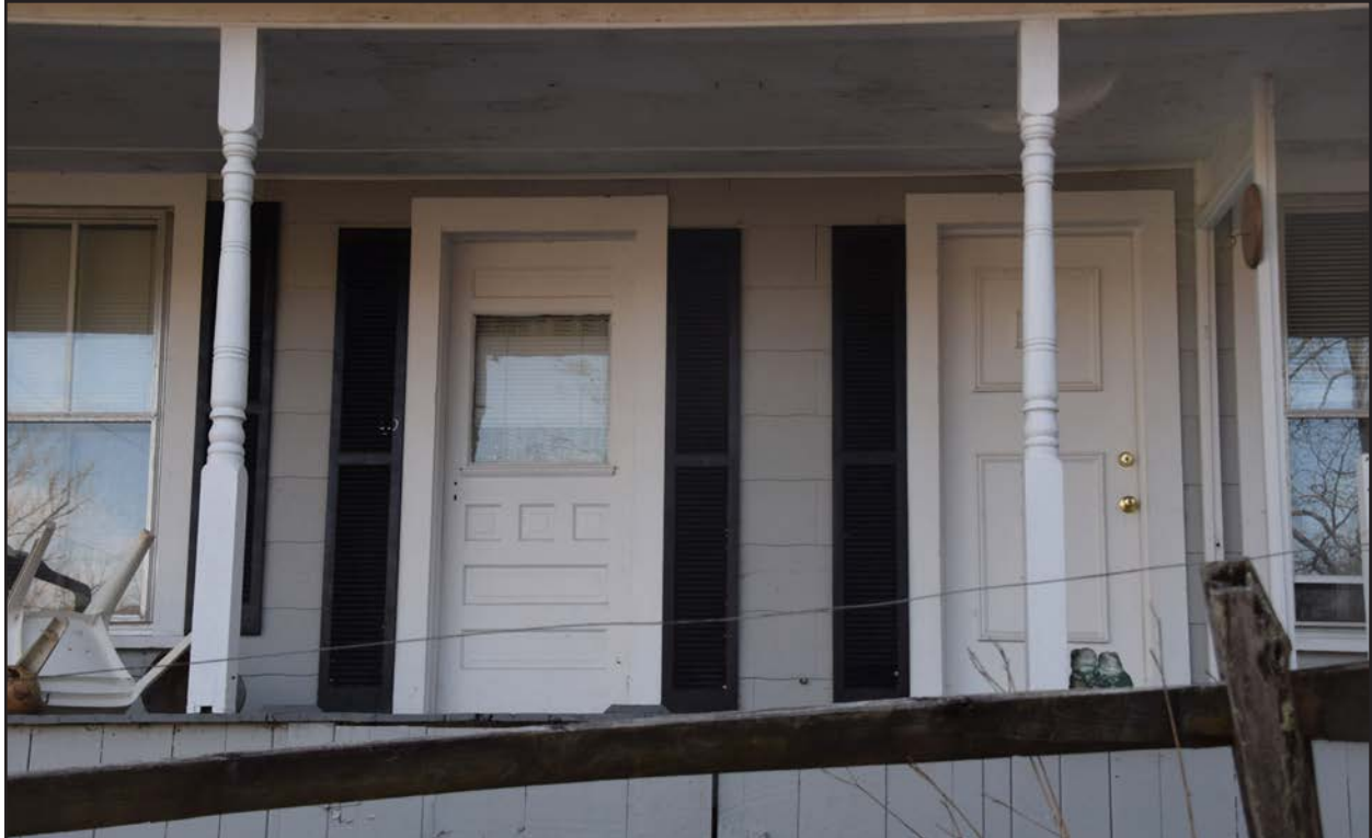
Photo 18. PH-0460, front detail, facing south.
