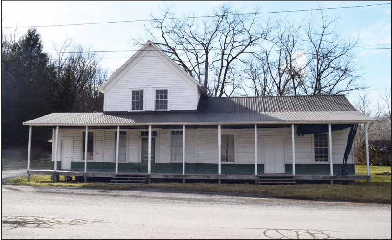
Photo 7. PH-0037-65, store, facing west.
