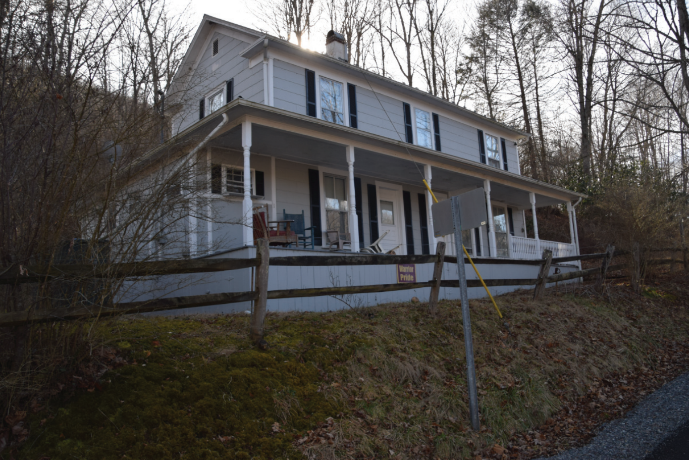
PH-0470, facing southwest.
