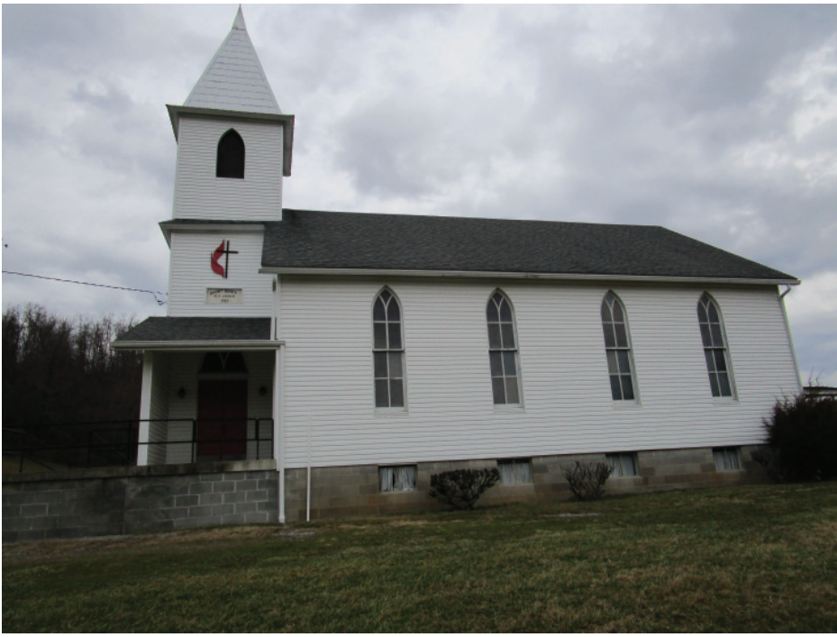
UP-0113, Gothic Revival Church, facing north.
