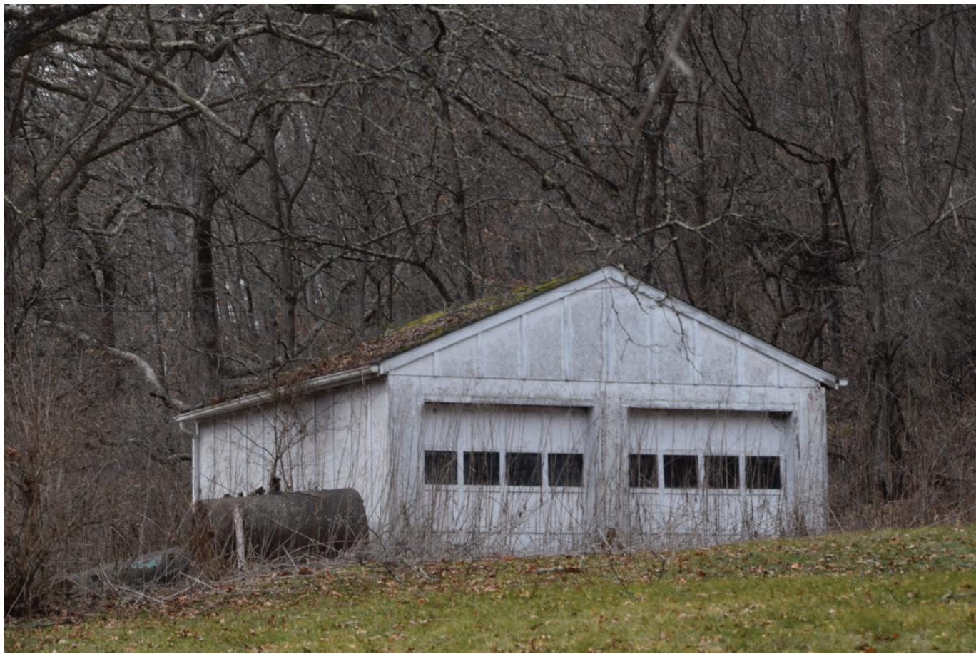
PH-0037-64, garage, facing west.
