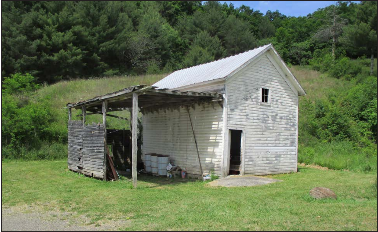
Photo 29. PH-0954, shed, facing west.
