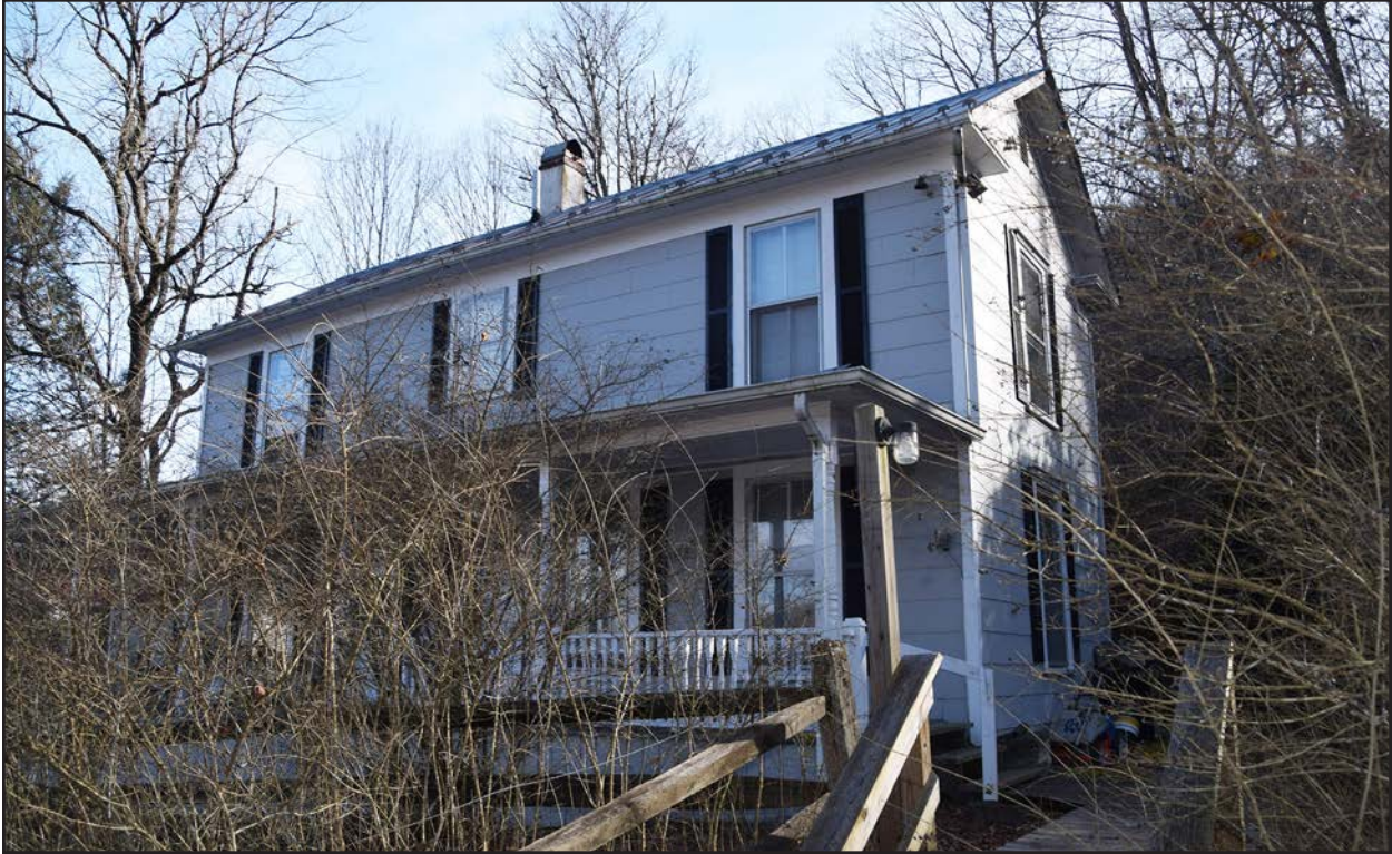
Photo 19. PH-0470, facing southeast.
