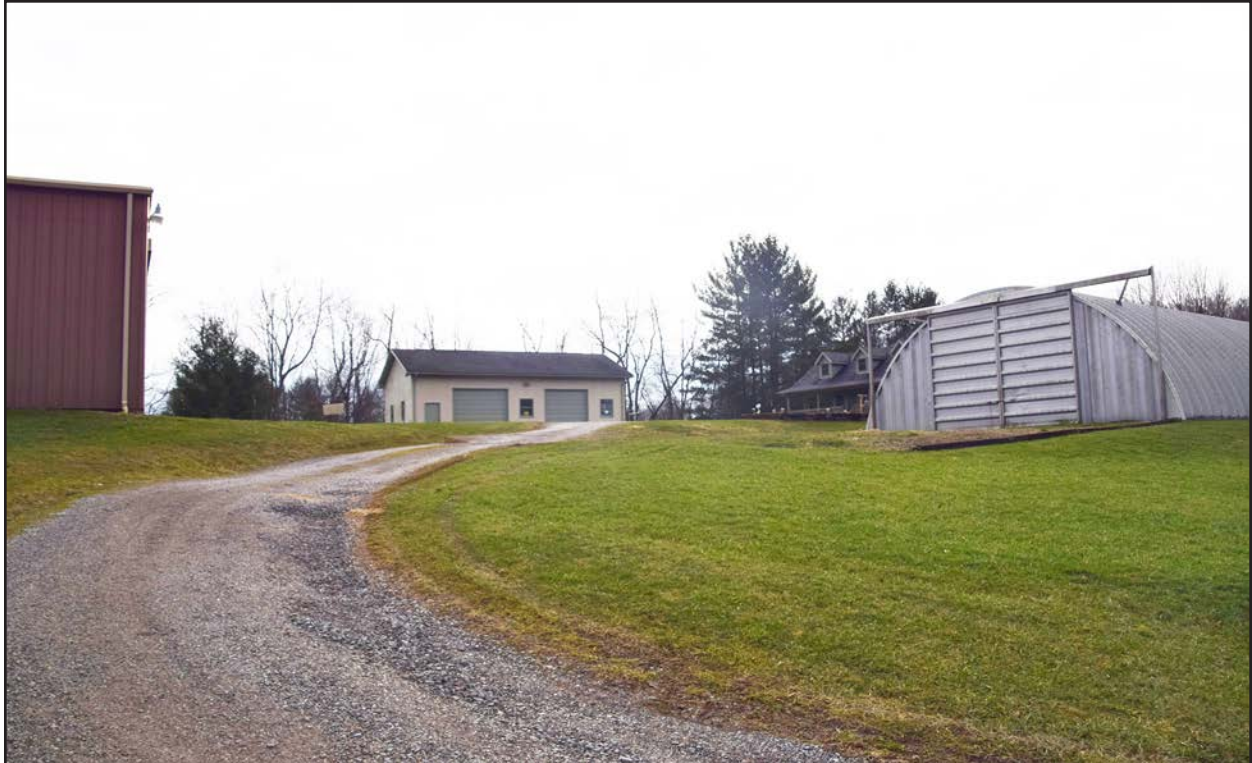
Photo 34. UP-0818, outbuildings, facing southeast.
