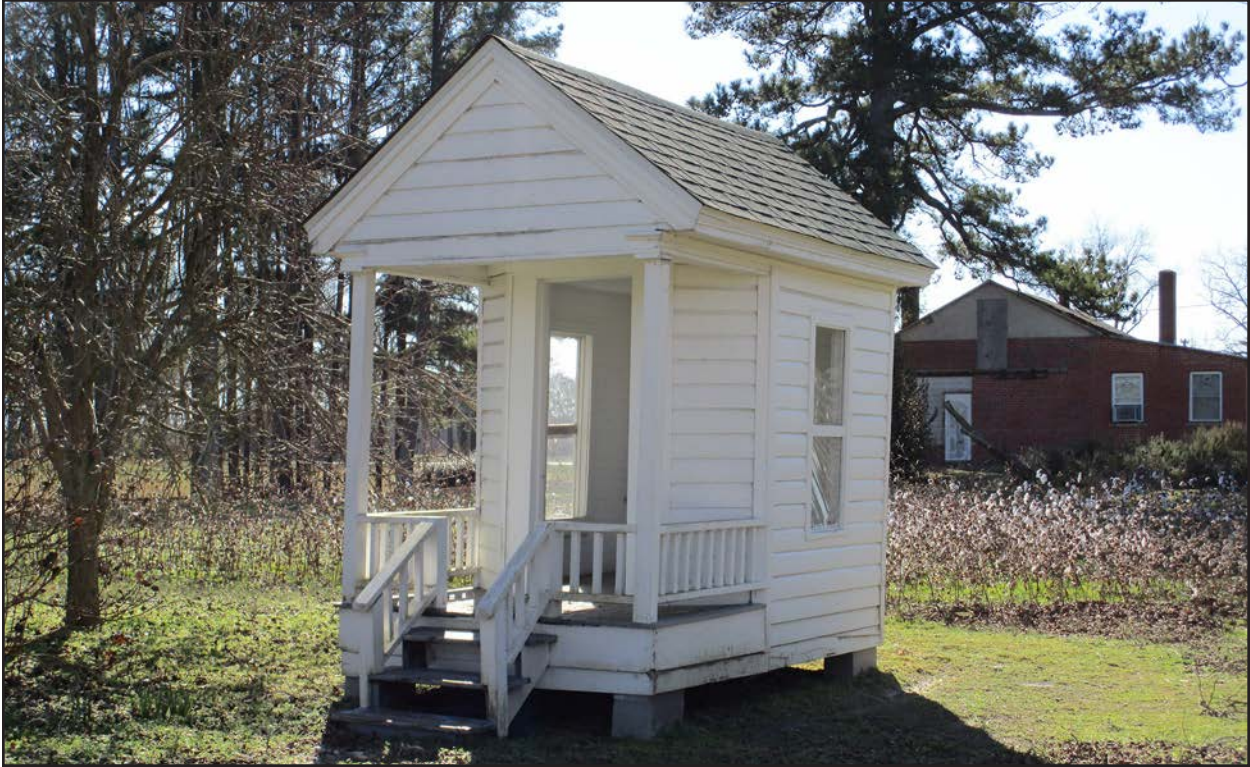
Photo 15. HX0021, accessory building, facing south-southwest.
