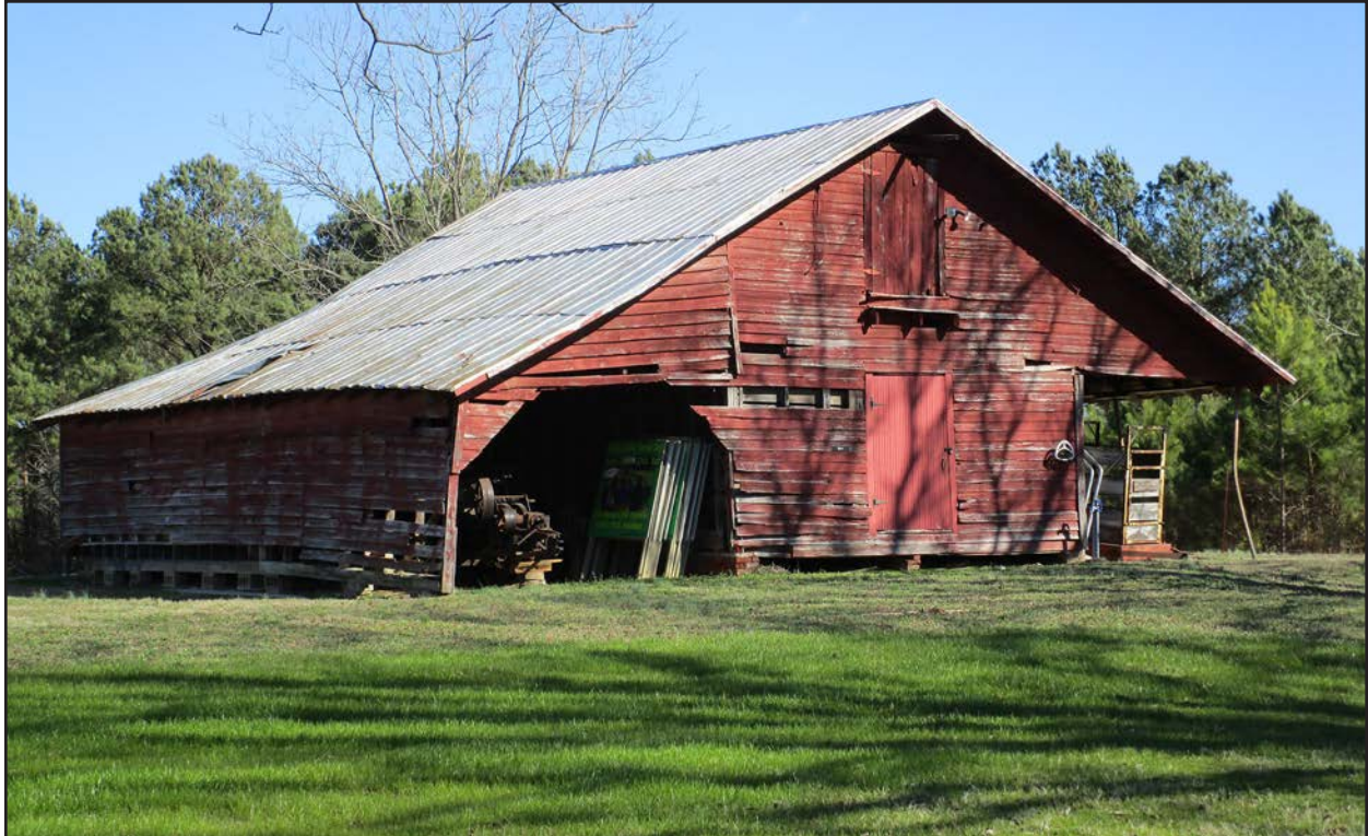
Photo 14. HX0021, corn and equipment barn, facing east-northeast.
