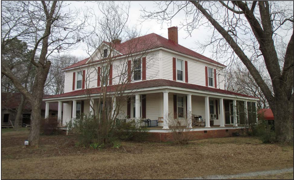
Photo 53. NS0650, house, facing northeast.
