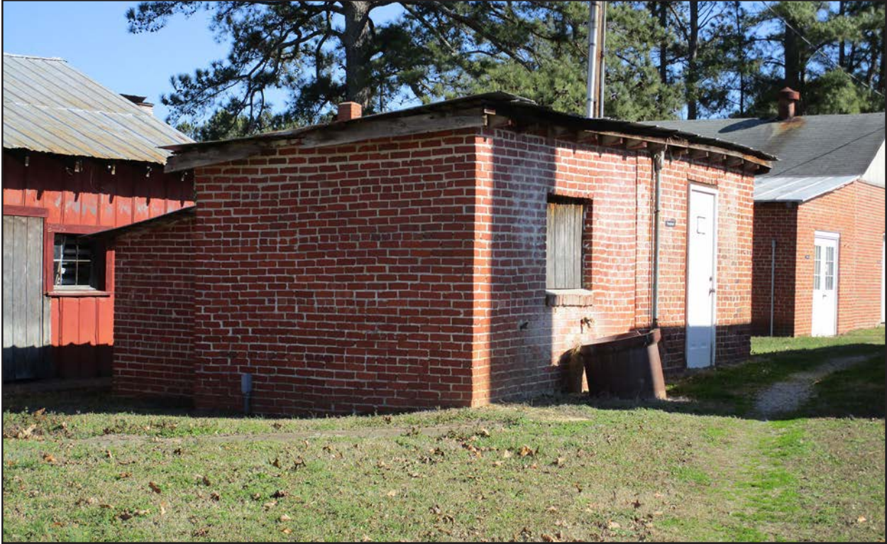
Photo 21. HX0021, pumphouse, facing east.
