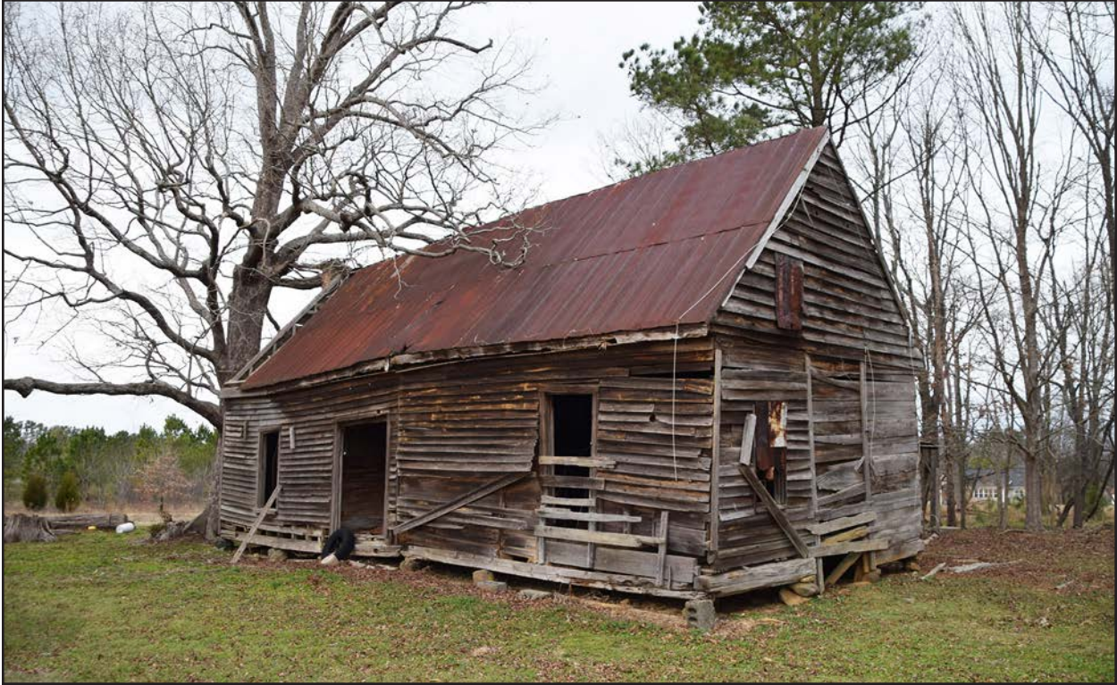
Photo 59. NS0650, cabin, facing northwest.
