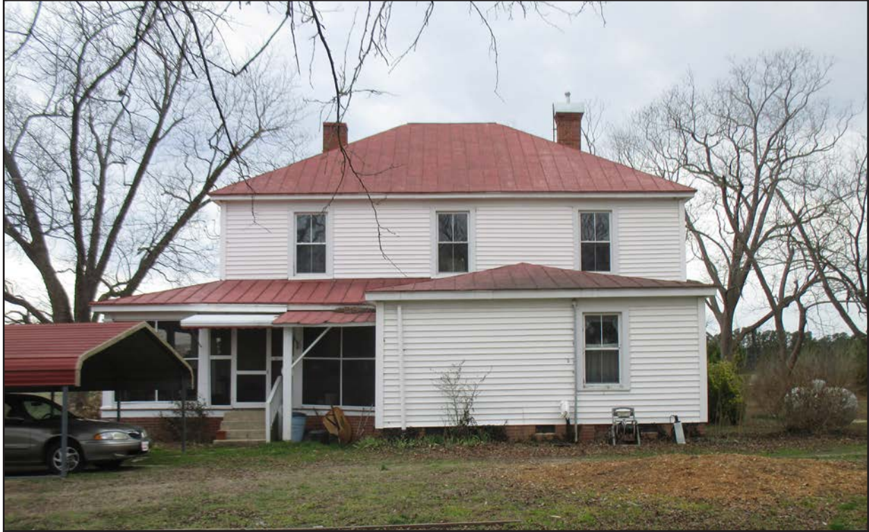
Photo 55. NS0650, house, facing west.
