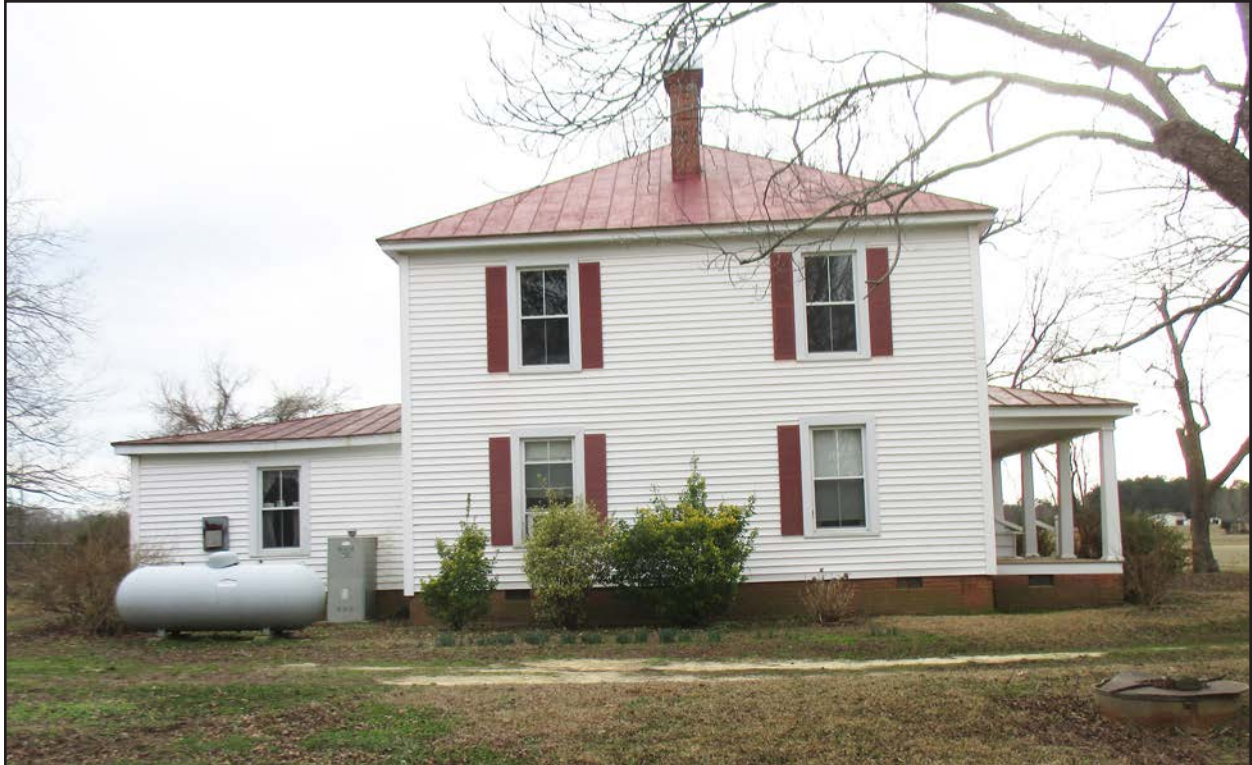
Photo 56. NS0650, house, facing south.
