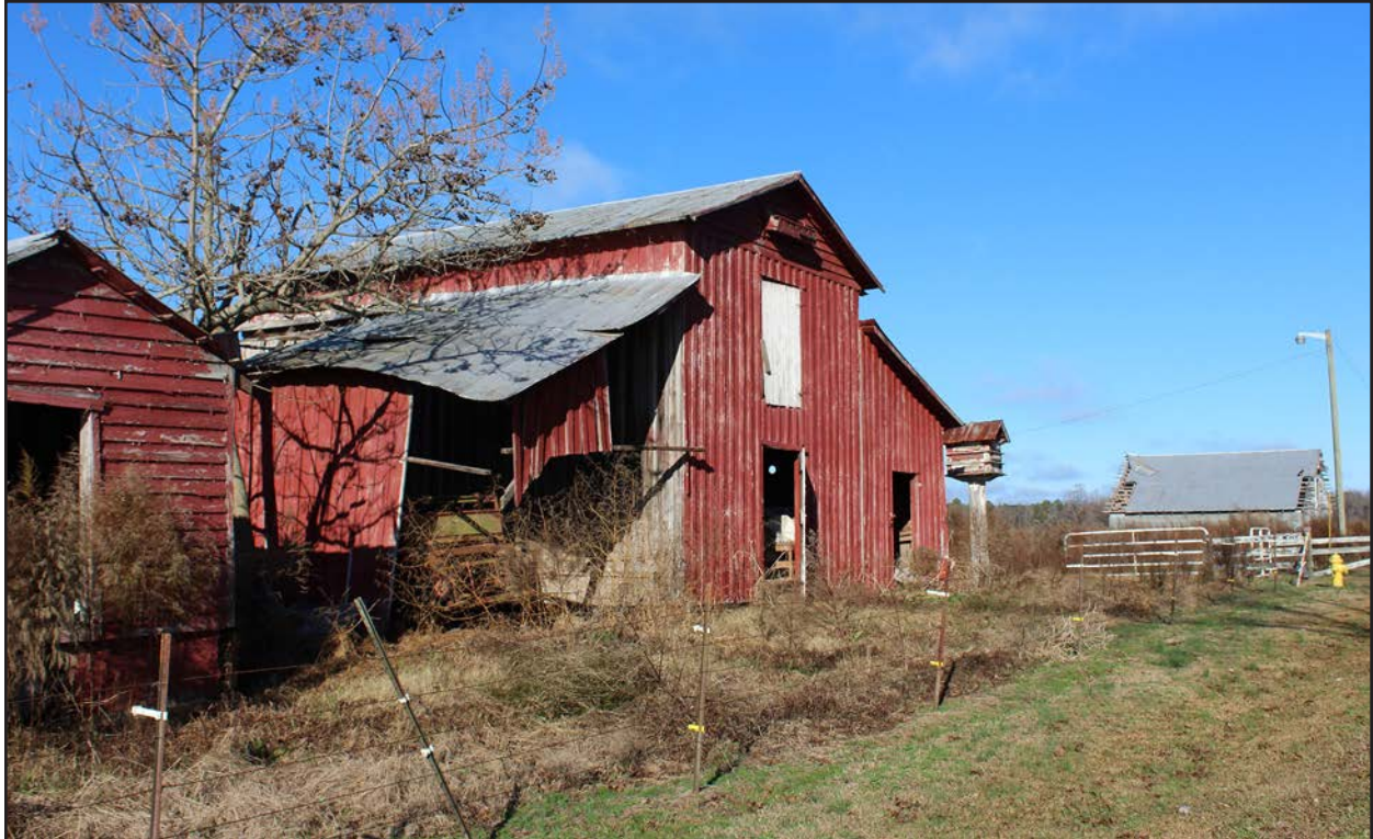
Photo 36. HX0229, facing north-northwest.
