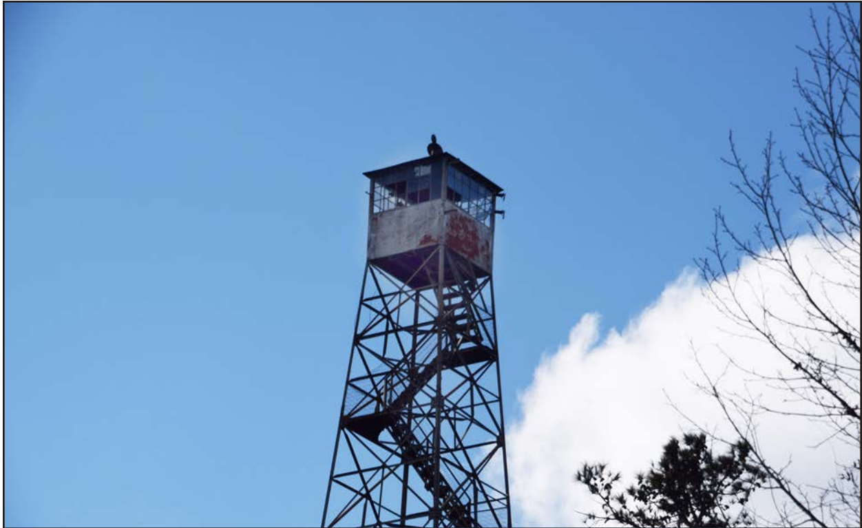
Photo 45. JT1860 (Smithfield Fire Lookout Tower), fire tower observation box, facing west-southwest.
