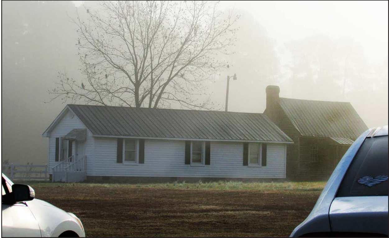
Photo 51. JT1920, accessory structure 2, facing southeast.
