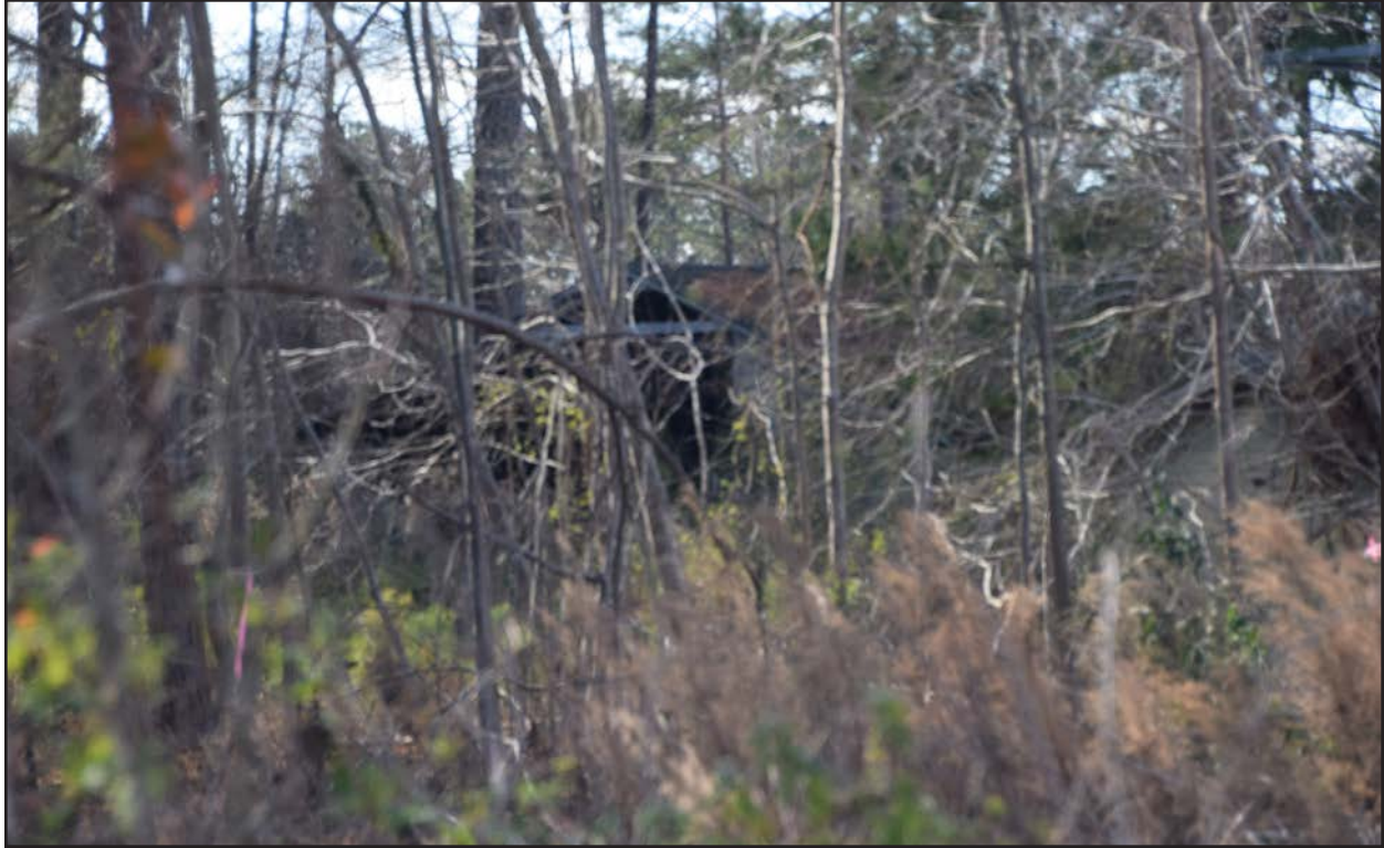
Photo 47. JT1860 (Smithfield Fire Lookout Tower), equipment shed facing northwest.
