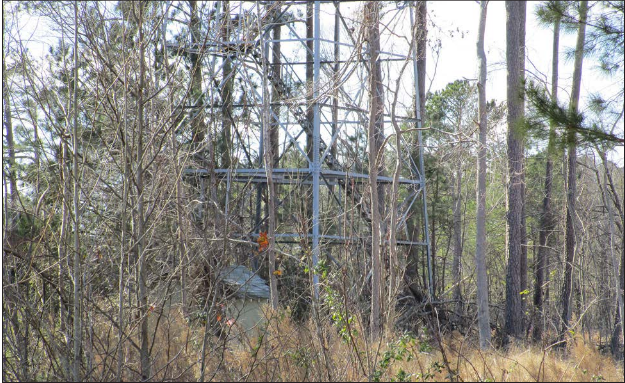
Photo 43. JT1860 (Smithfield Fire Lookout Tower), fire tower base, facing northwest.
