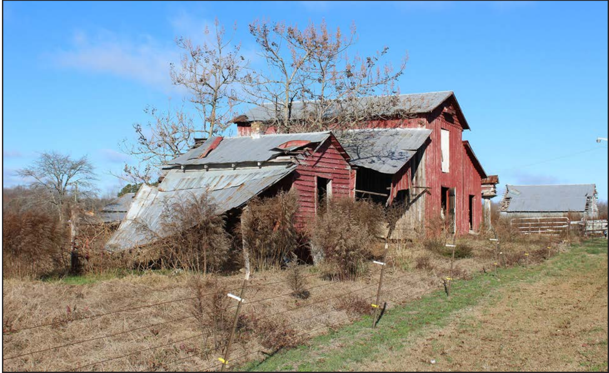
Photo 35. HX0229, facing northwest.
