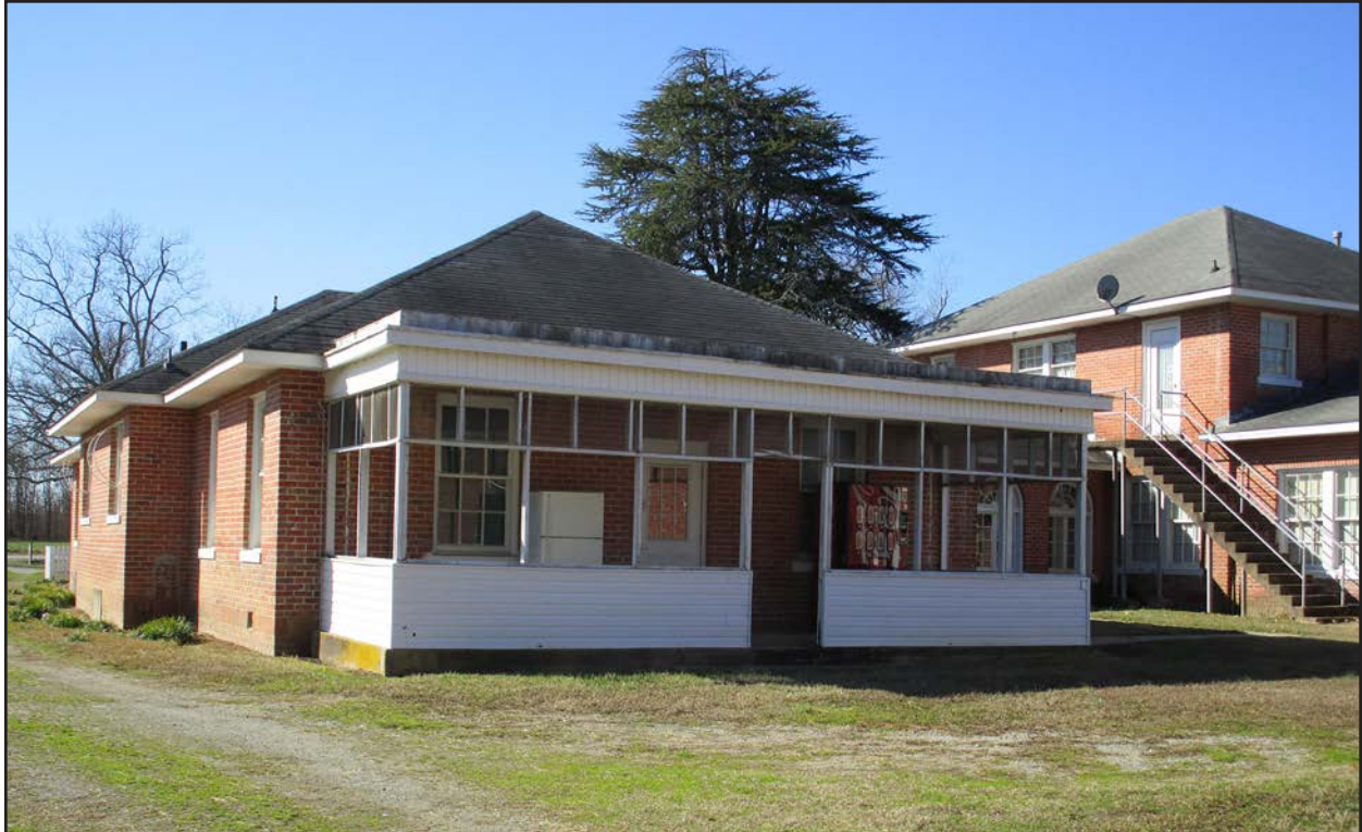
Photo 8. HX0021, facing southwest.
