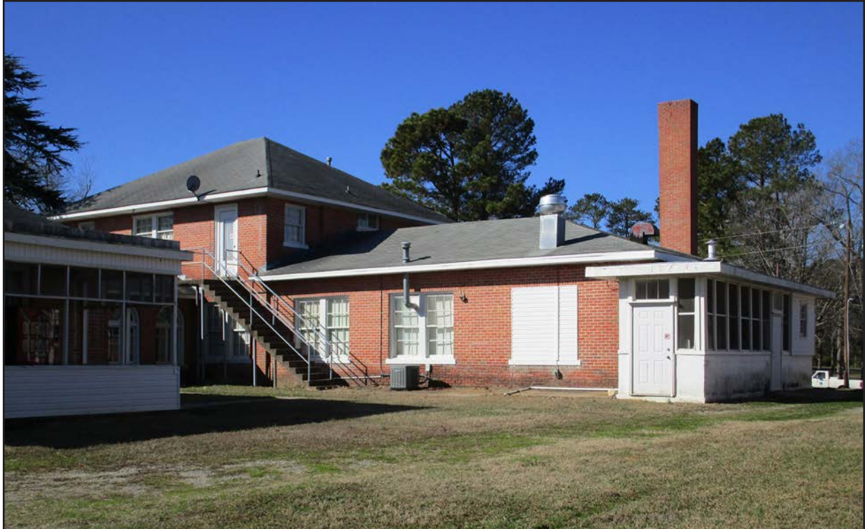
Photo 6. HX0021, view to west.
