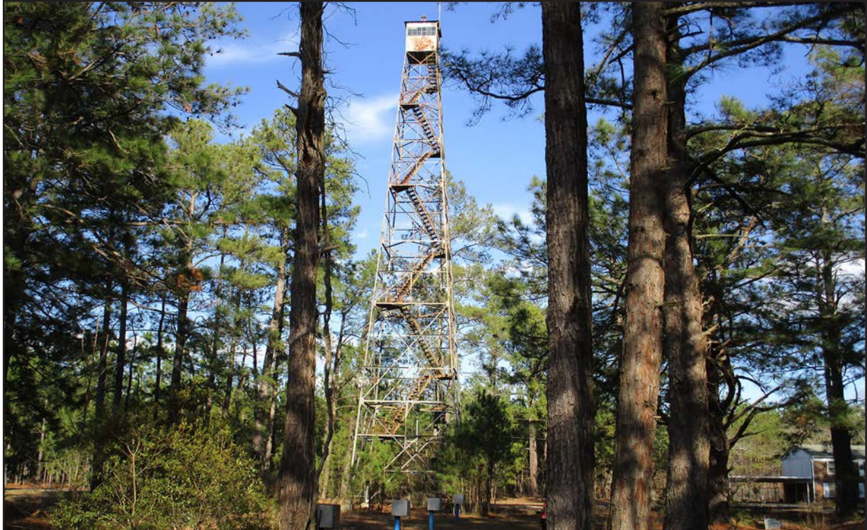
Photo 2. CD1477 (Cedar Creek Fire Tower), facing northeast.
