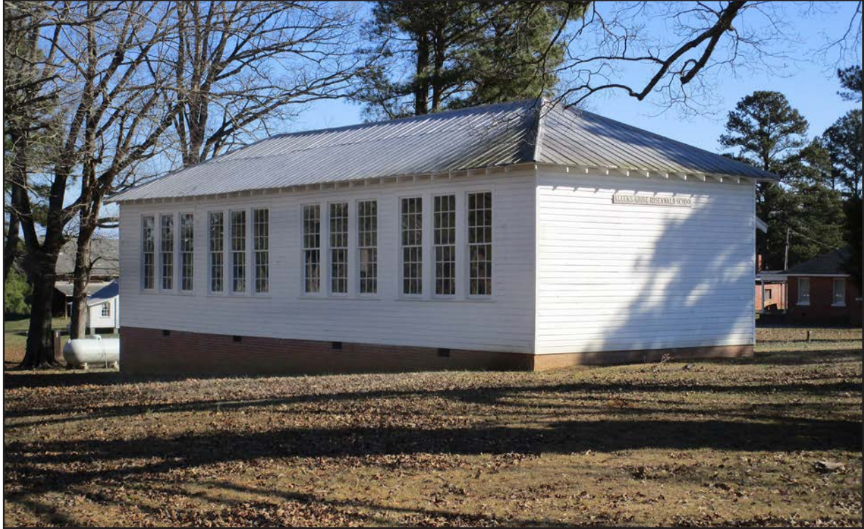
Photo 39. HX1556 (Allen Grove Rosenwald School), facing east.
