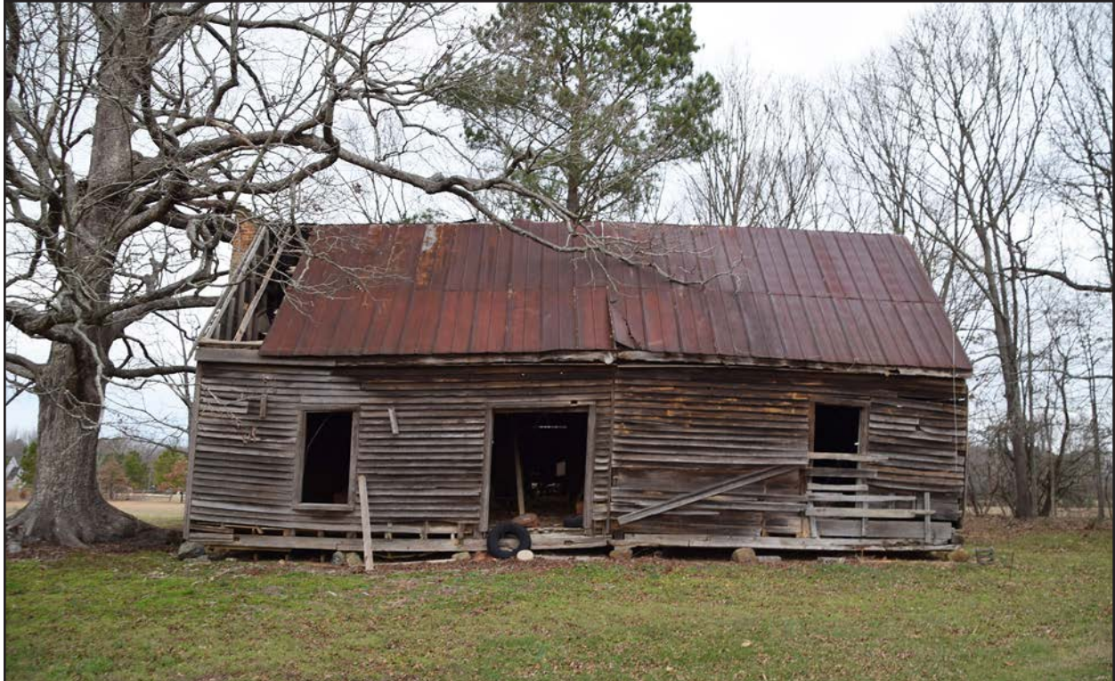
Photo 58. NS0650, cabin, facing north.
