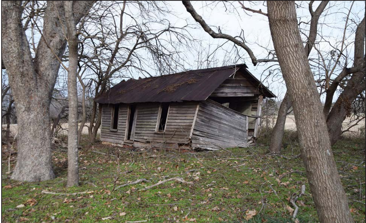
Photo 62. NS0650, summer kitchen, facing northeast
