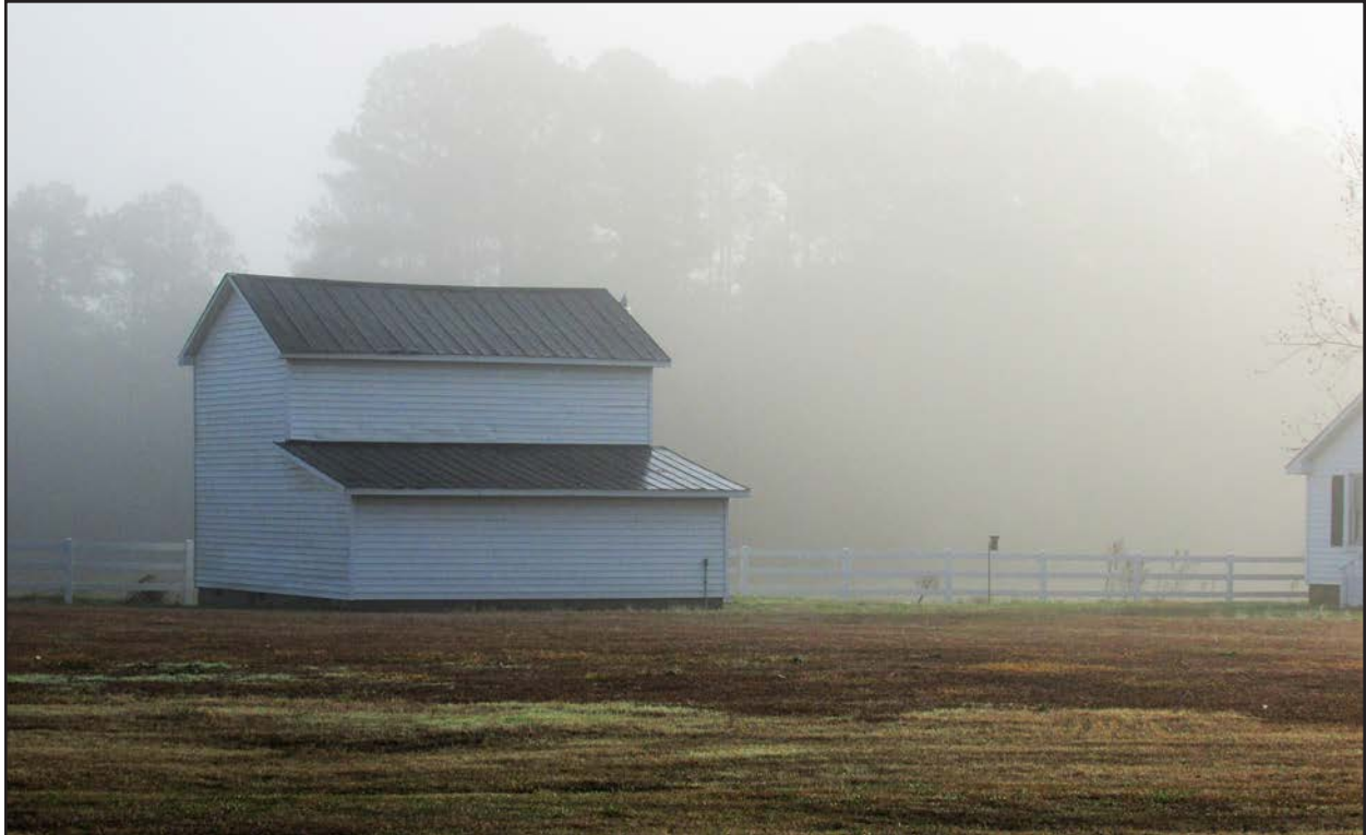
Photo 52. JT1920, tobacco packhouse, facing east-southeast.
