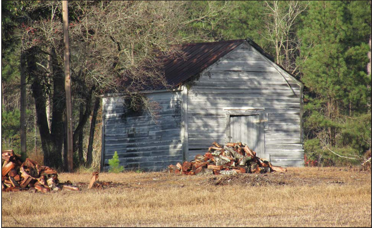
Photo 67. RB0678, shed, facing north.
