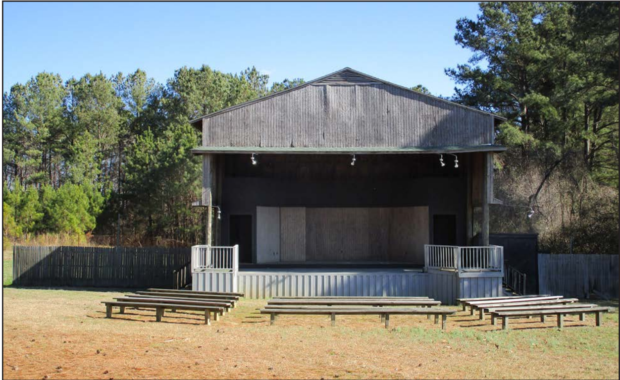
Photo 17. HX0021, amphitheater, facing east.
