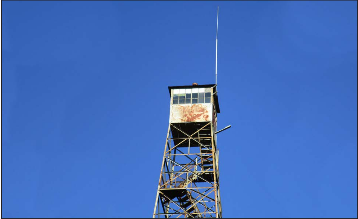
Photo 3. CD1477 (Cedar Creek Fire Tower), facing northeast.
