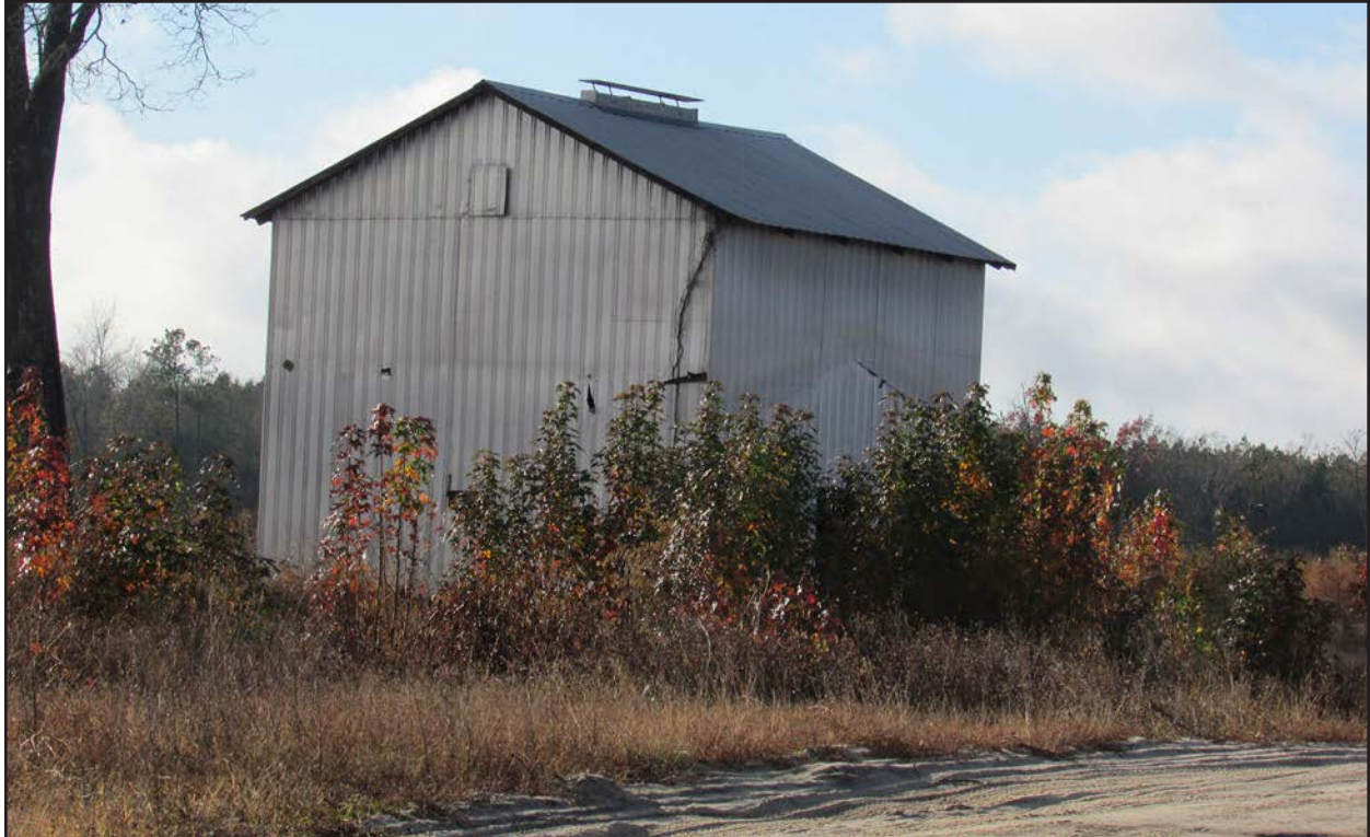
Photo 68. RB0678, tobacco barn, facing north.
