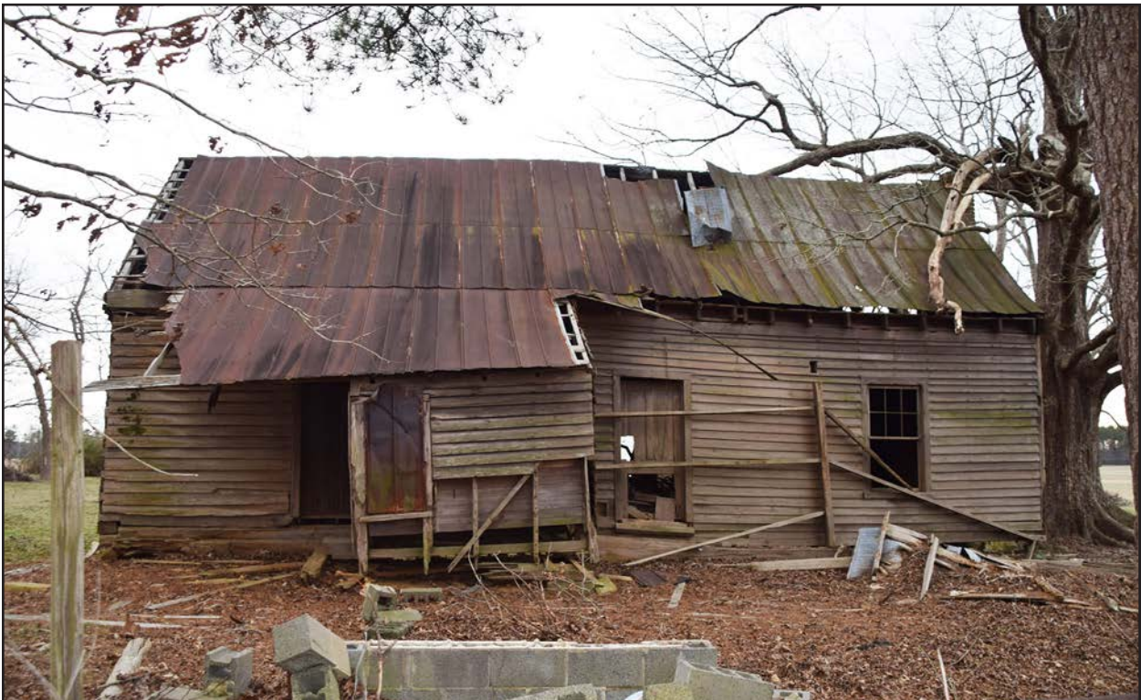
Photo 60. NS0650, cabin, facing south.
