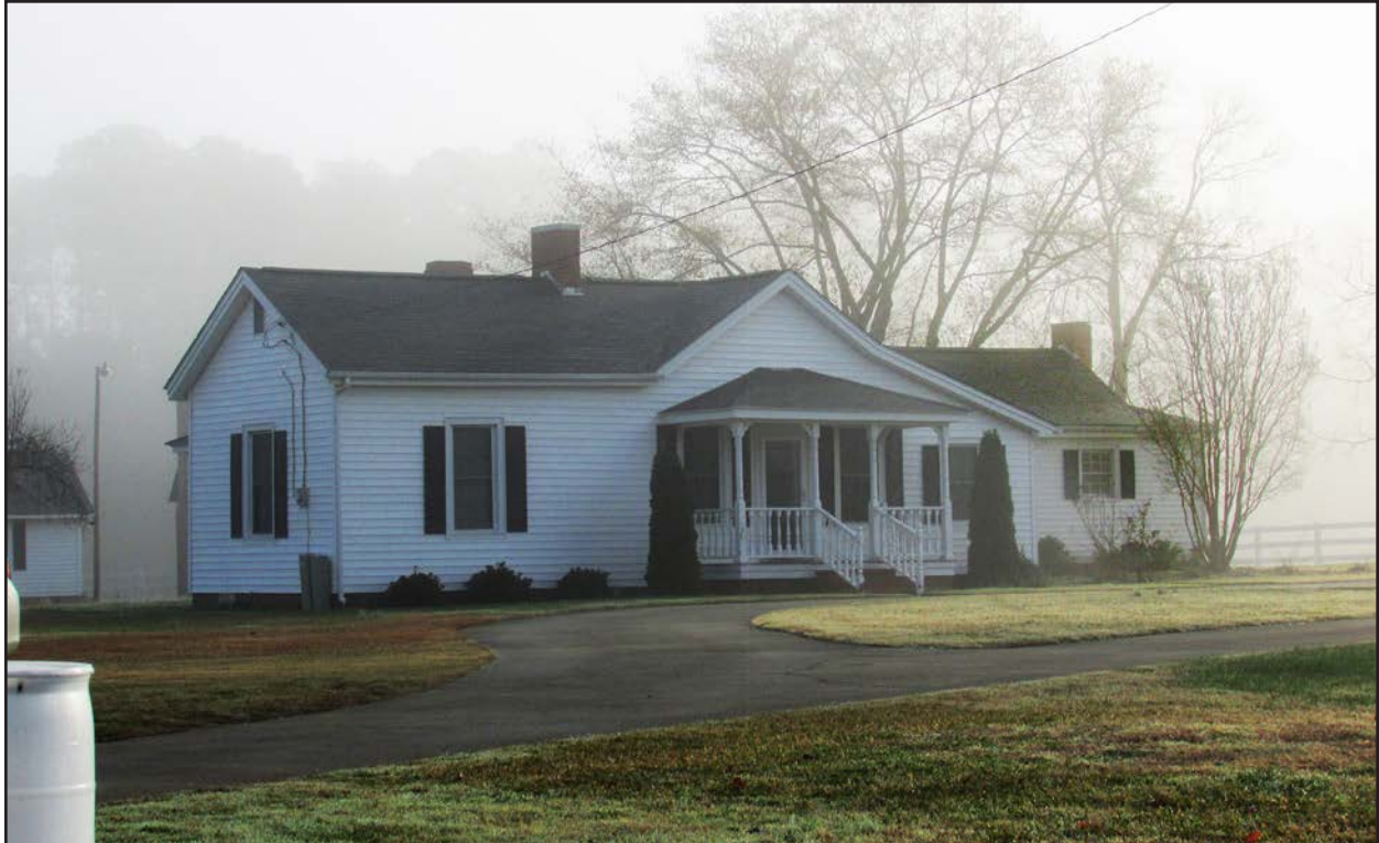
Photo 48. JT1920, facing east-southeast.
