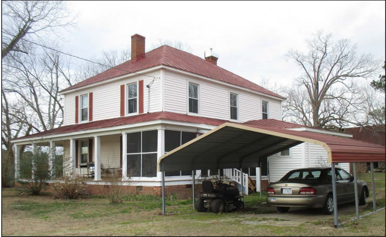
Photo 65. NS0650, carport, facing northwest.
