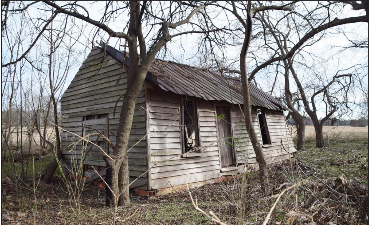
Photo 64. NS0650 summer kitchen, facing northeast.
