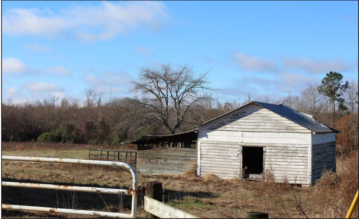
Photo 37. HX0229, facing southwest.
