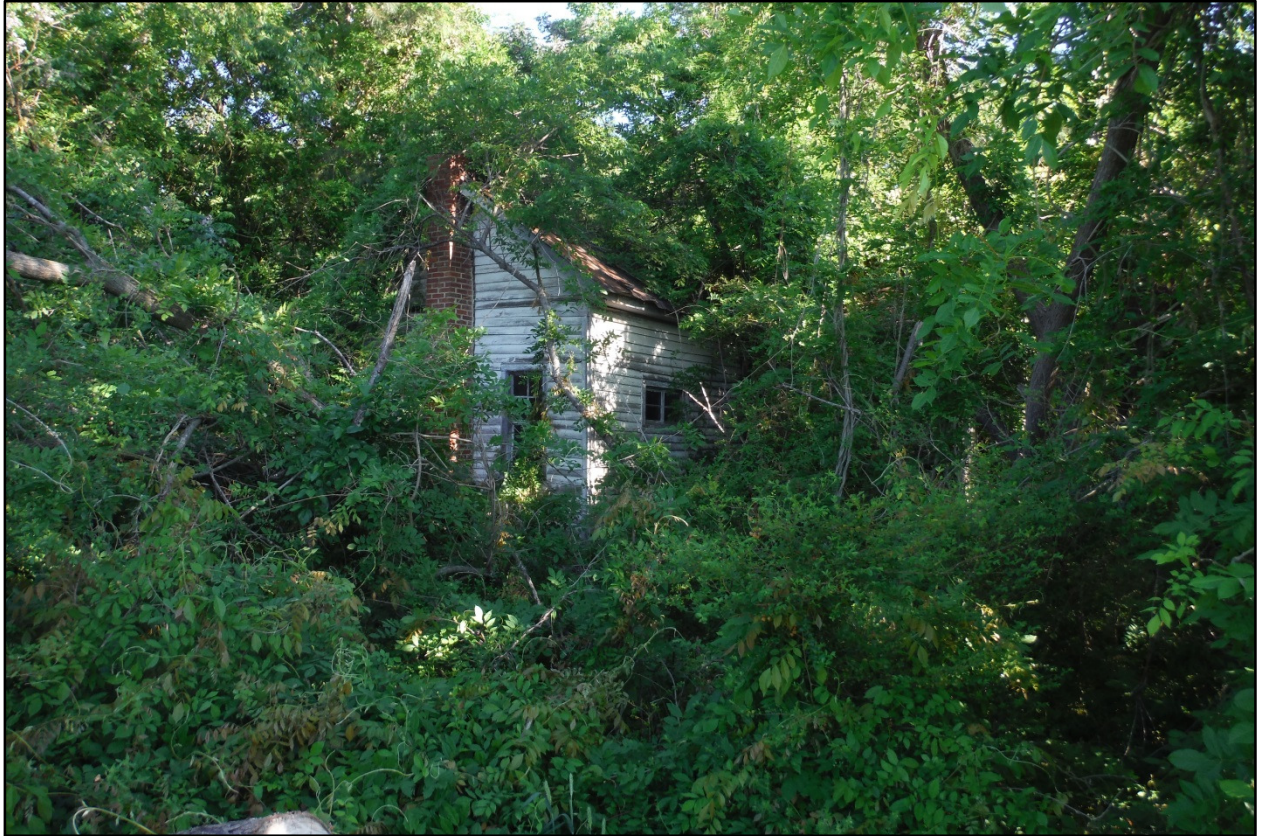
Figure 3. WL2114, view to the northwest.
