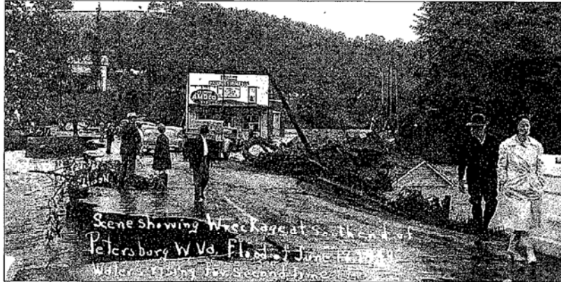
The 1949 flood hit region-wide in Virginia and West Virginia, nearly mimicking the flooding that occurred in 1985. This photo, from the Kent Botkin collection, depicts the damage at the southern end of Petersburg, W. Va., following that storm.
