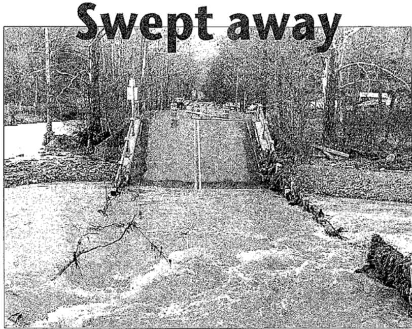
On Nov. 7, 1985, this was The Recorder's powerful front-page image of the bridge across Back Creek on U.S. 84, just east of Route 600, destroyed when high waters pulled the west end of the bridge from its supports shortly after noon on Monday, Nov. 4. It was captured by then news editor Winnie Richardson.
