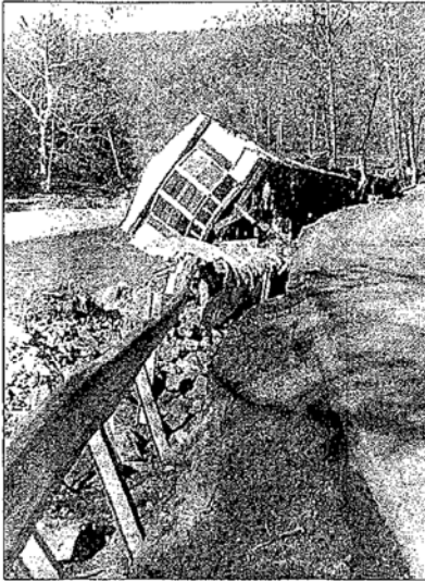
The fast-moving current of the South Branch of the Potomac carried this home down river about a half mile before it came to rest on the riverbank at U.S. 220 south of Franklin, W.Va. (Recorder file photo)
