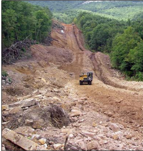
FIGURE VII(o) – A comparatively small 2014 pipeline replacement project in the Jefferson National Forest on Peters Mountain in Giles County, Virginia. A variance to the 500-foot open trench limit was requested for this project. Although slopes exceeded 40%, the DEQ approved the variance request, allowing a 2,000-foot open trench. No water interceptor diversions were installed during trenching. Following a rain event that occurred shortly before the above photo was taken, a Forest Service employee described having “never seen that much sediment move off site before.” A case-study report is posted at www.pipelineupdate.org/case-study-no-1/ . The Dominion Pipeline Monitoring Coalition conducted a study of open-trench variance requests for pipeline construction projects in Virginia. Fifteen variance requests were submitted between January 2011 and July 2014, and all were approved. The authorized open-trench lengths ranged between 500 feet and 15 miles, with an average length of 2.3 miles. Nothing was discovered in DEQ documents to indicate that an analysis was conducted to ensure that these variances would not cause illegal discharges and water quality degradation.
