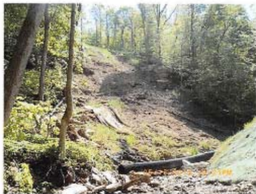
Photo 3: N 39° 52.3773' W 80° 41.1271' Bartlett's Run. Flume pipe, sand bags and slip material in stream.
