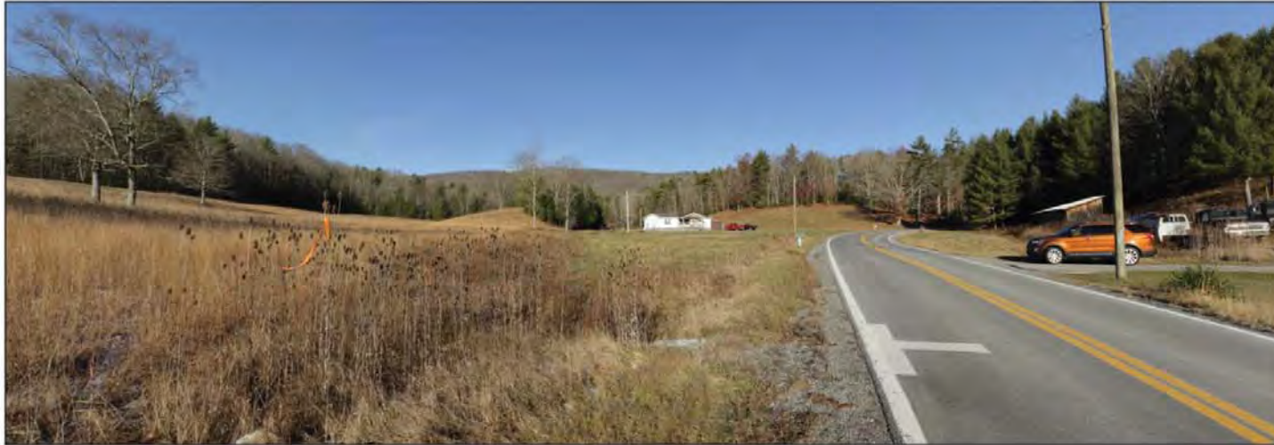
SSF 08 - State Route 96, Looking Northwest - Existing View
