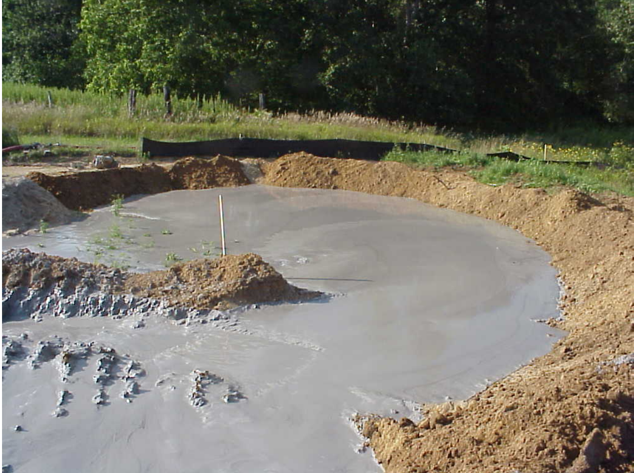
Figure 4. Inadvertent Drilling Fluid Return
