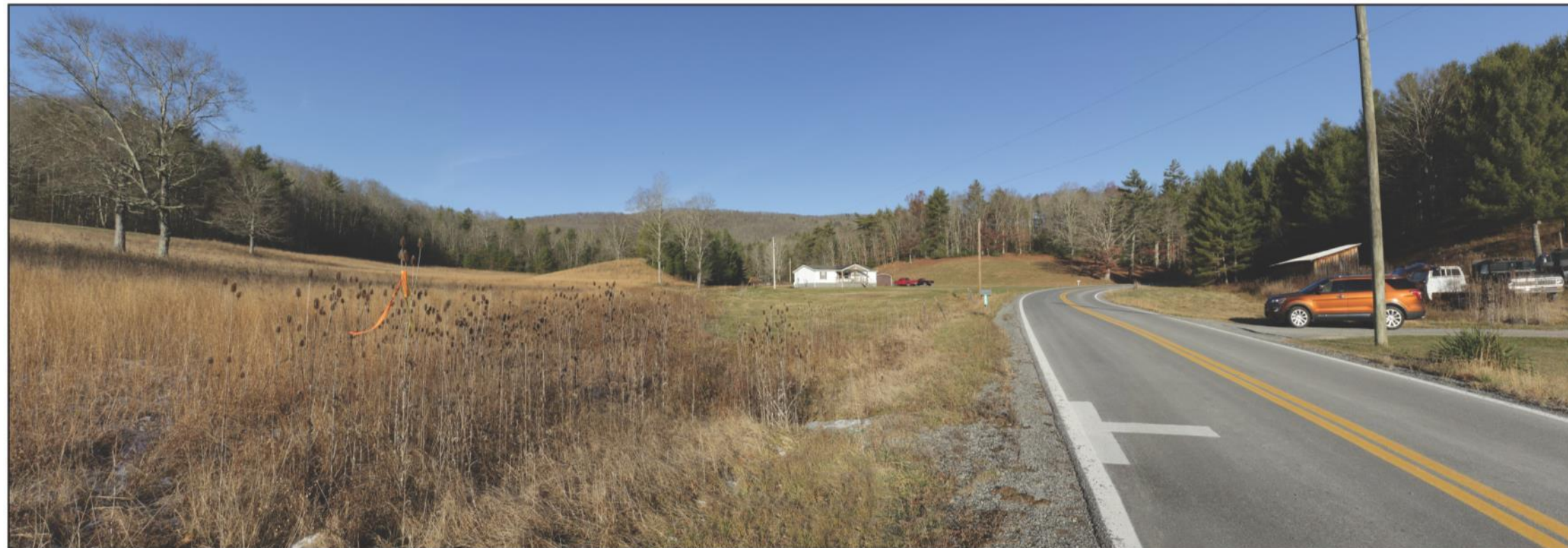
SSF 08 - State Route 96, Looking Northwest - Existing View
