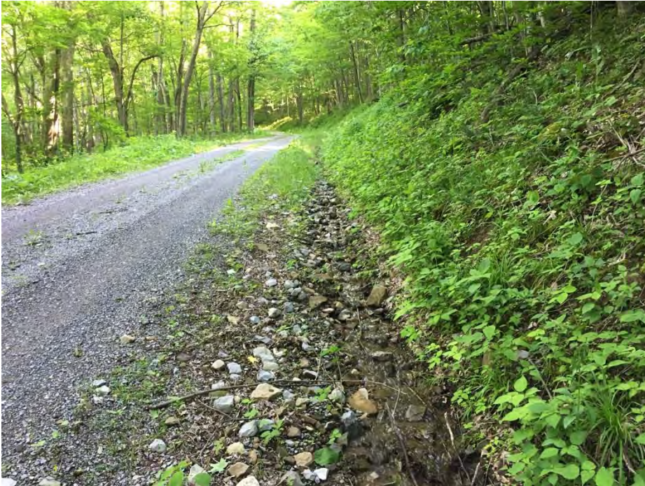
Waterbody SPOA434 facing north upstream
