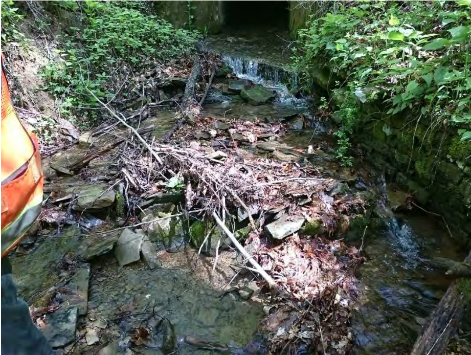
Waterbody SPOA404 facing north upstream
