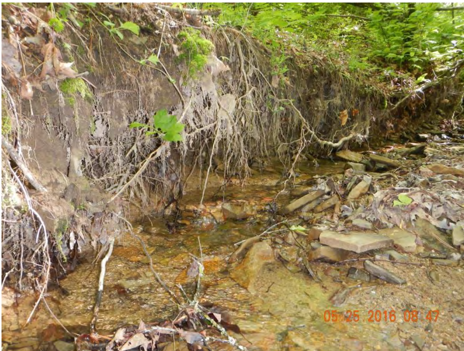
Waterbody SPOA408 scouring facing northwest across
