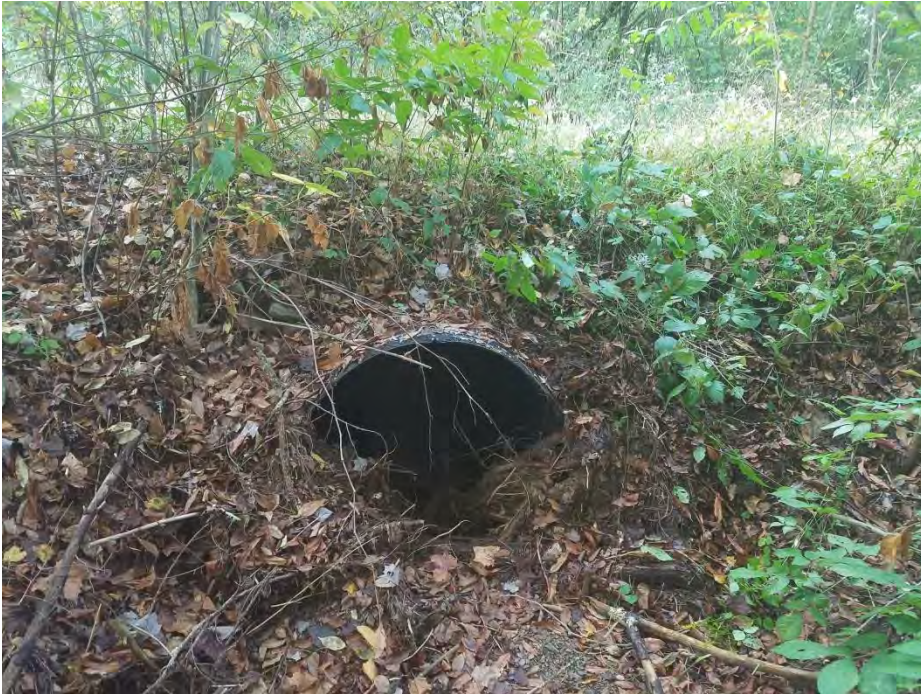
Waterbody sau418 facing south - culvert
