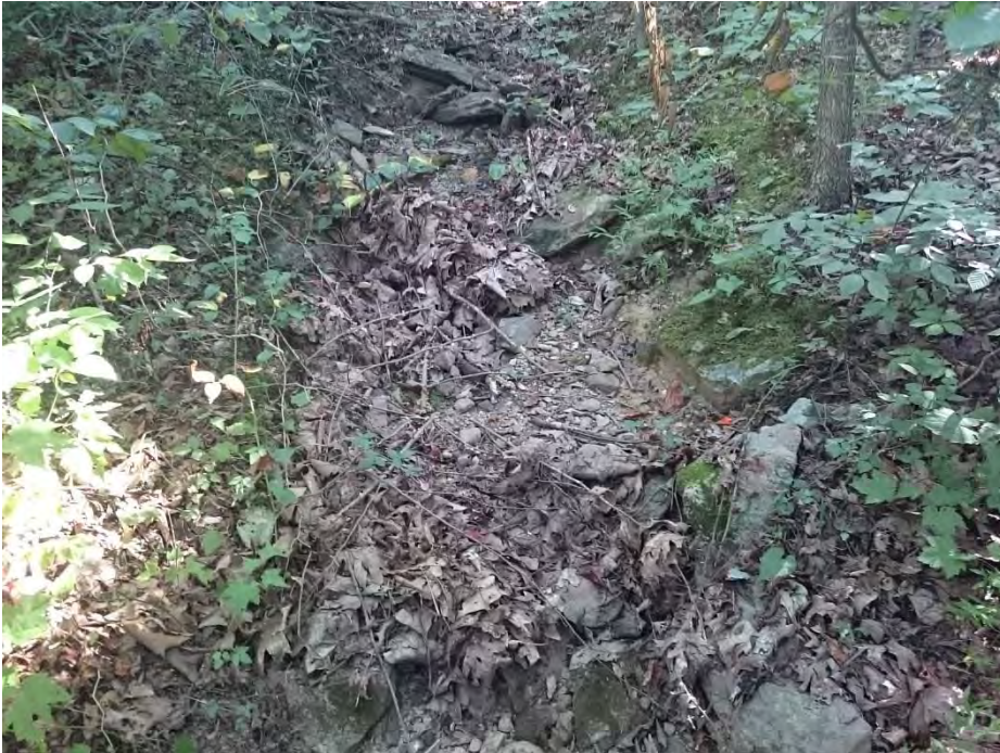
Waterbody SAUA430 facing east upstream
