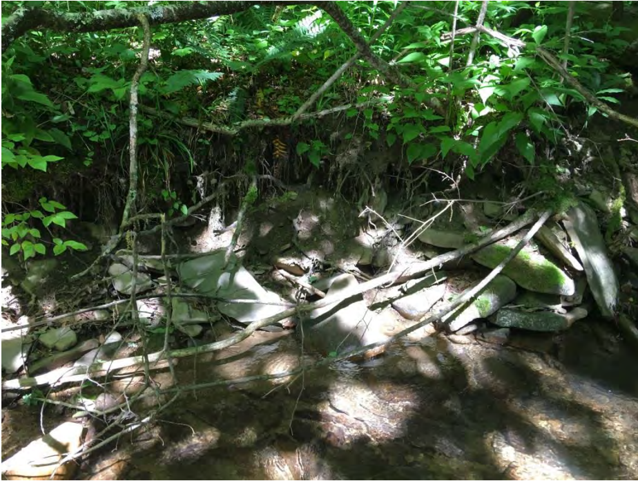
Waterbody SHIA411 scouring facing west across
