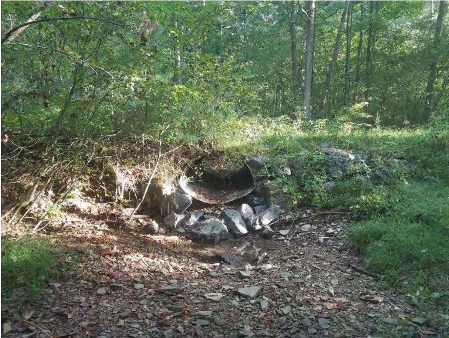
Waterbody sau416 facing north upstream - culvert
