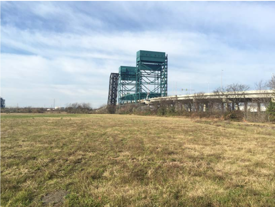
Non-water point nochp001 facing west. (stormwater pond, not present)
