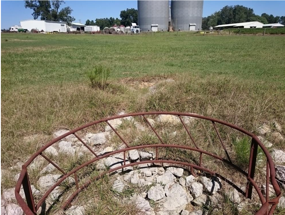
Non-water data point nosoa070 facing northeast
