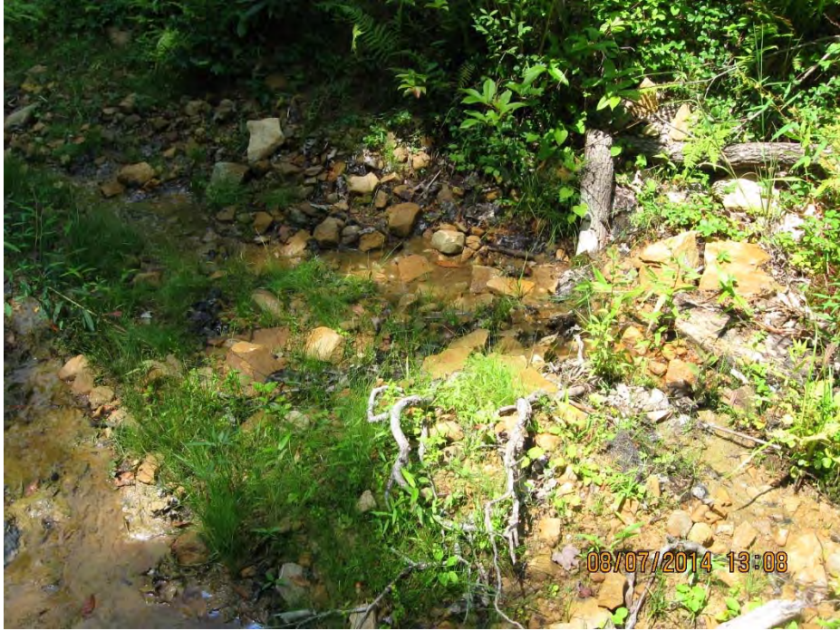
Seep point PUPB102 facing west
