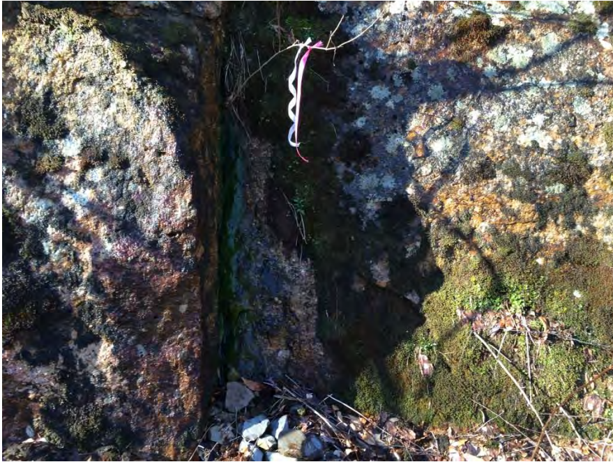
Seep data point PRAA443 facing west
