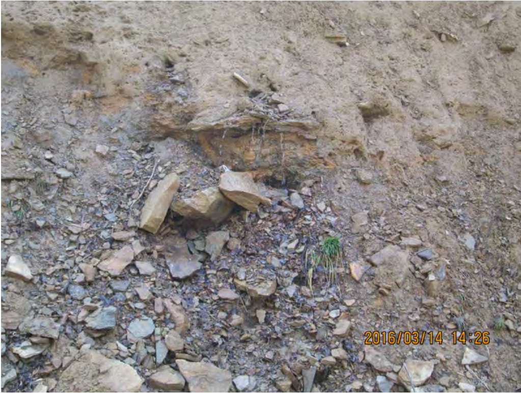
Seep data point prap004 facing south.
