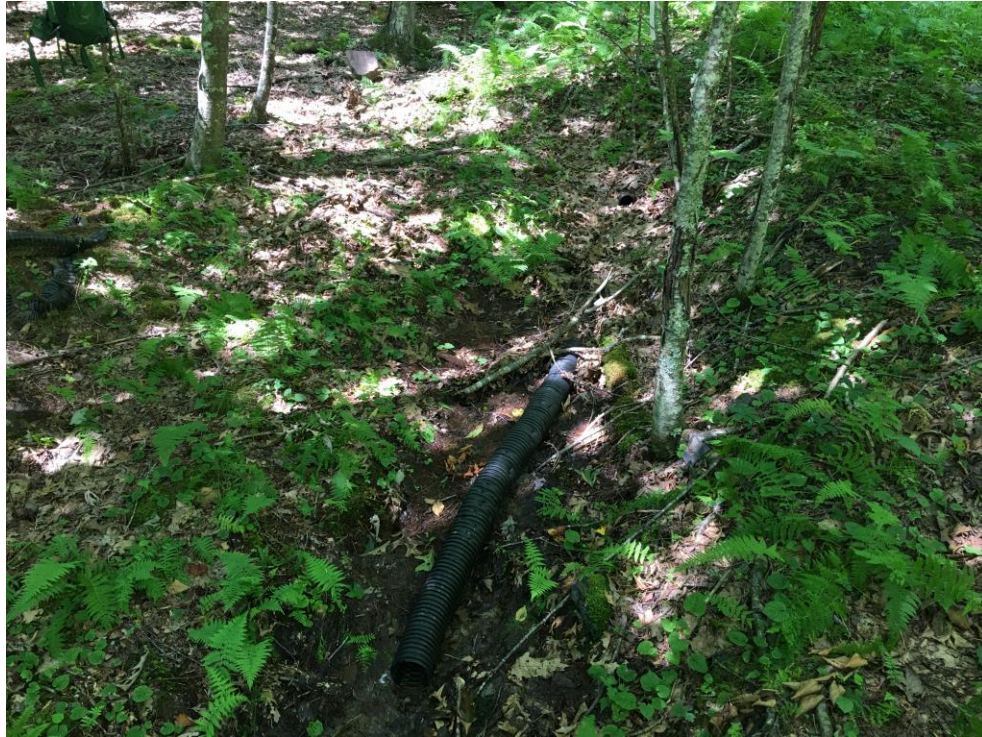
Seep data point PHIA410 facing west
