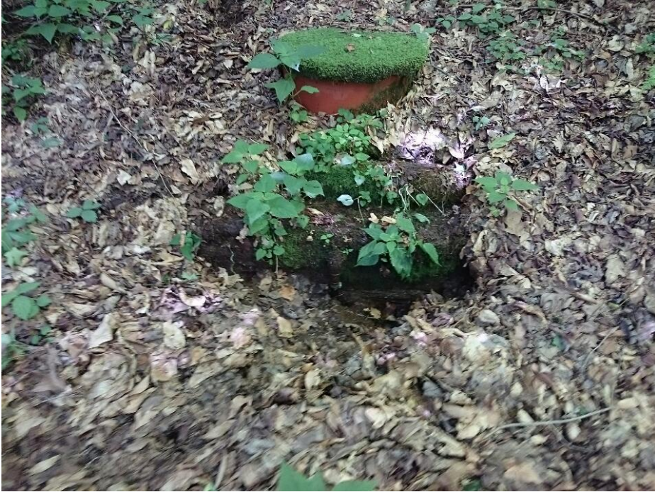
Seep point PPOE016 facing southeast
