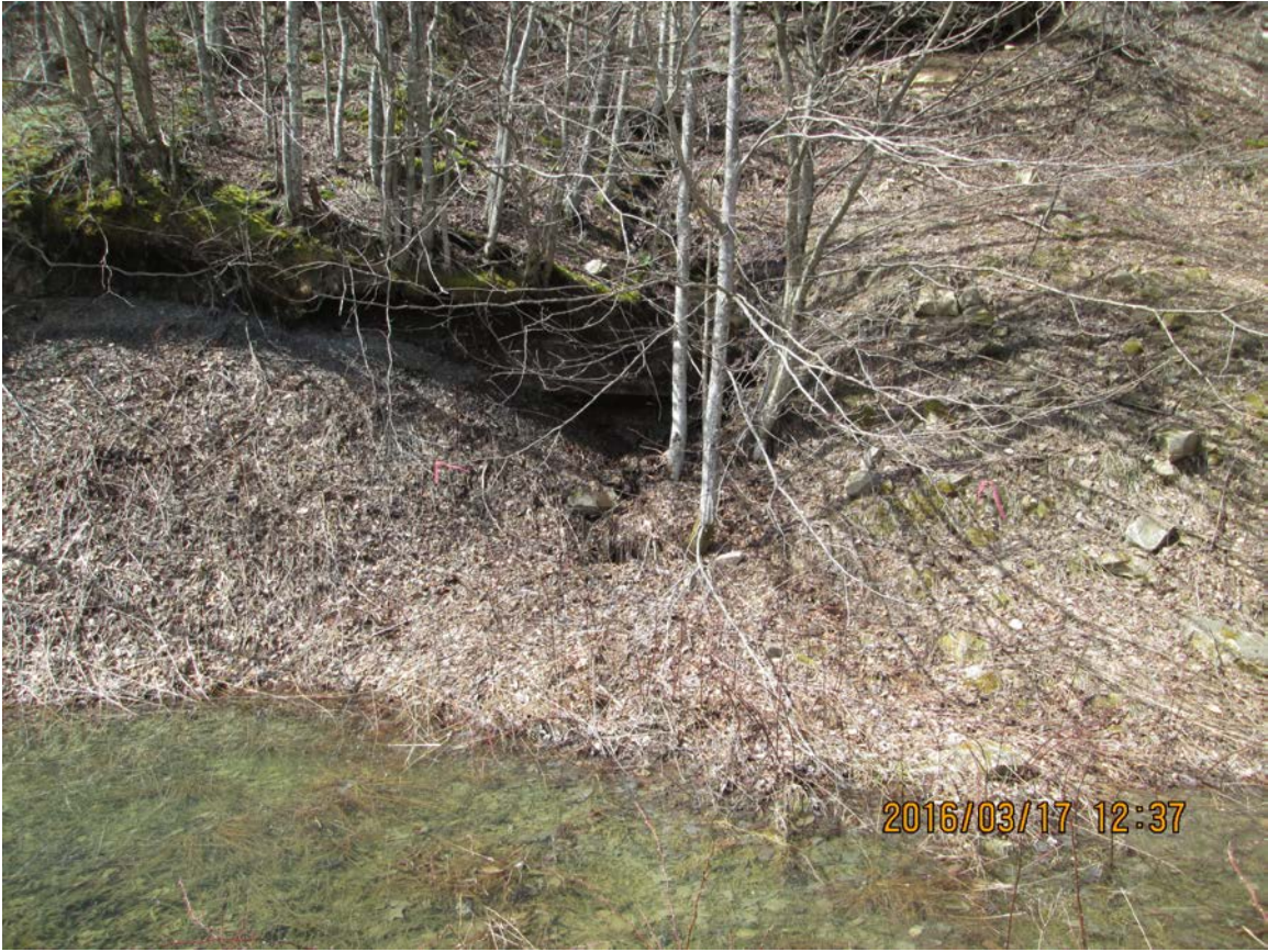
Seep data point prap019 facing west.
