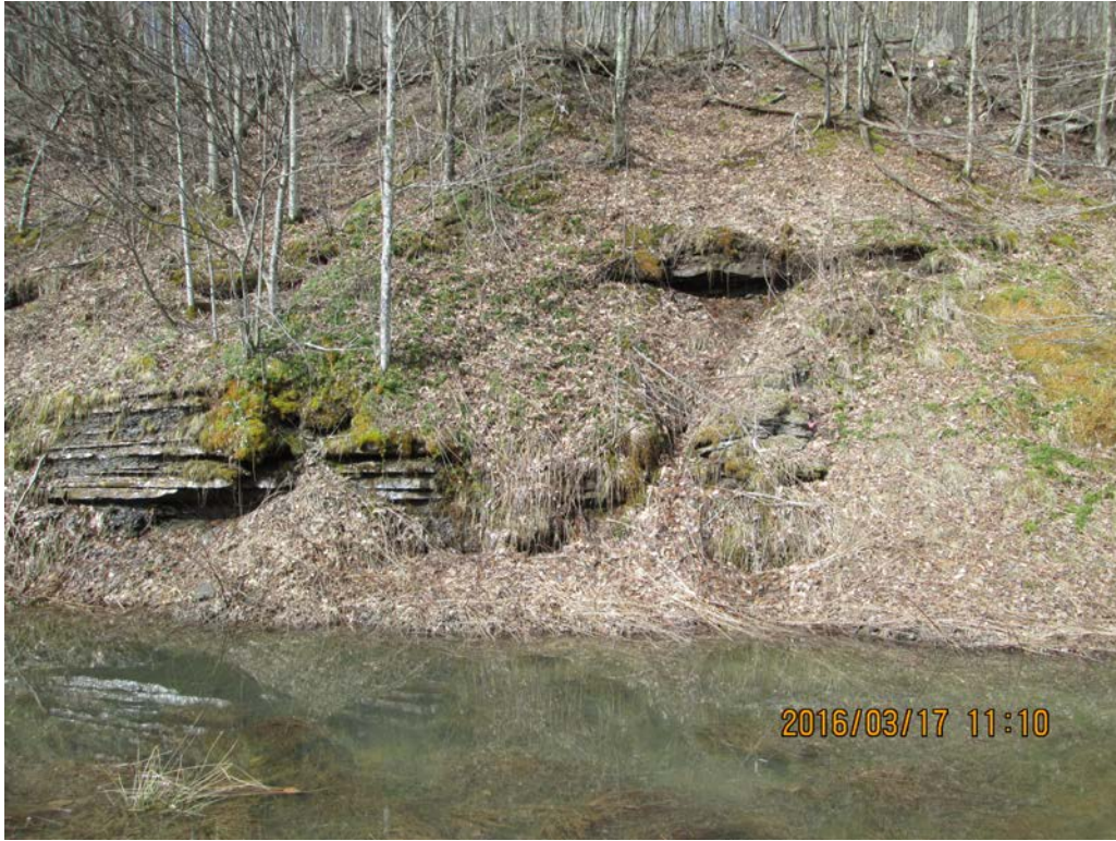
Seep data point prap014 facing west.
