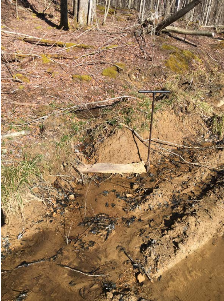
Seep data point prap024 facing northwest.
