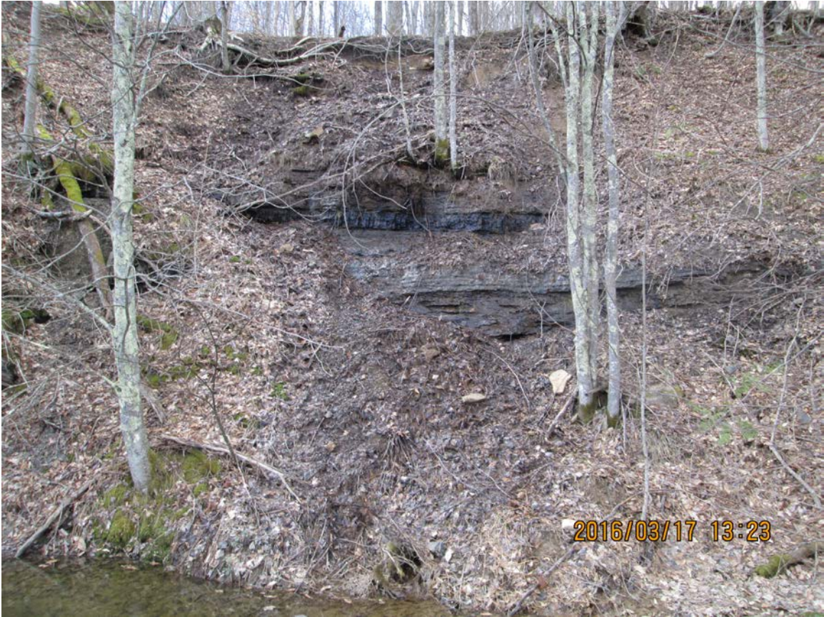
Seep data point prap022 facing west.
