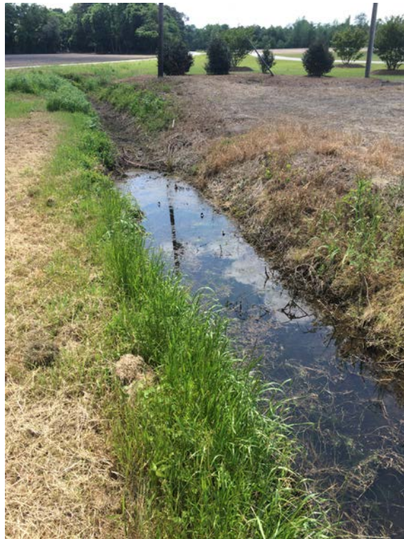
Waterbody ssap001 facing southwest downstream.
