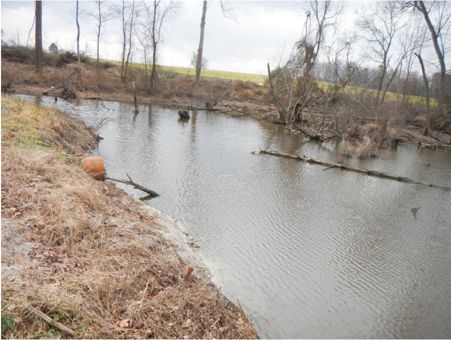
ONAG002 facing west
