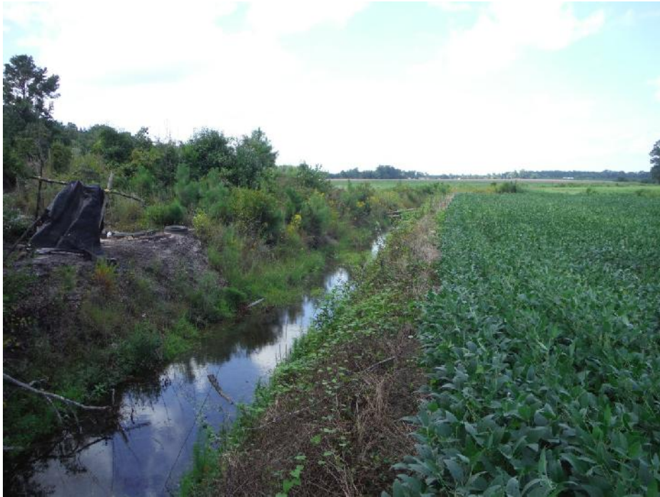
scmg001 facing upstream
