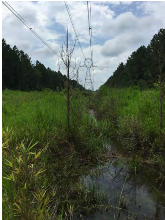
Waterbody data point scm002 facing south downstream.
