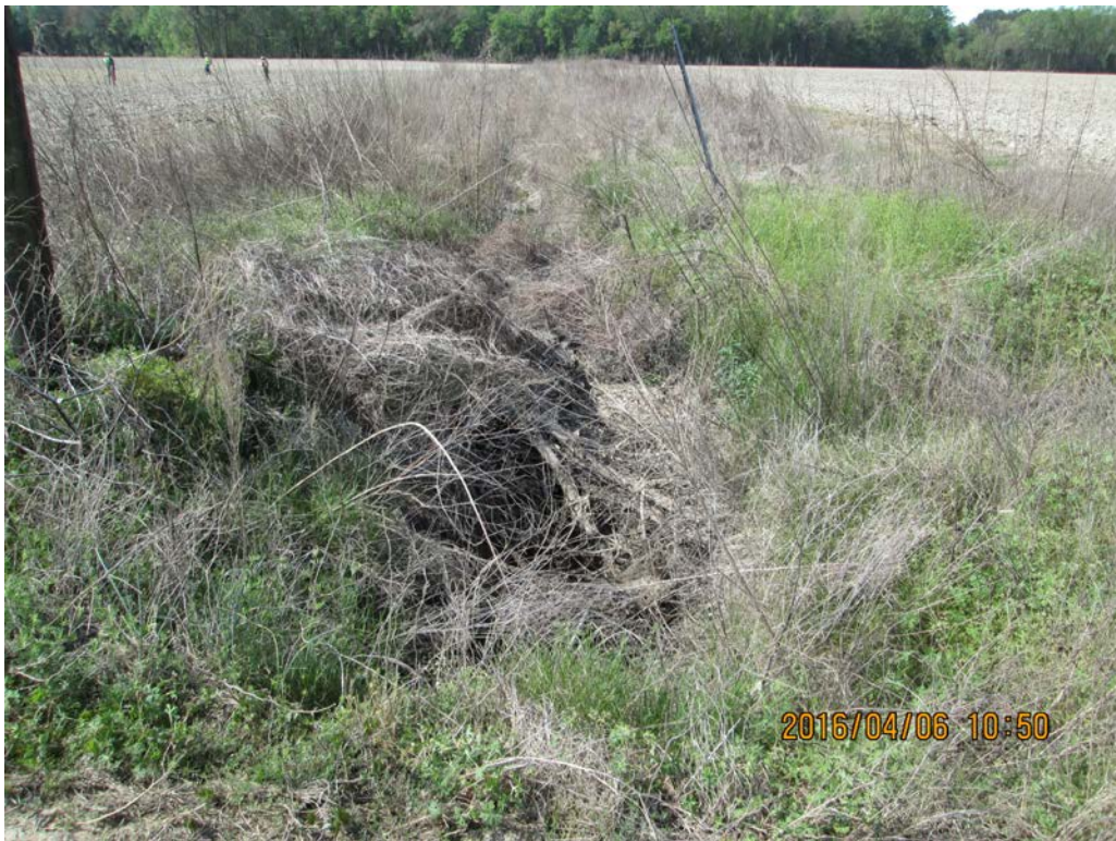
Waterbody scmp100 facing southwest downstream on access road.
