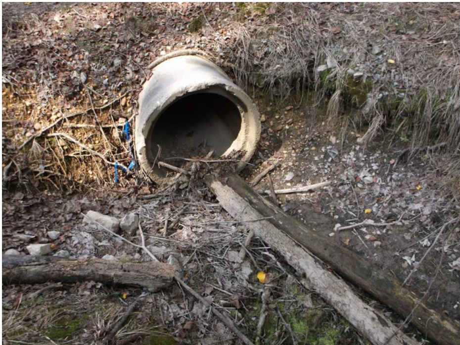
Waterbody scmp021 facing southwest downstream.
