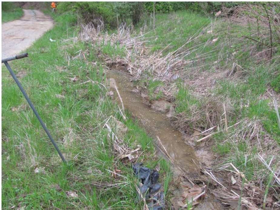
Waterbody swzg015 facing downstream
