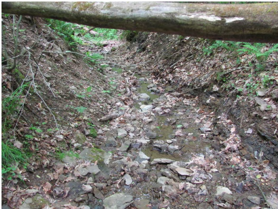
Waterbody swzg028 facing downstream
