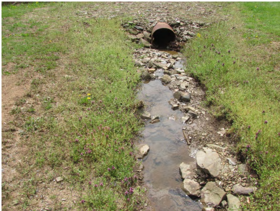
Waterbody swzg020 facing downstream
