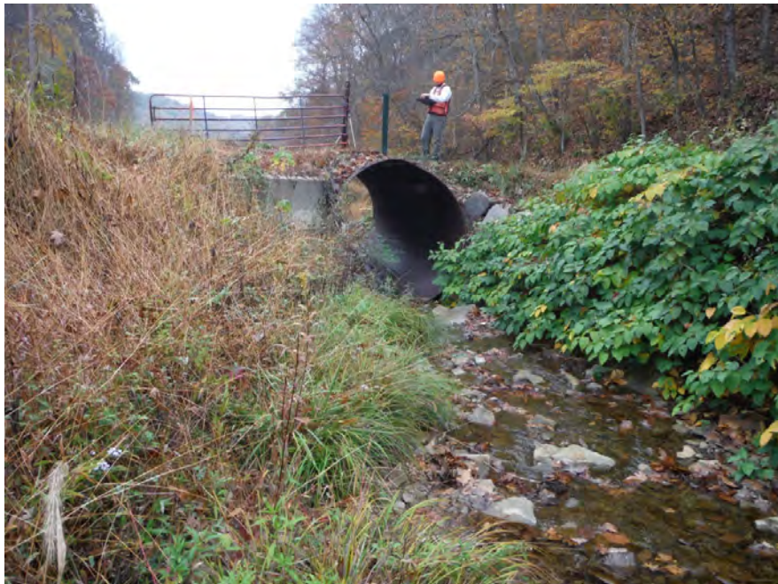
sdoh010 facing downstream
