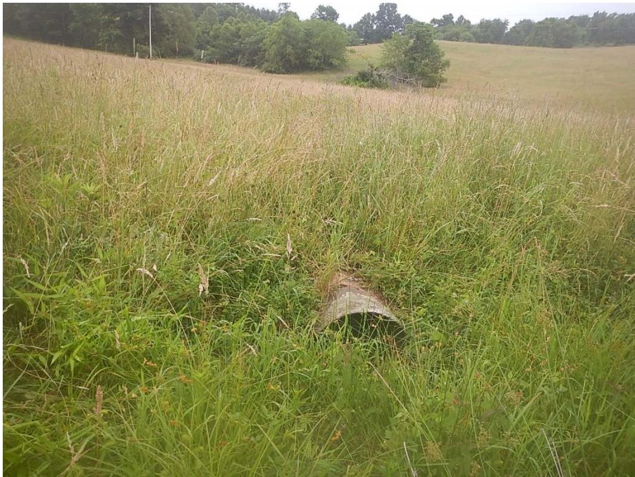
Waterbody SUPA003 facing south downstream
