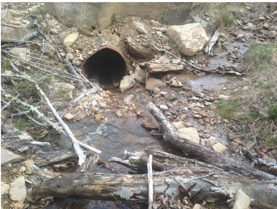
Waterbody SRAC130 facing northeast downstream
