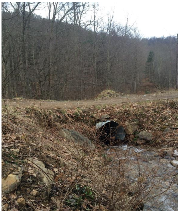
Waterbody SRAA416 facing south downstream
