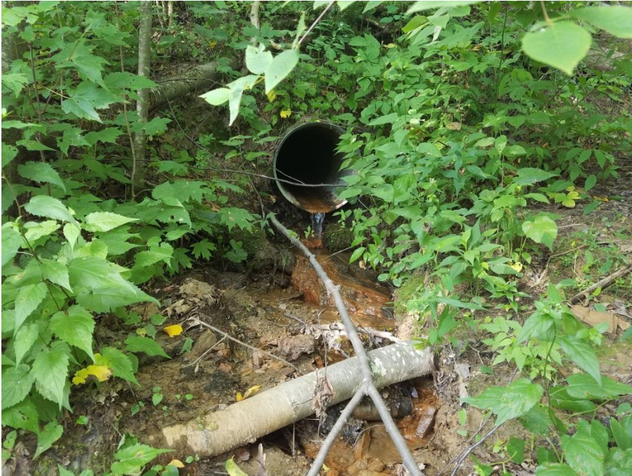
Waterbody srae202 facing southwest upstream
