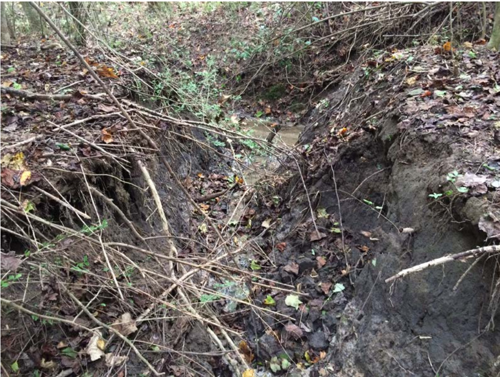
Waterbody ssuo017facing west downstream.
