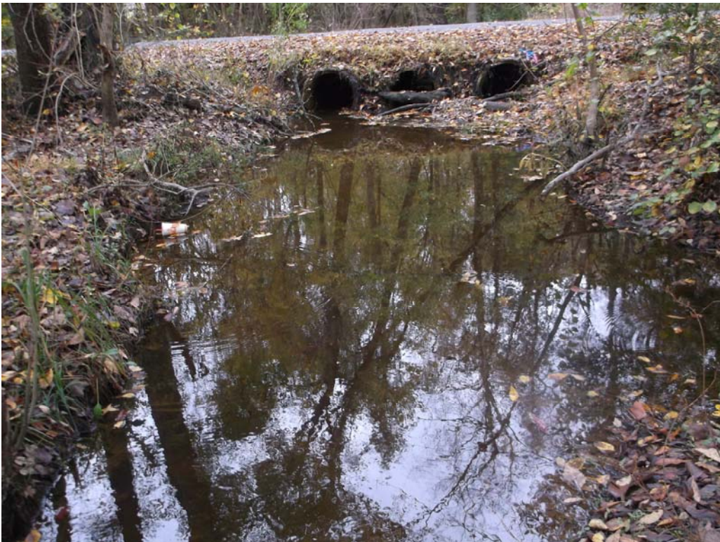
Waterbody ssuo010 facing west downstream.
