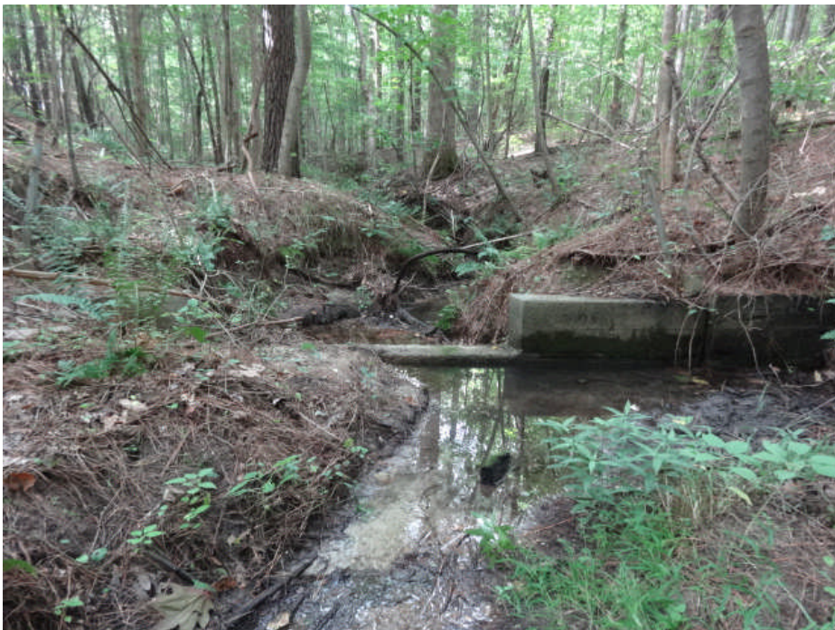
Waterbody point snok026b old dam facing Northwest
