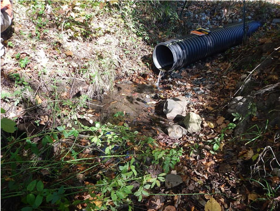
SBUA005 facing northeast upstream
