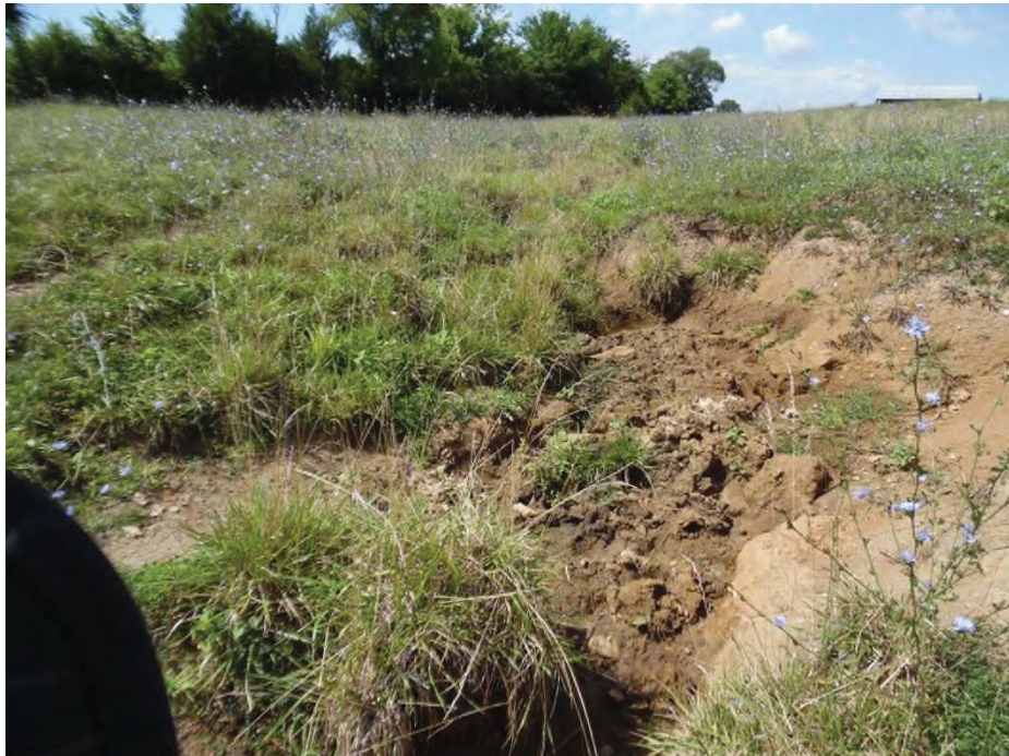
Waterbody point sbuk001 facing southwest and upstream
