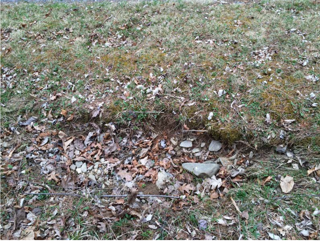
Waterbody data point sbar010_e facing north across bank.
