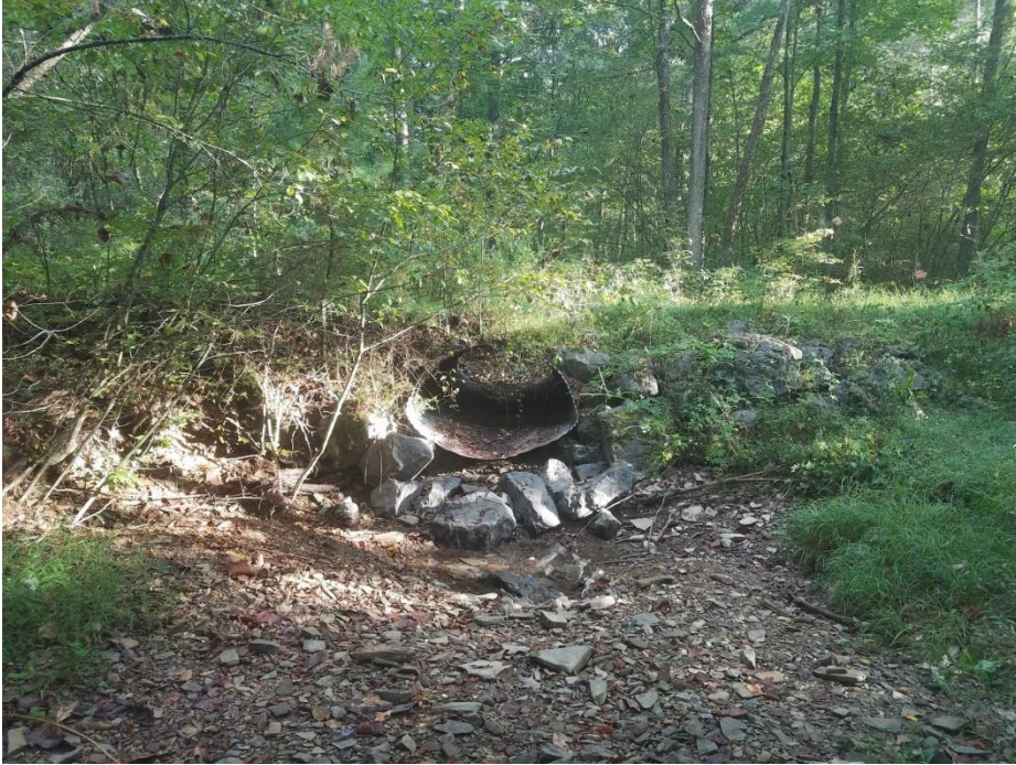
Waterbody sau416 facing north upstream - culvert
