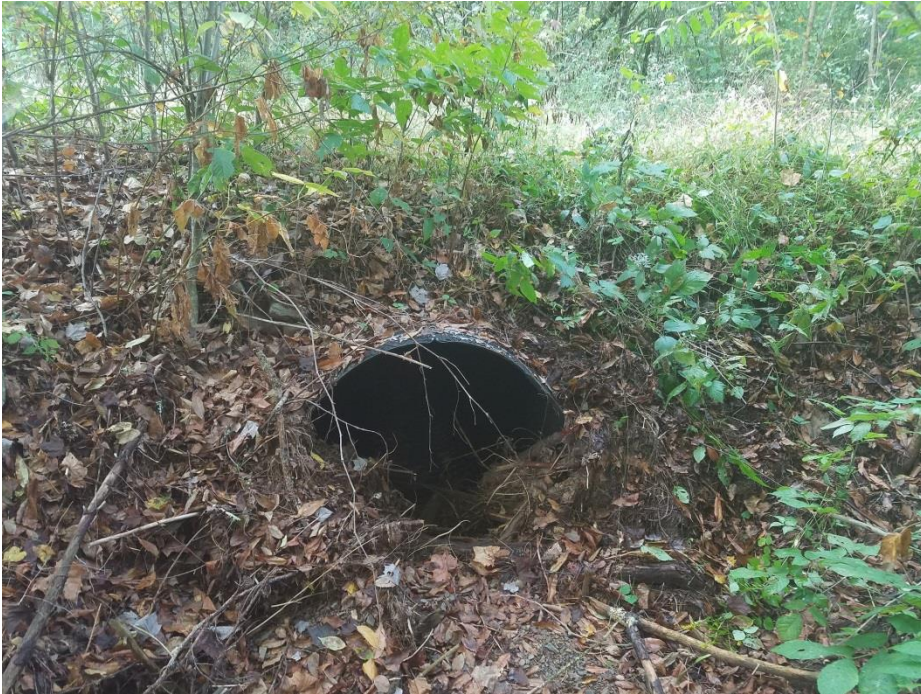
Waterbody sau418 facing south - culvert
