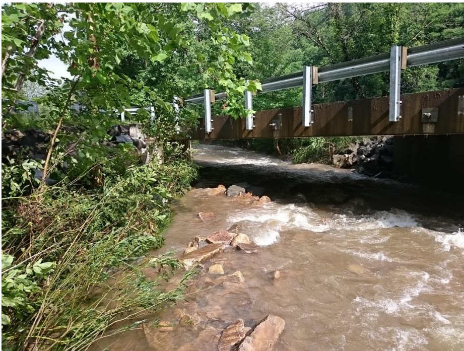
Waterbody SRAE188 facing northwest downstream
