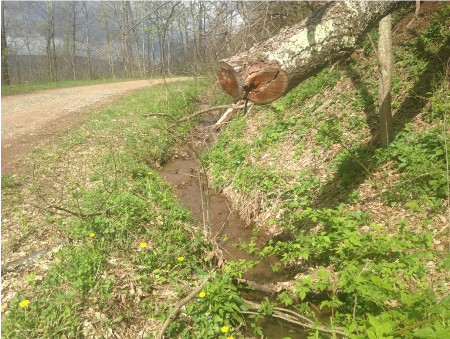
Waterbody SRAC155 facing west upstream
