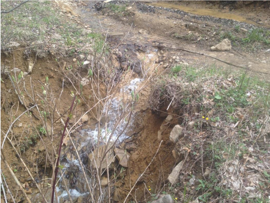
Waterbody SRAC157 facing east upstream
